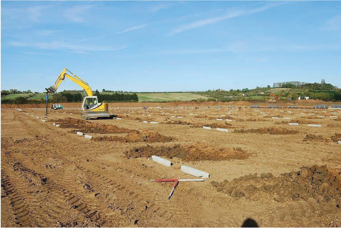
Plate 6 Excavation of the auger holes for the greenhouse, view north-east
