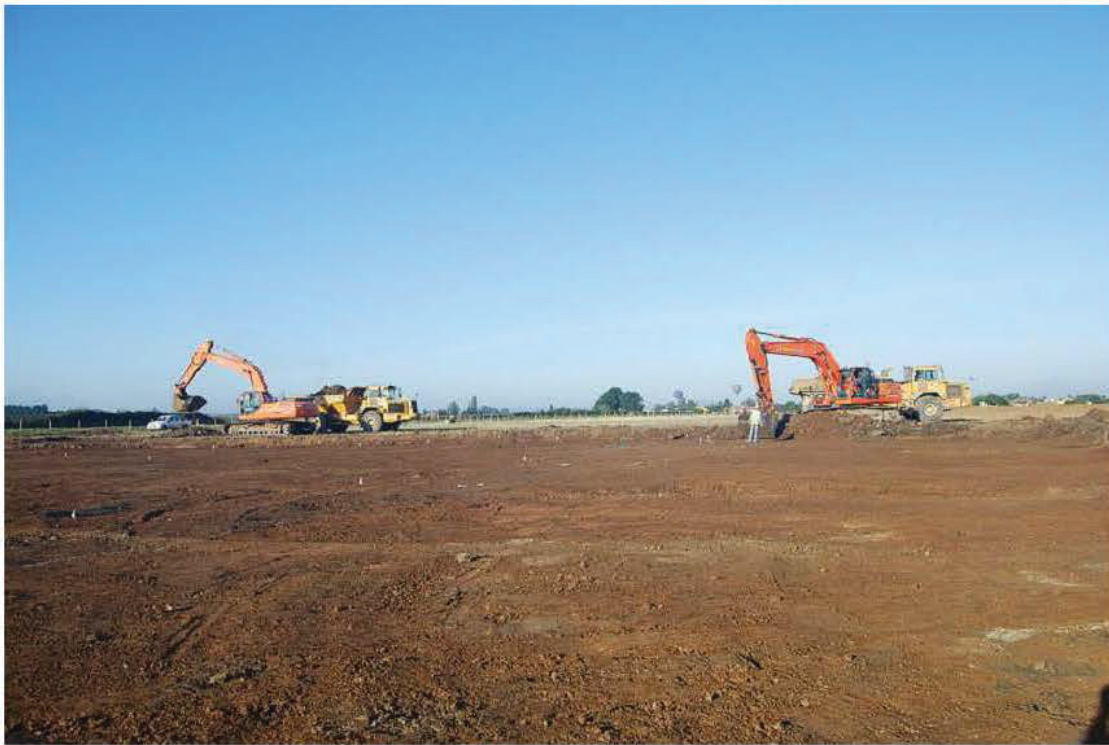
Plate 1 Excavation of Trench 80, the lagoon area, view west
