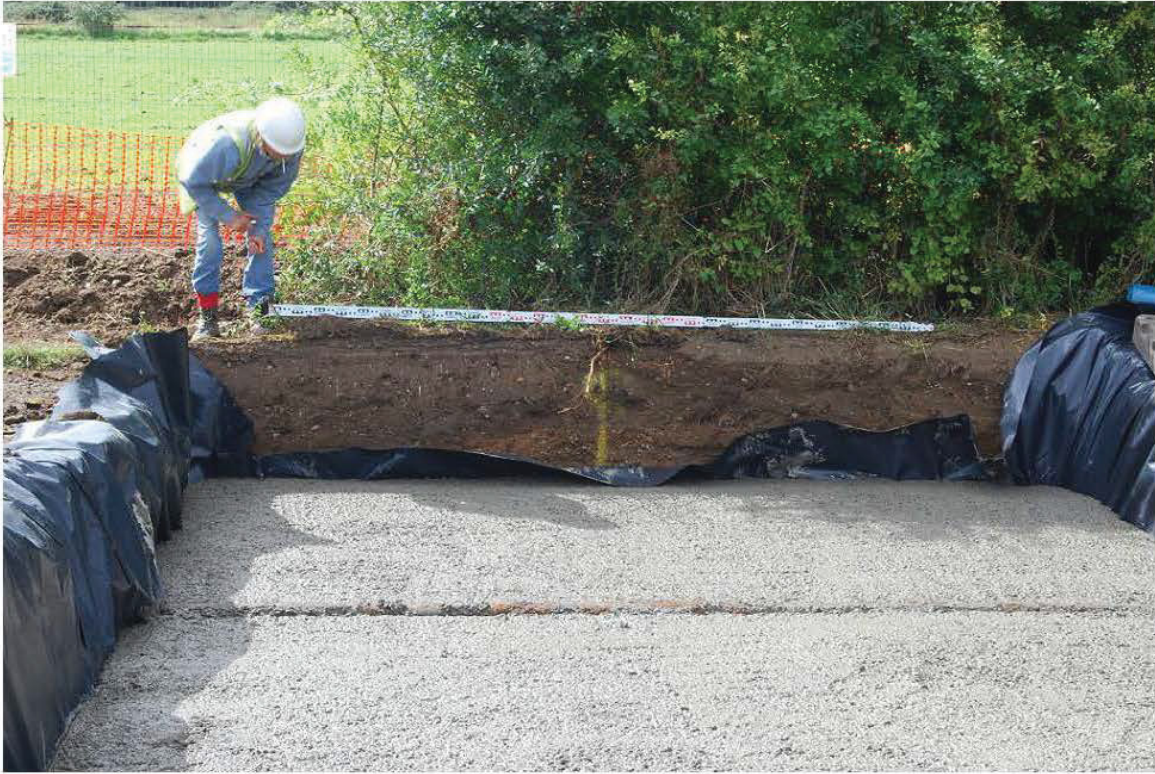
Plate 12 View south of trench for reinforcement over water pipe
