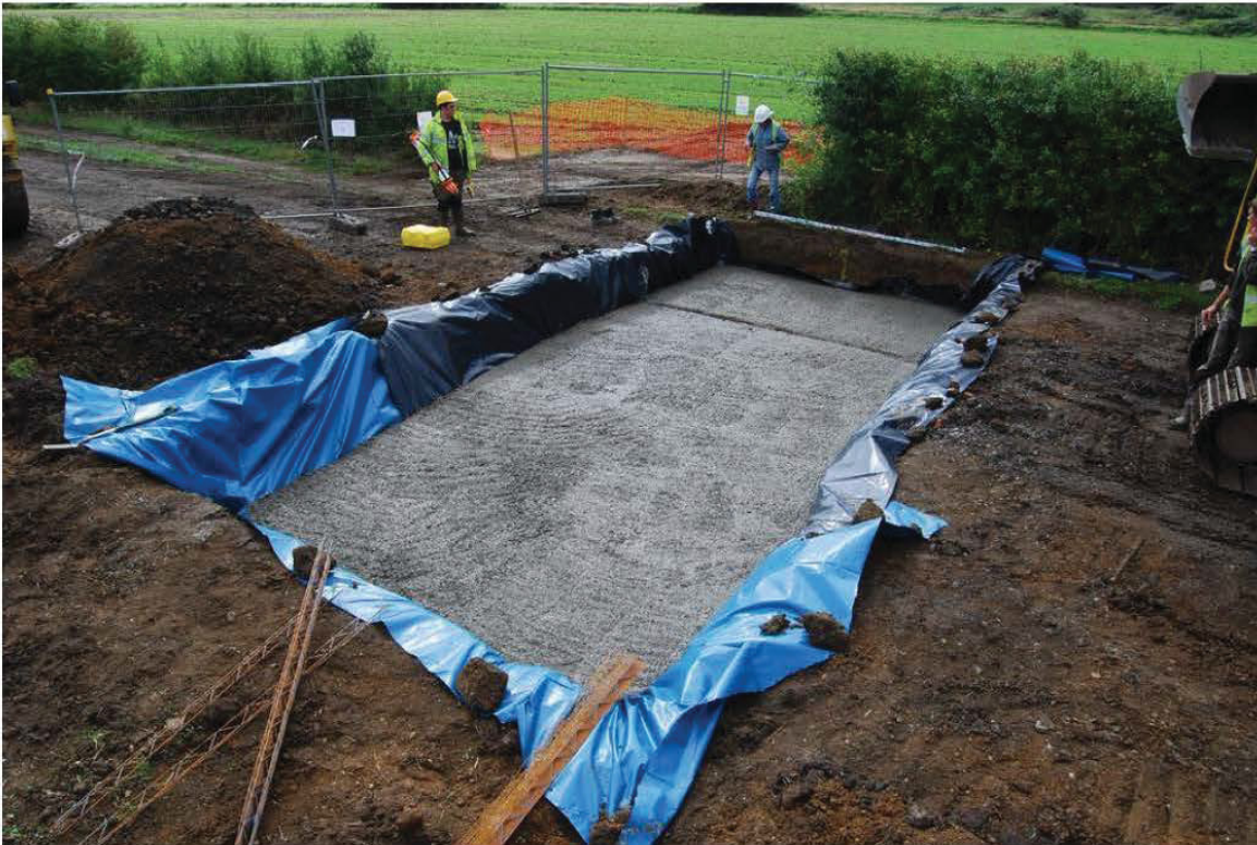
Plate 11 General view south-east of trench for reinforcement over water pipe
