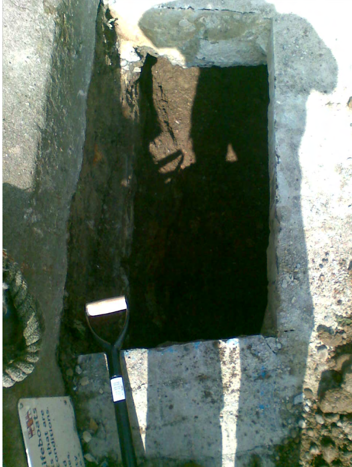
Plate 1. View of area behind wall.
