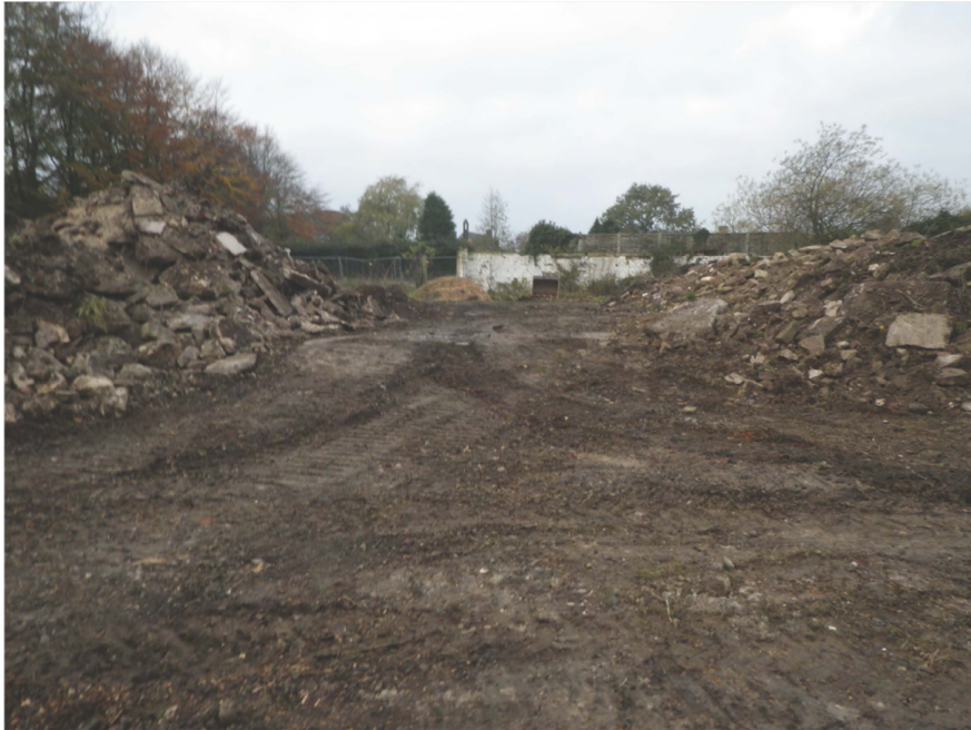
Plate 3. View of Site (Evaluation Trench 3). Facing West.
