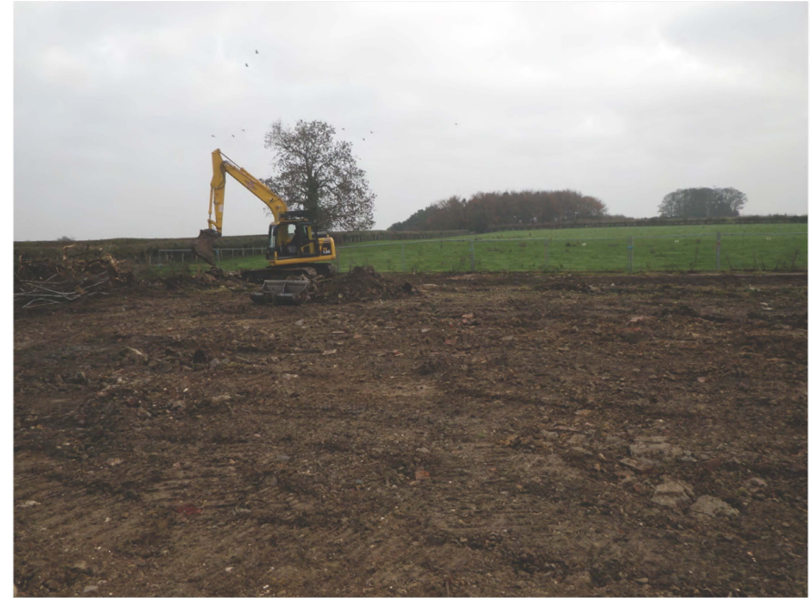
Plate 2. View of Site (Evaluation Trenches 1 and 2). Facing East.
