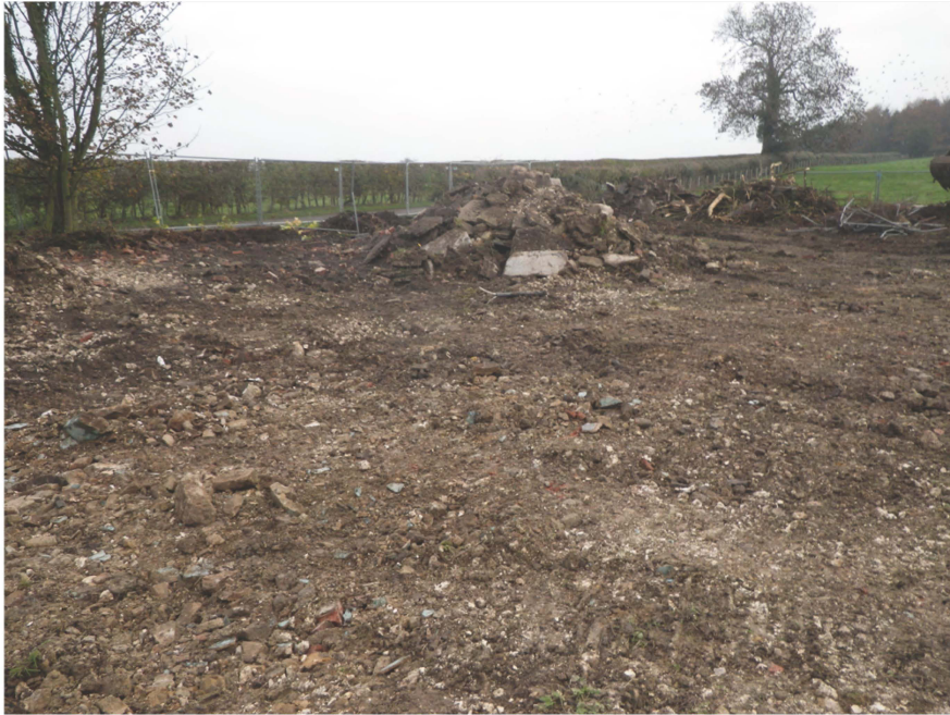
Plate 1. View of Site (Evaluation Trench 1). Facing East.
