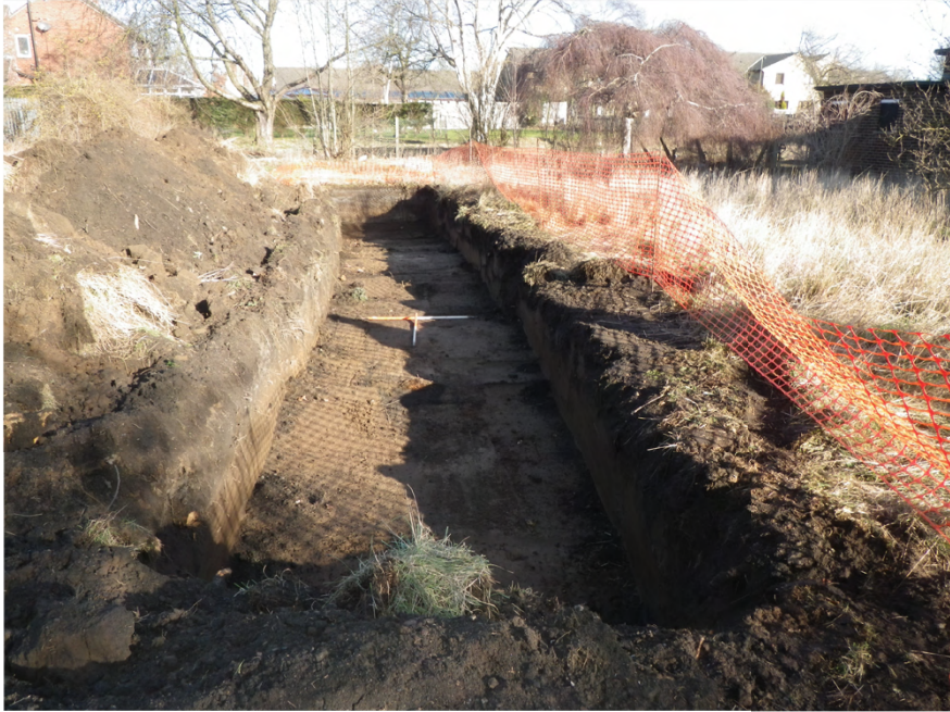
Plate 6. Evaluation Trench 2. Facing North.
