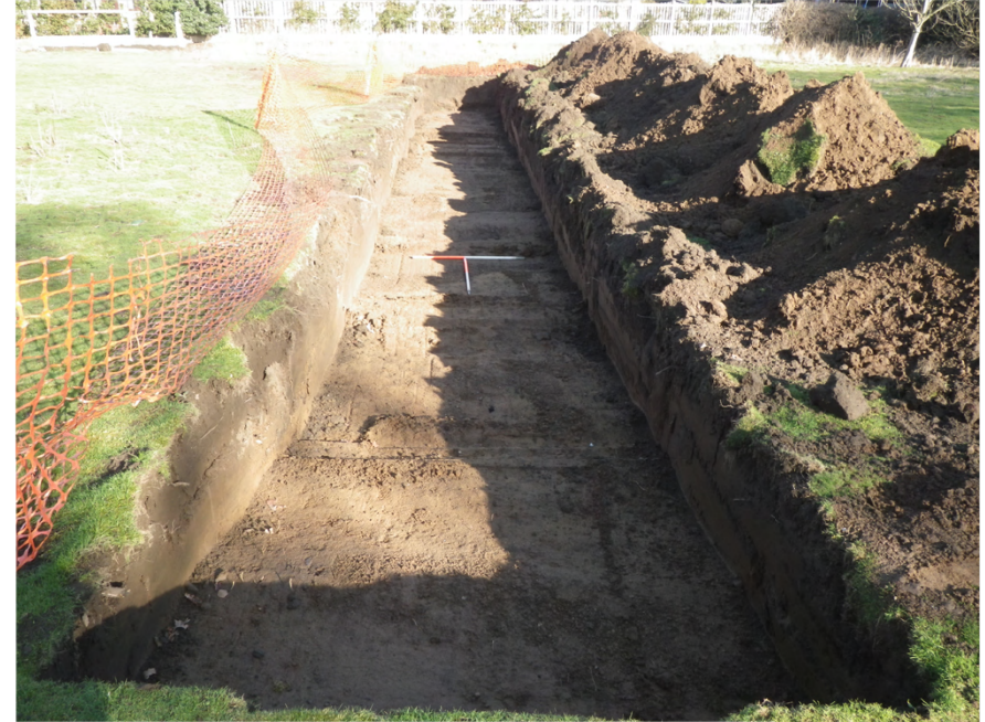
Plate 2. Evaluation Trench 1. Facing North.
