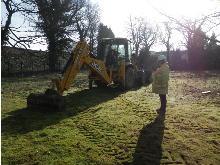
Plate 13. Area of Evaluation Trench 5 before Excavation. Facing South-east.
