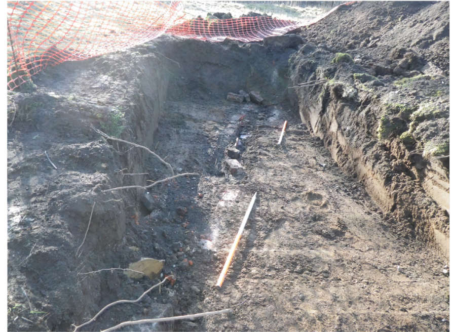
Plate 16. Evaluation Trench 5: Modern Drain 5003. Facing South.
