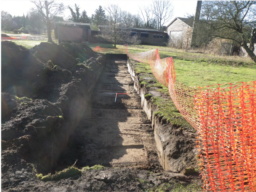
Plate 3. Evaluation Trench 1. Facing South.
