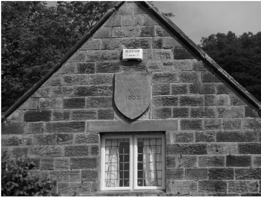
Plate 19. View of Stables. Facing North.
