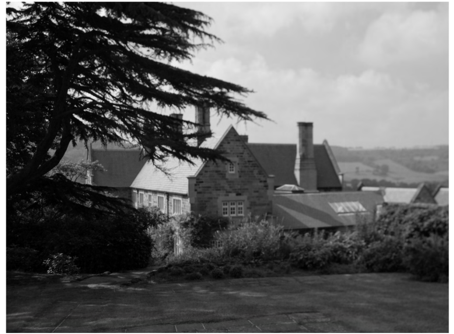
Plate 10. View of Cowesby Hall. Facing South-west.
