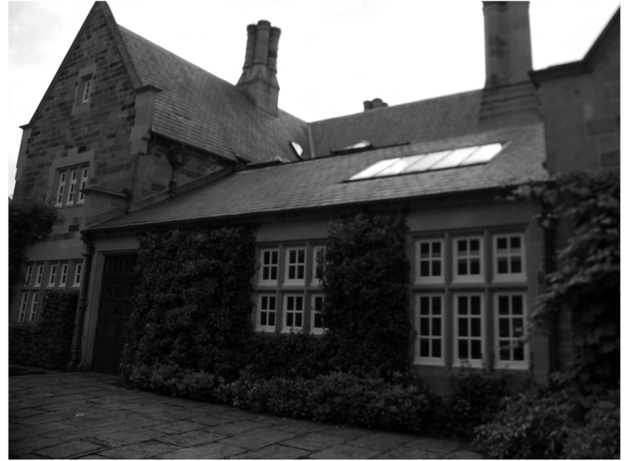
Plate 16. View of Stables. Facing East.
