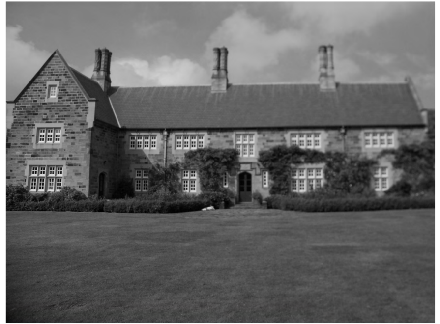
Plate 8. View of Cowesby Hall. Facing West.
