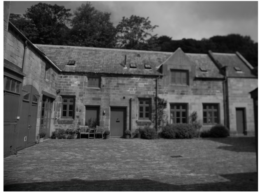
Plate 20. View of Stables. Facing North.
