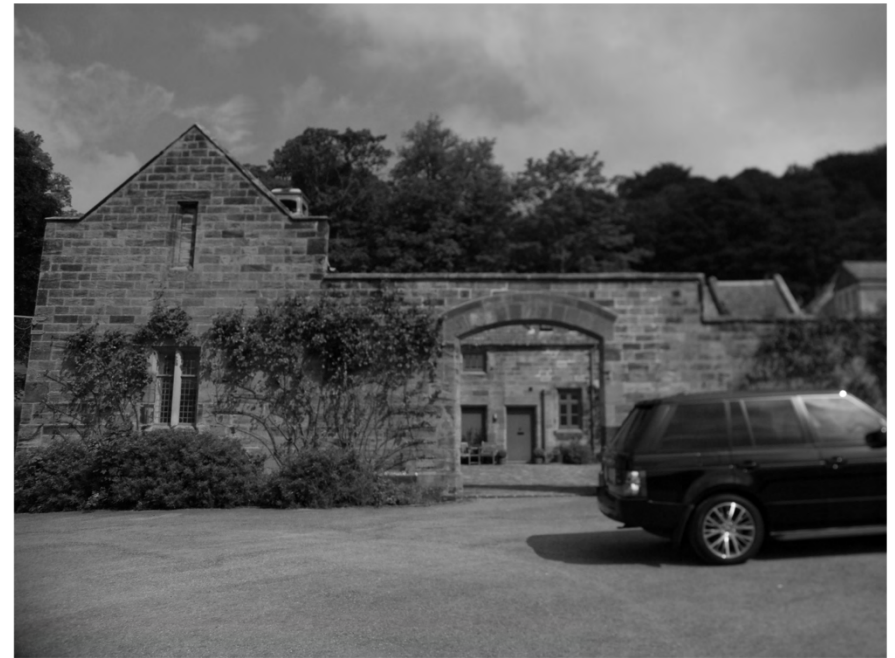
Plate 14. View of Stables. Facing North.
