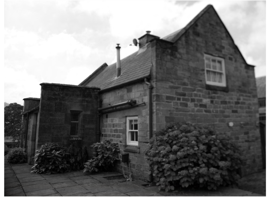
Plate 18. View of Stables. Facing South-west.
