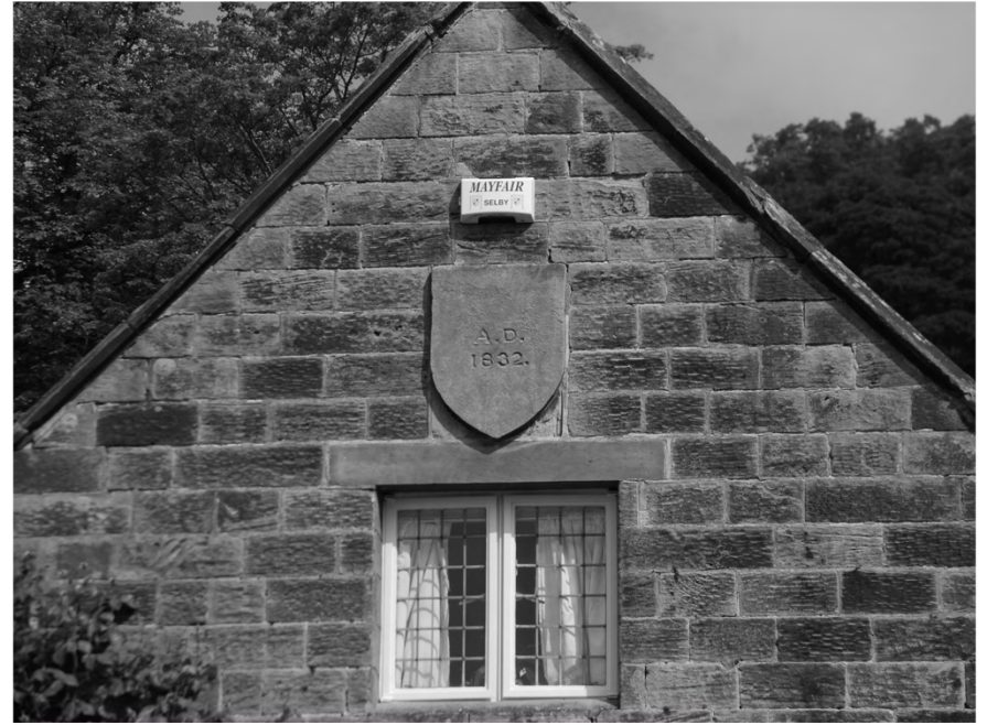
Plate 24. View of Pool House. Facing North.
