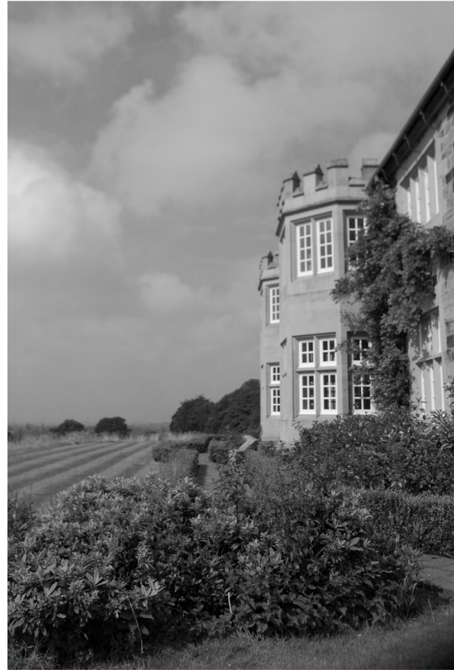
Plate 6. View of Cowesby Hall. Facing West.
