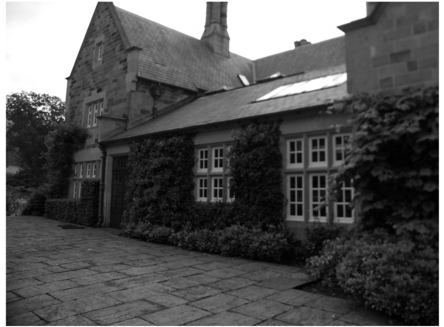
Plate 12. View of Cowesby Hall. Facing South-east.
