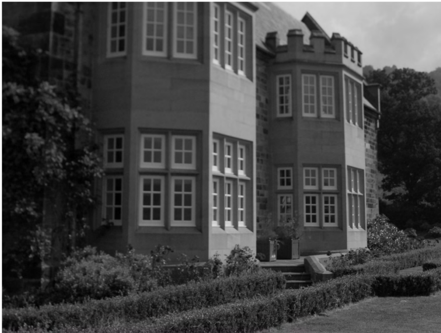
Plate 5. View of Cowesby Hall. Facing East.
