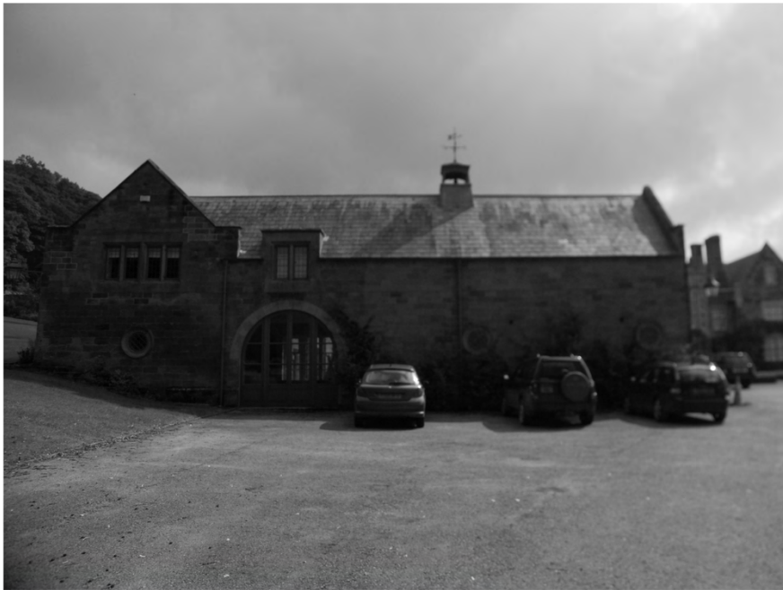
Plate 13. View of Stables. Facing East.
