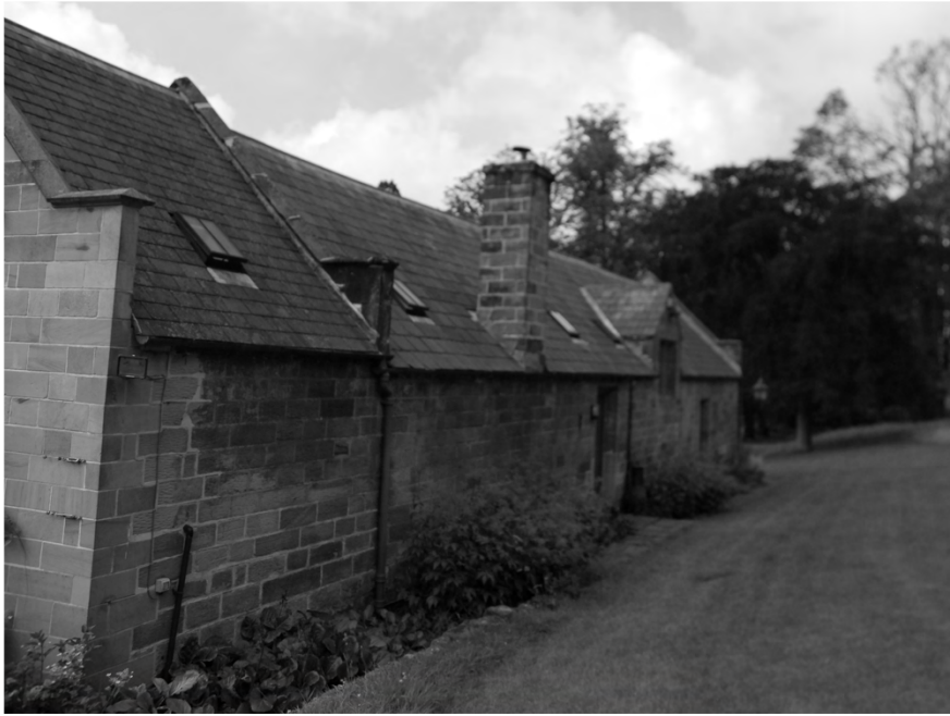
Plate 17. View of Stables. Facing South-west.
