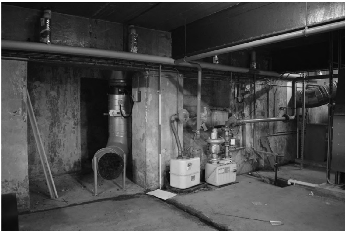
Plate 34. Gymnasium Interior – Basement. Facing South.
