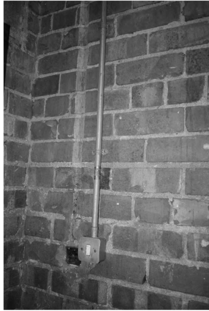
Plate 70. Gymnasium Interior – Ground Floor. Facing East.
