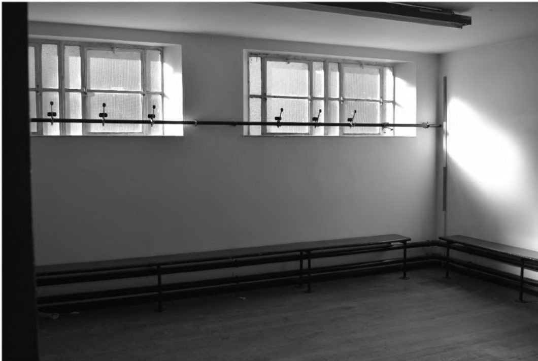
Plate 54. Gymnasium Interior – Ground Floor. Facing West.
