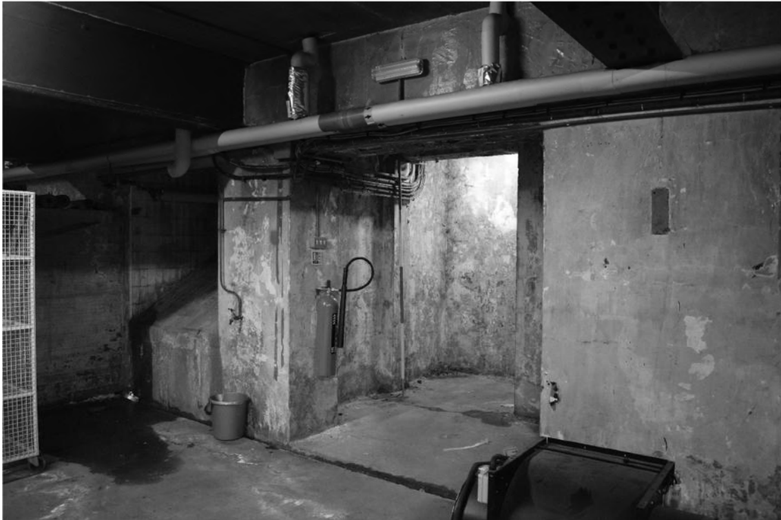
Plate 32. Gymnasium Interior – Basement. Facing South-east.
