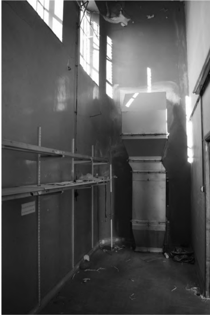
Plate 51. Gymnasium Interior – Ground Floor. Facing North-west.
