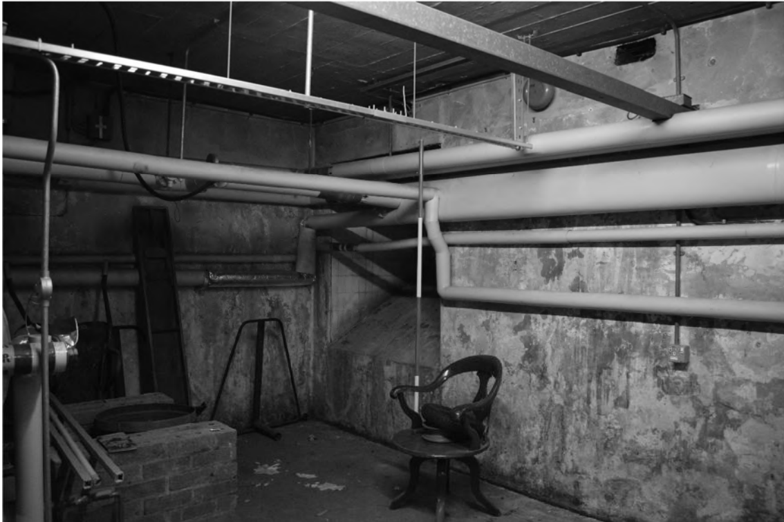
Plate 29. Gymnasium Interior – Basement. Facing North-west.
