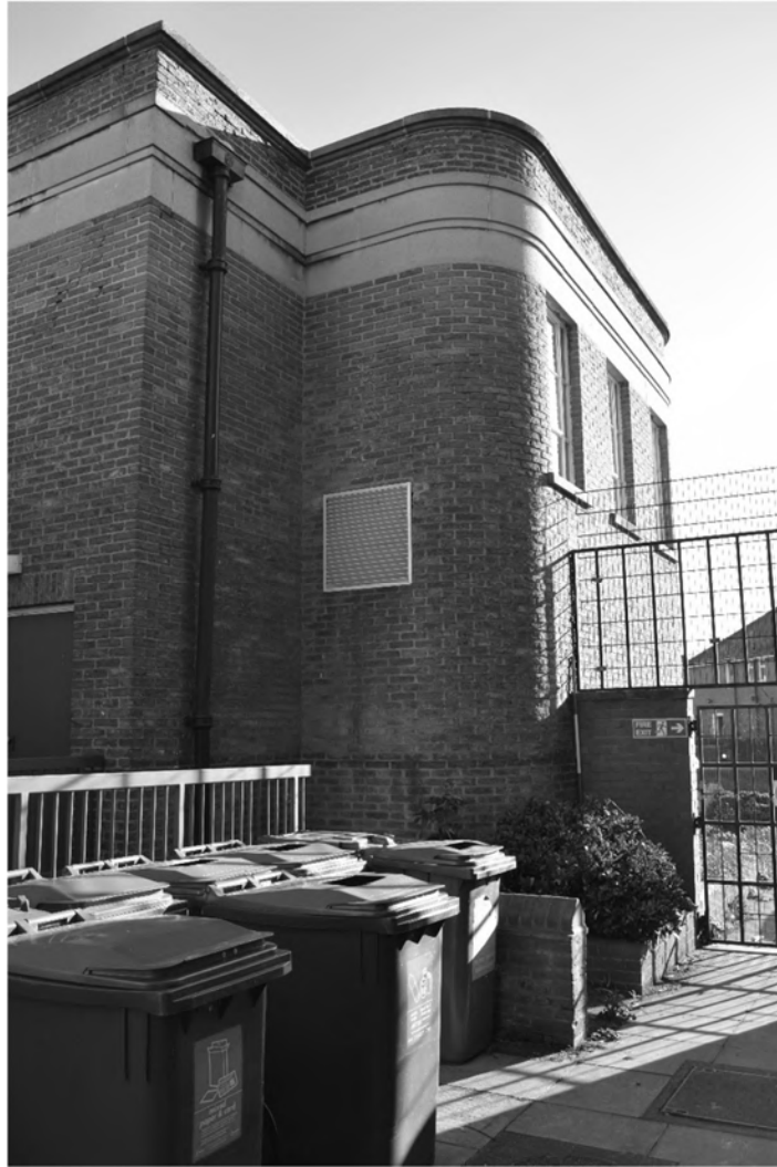
Plate 11. Gymnasium Exterior – South-west Elevation. Facing North-east.
