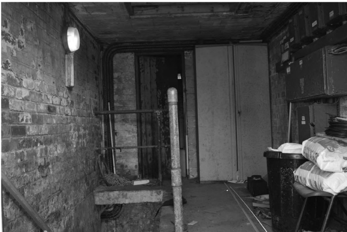
Plate 22. Gymnasium Interior: Boiler House Ground Floor. Facing North-east.
