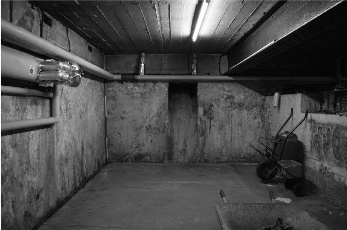
Plate 28. Gymnasium Interior – Basement. Facing South-east.
