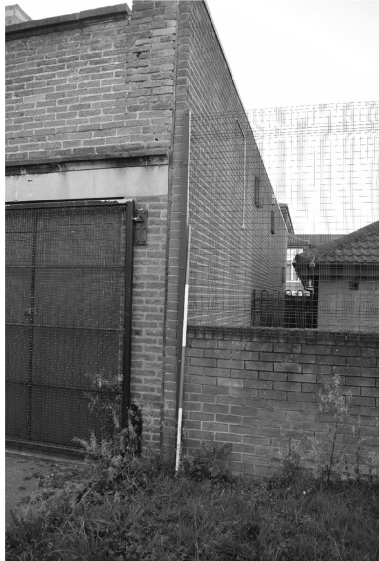
Plate 20. Gymnasium Exterior – North-west Elevation. Facing South.
