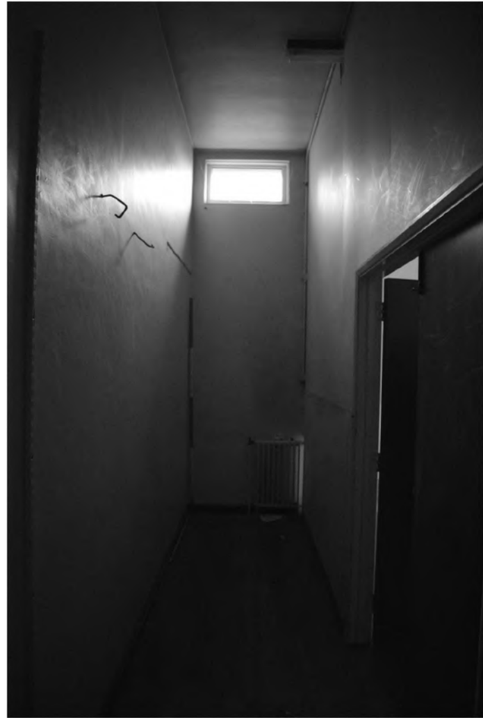
Plate 64. Gymnasium Interior – Ground Floor. Facing South-west.
