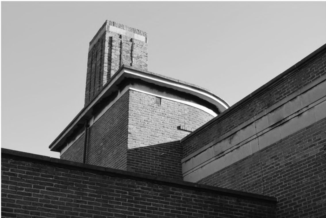
Plate 14. Gymnasium Exterior – Roof Structure & Chimney. Facing North-east.
