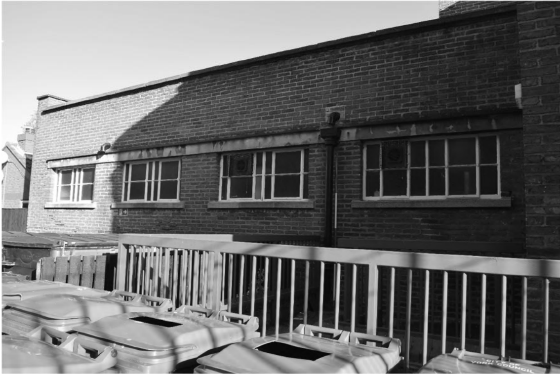
Plate 13. Gymnasium Exterior – South-west Elevation. Facing North.
