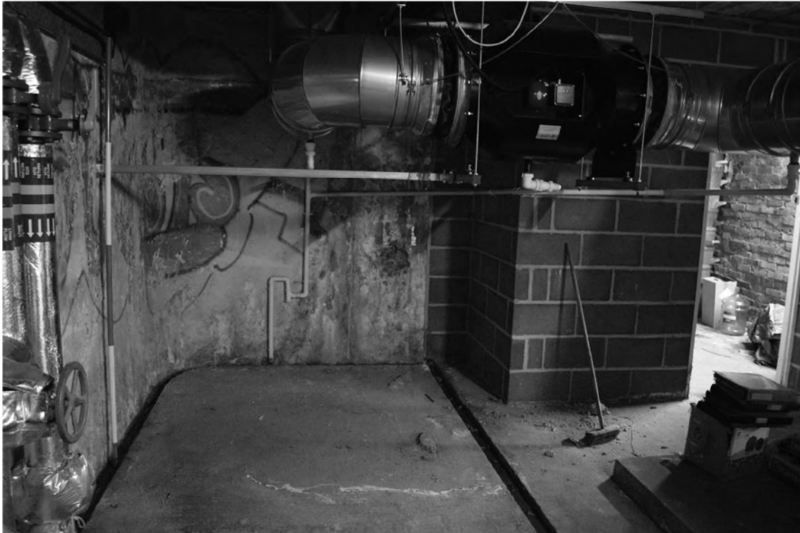
Plate 41. Gymnasium Interior – Basement. Facing North-west.
