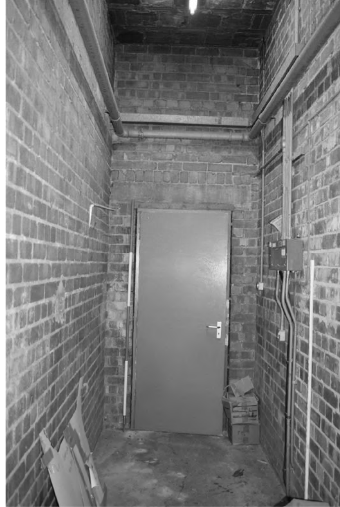
Plate 68. Gymnasium Interior – Ground Floor. Facing North-east.
