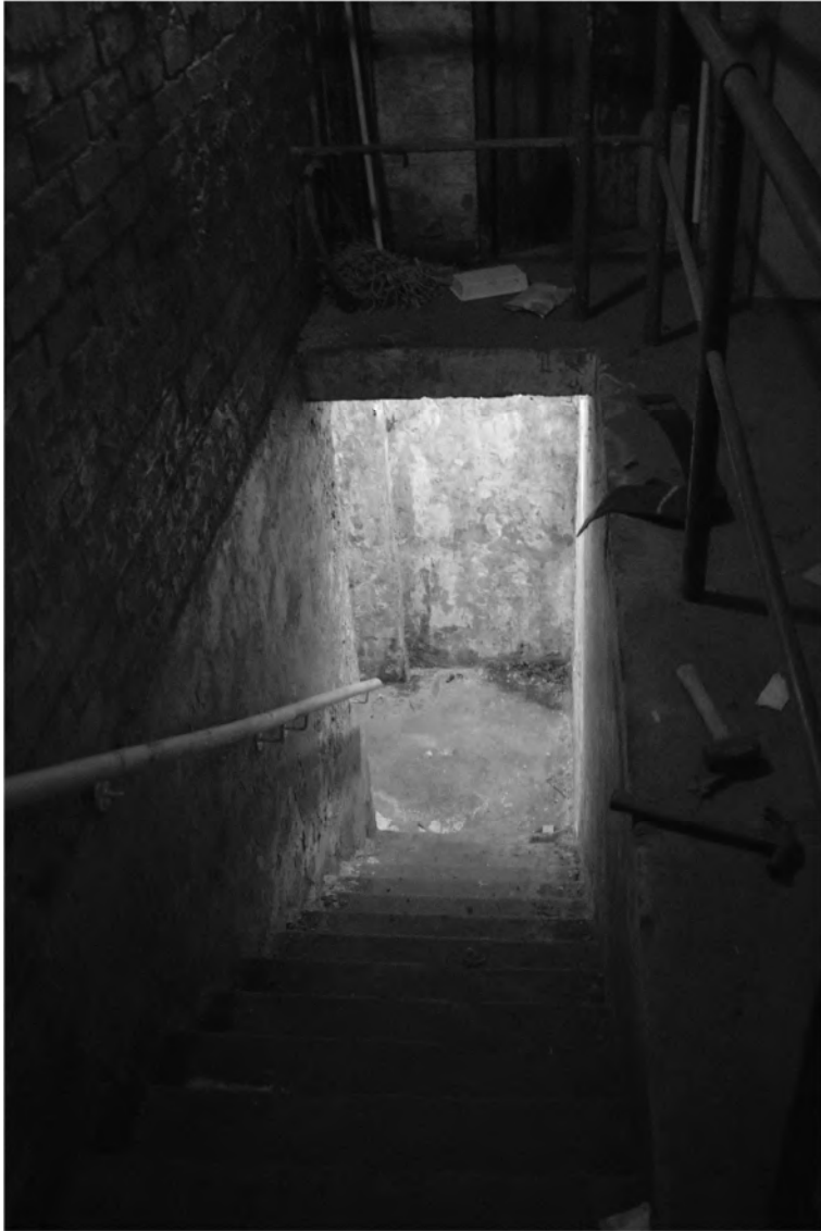
Plate 23. Gymnasium Interior – Basement. Facing North-east.
