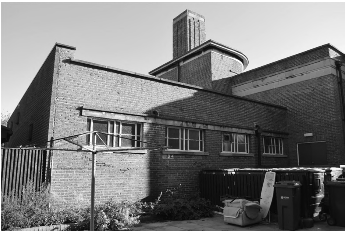
Plate 10. Gymnasium Exterior – South-west Elevation. Facing North-east.
