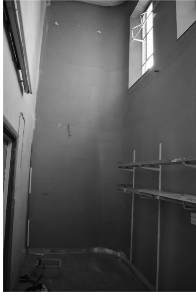
Plate 50. Gymnasium Interior – Ground Floor. Facing South-east.
