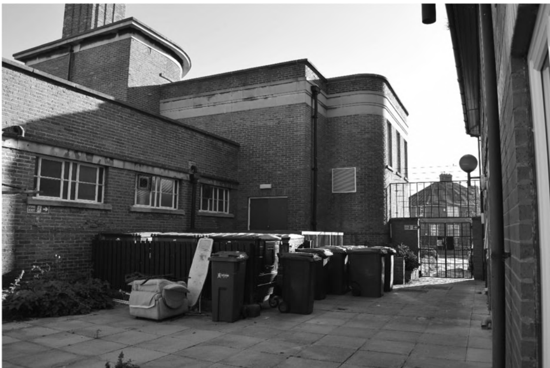
Plate 12. Gymnasium Exterior – South-west Elevation. Facing North-east.
