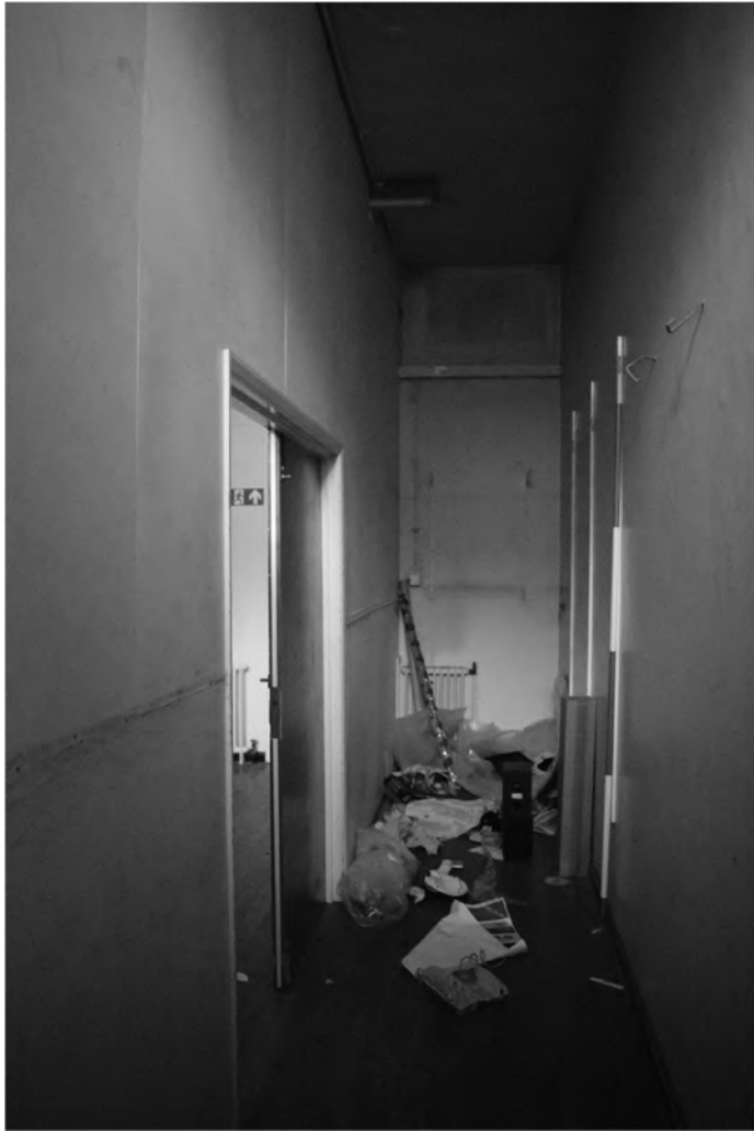
Plate 63. Gymnasium Interior – Ground Floor. Facing North-east.
