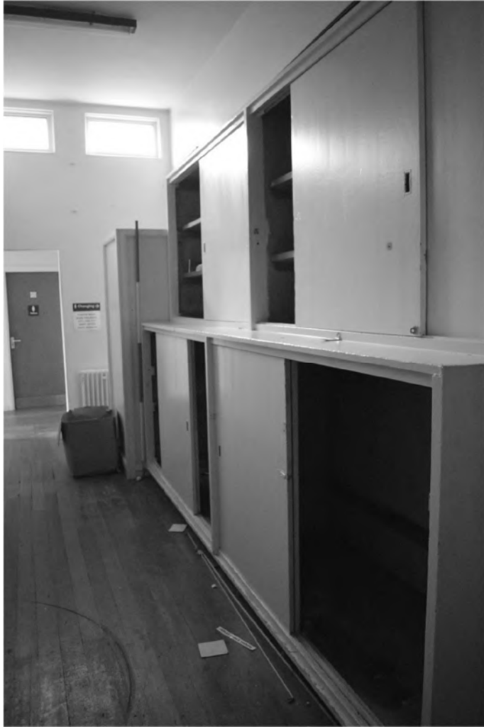
Plate 61. Gymnasium Interior – Ground Floor. Facing South-west.
