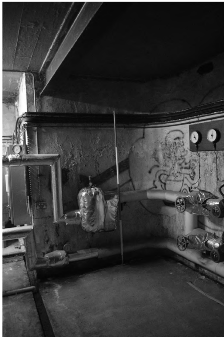
Plate 40. Gymnasium Interior – Basement. Facing South.
