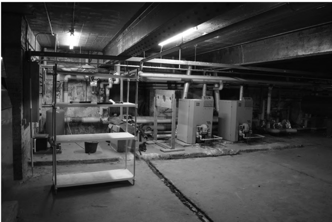
Plate 36. Gymnasium Interior – Basement. Facing North-west.
