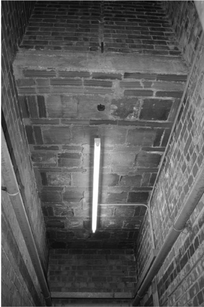
Plate 69. Gymnasium Interior – Ground Floor. Facing North-east.
