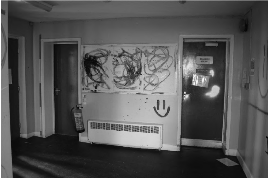
Plate 71. Gymnasium Interior – Ground Floor. Facing South-west.
