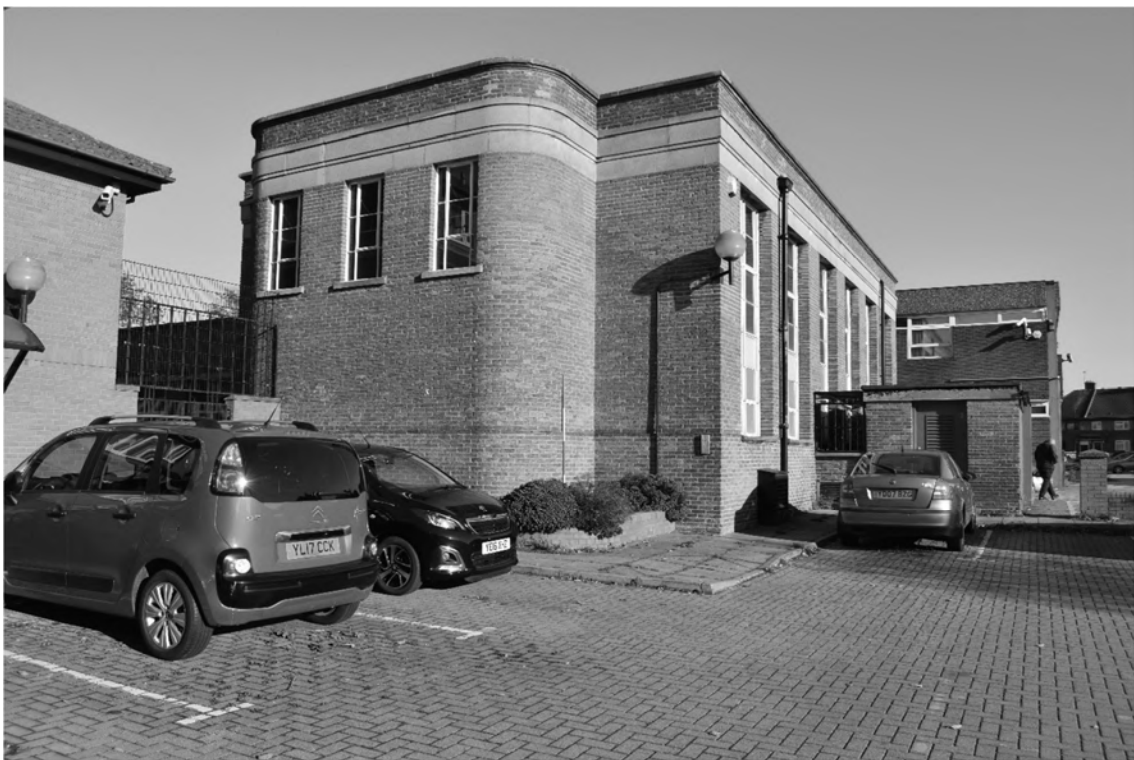
Plate 8. Gymnasium Exterior – South-west Elevation. Facing North.
