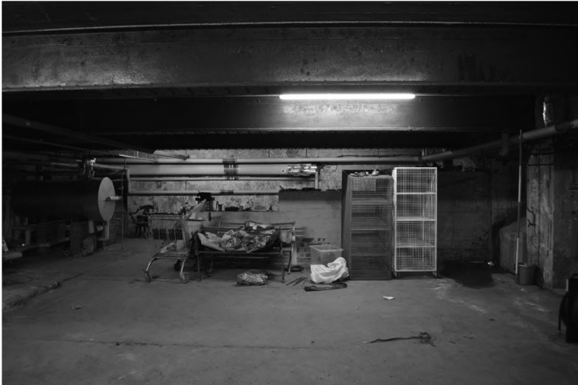
Plate 25. Gymnasium Interior – Basement. Facing North-east.
