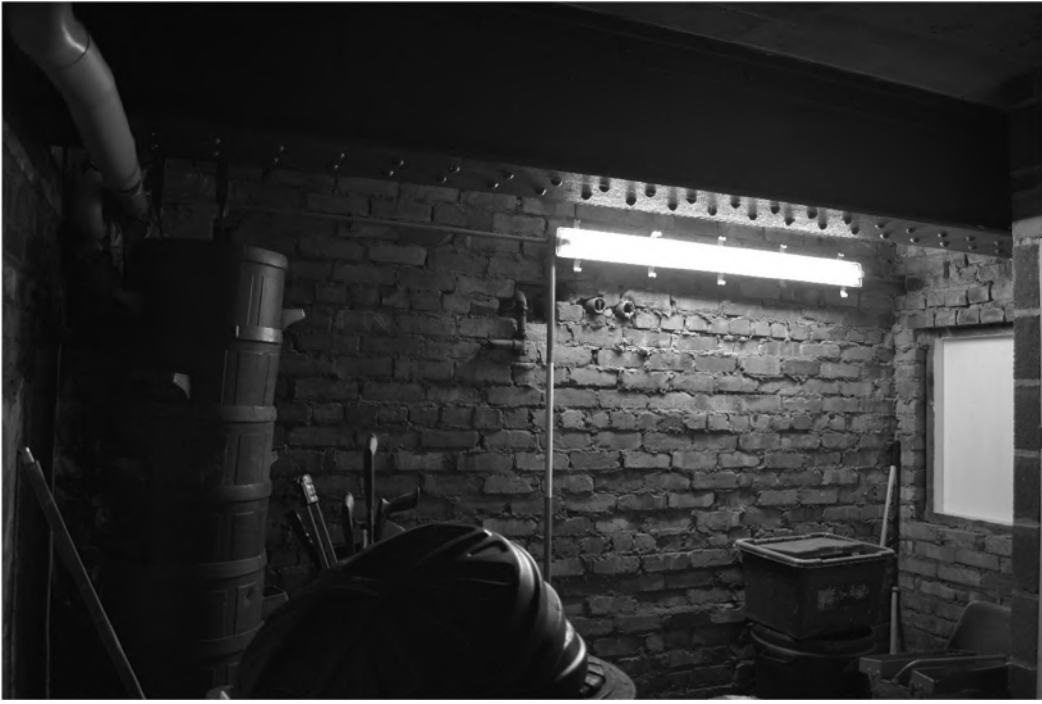
Plate 39. Gymnasium Interior – Basement. Facing North-east.
