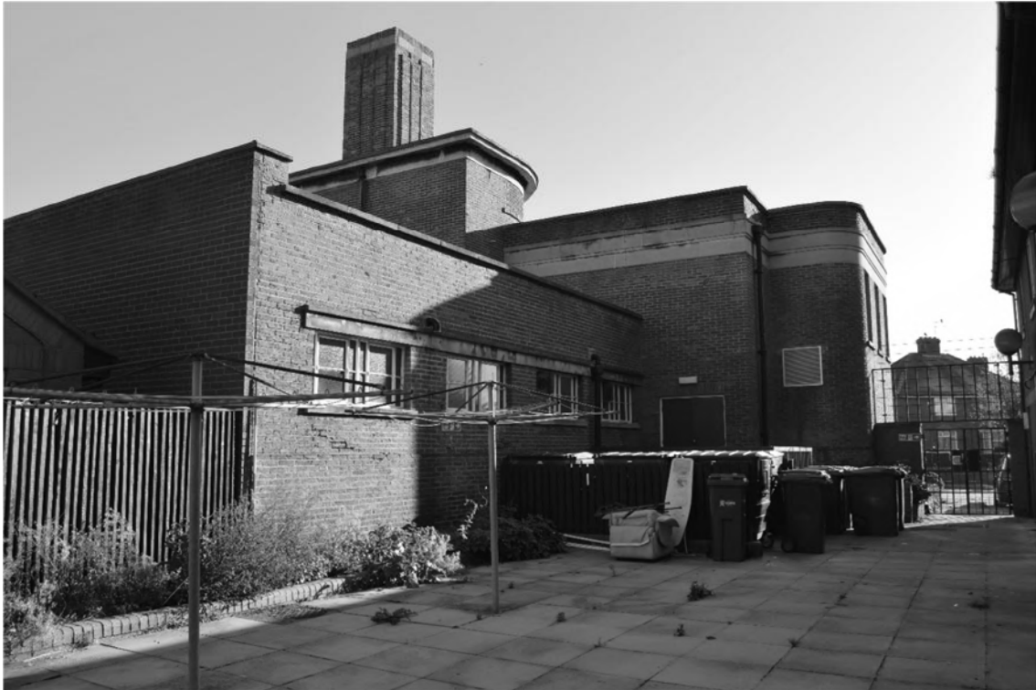
Plate 9. Gymnasium Exterior – South-west Elevation. Facing North-east.
