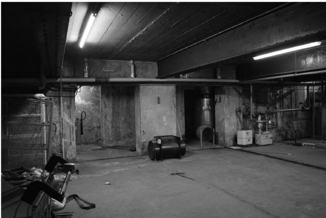
Plate 32. Gymnasium Interior – Basement. Facing South.
