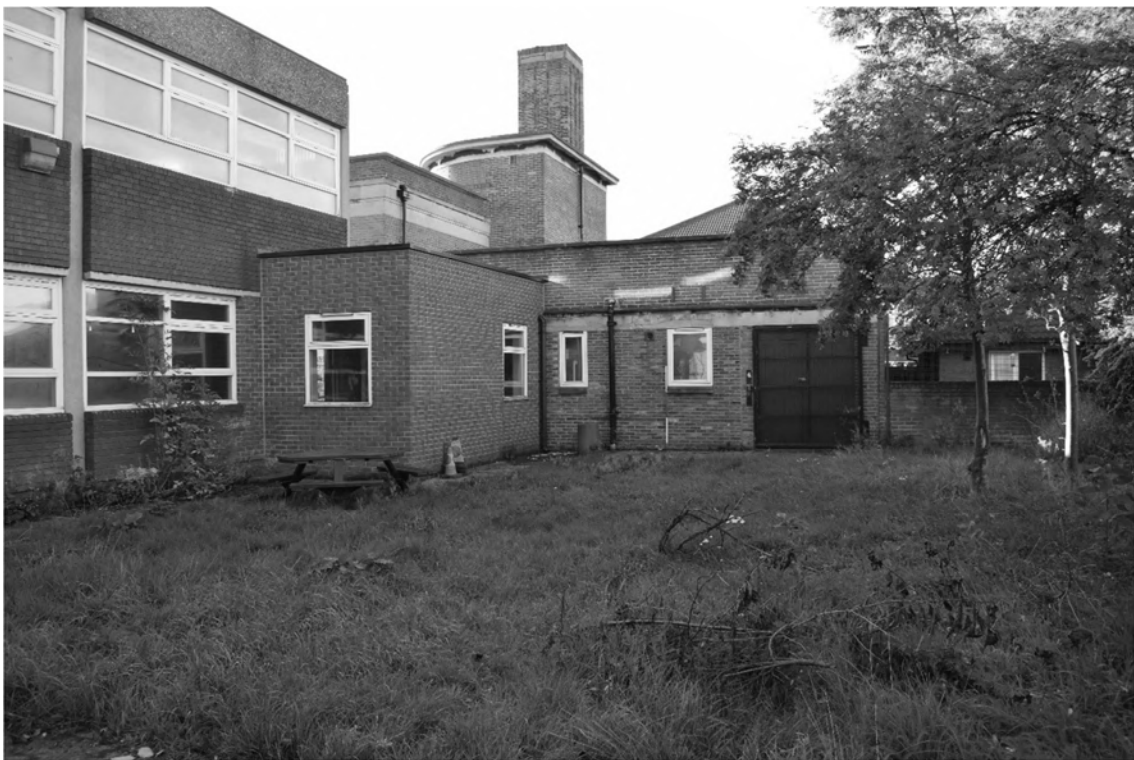
Plate 16. Gymnasium Exterior – North-east Elevation. Facing South-west.
