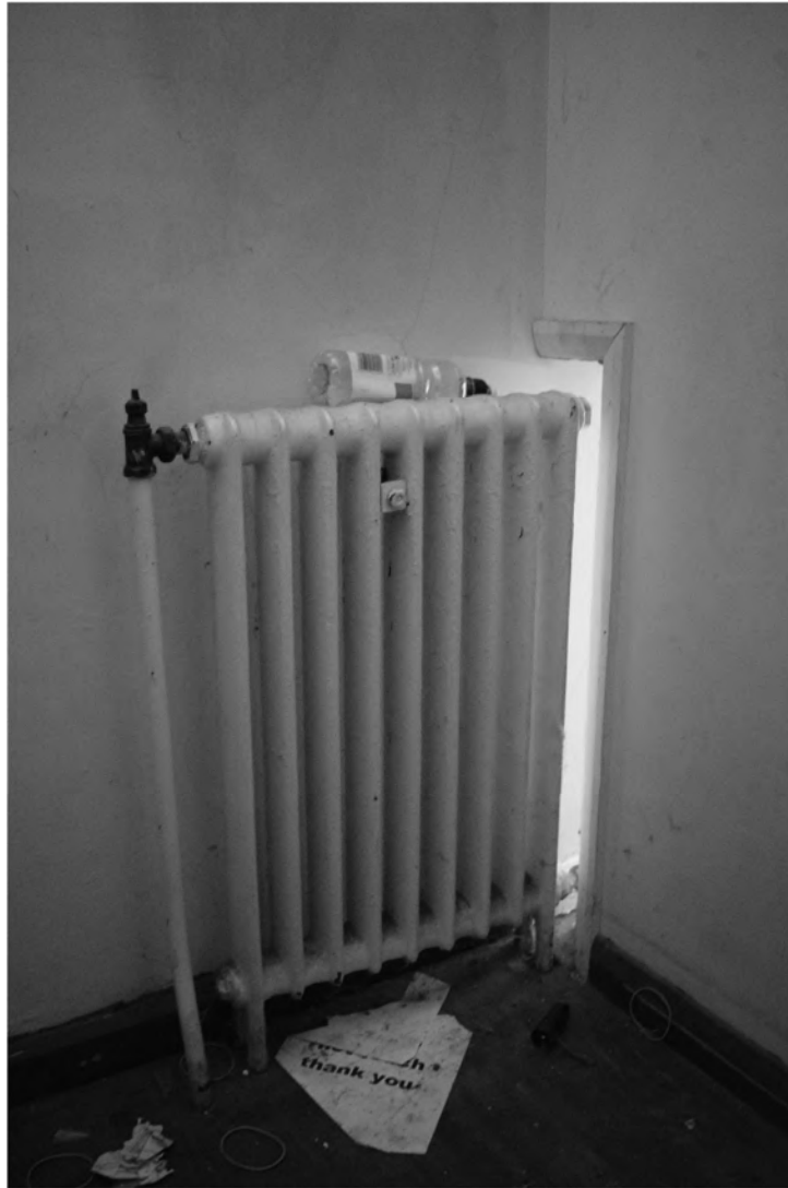
Plate 65. Gymnasium Interior – Ground Floor. Facing South-west.
