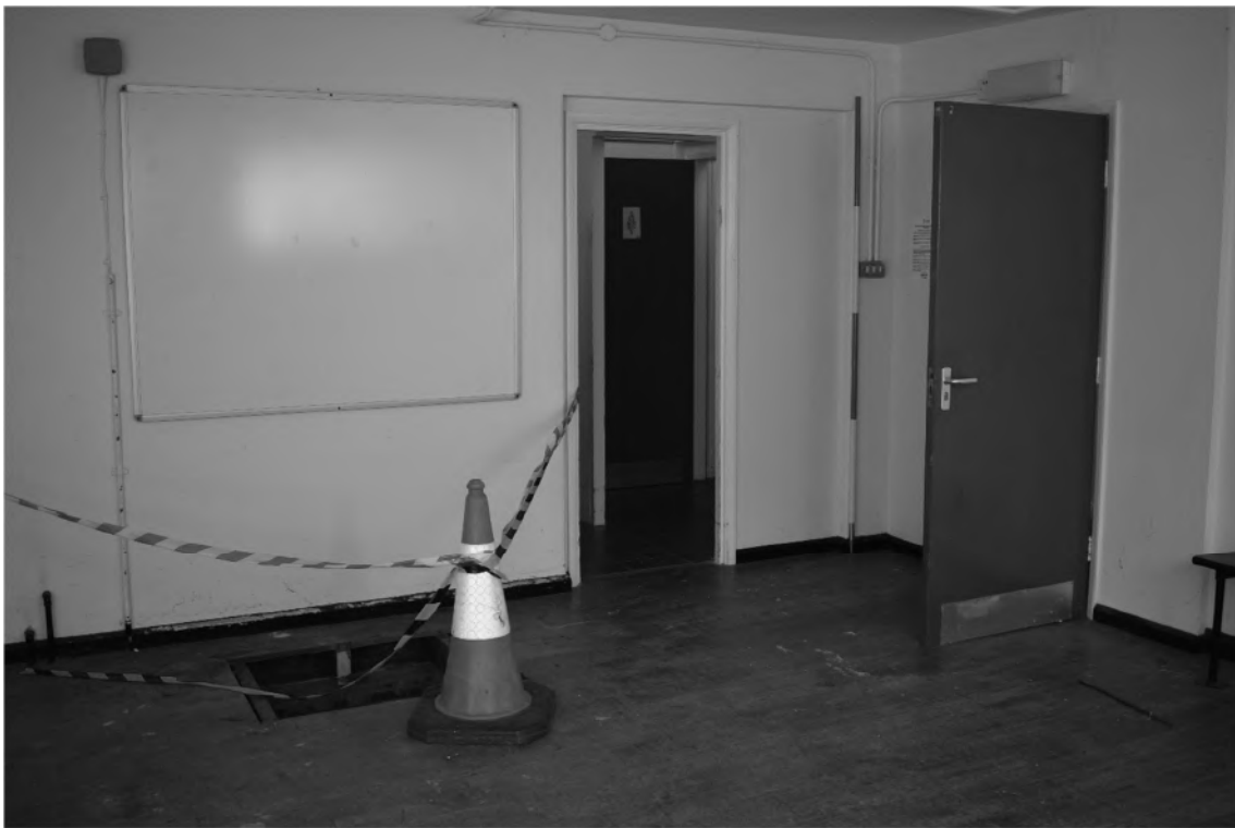
Plate 56. Gymnasium Interior – Ground Floor. Facing East.
