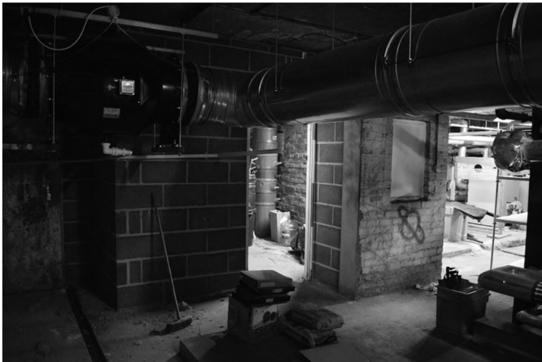
Plate 38. Gymnasium Interior – Basement. Facing North-west.
