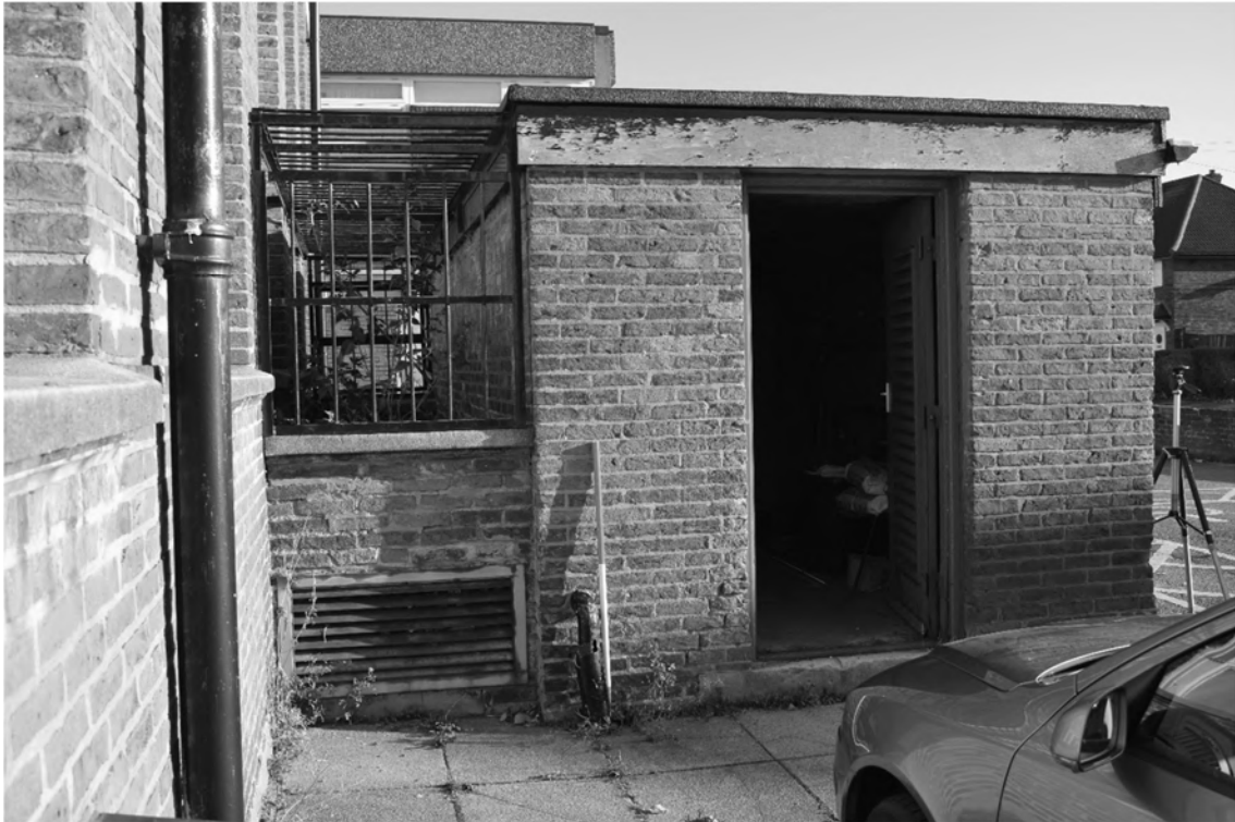
Plate 21. Gymnasium: Entrance to Boiler Room Basement. Facing North-east.
