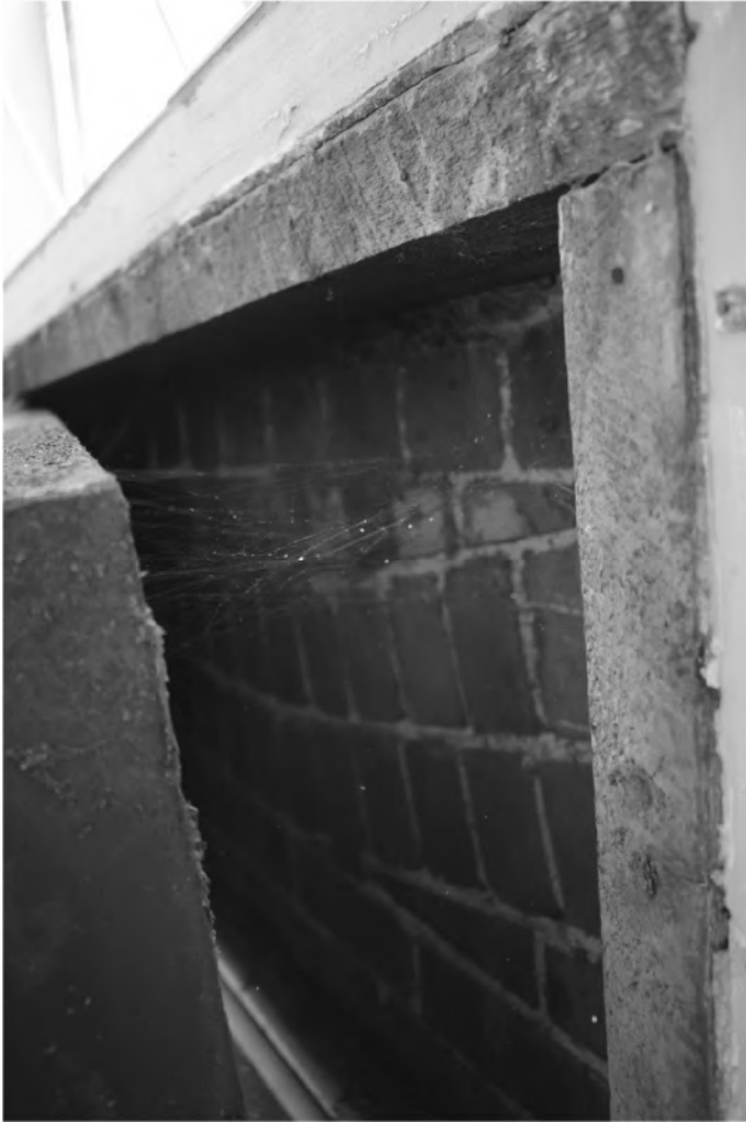
Plate 49. Gymnasium Interior – Ground Floor. Facing East.
