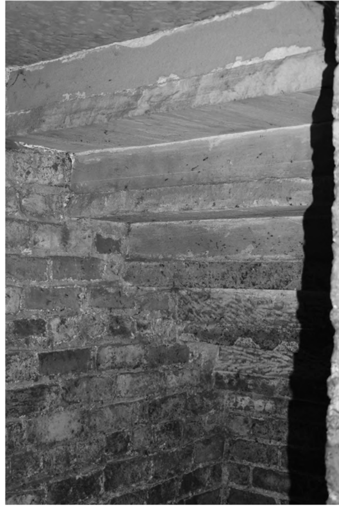
Plate 36. Farmhouse: Coal Store. Facing South (Photo: DSC_1027).
