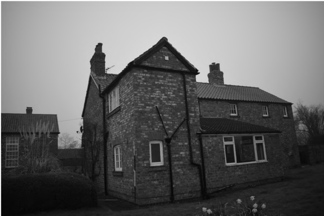
Plate 8. Farmhouse: Exterior – North and East Elevations. Facing South-west (Photo DSC_0971).
