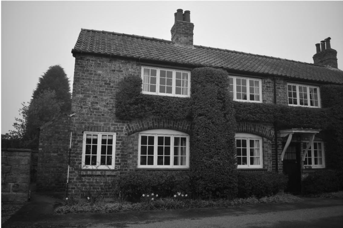
Plate 3. Farmhouse: Exterior – South Elevation. Facing North-east (Photo DSC_0958).
