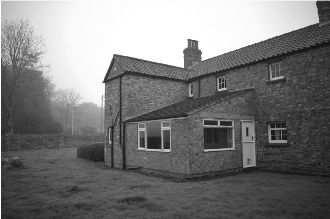
Plate 9. Farmhouse: Exterior – North and West Elevations. Facing South (Photo DSC_0976).
