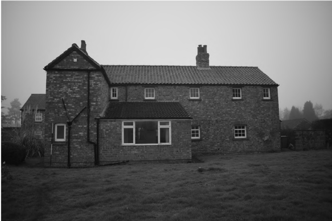
Plate 7. Farmhouse: Exterior – North Elevation. Facing South-west (Photo DSC_072).
