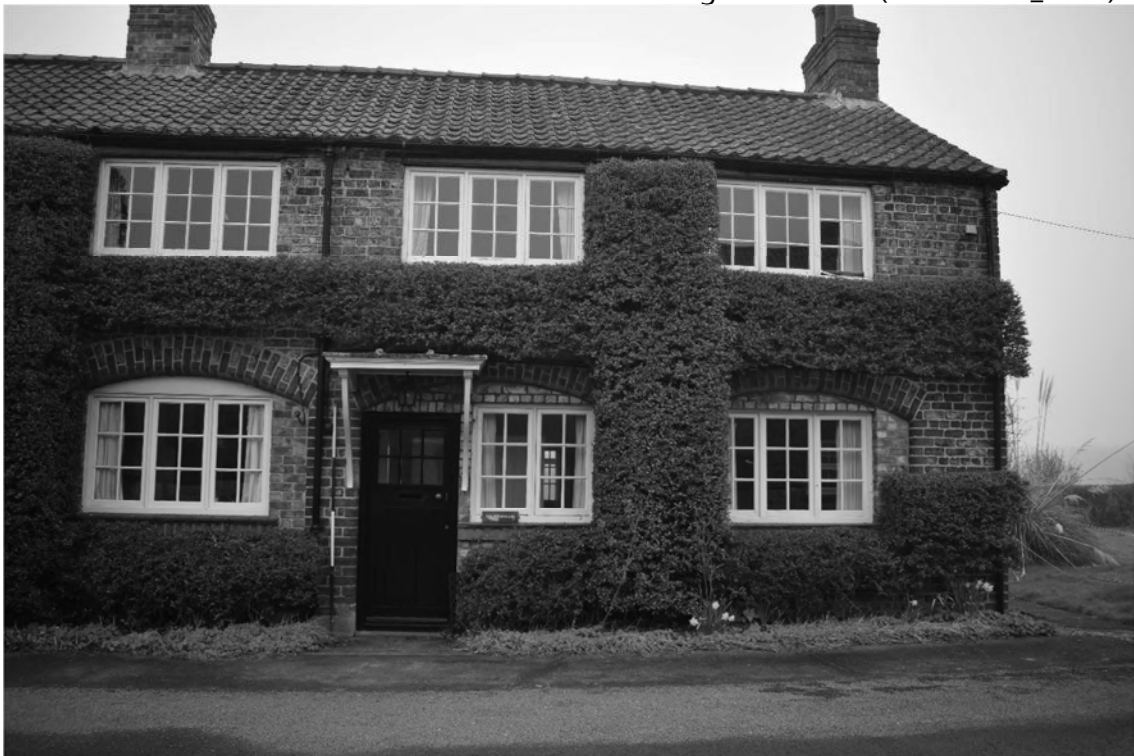
Plate 4. Farmhouse: Exterior – South Elevation. Facing North-east (Photo DSC_0960).
