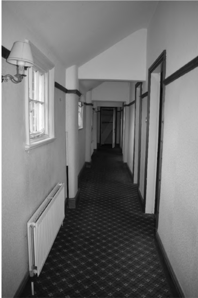
Plate 27. Farmhouse: Interior – First Floor. Facing South-east (Photo: DSC_1008).
