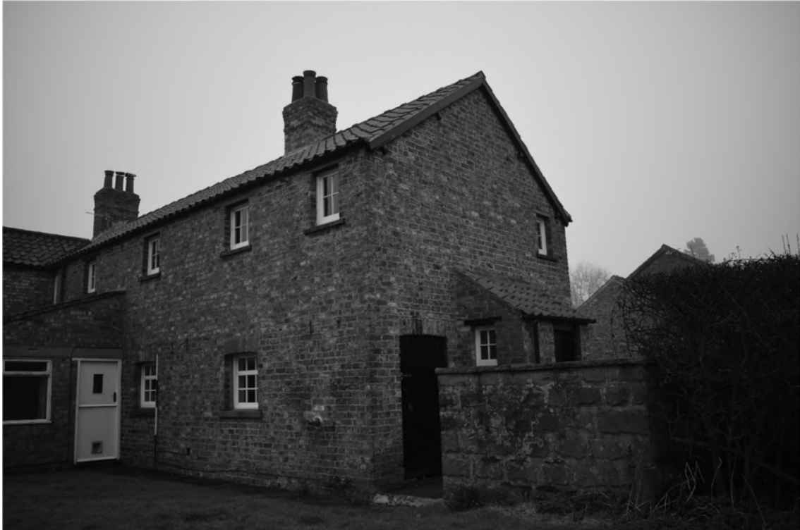
Plate 6. Farmhouse: Exterior – North and West Elevations. Facing South (Photo DSC_0981).
