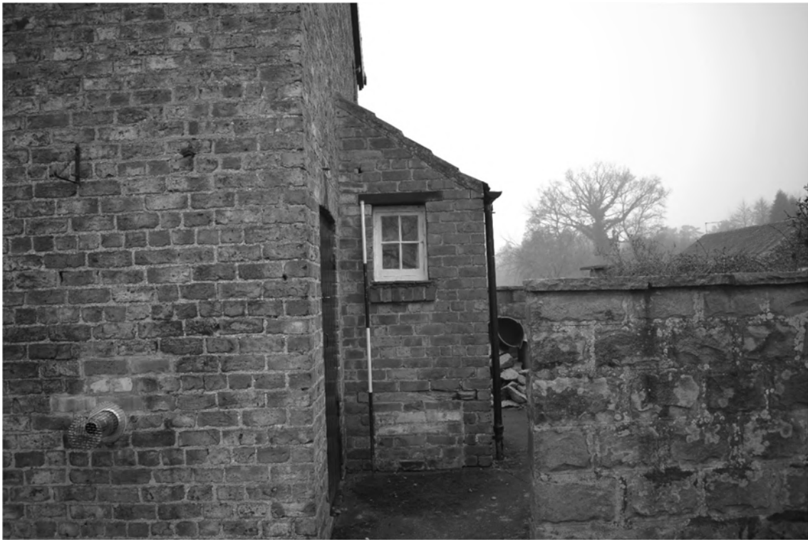
Plate 13. Farmhouse: Exterior – North Elevation. Facing South-west (Photo DSC_0982).
