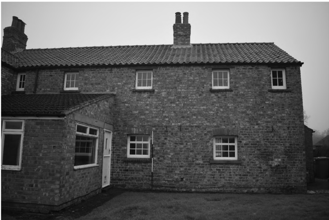
Plate 10. Farmhouse: Exterior – North Elevation. Facing South-west (Photo DSC_0977).
