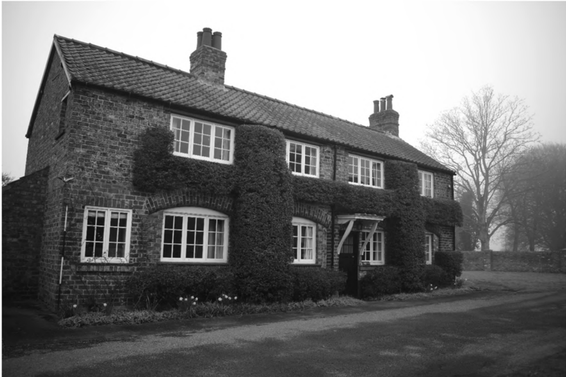
Plate 1. Farmhouse: Exterior – South Elevation. Facing North-east (Photo DSC_0957).
