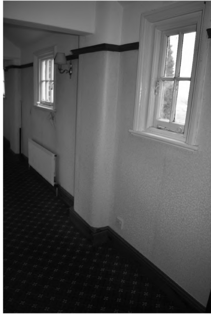
Plate 30. Farmhouse: Interior – First Floor. Facing North-west (Photo: DSC_1023).
