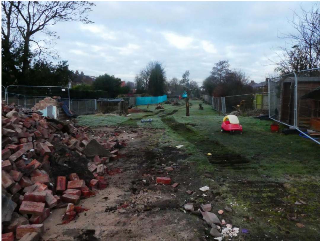
Plate 1: General view of the site. Facing North-West.
