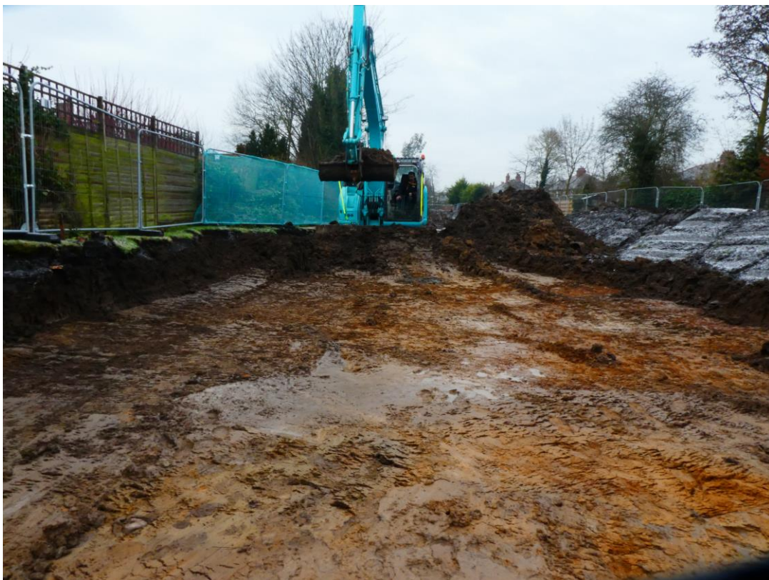
Plate 4: Stripping the site. Facing Southeast.
