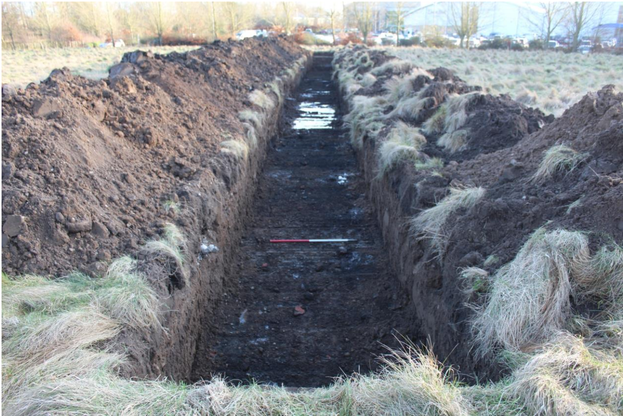
Plate 3: Trench 1. Facing South-East. 1m Scale.
