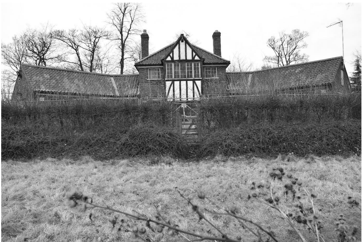
Plate 2. Pavilion: Exterior - South Elevation (DSC_0054). Facing North.
