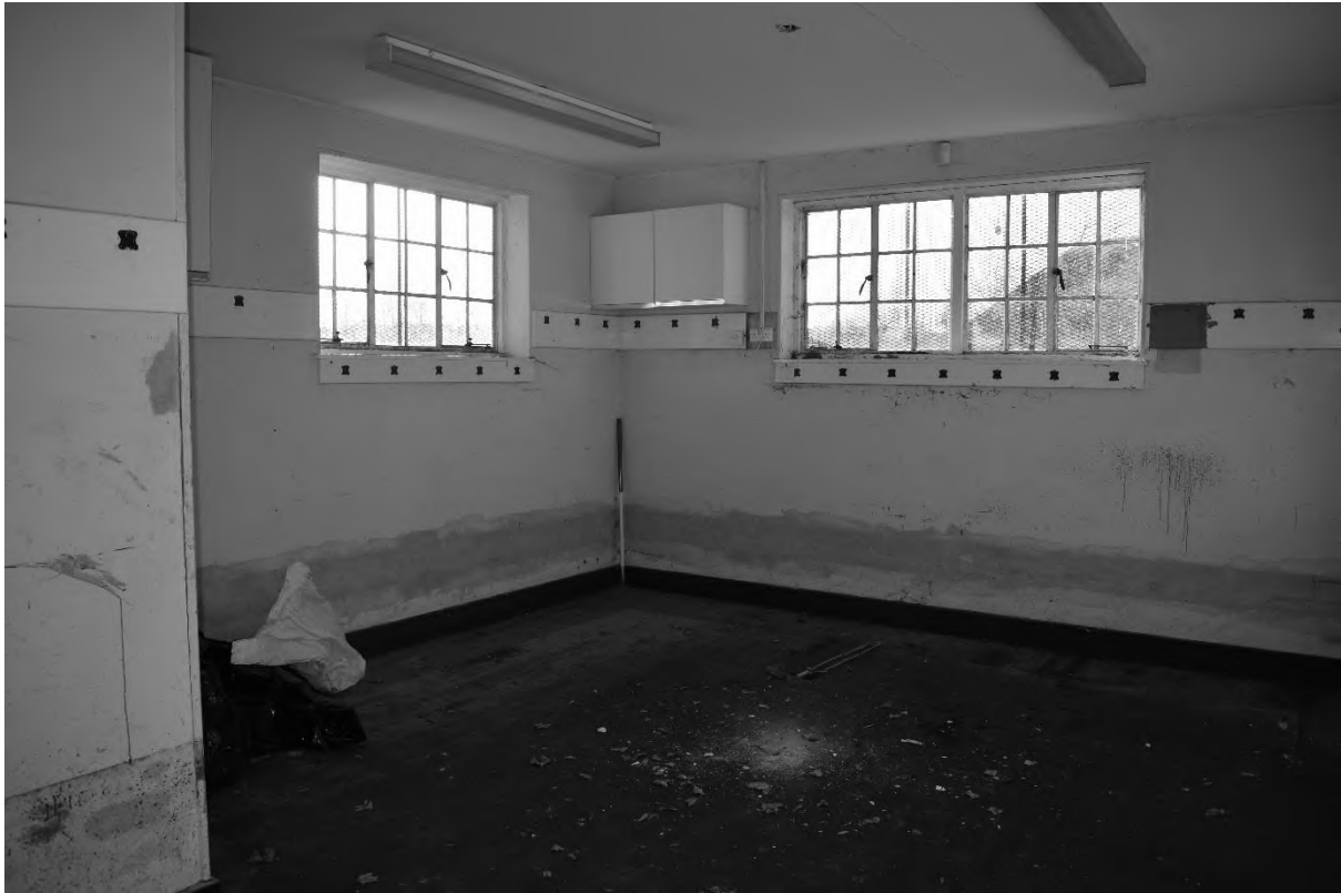
Plate 37. Pavilion: Interior – Ground Floor (DSC_0094). Facing West.
