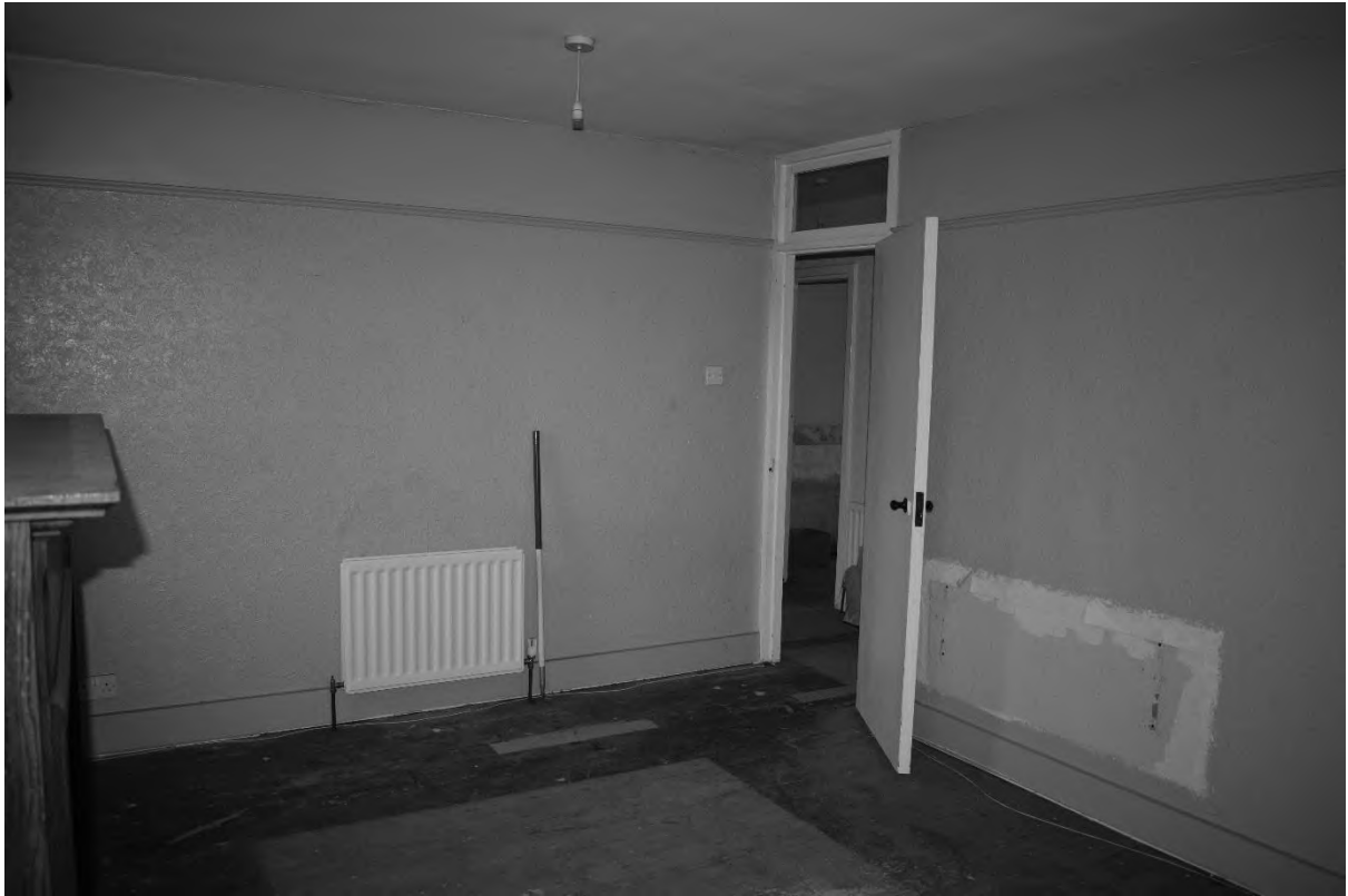
Plate 45. Pavilion: Interior – First Floor (DSC_0062). Facing North.
