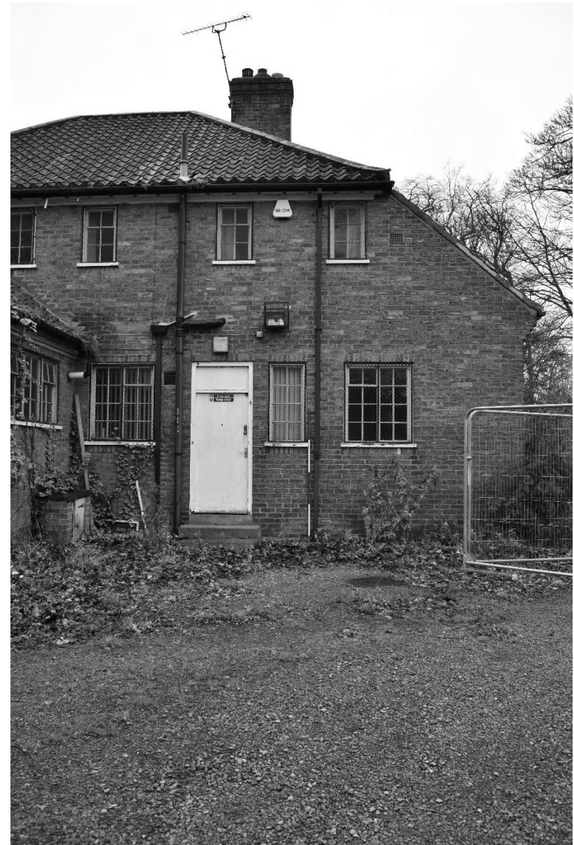
Plate 16. Pavilion: Exterior – East Elevation (DSC_0037). Facing West.
