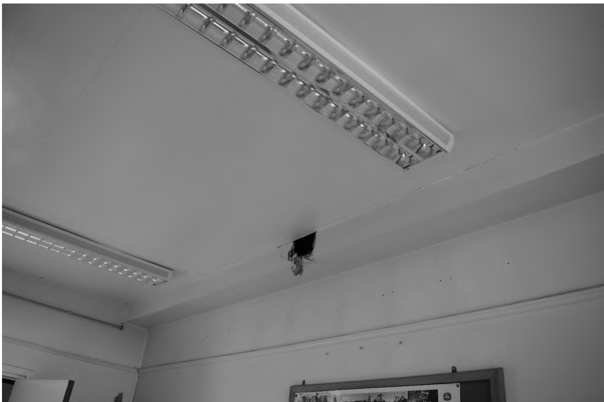
Plate 26. Pavilion: Interior – Ground Floor (DSC_0082). Facing East.
