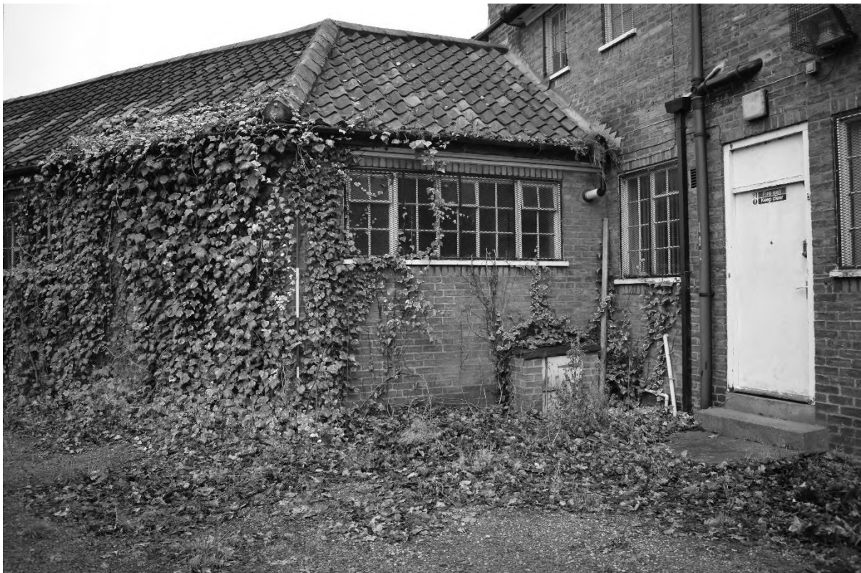
Plate 14. Pavilion: Exterior – North, North-east & East Elevations (DSC_0034). Facing South.
