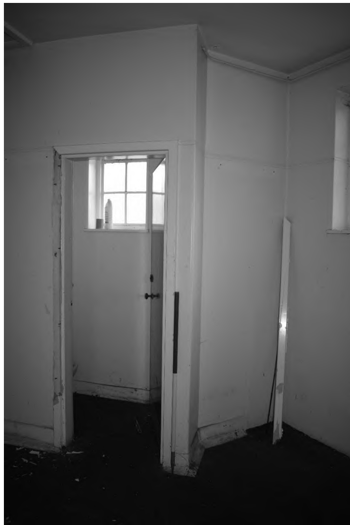
Plate 32. Pavilion: Interior – Ground Floor (DSC_0089). Facing North.
