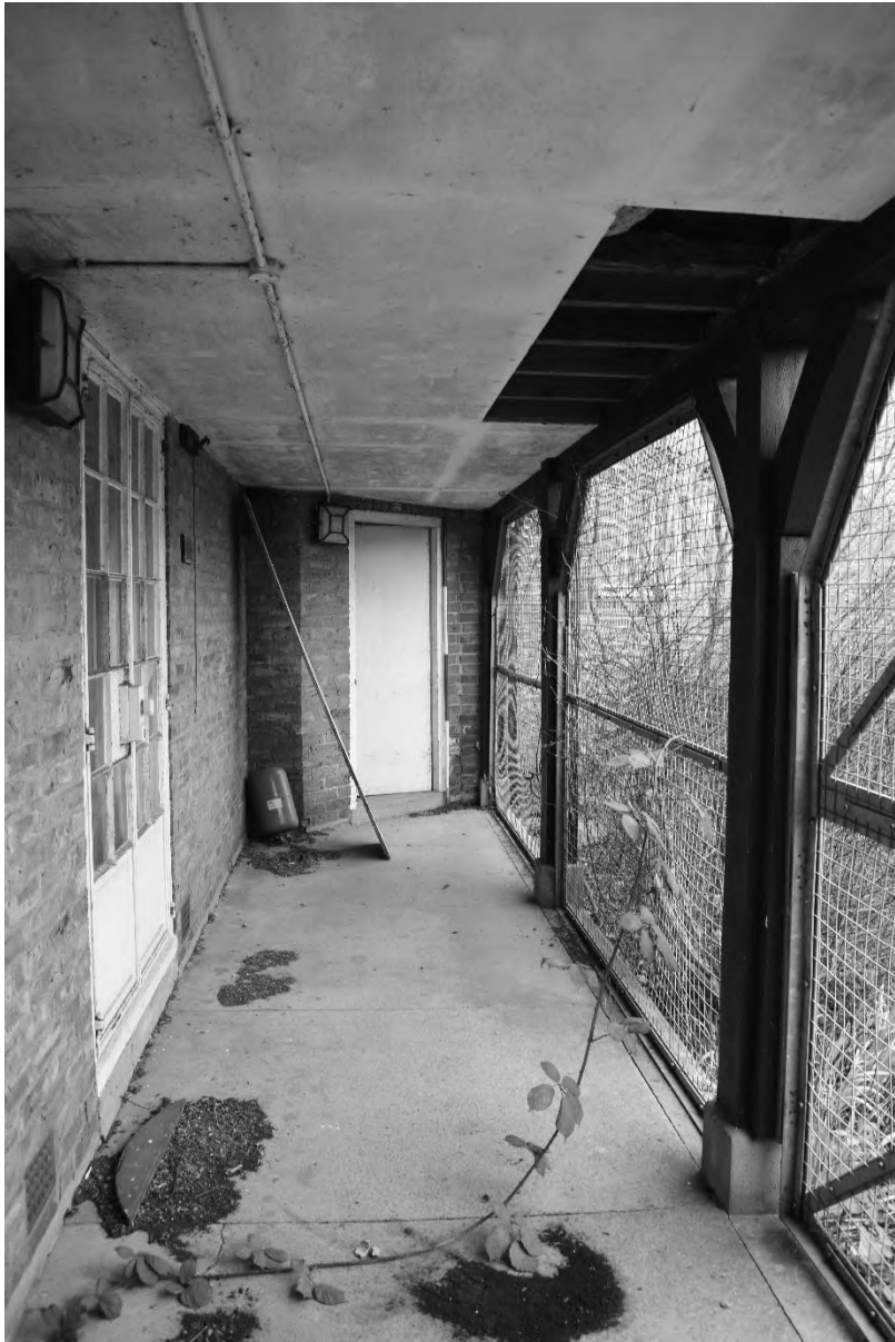
Plate 9. Pavilion: Exterior – Veranda (DSC_0057). Facing South-east.
