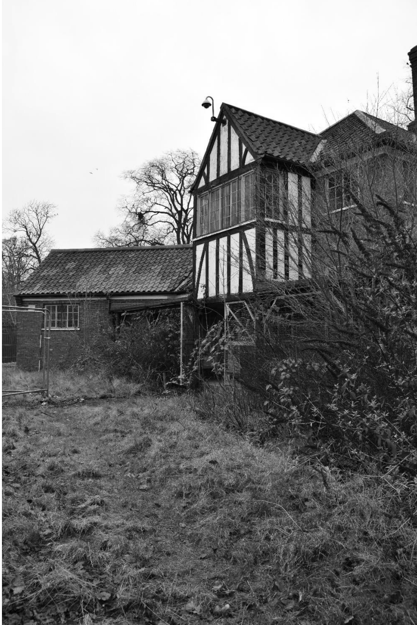
Plate 3. Pavilion: Exterior – South and South-east Elevations (DSC_0040). Facing North-west. 16/02358/OUTM
