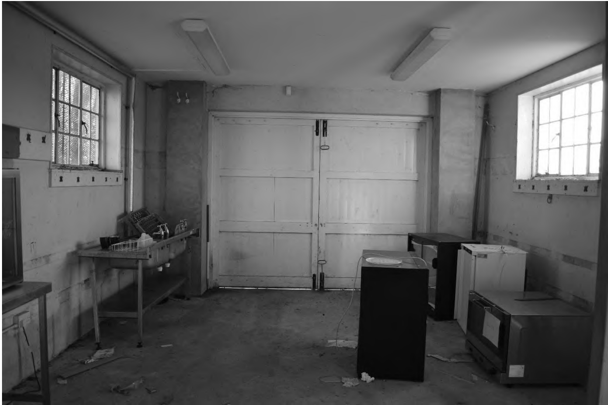
Plate 39. Pavilion: Interior – Ground Floor (DSC_0096). Facing South-east.
