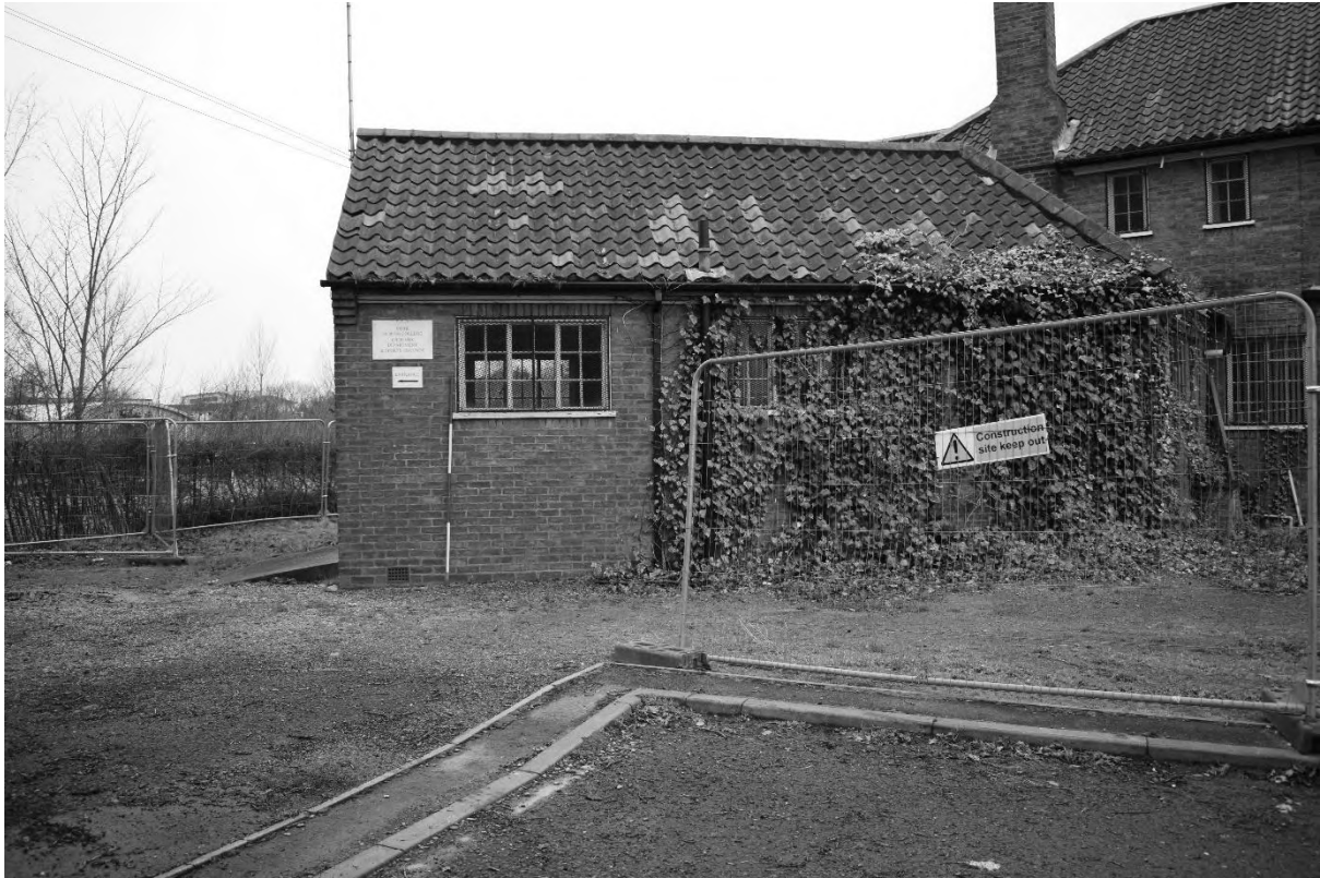
Plate 13. Pavilion: Exterior – North-east and North Elevations (DSC_0033). Facing South-west.
