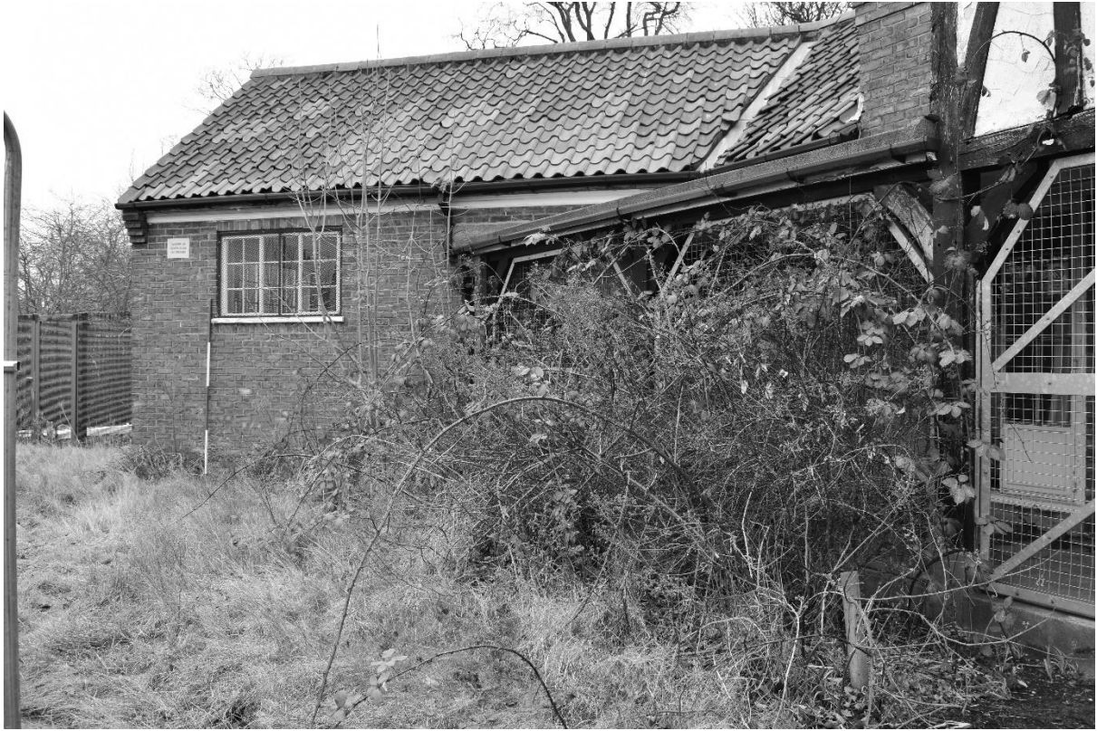
Plate 7. Pavilion: Exterior – South-west Elevation (DSC_0046). Facing West.
