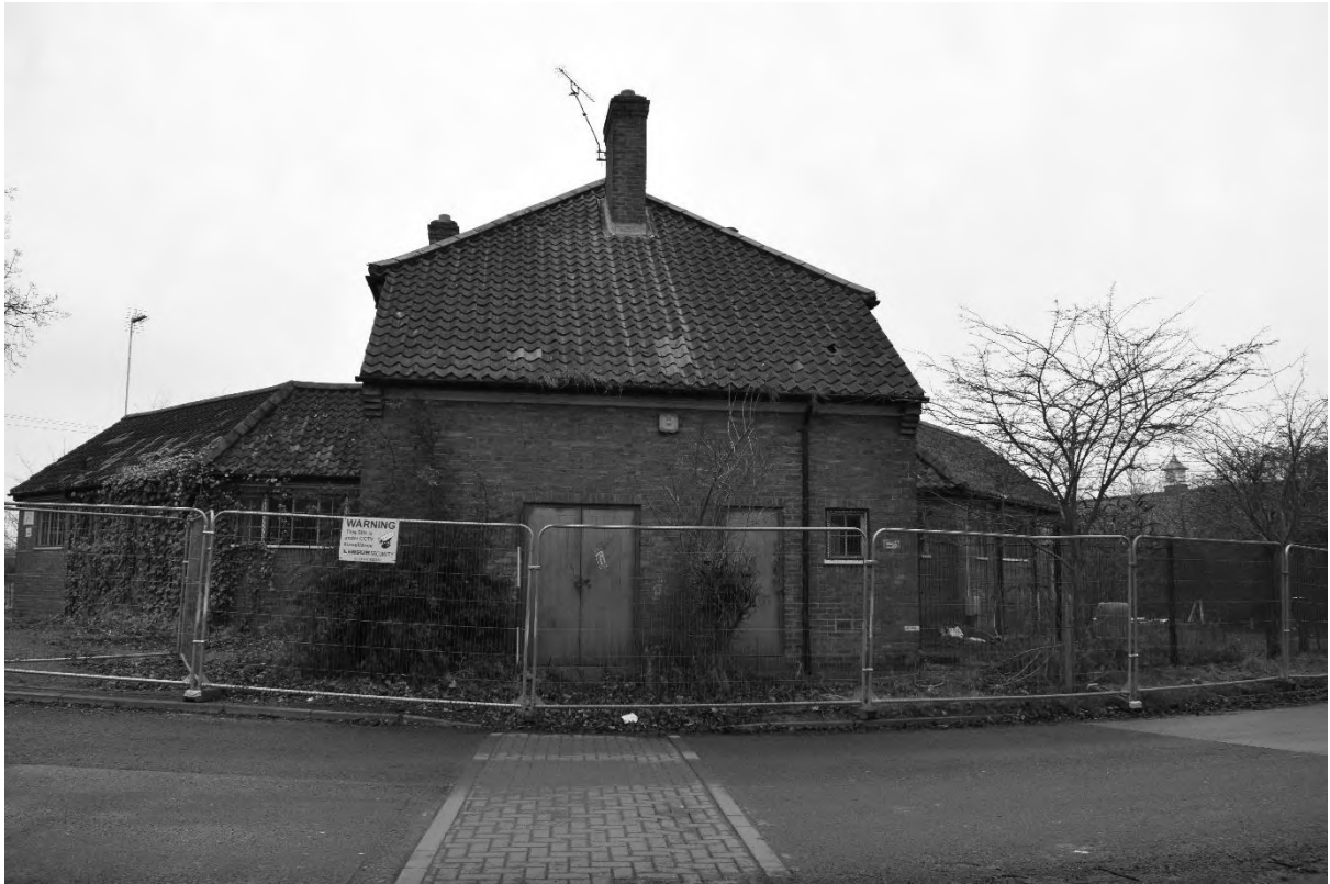
Plate 17. Pavilion: Exterior – North Elevation (DSC_0038). Facing South.
