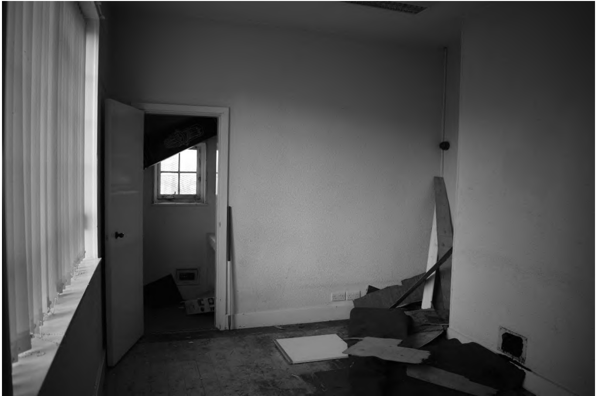
Plate 29. Pavilion: Interior – Ground Floor (DSC_0086). Facing North.
