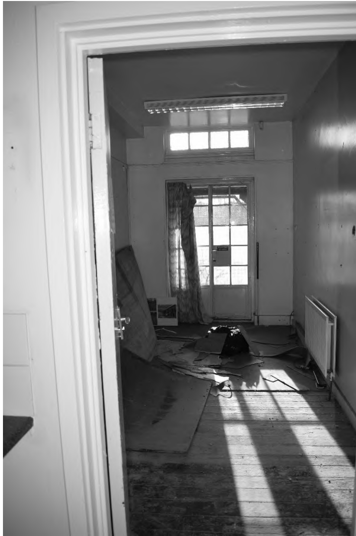
Plate 25. Pavilion: Interior – Ground Floor (DSC_0081). Facing South.
