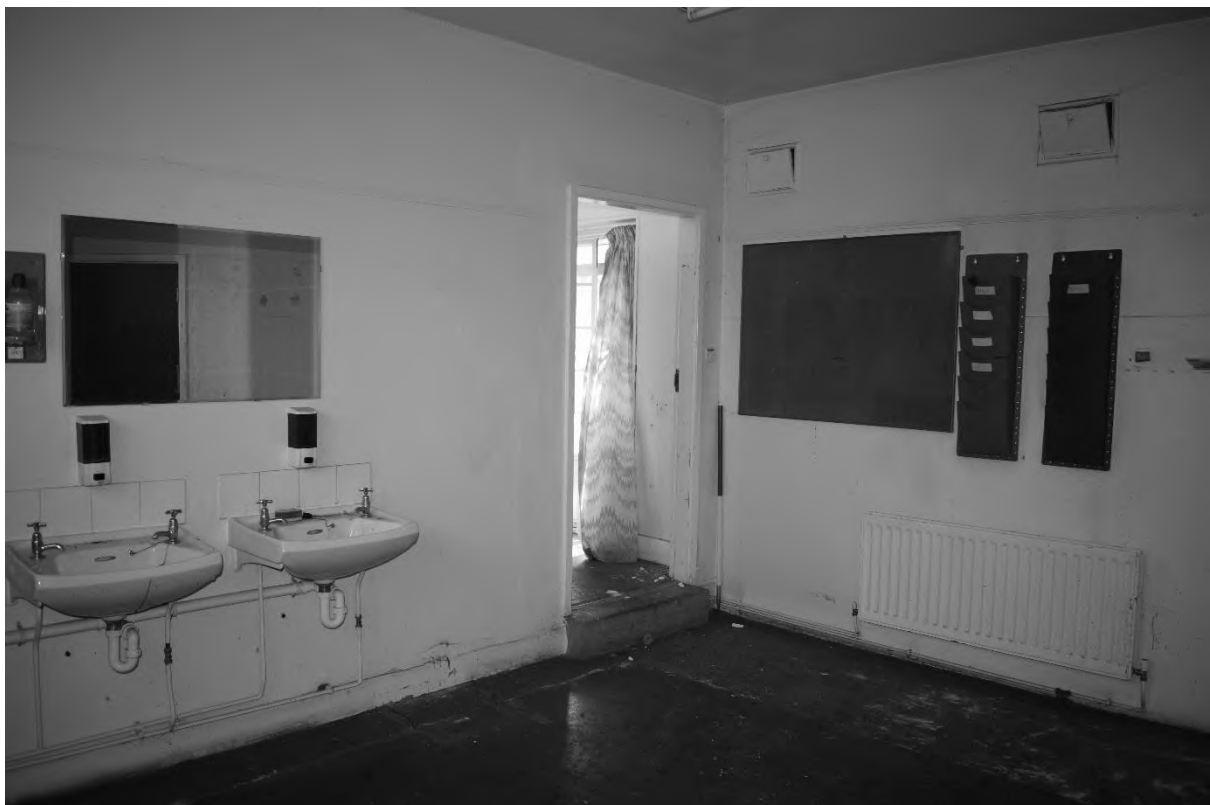
Plate 34. Pavilion: Interior – Ground Floor (DSC_0091). Facing South.
