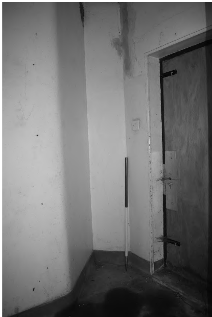
Plate 38. Pavilion: Interior – Ground Floor (DSC_0095). Facing East.
