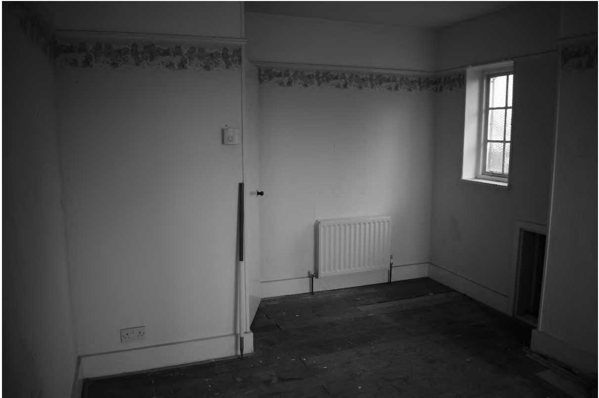
Plate 49. Pavilion Interior – First Floor (DSC_0069). Facing North.
