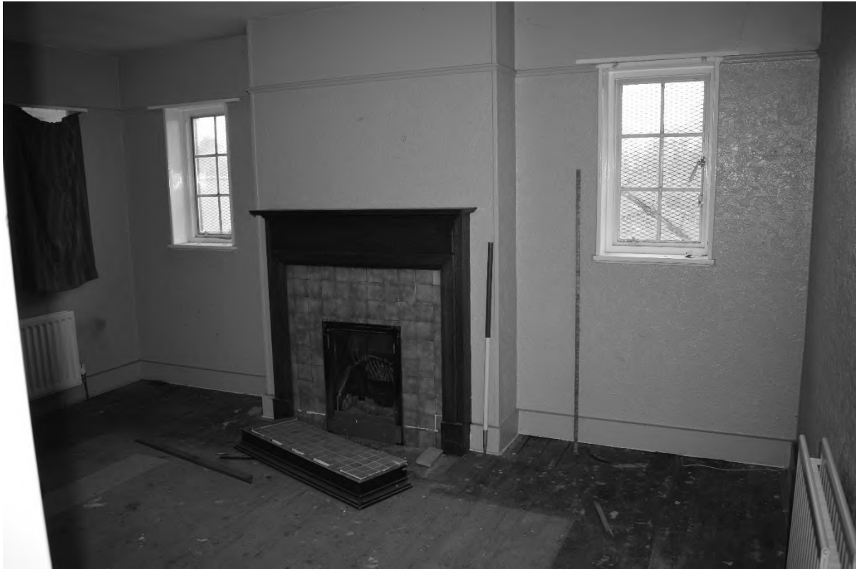
Plate 43. Pavilion: Interior – First Floor (DSC_0059). Facing West.
