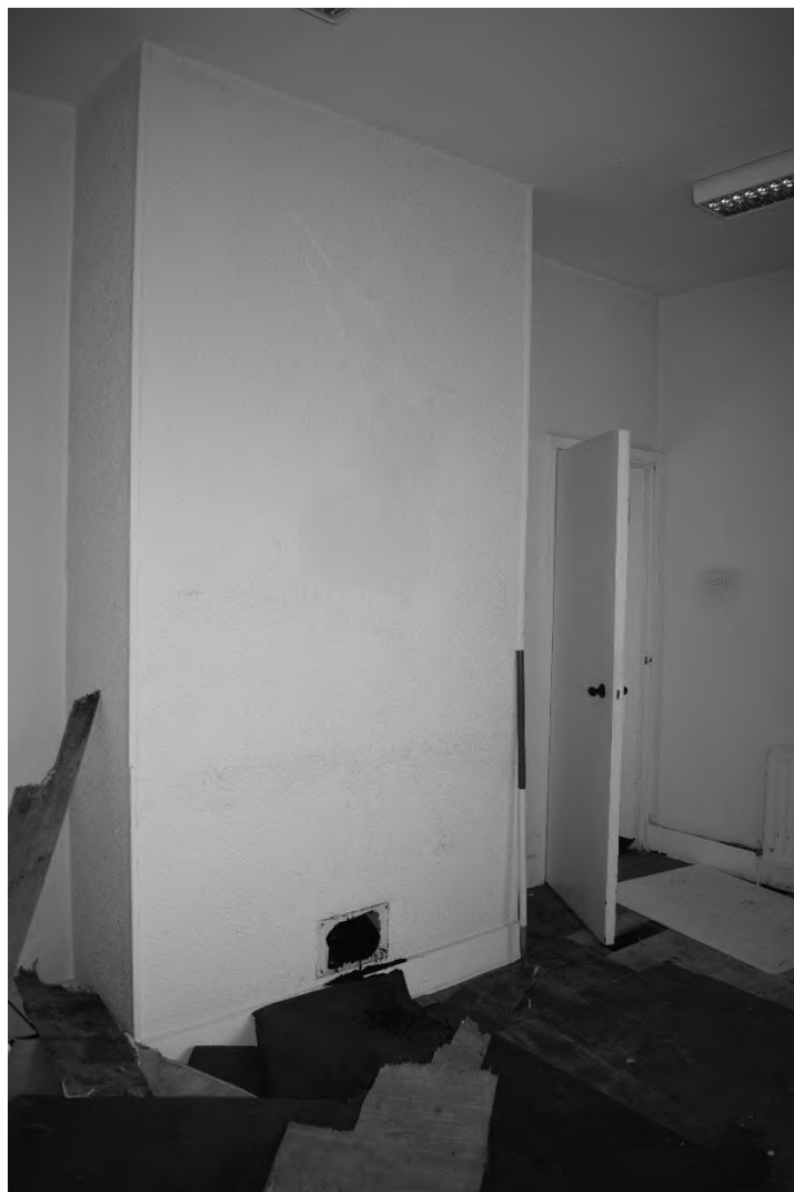
Plate 30. Pavilion: Interior – Ground Floor (DSC_0087). Facing East.
