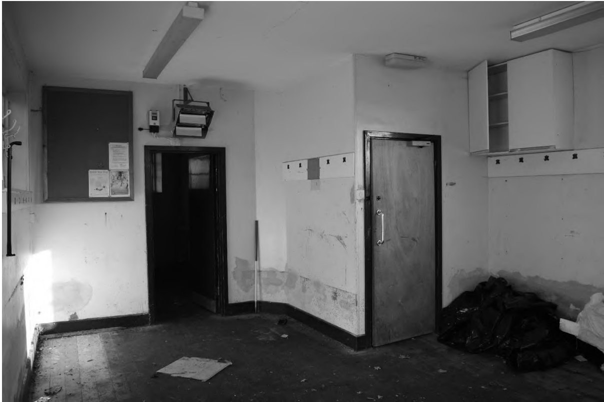
Plate 35. Pavilion: Interior – Ground Floor (DSC_0092). Facing East.
