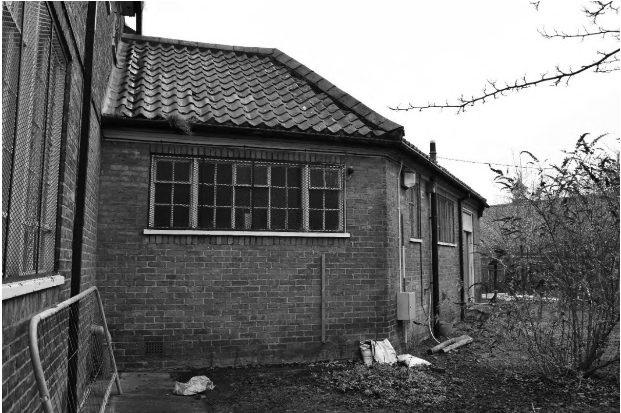
Plate 21. Pavilion: Exterior – North Elevation (DSC_0051). Facing South.
