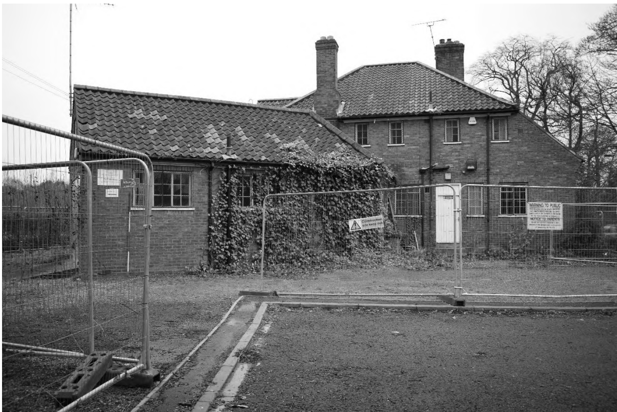
Plate 12. Pavilion: Exterior – North-east, North & East Elevations (DSC_0032). Facing West.
