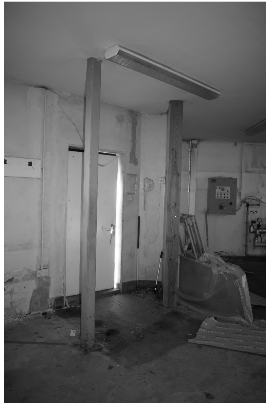
Plate 42. Pavilion: Interior – Ground Floor (DSC_0100). Facing South-east.
