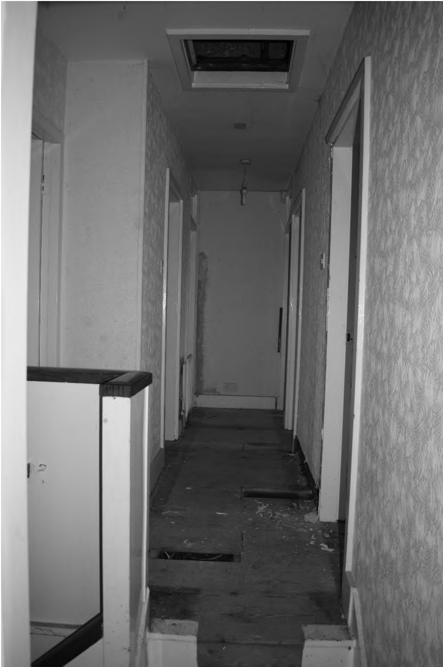
Plate 51. Pavilion Interior – First Floor (DSC_0071). Facing North.
