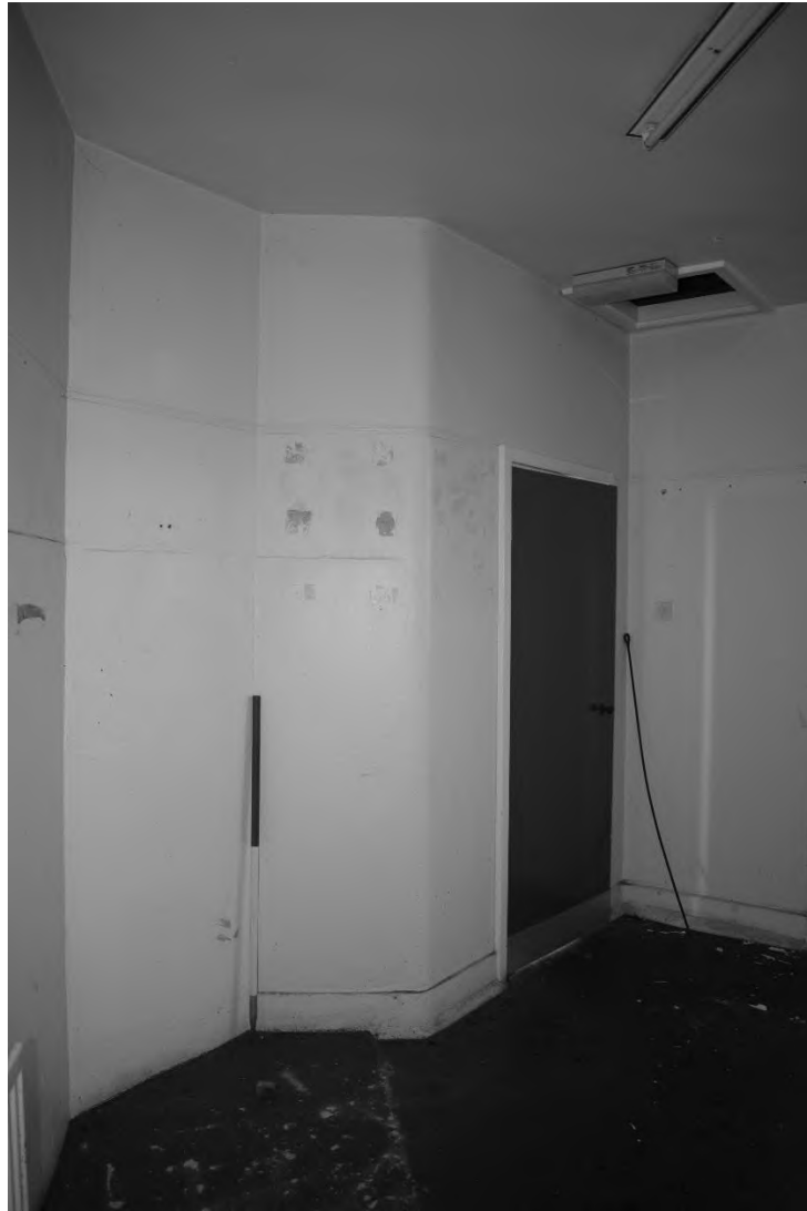
Plate 33. Pavilion: Interior – Ground Floor (DSC_0090). Facing North.
