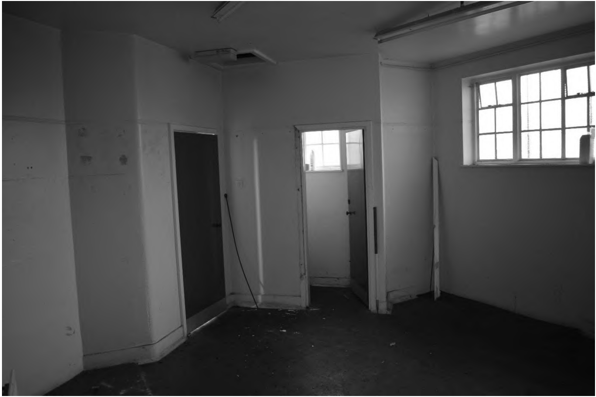
Plate 31. Pavilion: Interior – Ground Floor (DSC_0088). Facing North.
