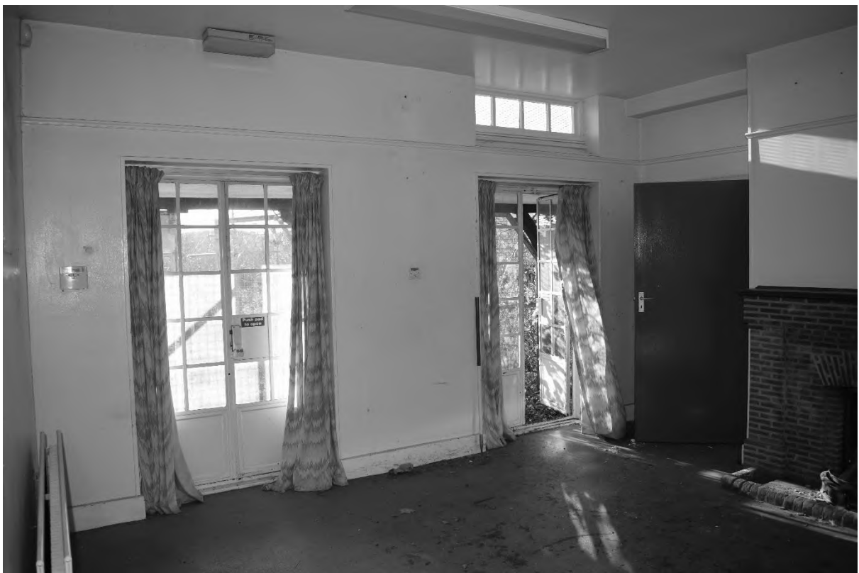
Plate 22. Pavilion: Interior – Ground Floor (DSC_0079). Facing South-west.
