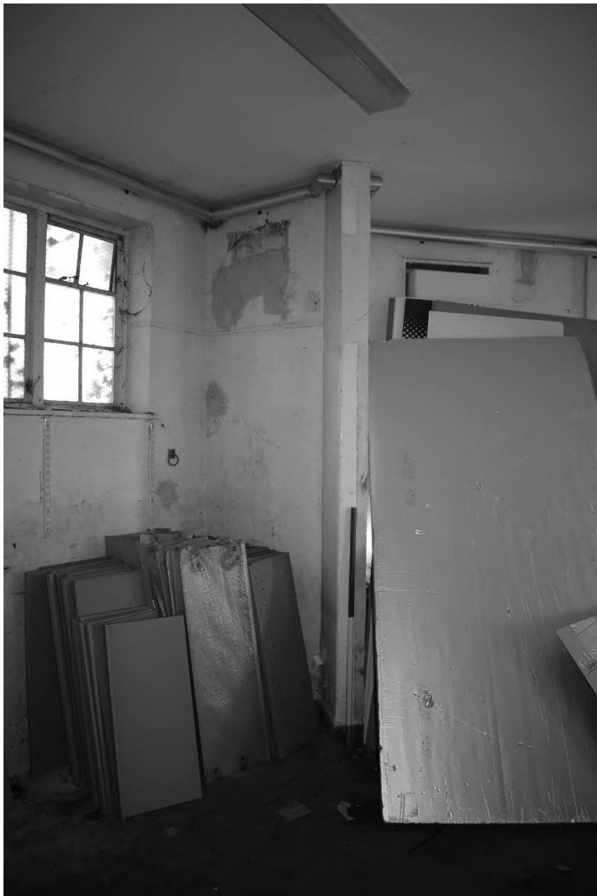
Plate 41. Pavilion: Interior – Ground Floor (DSC_0098). Facing North-east.
