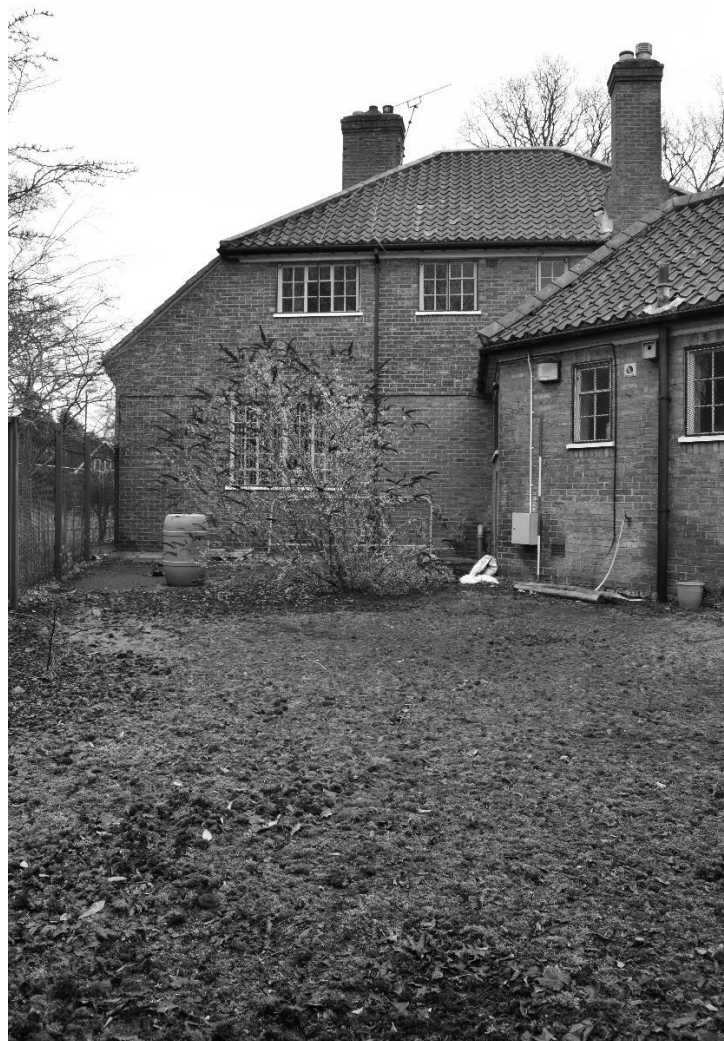
Plate 20. Pavilion: Exterior - West Elevation (DSC_0049). Facing East.
