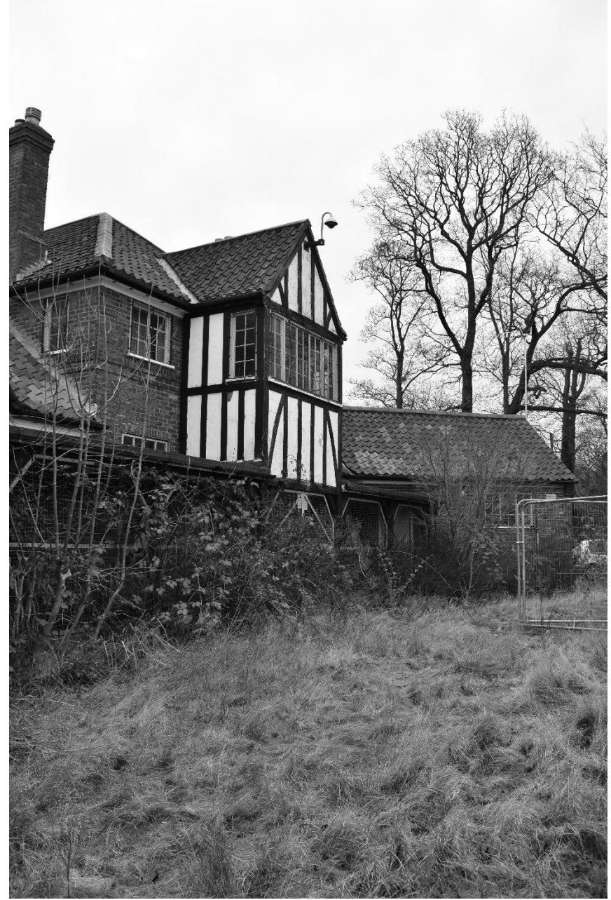
Plate 4. Pavilion: Exterior – South and South-west Elevations (DSC_0045). Facing North-east
