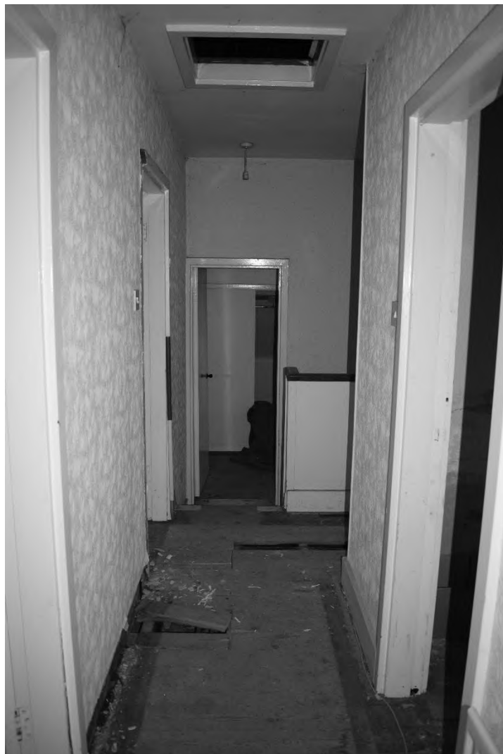
Plate 50. Pavilion Interior – First Floor (DSC_0070). Facing North.
