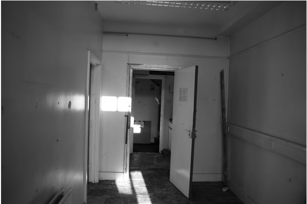
Plate 27. Pavilion: Interior – Ground Floor (DSC_0084). Facing North.
