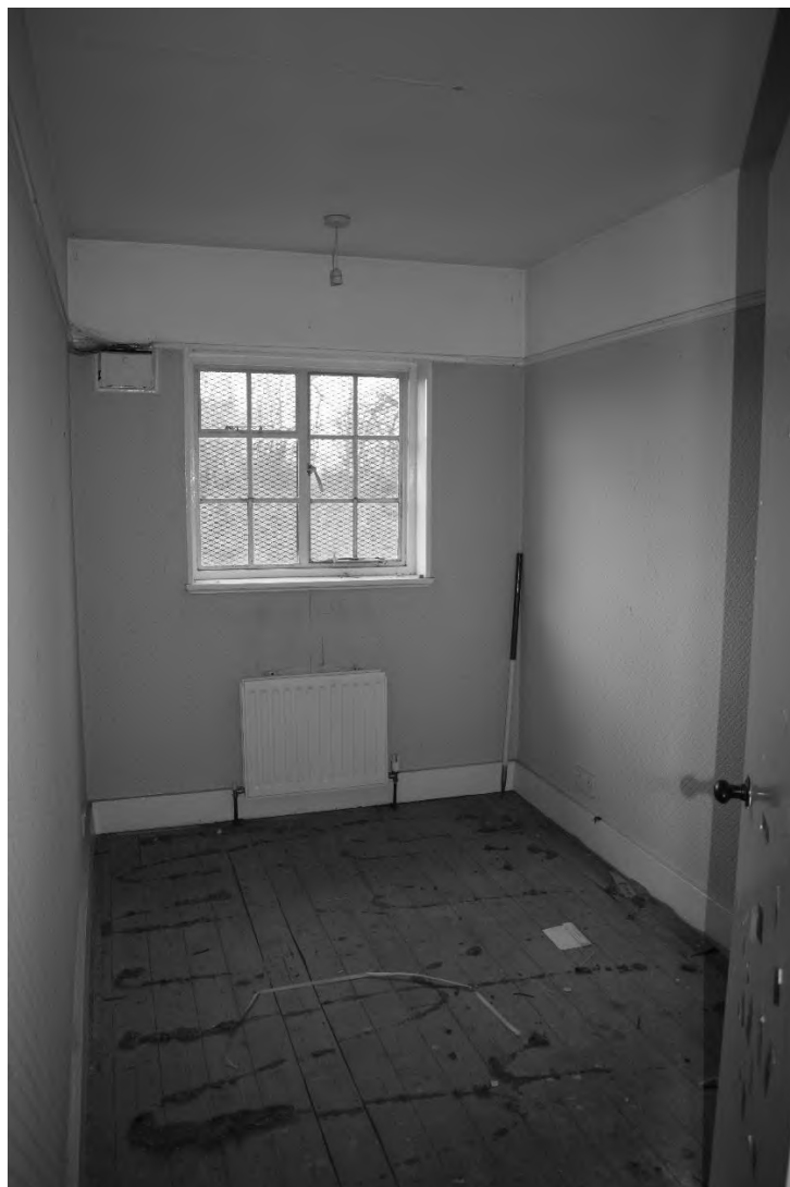
Plate. 54. Pavilion Interior – First Floor (DSC_0075). Facing West.
