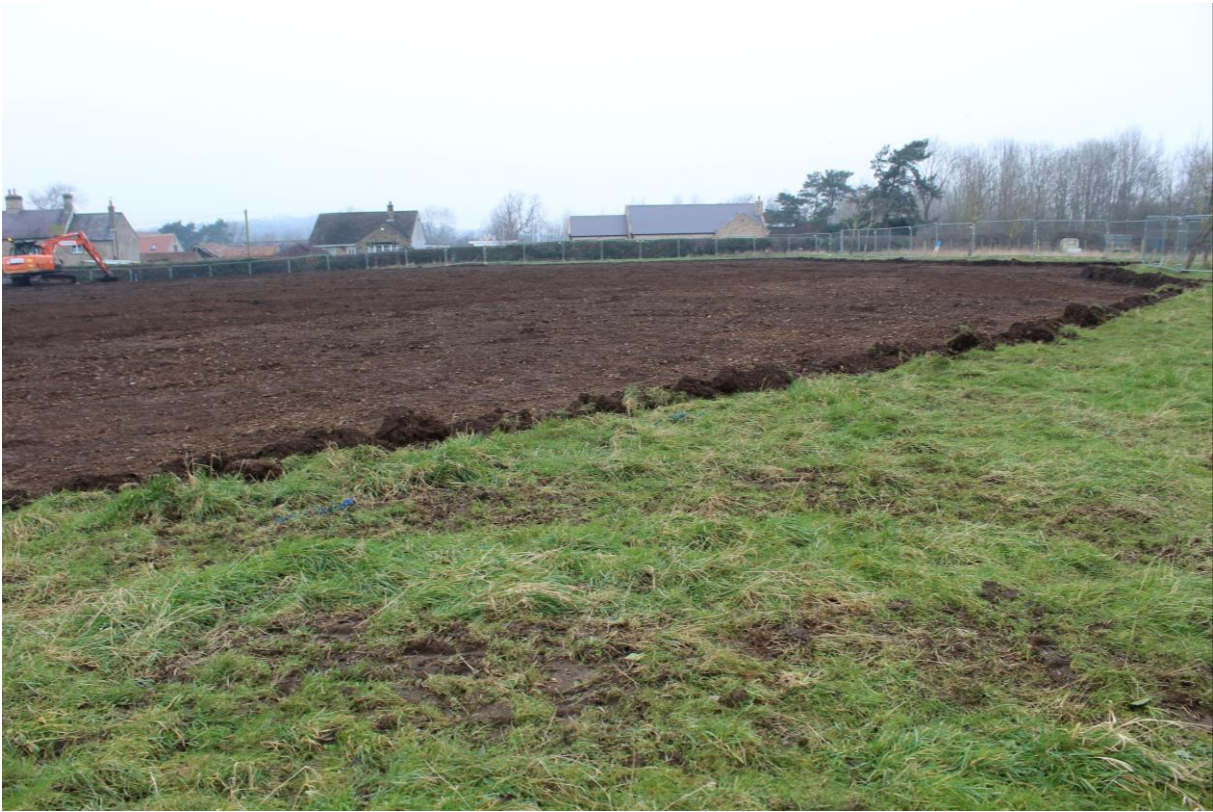
Plate 3: General view of site, facing North-west.
