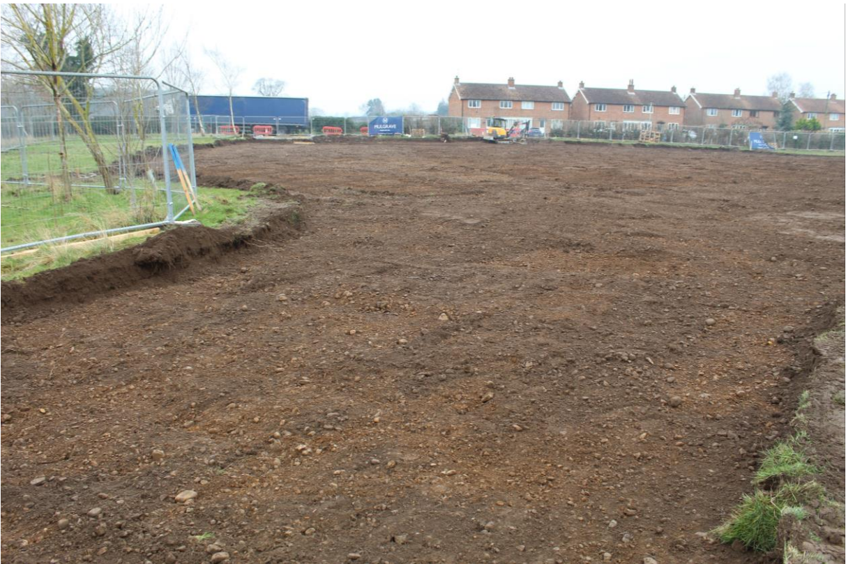
Plate 4: General view of site, facing South.
