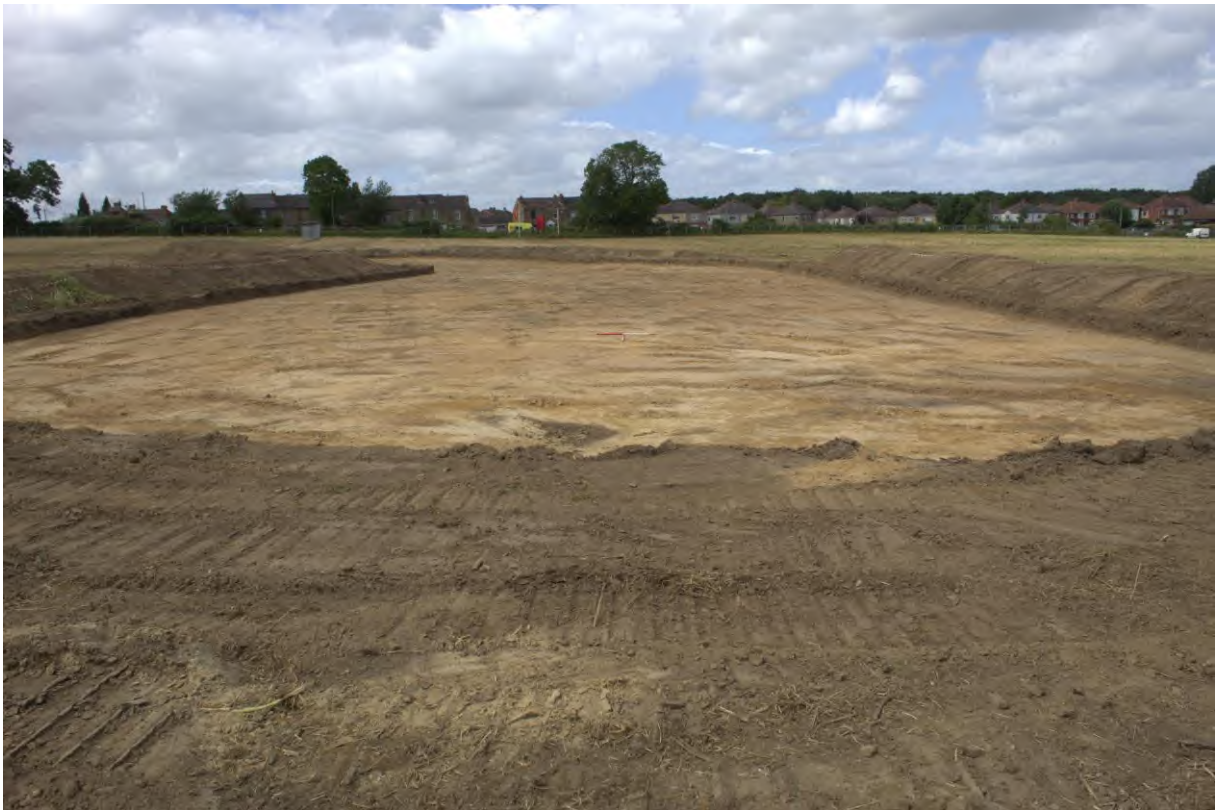
Plate 5: General View of Site, facing North-west.
