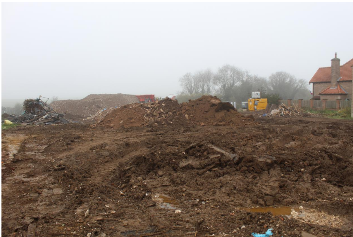
Plate 1: General View of Site, facing North-east.
