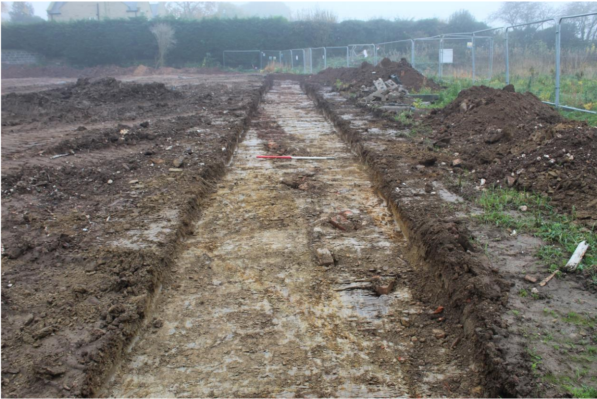
Plate 5: General View of Trench 2, facing South.
