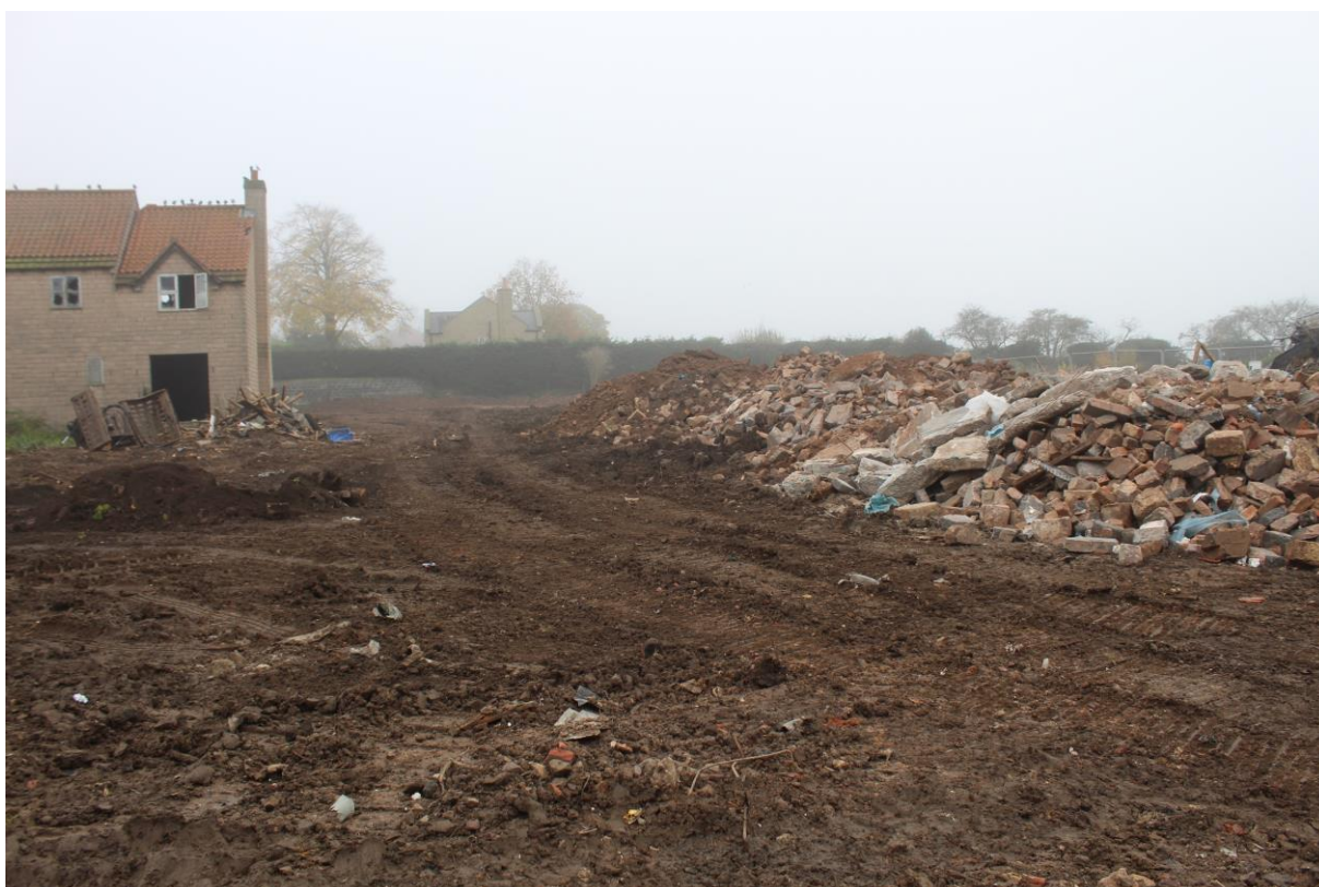
Plate 2: General View of Site, facing South.
