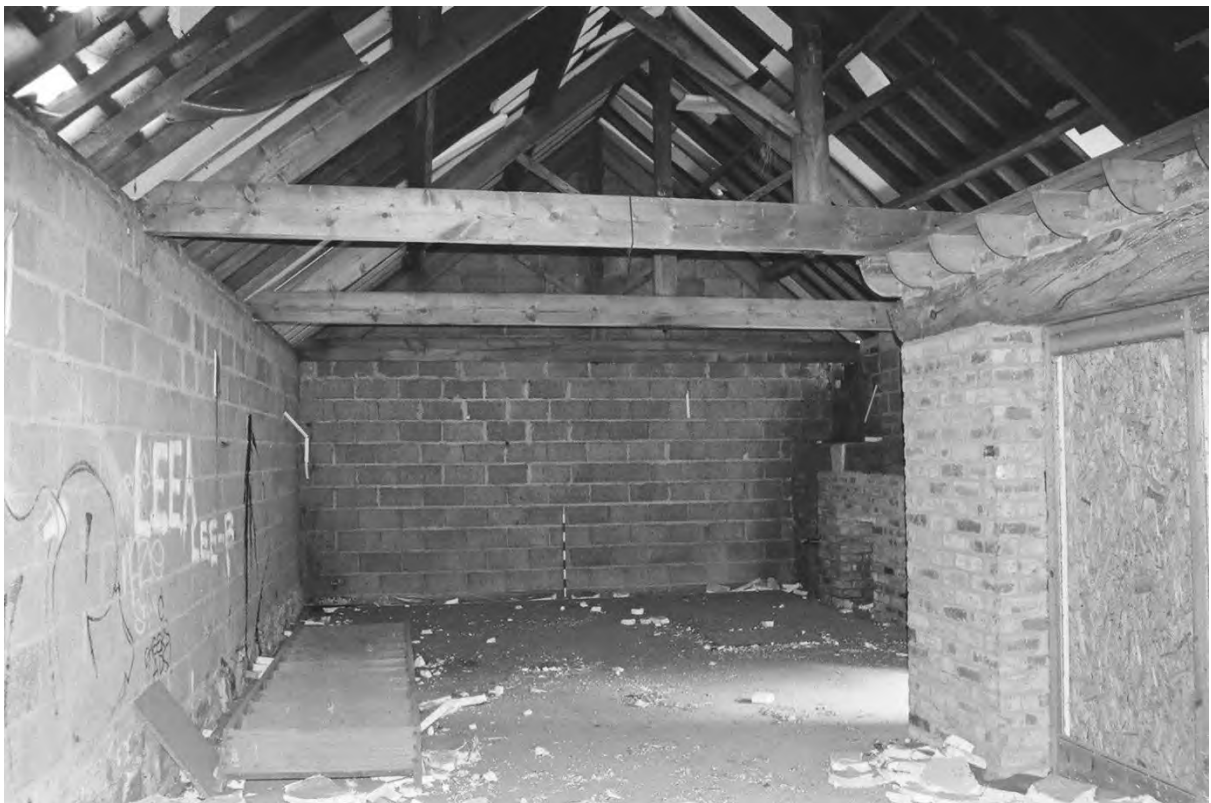
Plate 102. Farm Building 4: Room 4.1 Inserted Walls & Raised Roof (Film 1/7). Facing East.
