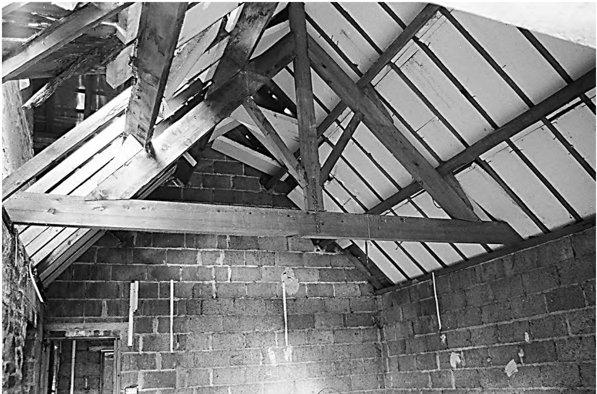
Plate 98. Farm Building 3: Room 3.2 Block walls & new Roof (Film 1/3). Facing North.
