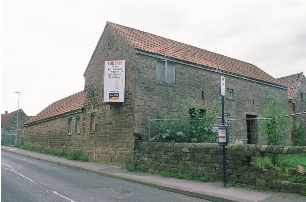
Plate 3. Farm Building 1: North & East Elevations (Film 5/21). Facing South-west.
