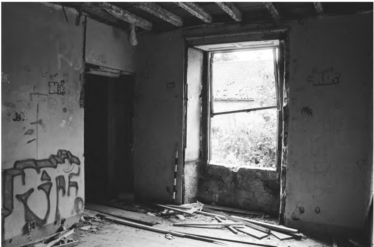
Plate 36. Farmhouse: Ground Floor Room 1 (Film 2/35). Facing South.
