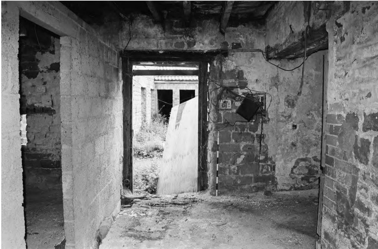
Plate 75. Farm Building 2: Ground Floor Room 2.2 Corridor (Film 2/10). Facing East.
