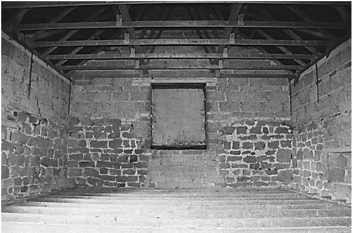
Plate 15. Farm Building 1 North: Room 1.3 Raised Roof (Film 2/5). Facing West.
