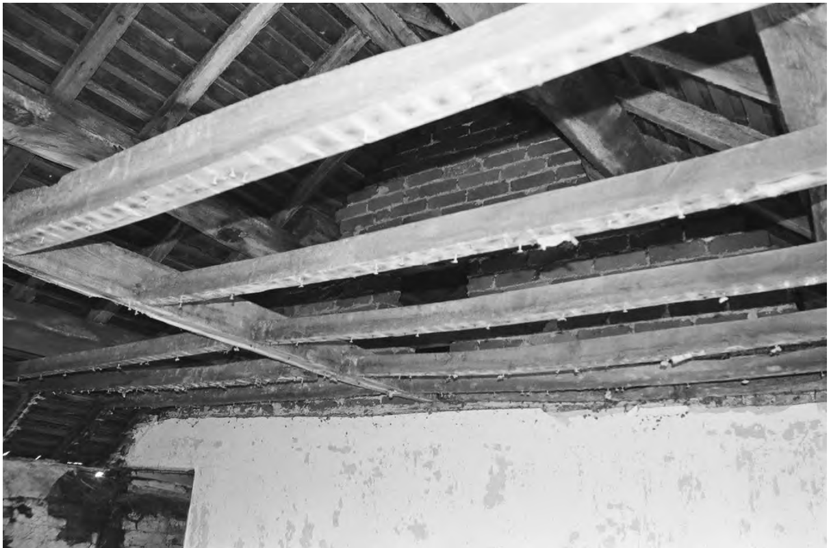
Plate 64. Farmhouse: Roof structure above Room 18 (Film 3/12). Facing West.
