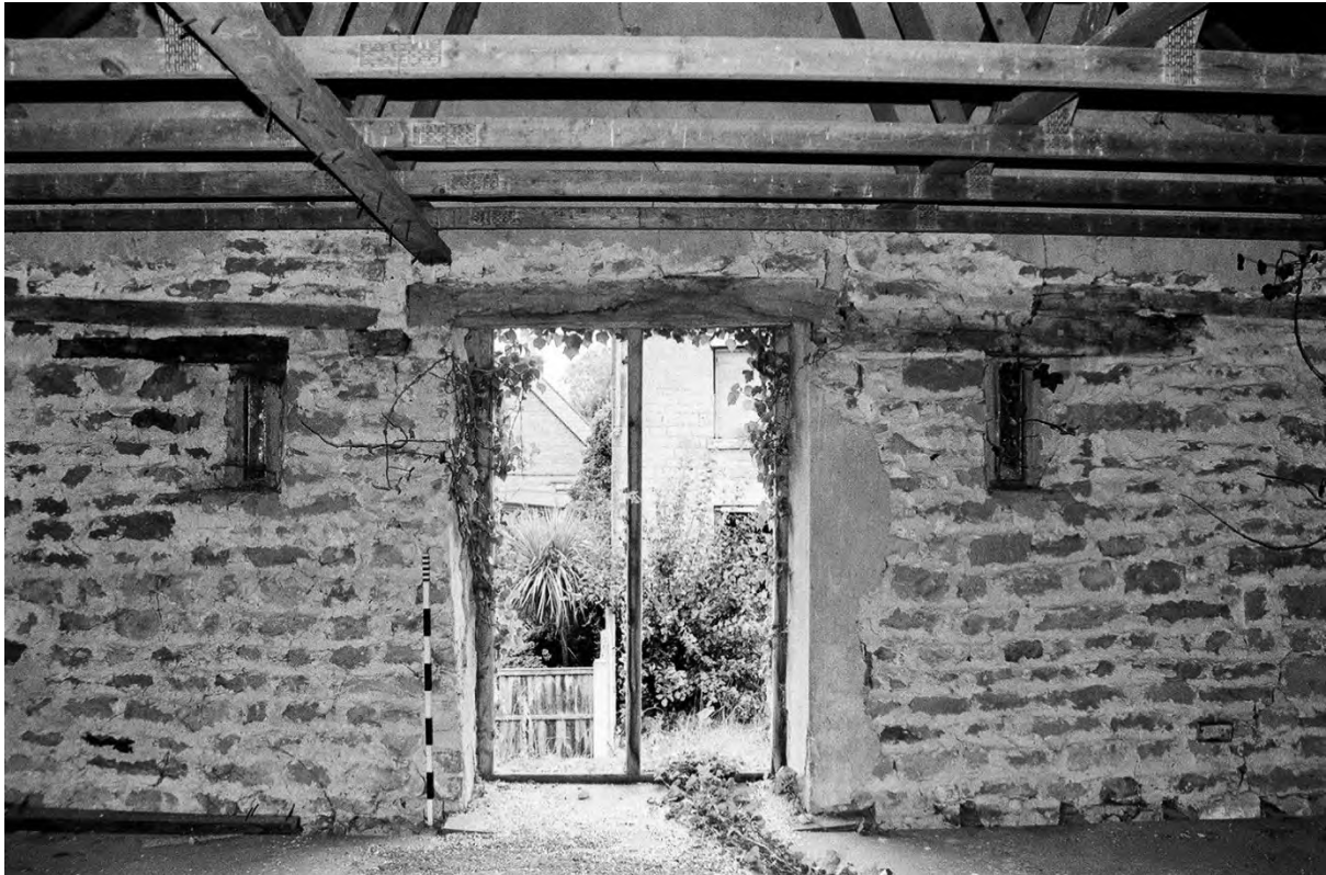
Plate 109. Farm Building 4: Room 4.7 Window & Ventilation Slits (Film 7/26). Facing North.
