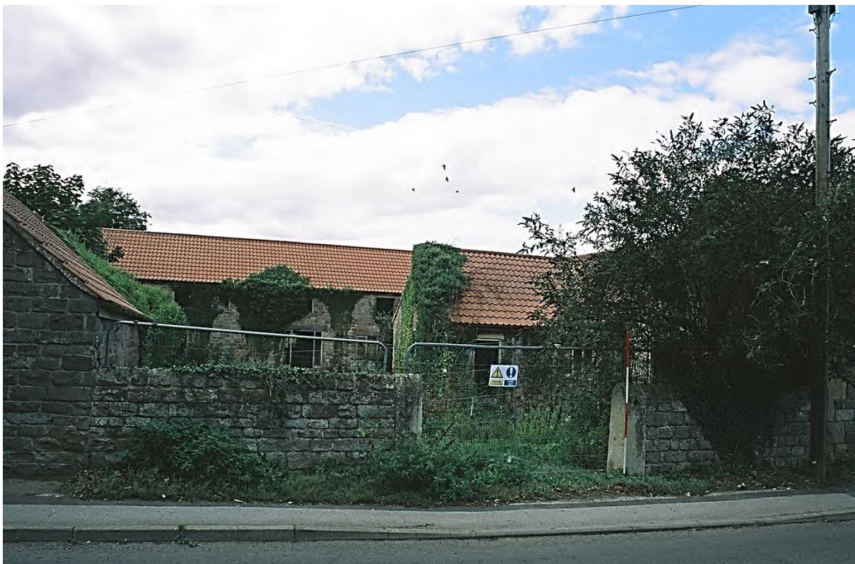
Plate 82. Farm Buildings 3, 4 & 5 from Hard Lane (Film 5/24). Facing West.
