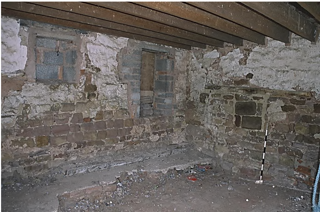
Plate 10. Farm Building 1 North: Ground Floor Room 1.1 (Film 6/24). Facing South-east.
