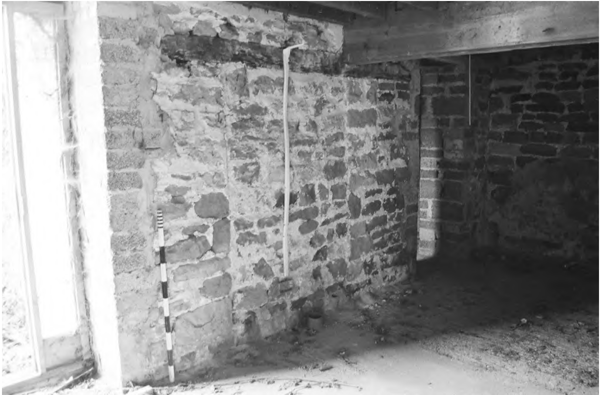
Plate 113. Farm Building 5: Room 5.5 Blocked Door (Film 1/16). Facing South-east.
