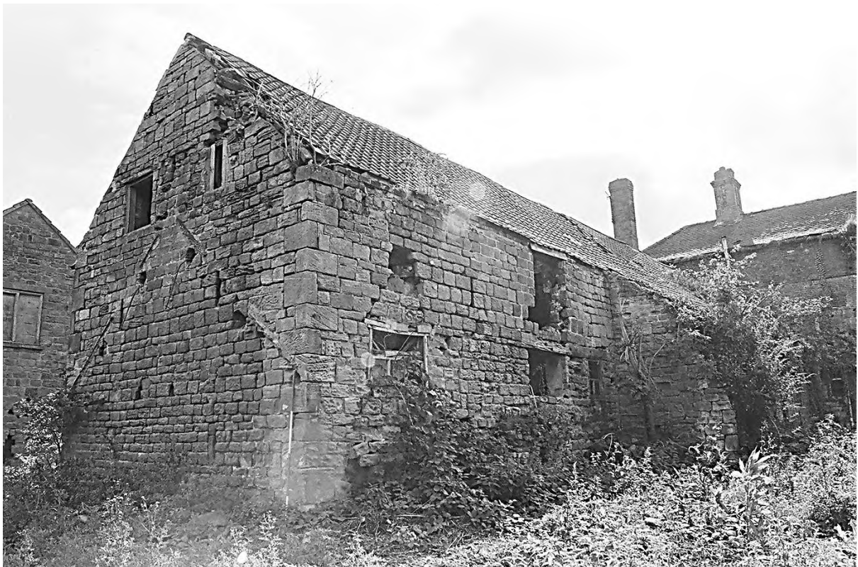
Plate 28. Farm Building 2: North & West Elevations (Film 3/35). Facing South-east.
