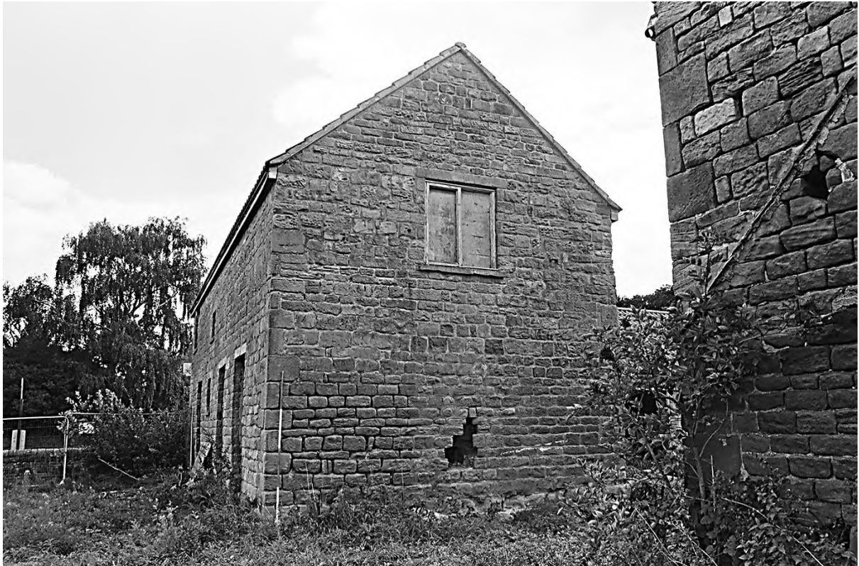
Plate 7. Farm Building 1: West Elevation (Film 3/22). Facing East.
