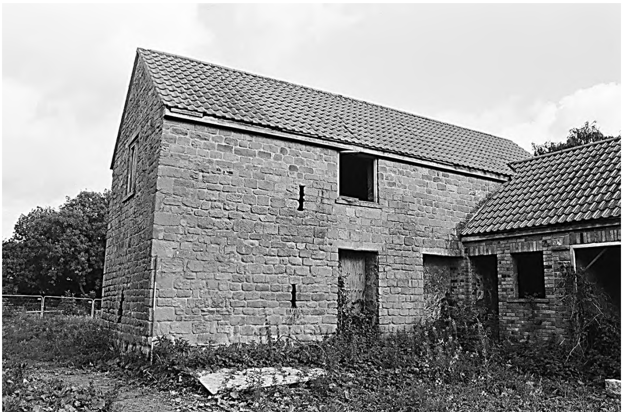
Plate 8. Farm Building 1 North: South Elevation (Film 3/31). Facing North-east.
