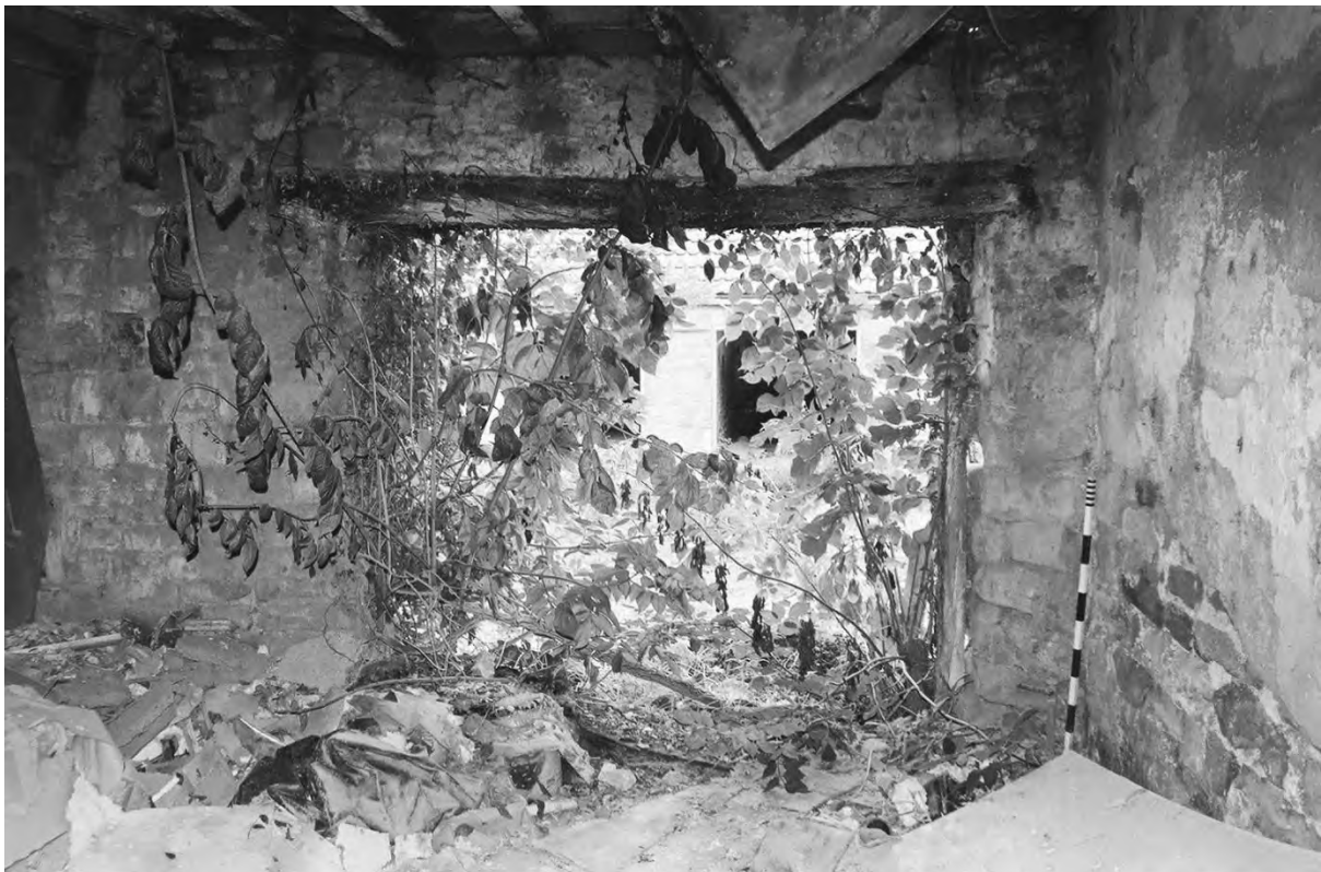
Plate 52. Farmhouse: Ground Floor Room 9 (Film 2/22). Facing East.
