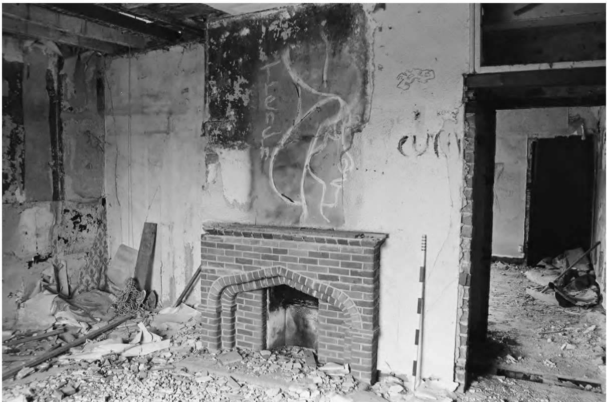
Plate 44. Farmhouse: Ground Floor Room 5 (Film 3/5). Facing West.
