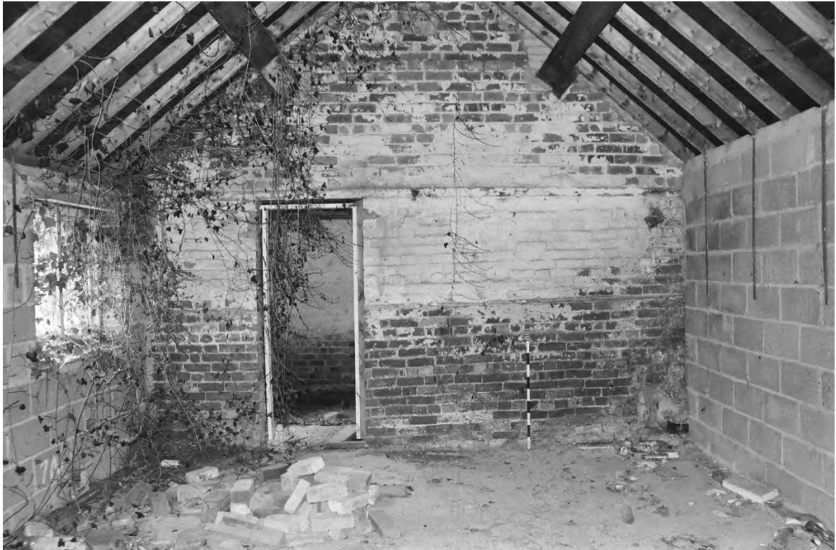
Plate 111. Farm Building 5: Room 5.3 Brick Partition Wall (Film 1/11). Facing East.
