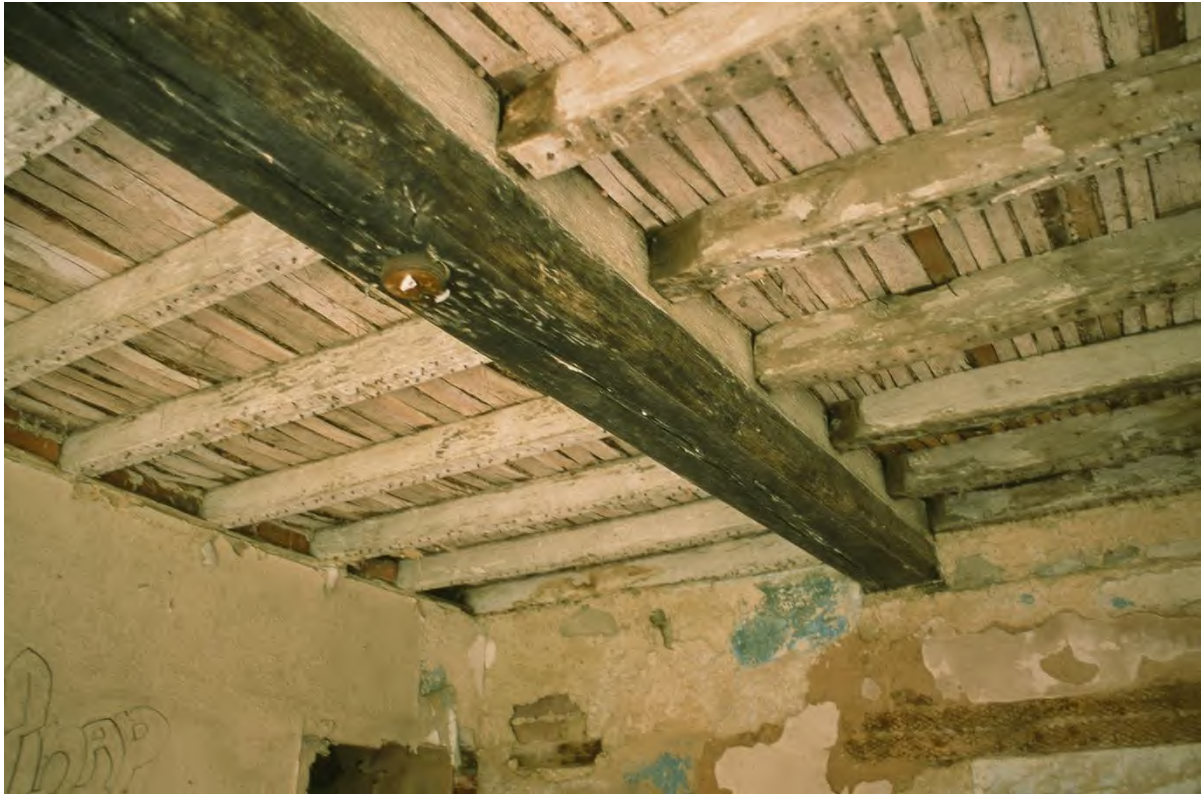
Plate 41. Farmhouse: Ground Floor Room 4 Beam (Film 5/28). Facing North.
