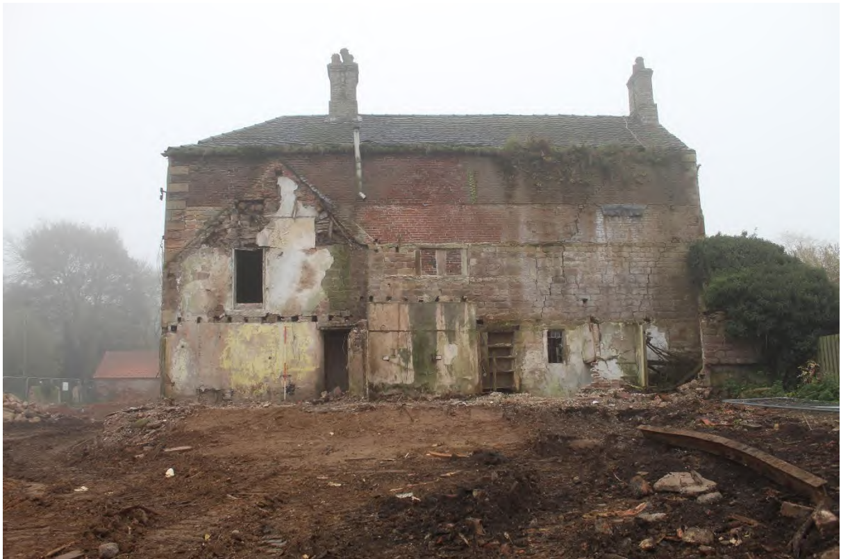
Plate 30. Farmhouse: North Elevation after partial demolition (IMG_0097). Facing South.
