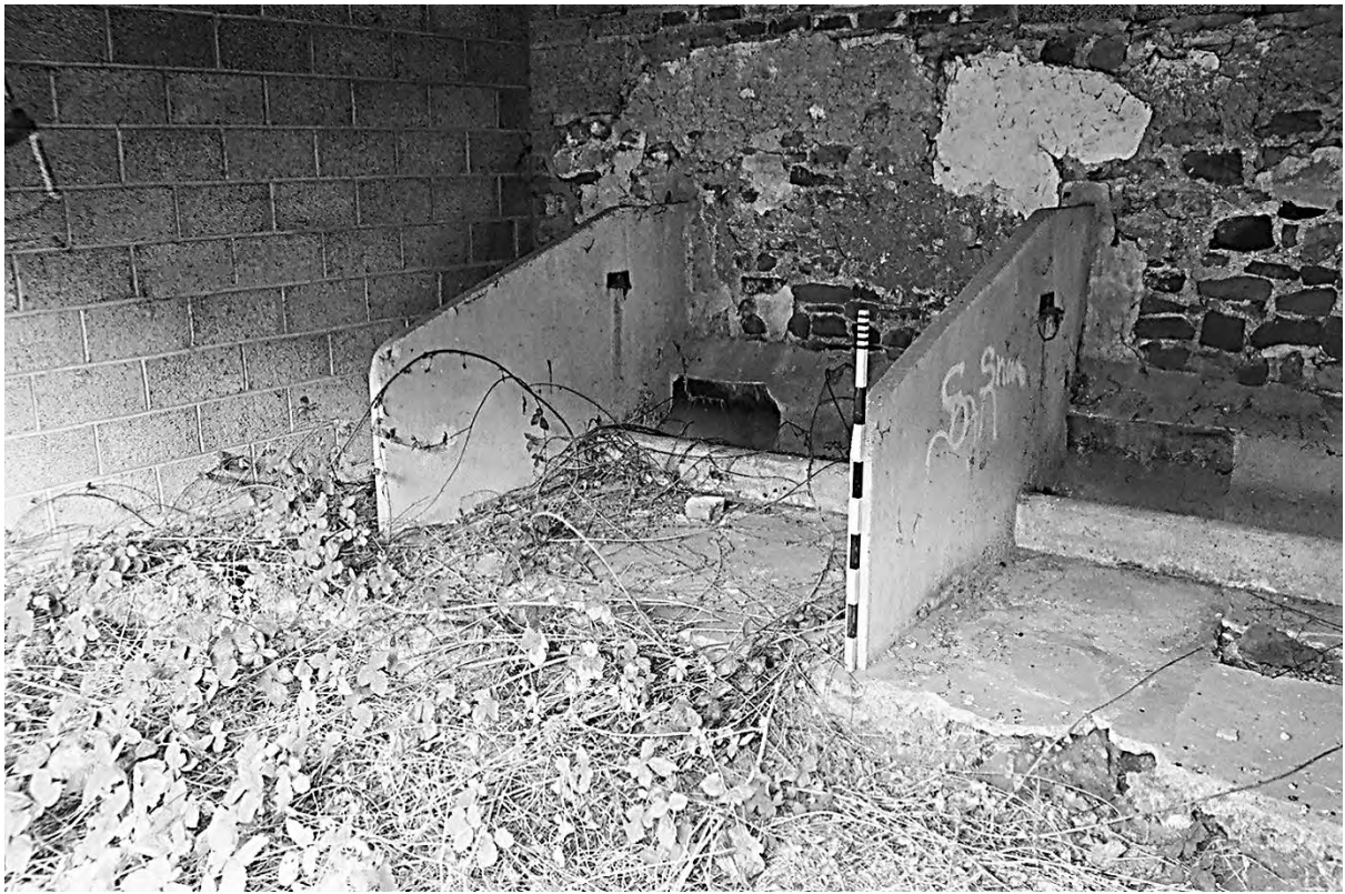
Plate 19. Farm Building 1 South: Room 1.5 Stalls & Mangers (Film 1/30). Facing North-east.
