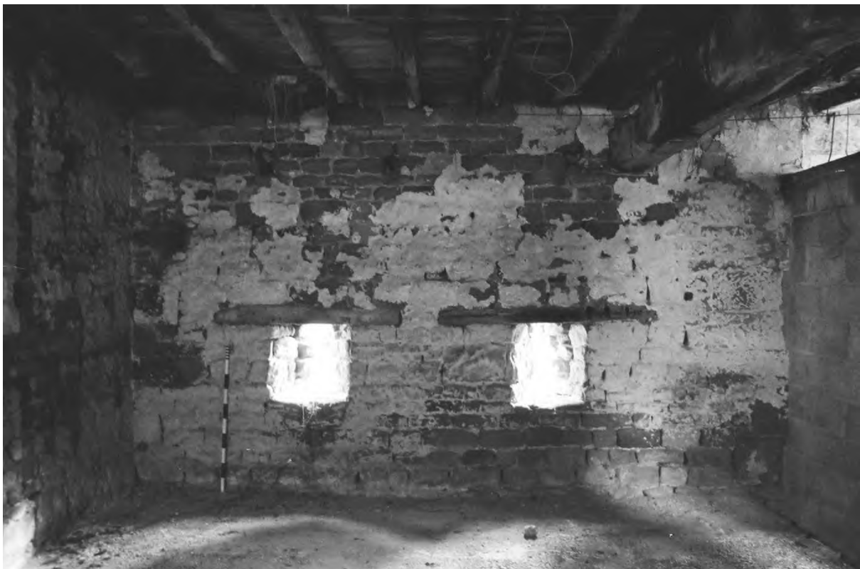
Plate 78. Farm Building 2: Ground Floor Rom 2.2 (Film 2/13). Facing East.
