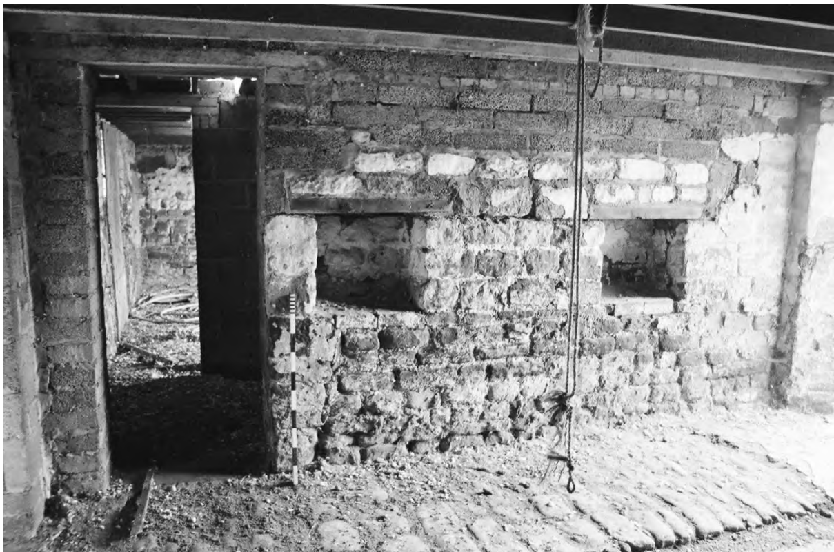
Plate 12. Farm Building 1 North: Ground Floor Room 1.1 Niches (Film 1/34). Facing West.
