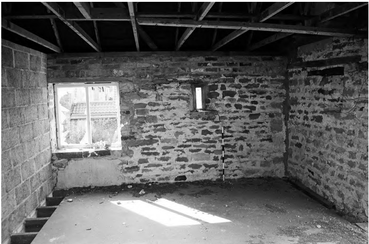
Plate 108. Farm Building 4: Room 4.7 Raised Roof (Film 1/26). Facing West.
