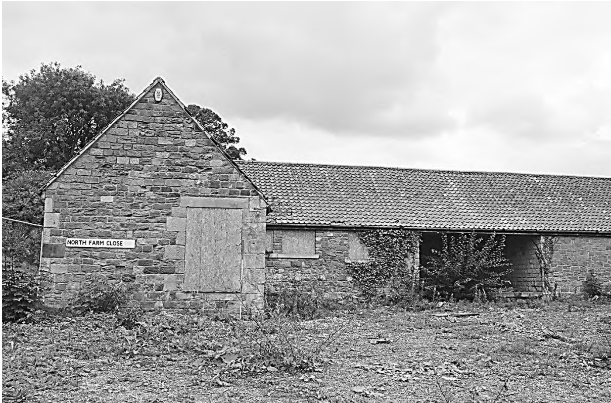
Plate 85. Farm Building 3: North Elevation (Film 4/18), Facing South.
