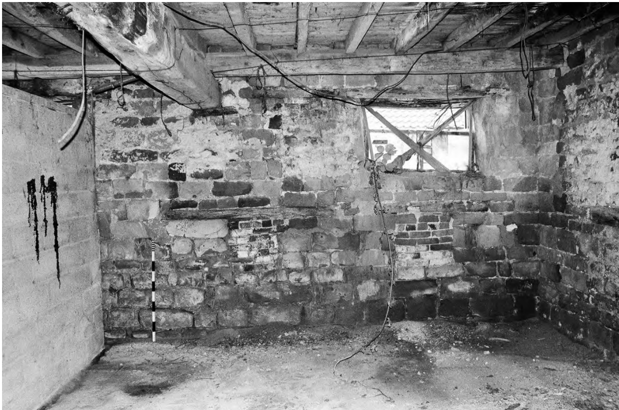
Plate 76. Farm Building 2: Ground Floor Room 2.2 (Film 7/28). Facing West.
