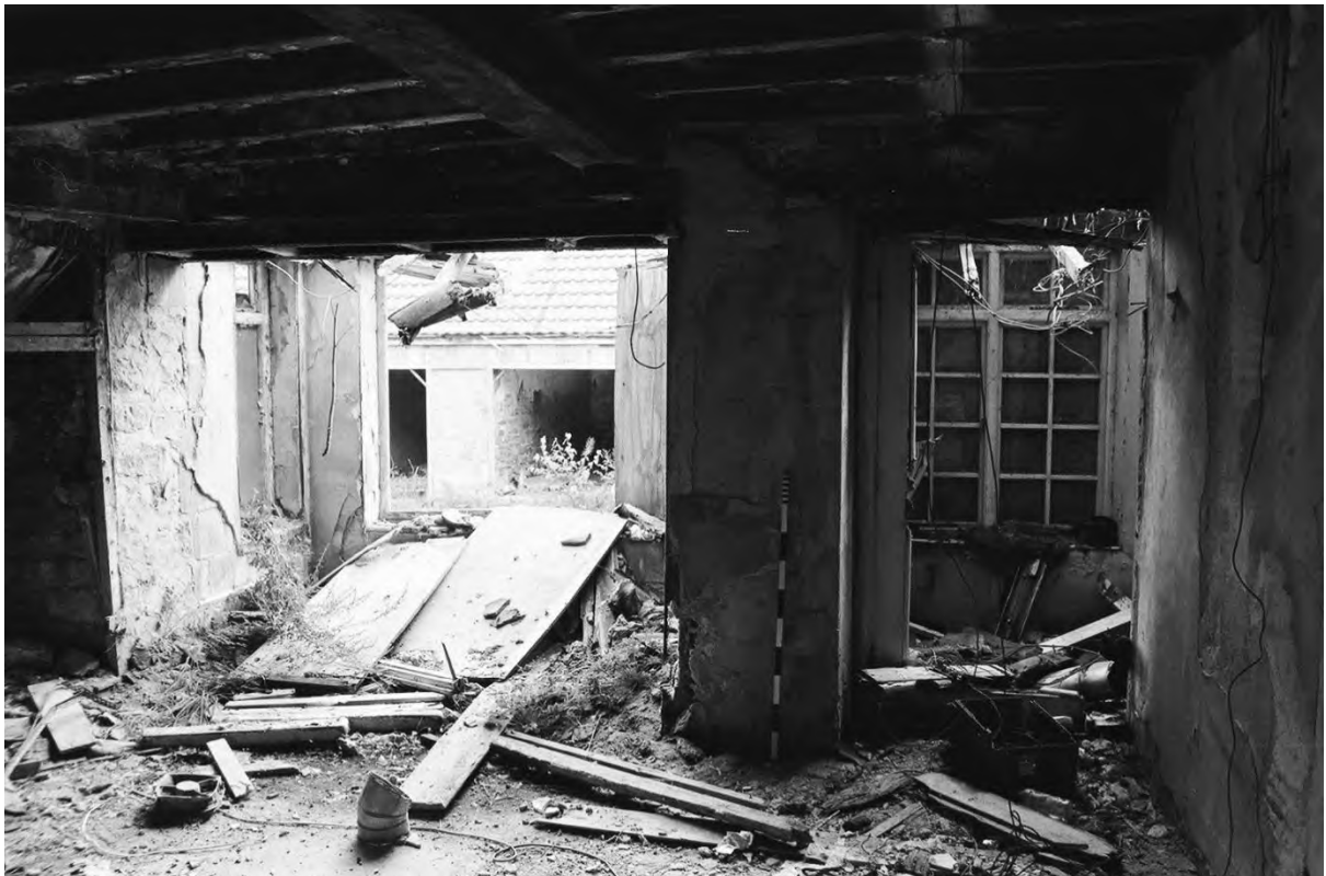
Plate 48. Farmhouse: Ground Floor Room 6 (Film 2/26). Facing East.
