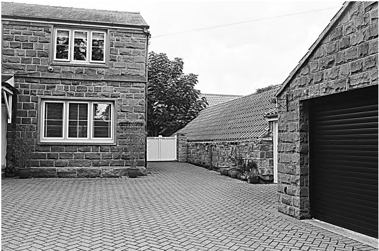
Plate 94. Farm Building 5: South Elevation (Film 3/27). Facing West.
