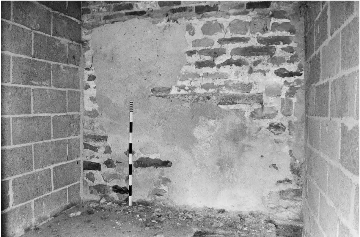
Plate 107. Farm Building 4: Room 4.6 Raised Roof & Lintel (Film 7/23). Facing East.
