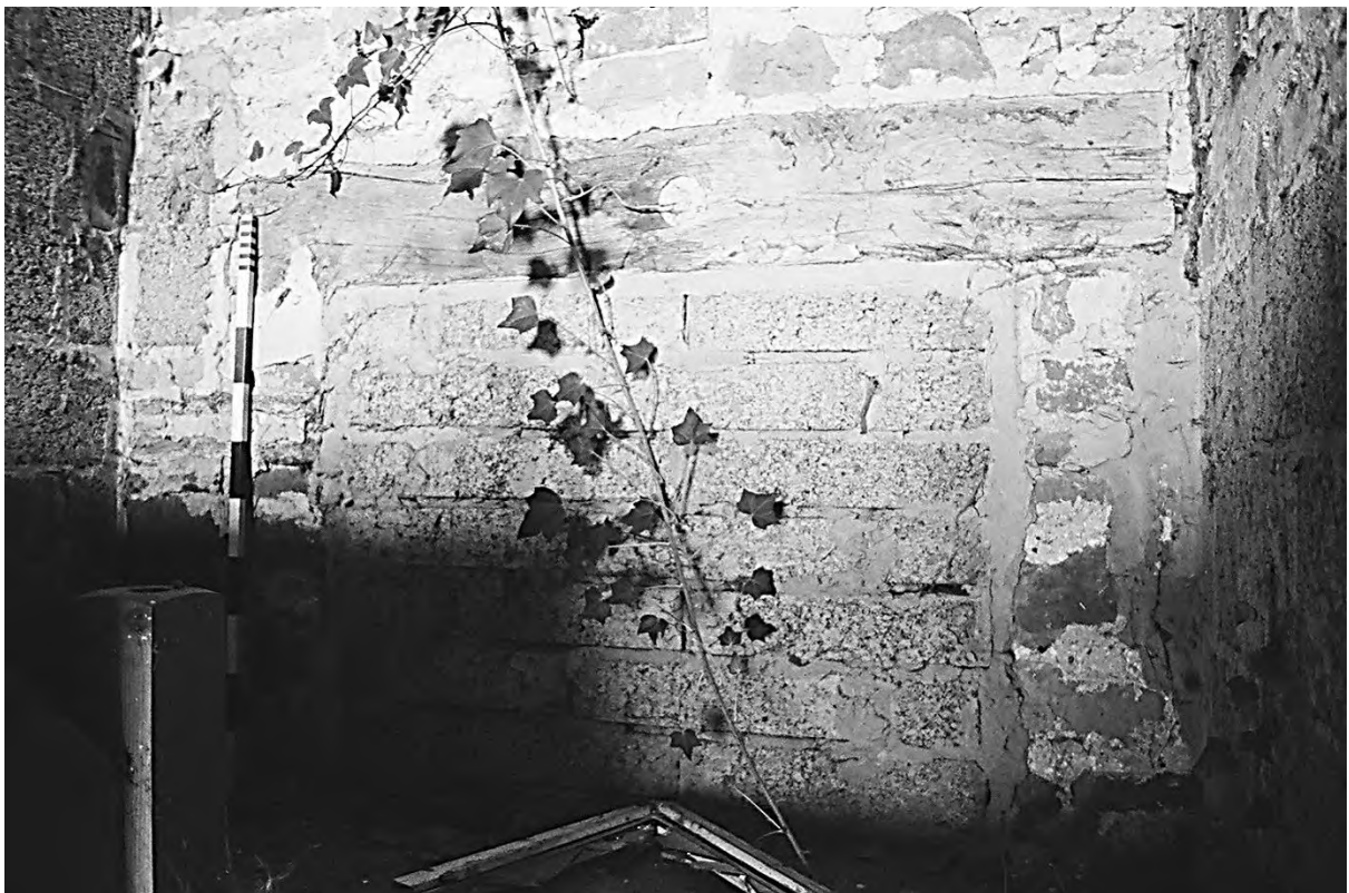
Plate 116. Farm Building 5. Room 5.5/5.8 Blocked Window (Film 1/14). Facing East.
