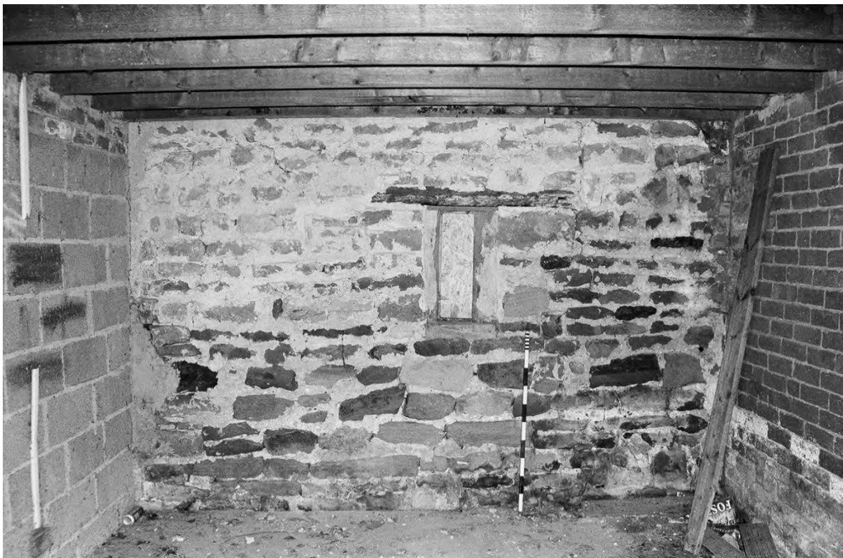
Plate 106. Farm Building 4: Room 4.4 Ground Floor Window (Film 7/18). Facing West.
