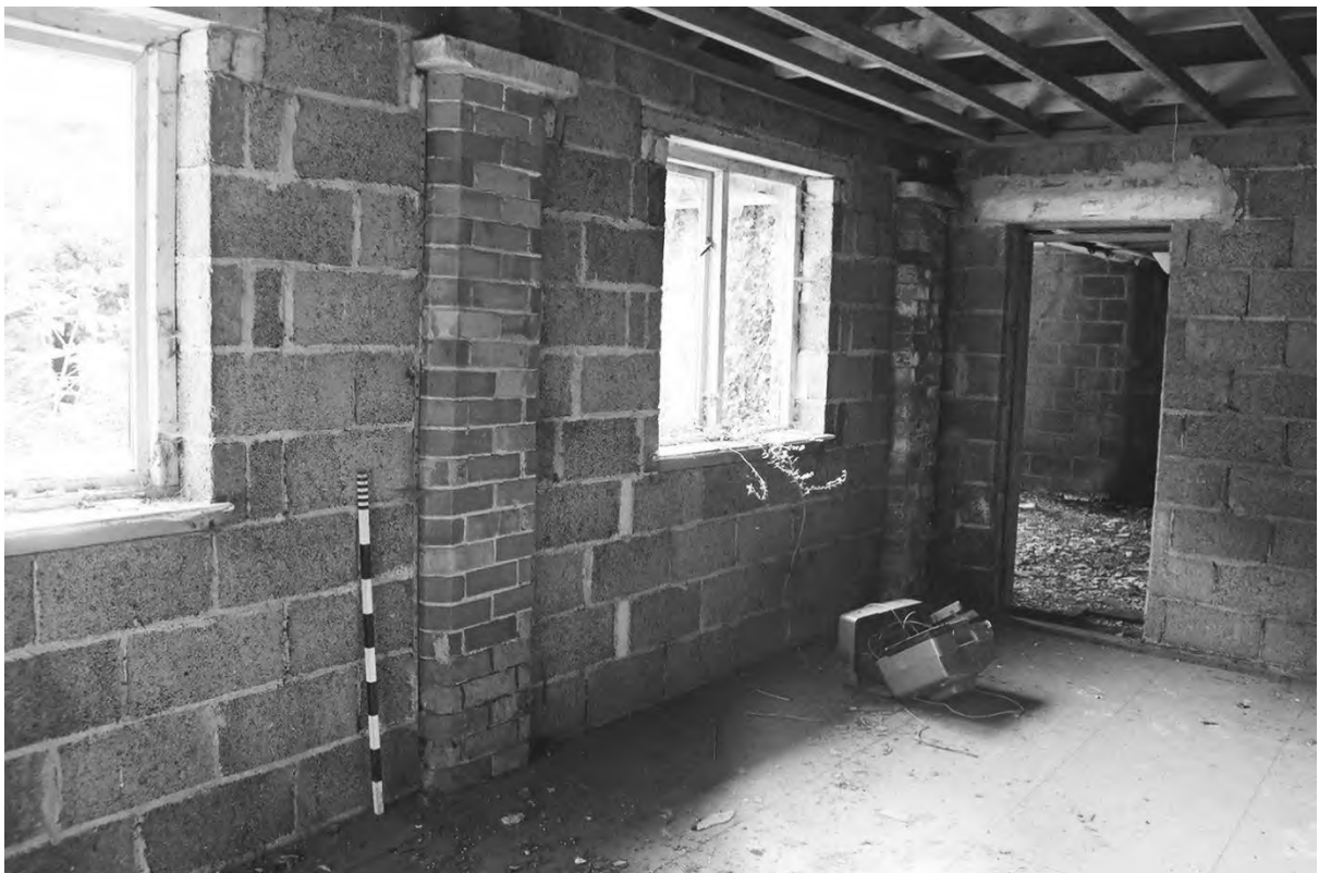
Plate 100. Farm Building 3: Room 3.2 Shelter Shed Brick Pier (Film 1/6). Facing West.
