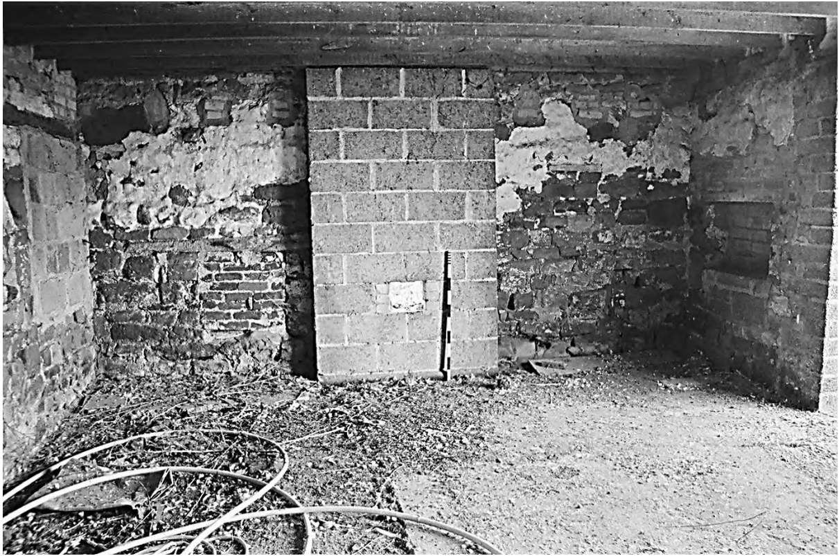
Plate 12. Farm Building 1 North: Ground Floor Room 1.2 (Film 2/2). Facing West.
