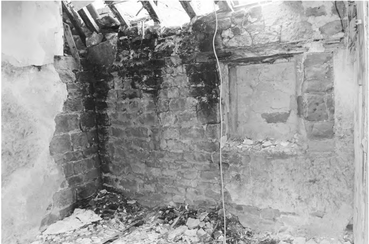
Plate 57. Farmhouse: First Floor Room 14 (Film 2/30). Facing West.
