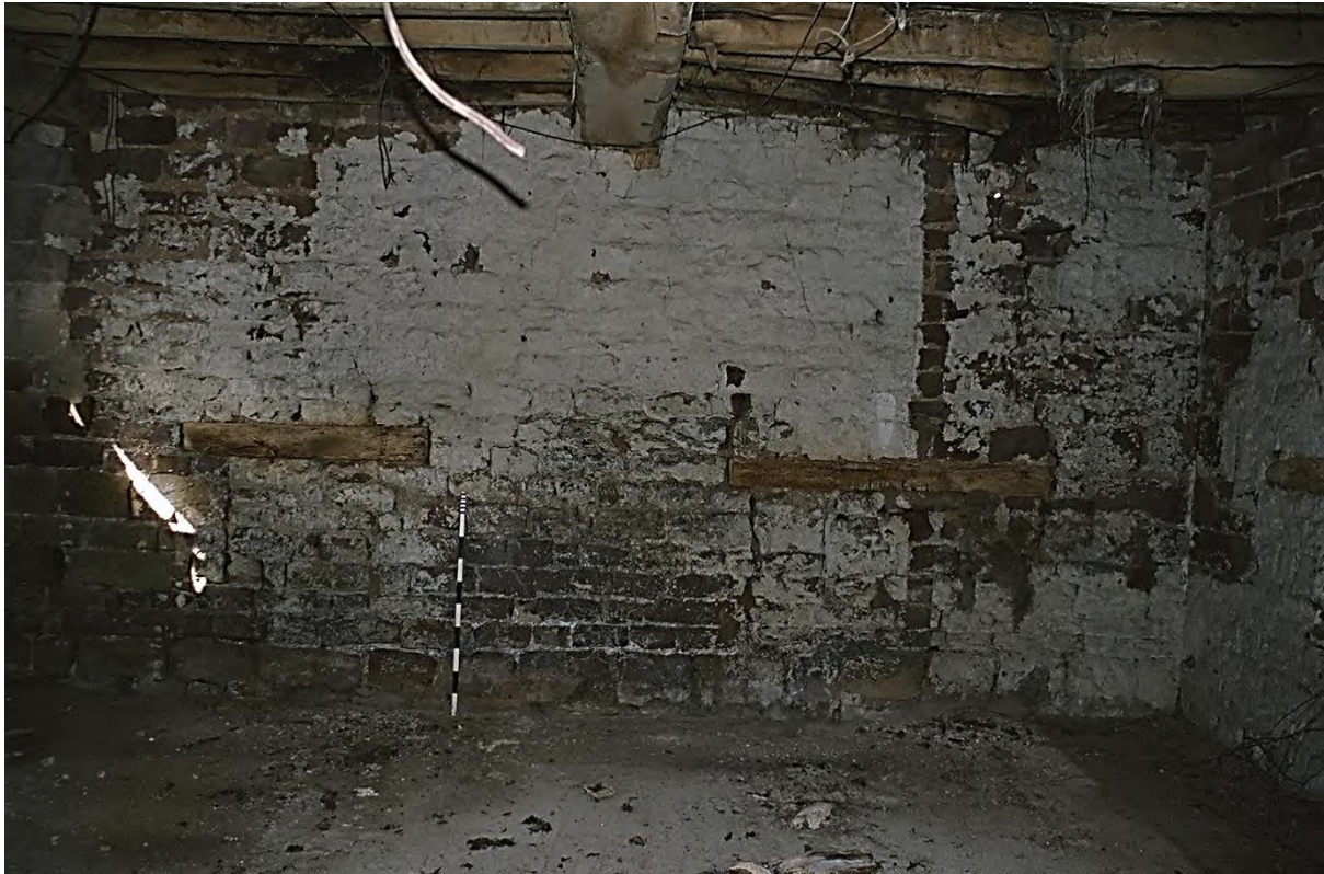
Plate 77. Farm Building 2: Ground Floor Room 2.2 (Film 6/20). Facing North.
