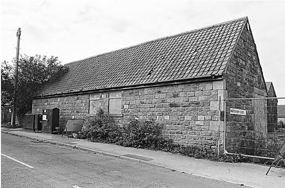
Plate 83. Farm Building 3: North & East Elevations (Film 3/25). Facing South-west.
