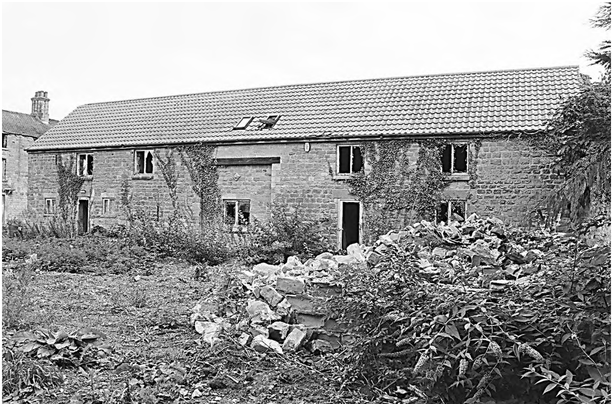
Plate 90. Farm Buildings 4 & 5: West Elevation (Film 4/24). Facing North-east.
