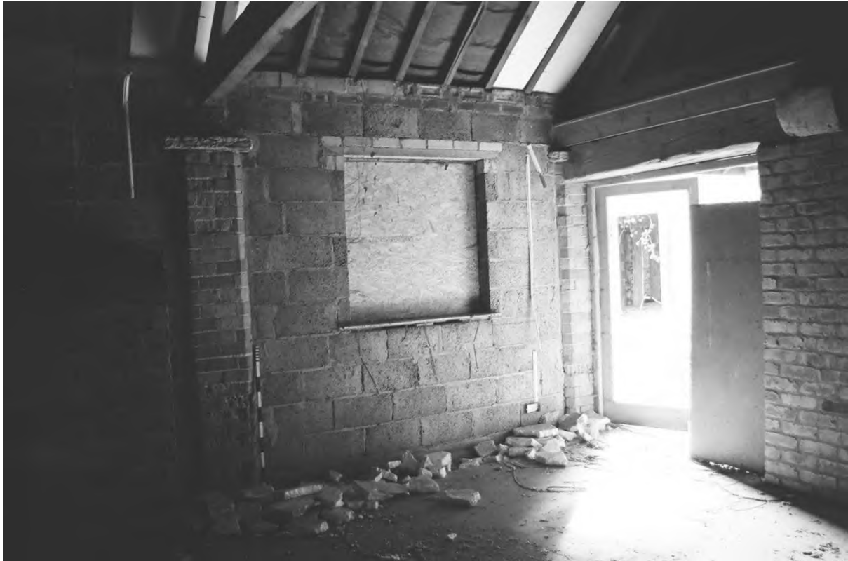
Plate 103. Farm Building 4: Room 4.1 Raised Roof (Film 1/18), Facing South.
