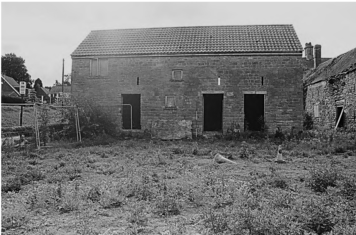
Plate 6. Farm Building 1: North Elevation (Film 3/33). Facing South.
