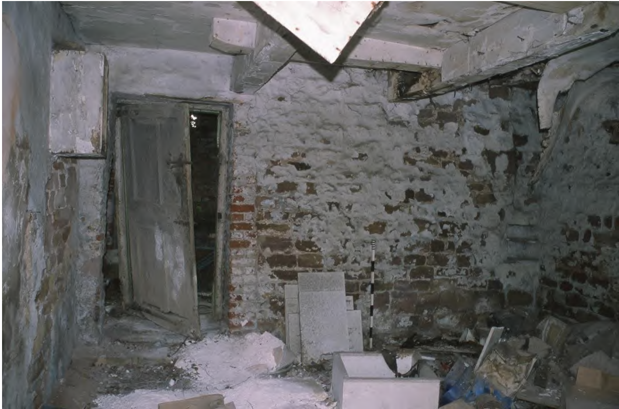
Plate 51. Farmhouse: Ground Floor Room 9 access from West Extension (Film 6/16). Facing West.
