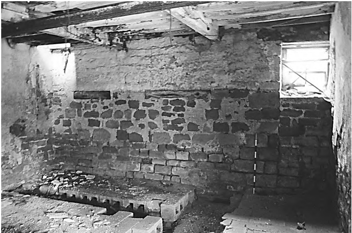
Plate 72. Farm Building 2: Ground Floor Room 2.1 (Film 2/8). Facing West.
