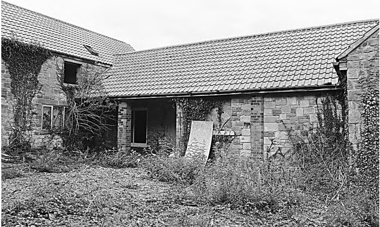
Plate 91. Farm Building 4: South & East Elevations (Film 4/25). Facing North-west.
