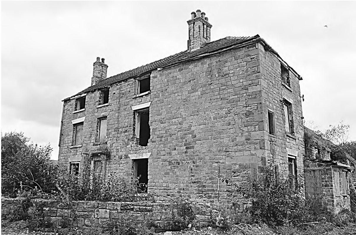
Plate 23. Farmhouse: South & East Elevations (Film 4/8). Facing North-west.
