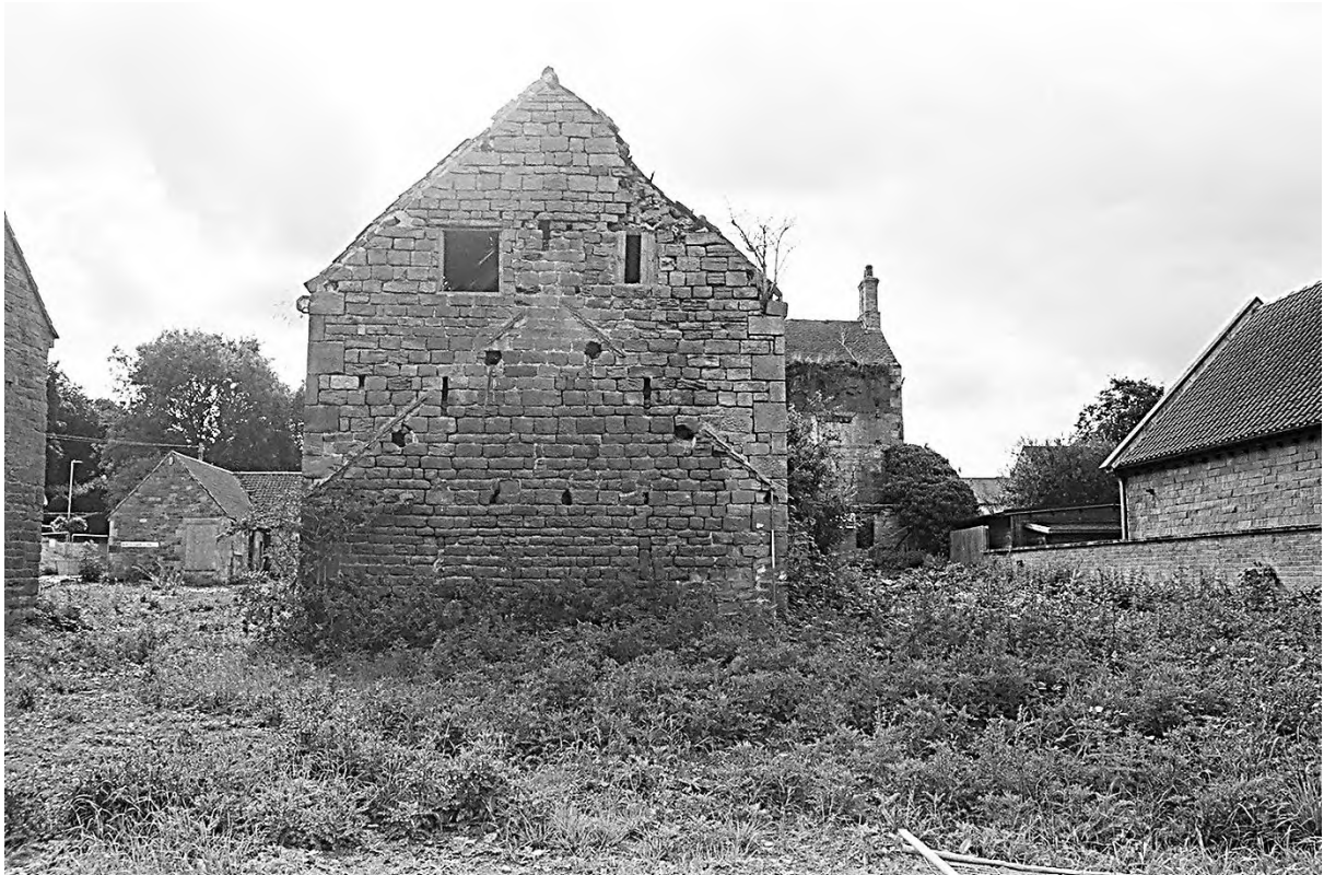
Plate 27. Farm Building 2: North Elevation (Film 3/34). Facing South.
