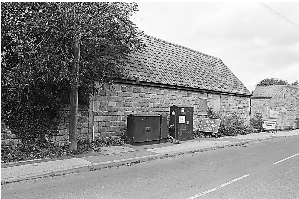
Plate 84. Farm Building 3: East Elevation (Film 3/26). Facing North-west.
