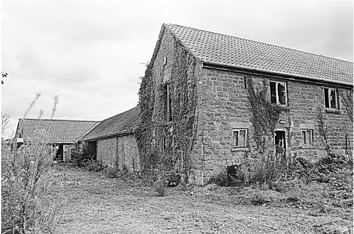
Plate 89. Farm Buildings 3 & 4: North & West Elevations (Film 4/21). Facing South-east.
