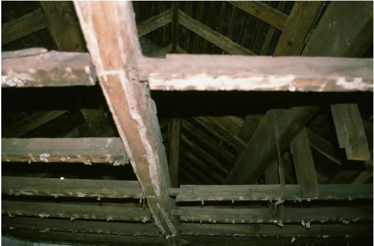
Plate 67. Farmhouse: Roof structure above Room 19 (Film 6/11). Facing West.
