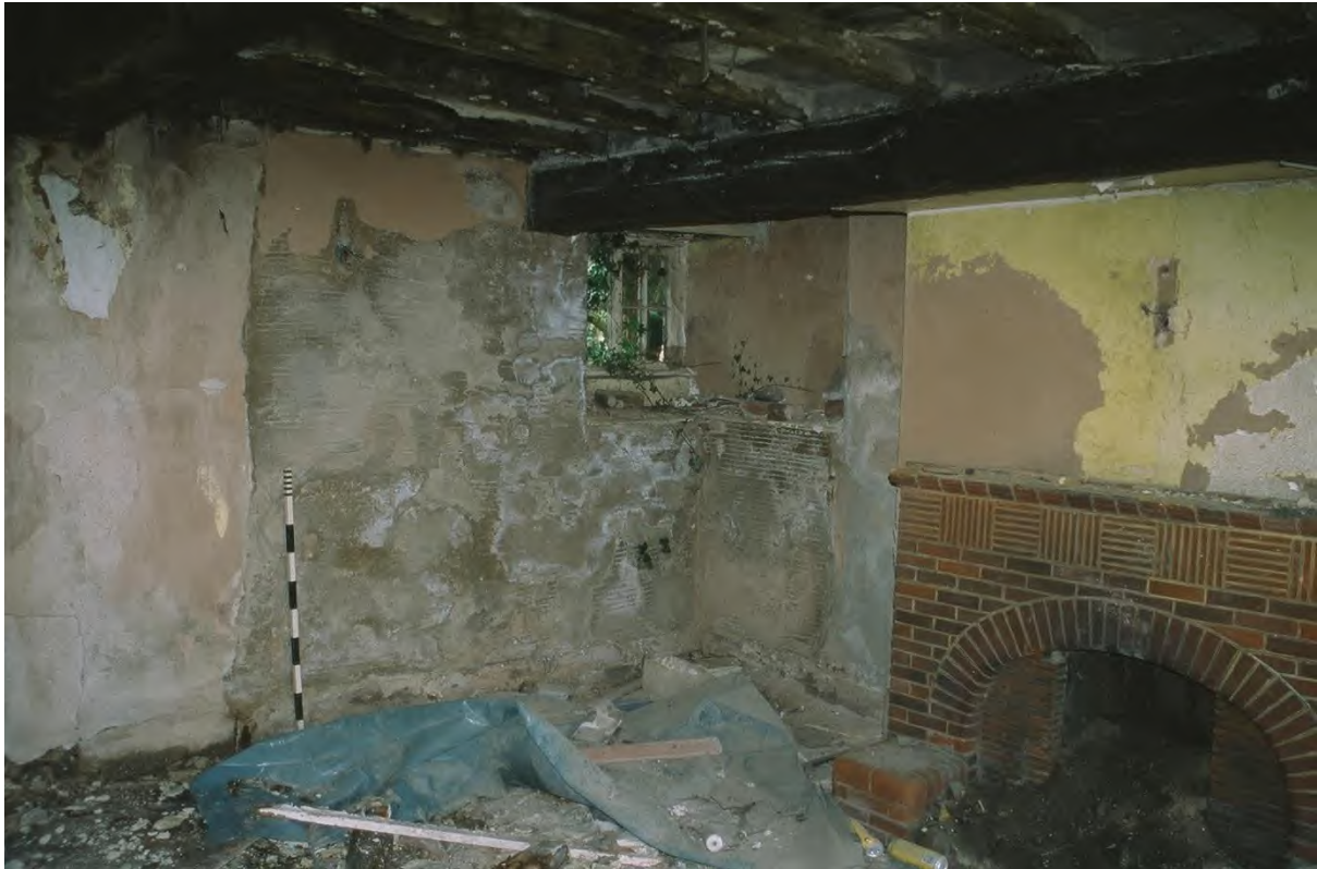
Plate 45. Farmhouse: Ground Floor North Room 6 (Film 5/36). Facing North-west.
