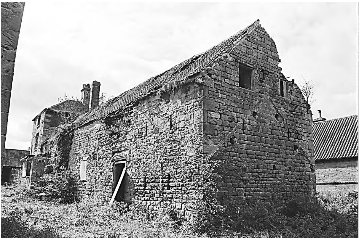
Plate 26. Farm Building 2: East & North Elevations (Film 3/36). Facing South-west.
