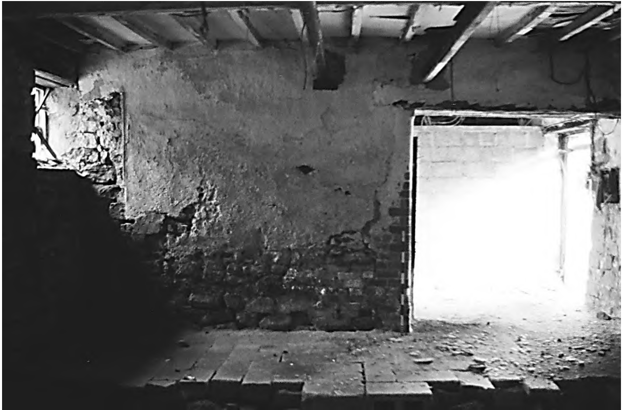
Plate 71. Farm Building 2: Ground Floor Room 2.1 (Film 2/7). Facing North.
