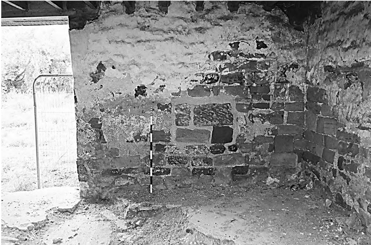
Plate 11. Farm Building 1 North: Ground Floor Room 1.1 (Film 1/36). Facing North.
