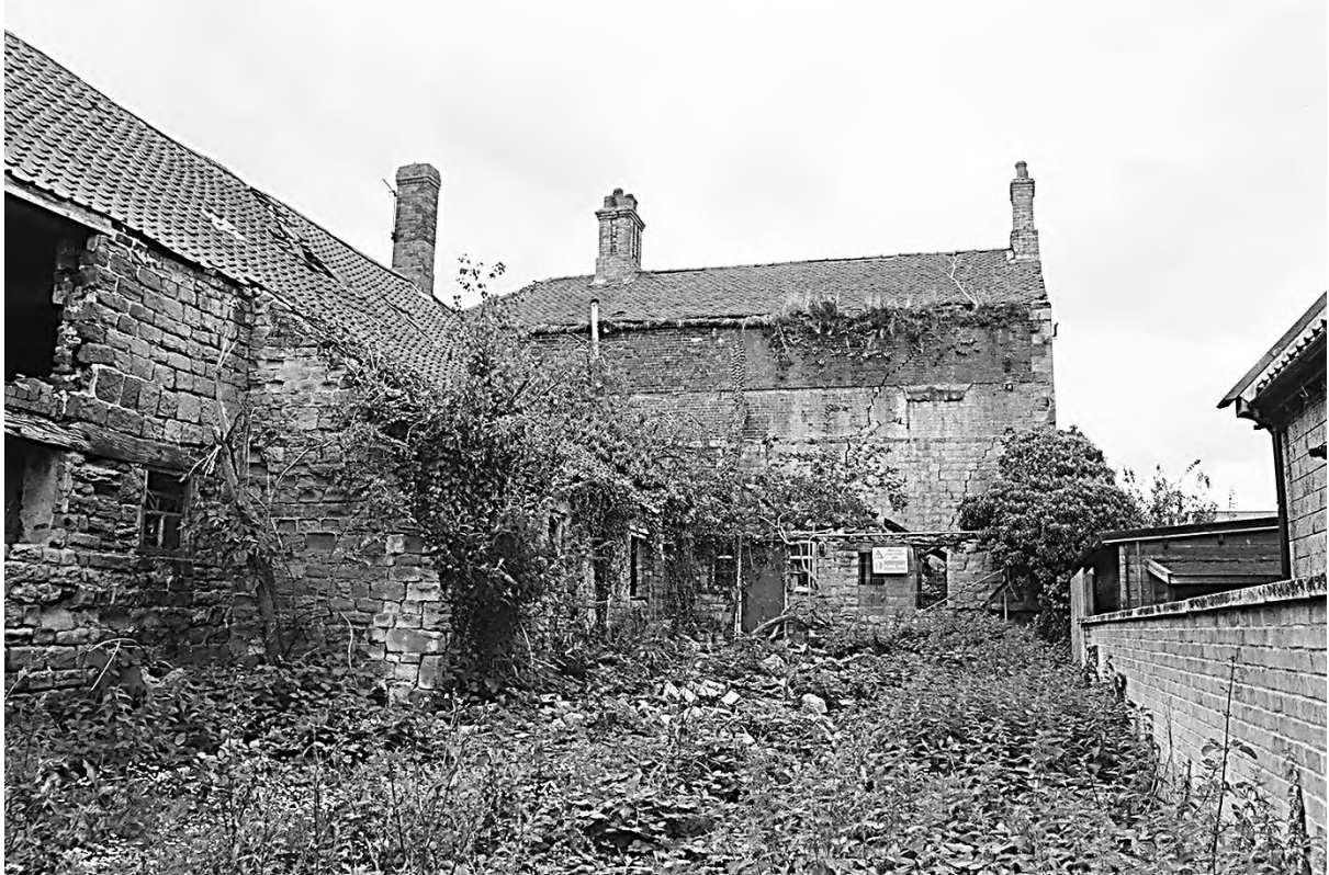
Plate 29. Farmhouse: South Elevation (Film 4/13). Facing South.
