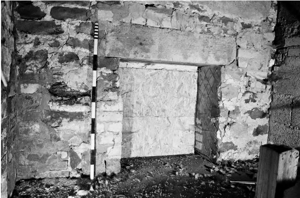
Plate 105. Farm Building 4: Room 4.3 Landing Inserted Window (Film 7/20). Facing West.
