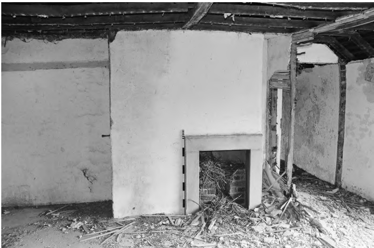
Plate 66. Farmhouse; Second Floor Room 19 (Film 3/15). Facing East.
