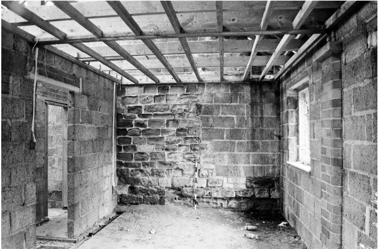
Plate 99. Farm Building 3: Room 3.2 Blocked Window (Film 7/11). Facing East.
