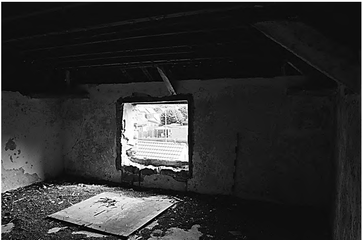
Plate 68. Farmhouse: Second Floor Room 20 (Film 3/18). Facing East.
