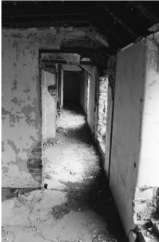
Plate 65. Farmhouse Second Floor Room 17 from Room 18 (Film 3/11) Facing East.
