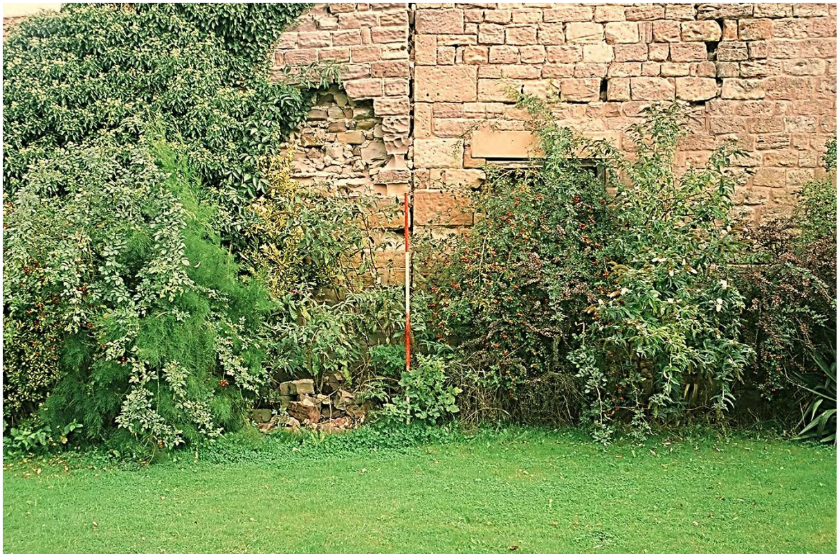
Plate 32. Farmhouse: East Elevation Exterior Door (Film 5/02). Facing East.
