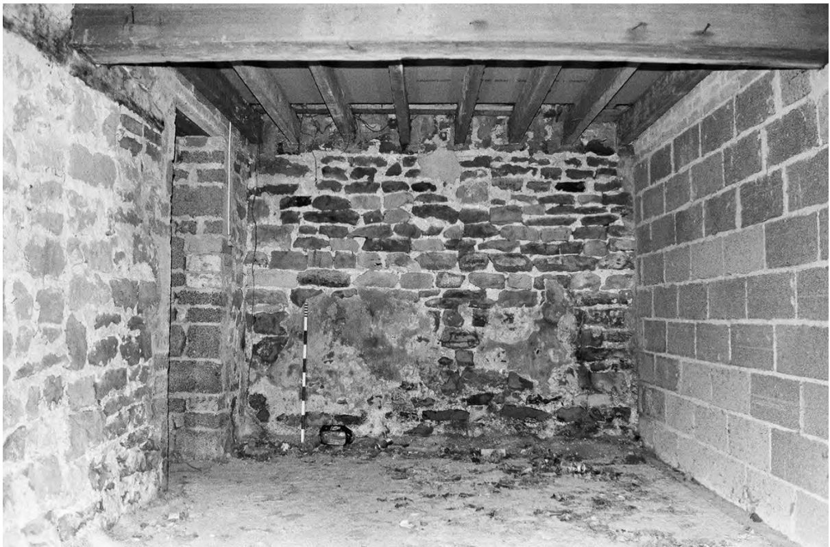
Plate 114. Farm Building 5: Room 5.5 Plaster (Film 7/7). Facing South.
