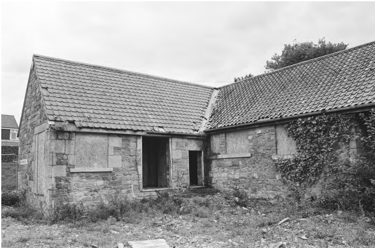
Plate 86. Farm Building 3: North & West Elevations (Film 4/20). Facing South-east.
