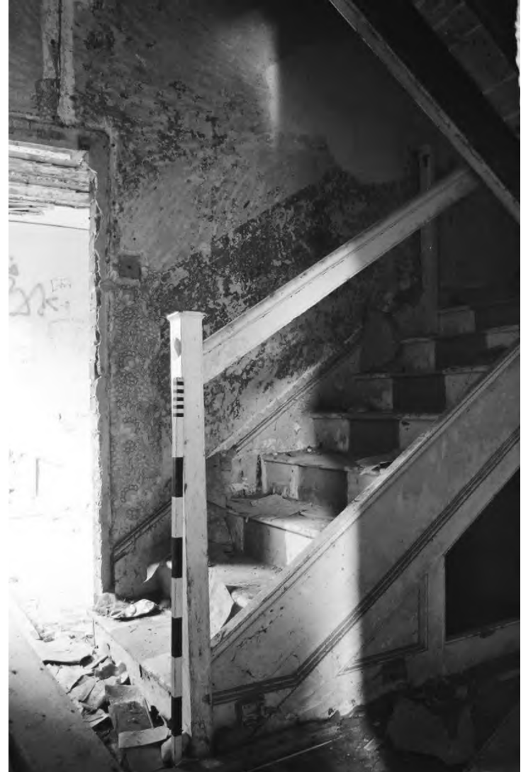
Plate 38. Farmhouse: Ground Floor Room 23 (Film 2/32). Facing West.
