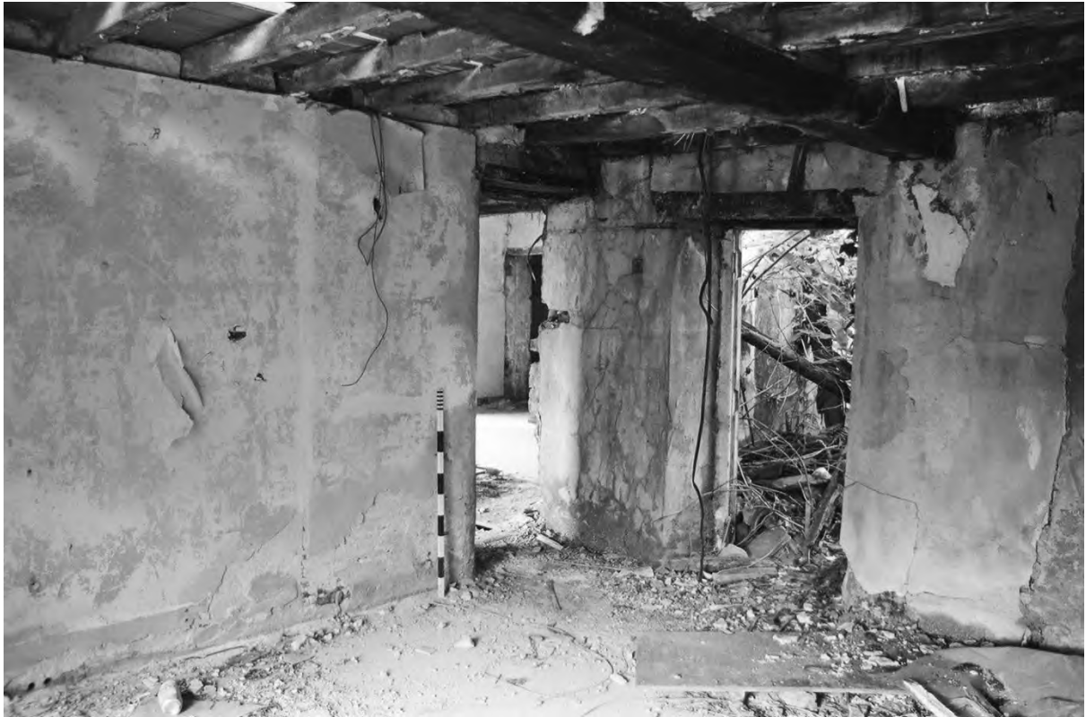
Plate 47. Farmhouse: Ground Floor Room 6 (Film 2/25). Facing South-west.
