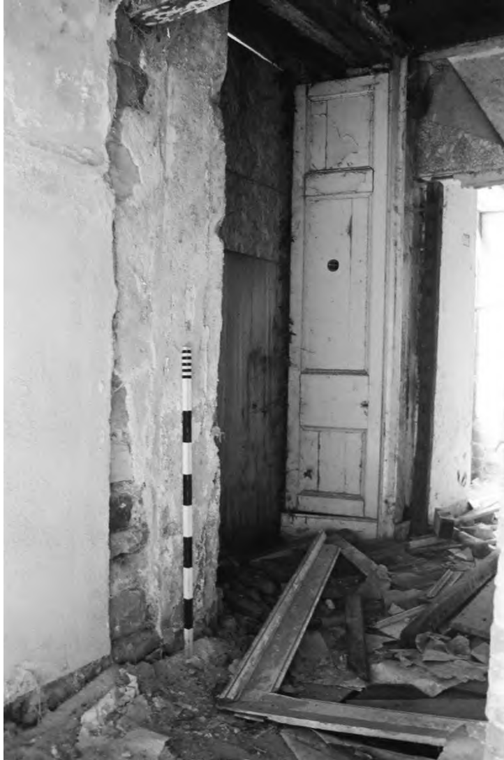
Plate 37. Farmhouse: Ground Floor Room 2 (Film 2/31), Facing West.
