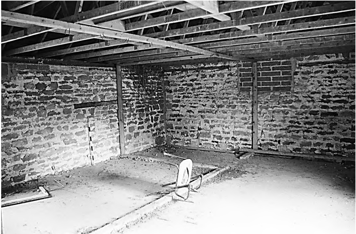
Plate 117. Farm Building 5: Room 5.8 Blocked Window & Slit (Film 1/12). Facing South-east.
