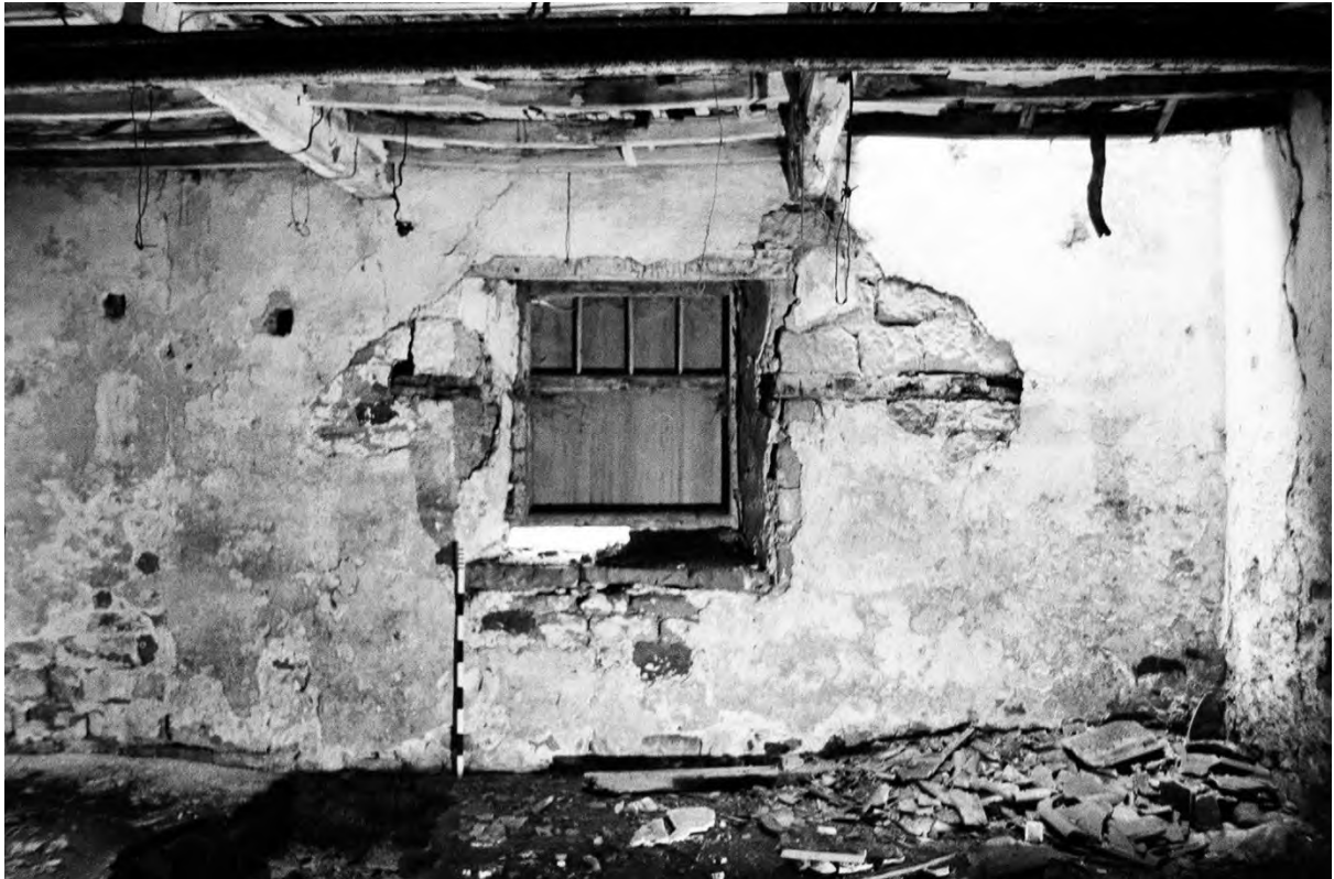
Plate 73. Farm Building 2: Ground Floor Room 2.1 (Film 7/32). Facing East.
