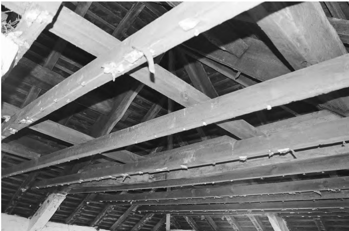
Plate 70. Farmhouse: Second Floor Hipped Roof Truss above Room 20 (Film 3/19). Facing North-east.
