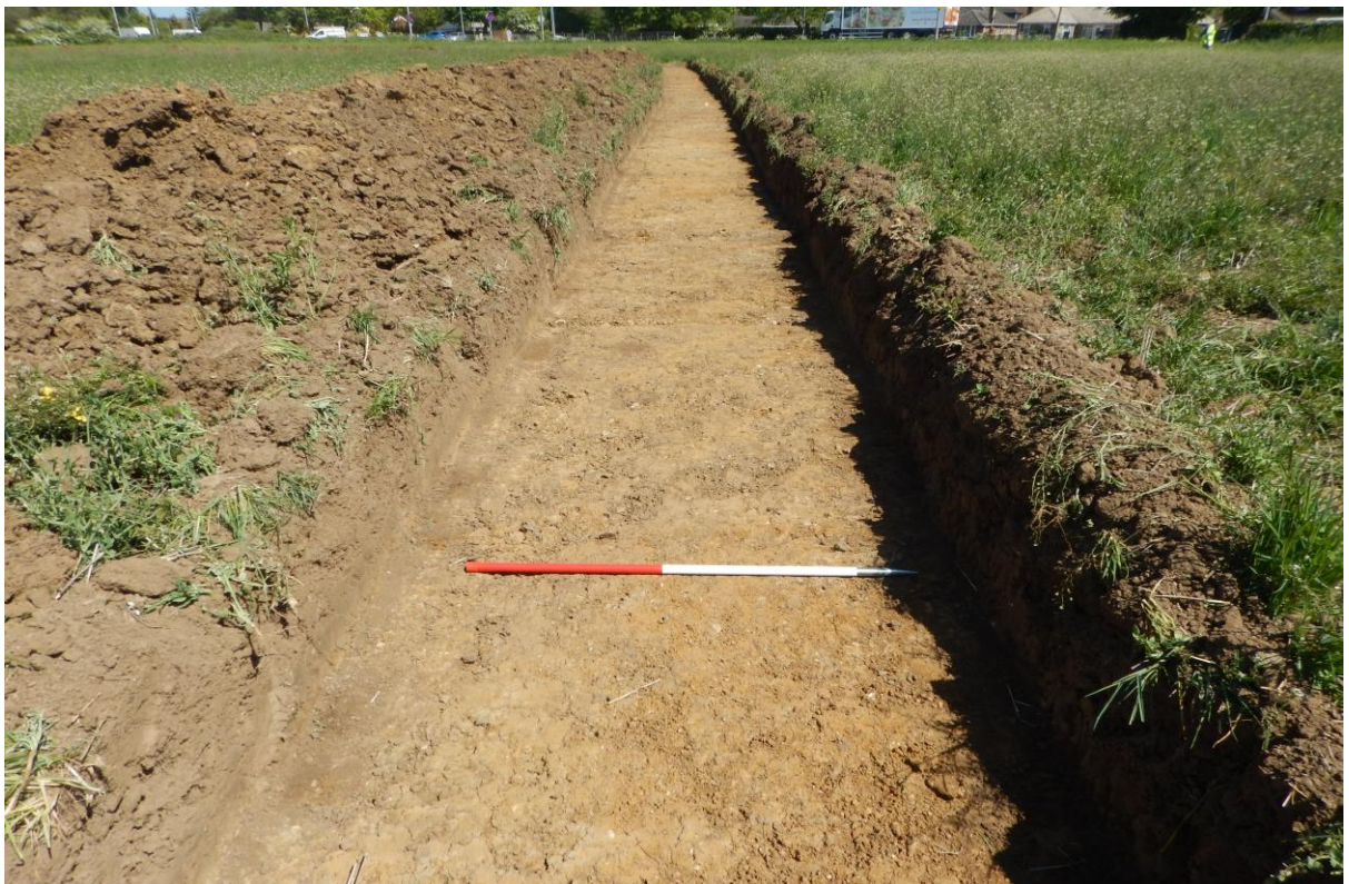
Plate 12 Trench 13. Facing South-West.
