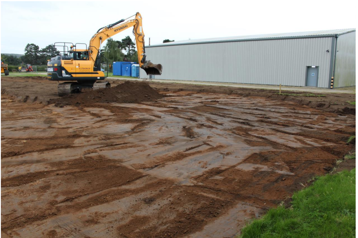
Plate 3. Site During Initial Strip. Facing South-West.
