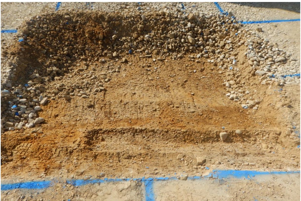
Plate 8. Typical Stanchion Base Showing Natural Deposits
