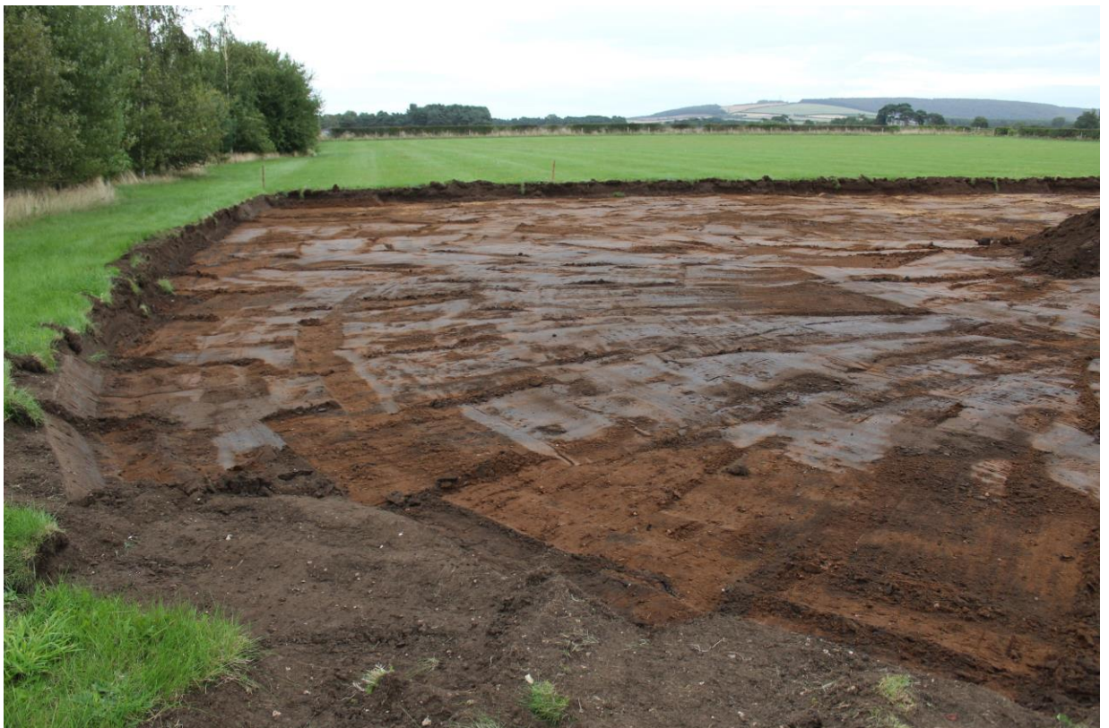
Plate 4. Site During Initial Strip. Facing North-East..
