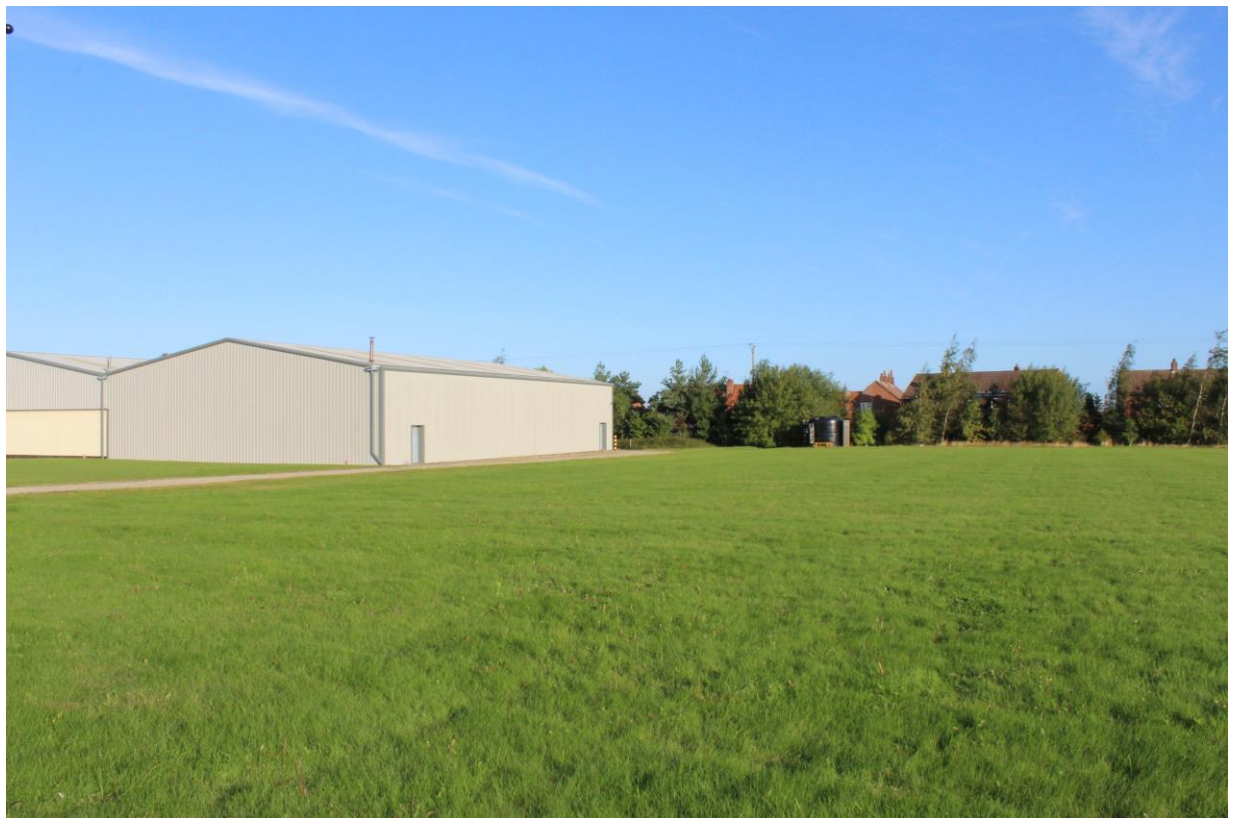
Plate 2. Site Prior to Stripping. Facing North-West.
