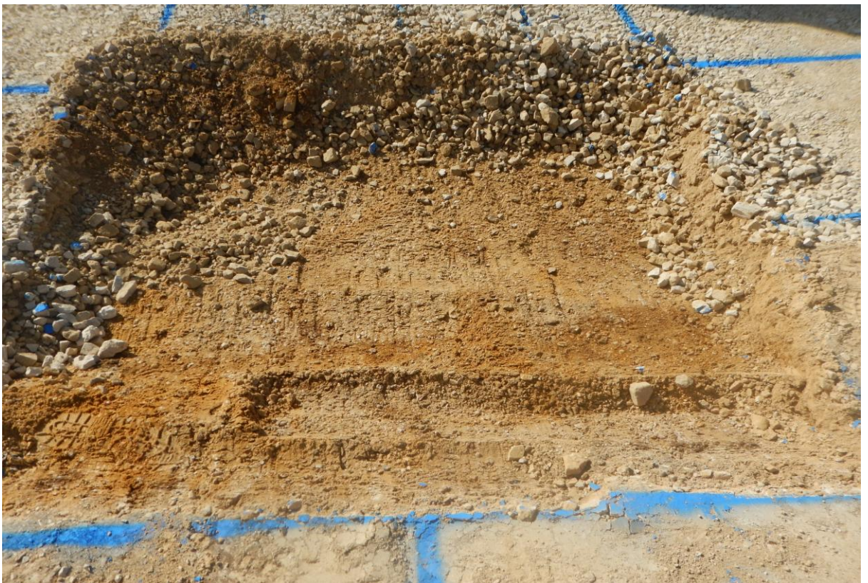
Plate 6. Typical Stanchion Base Showing Natural Deposits
