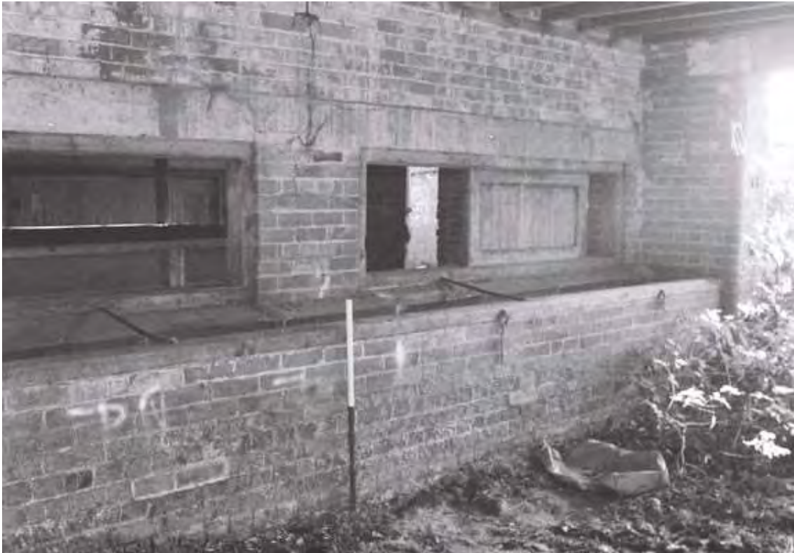
Plate 12. Dutch Barn: Interior – Ground Floor. Facing South-west.
