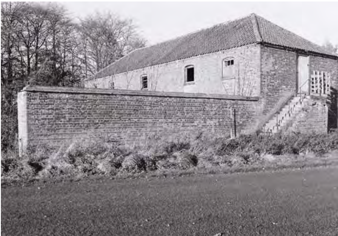
Plate 2. Dutch Barn: Exterior – East and South Elevations. Facing North-west.
