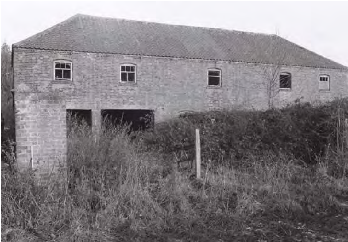
Plate 3. Dutch Barn: Exterior – South Elevation. Facing North.
