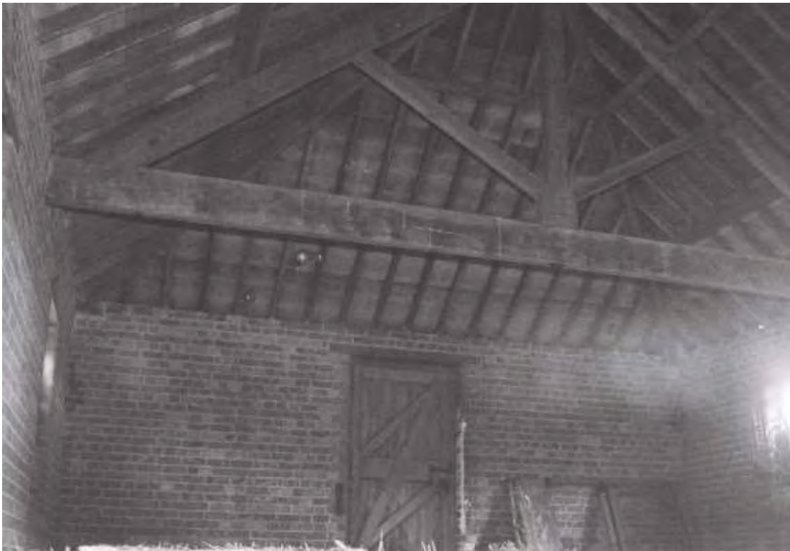
Plate 17. Dutch Barn: Interior – First Floor. Facing East.
