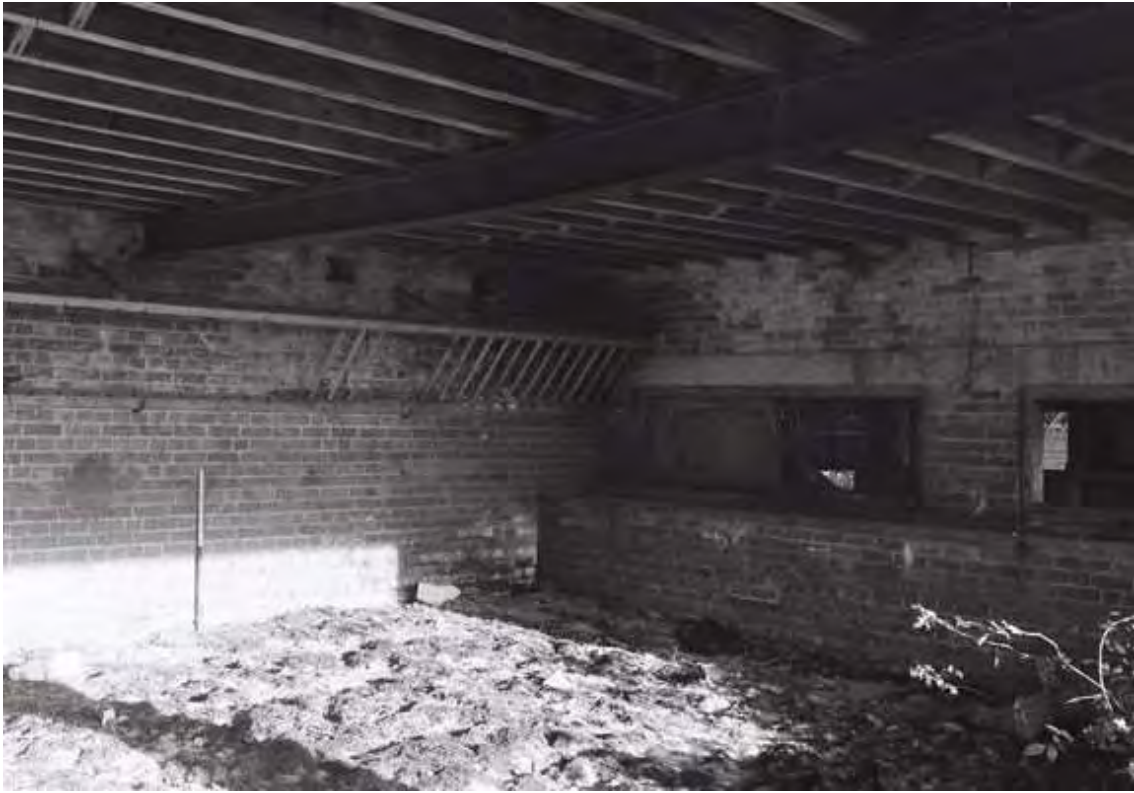
Plate 10. Dutch Barn: Interior – Ground Floor. Facing North-east.
