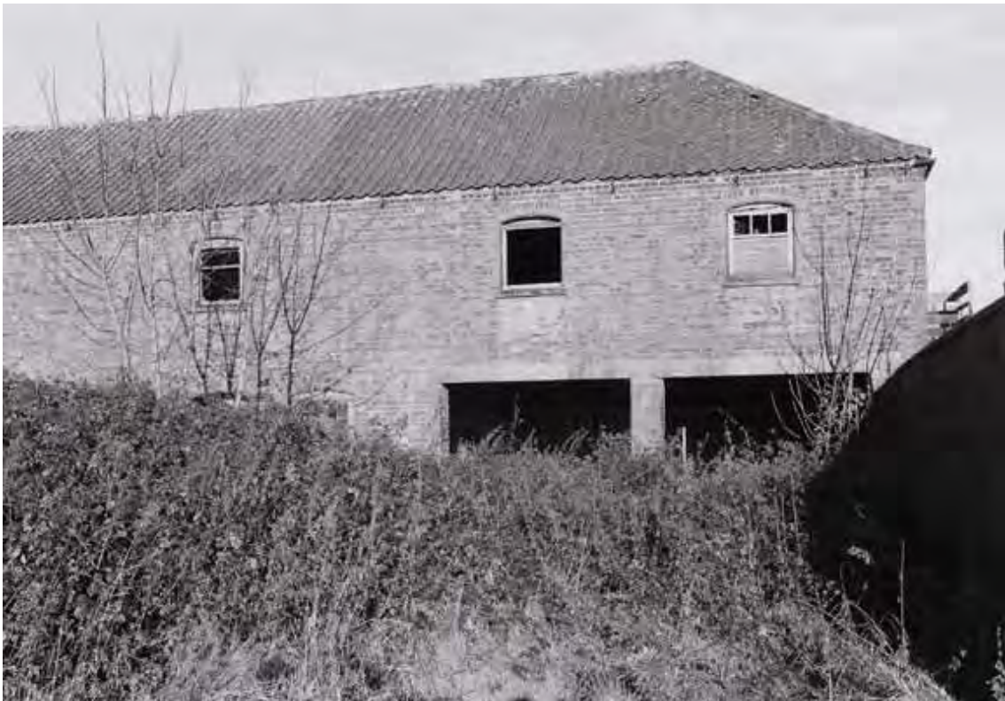
Plate 4. Dutch Barn: Exterior: South Elevation. Facing North.
