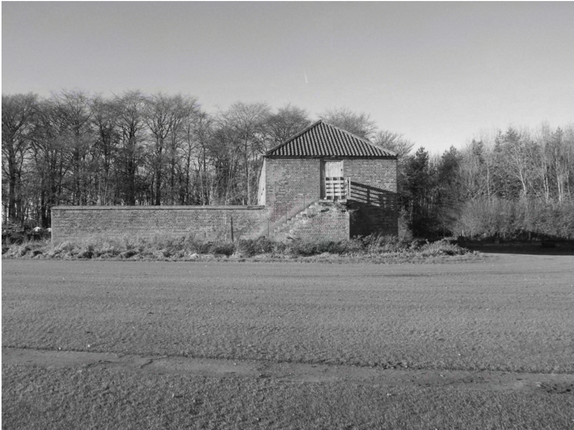
Plate 1. Dutch Barn: Exterior – East Elevation. Facing West.
