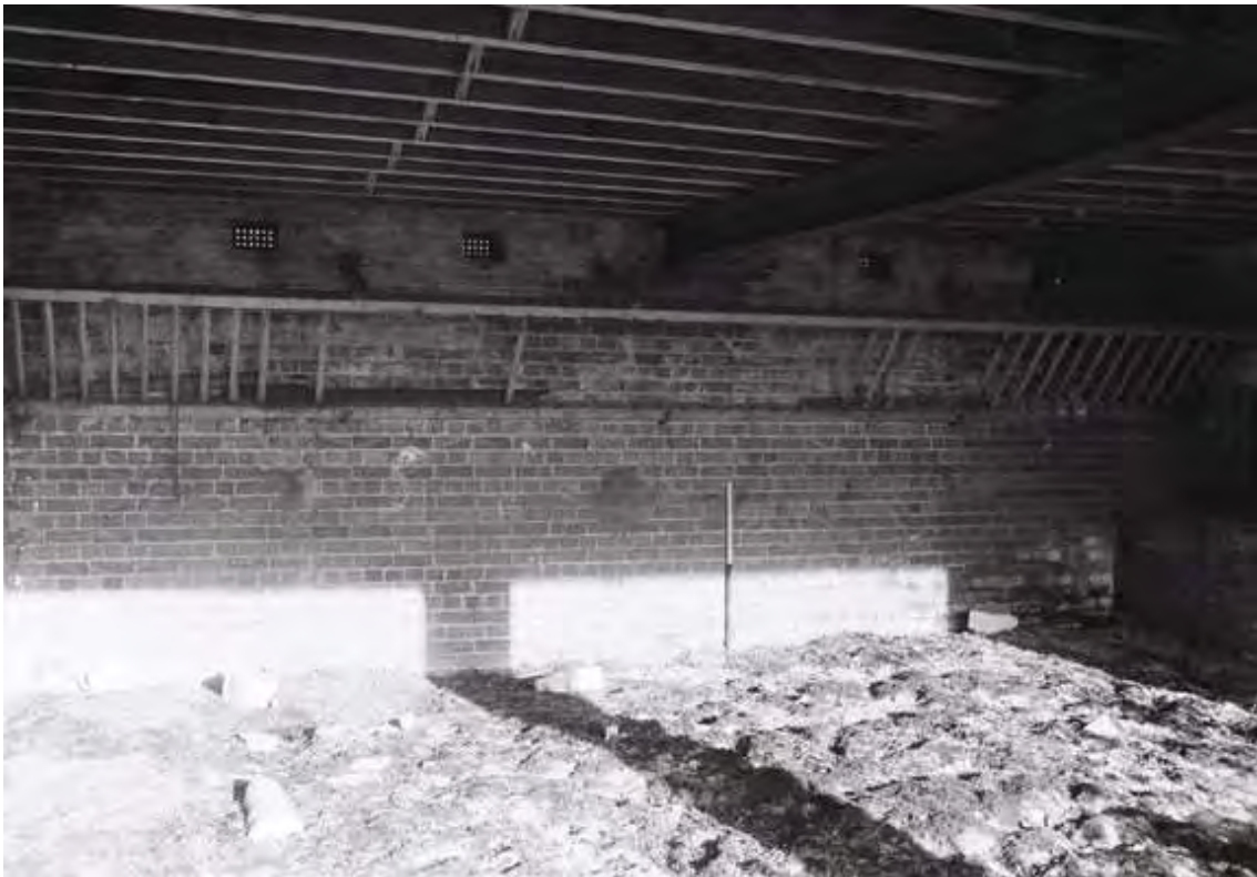
Plate 11. Dutch Barn: Interior – Ground Floor. Facing North.
