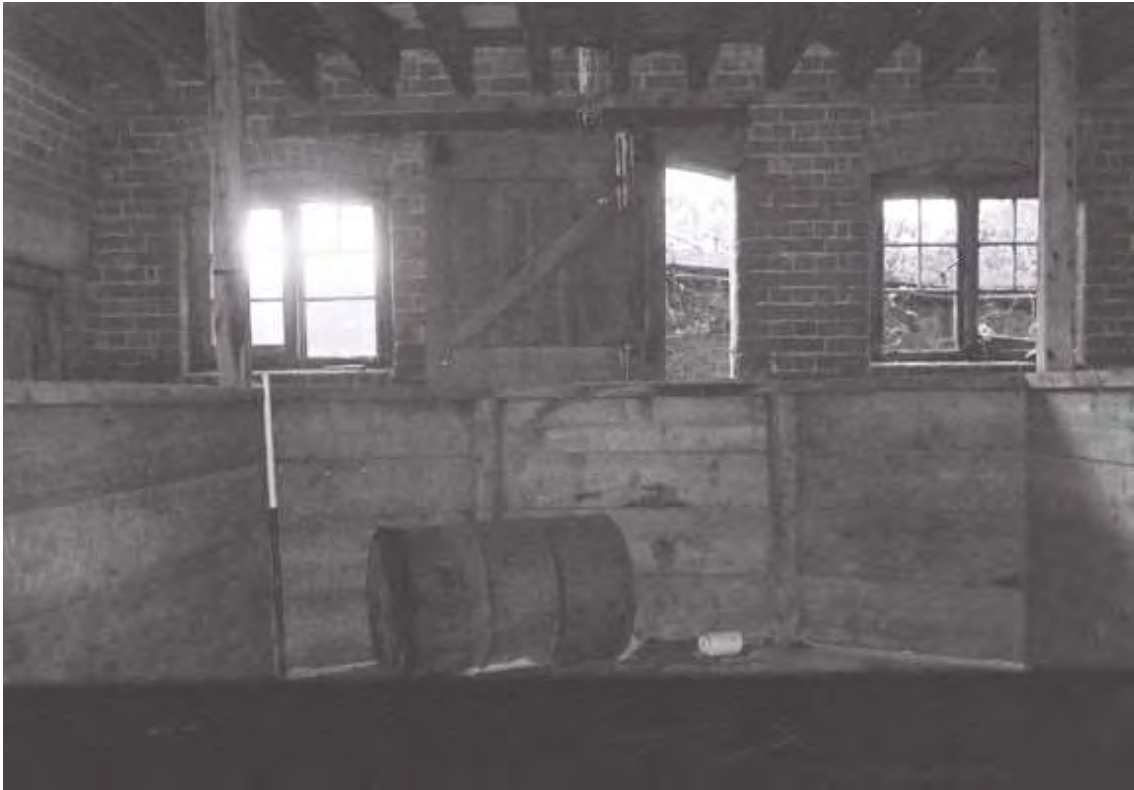
Plate 16. Dutch Barn: Interior – Ground Floor. Facing South.
