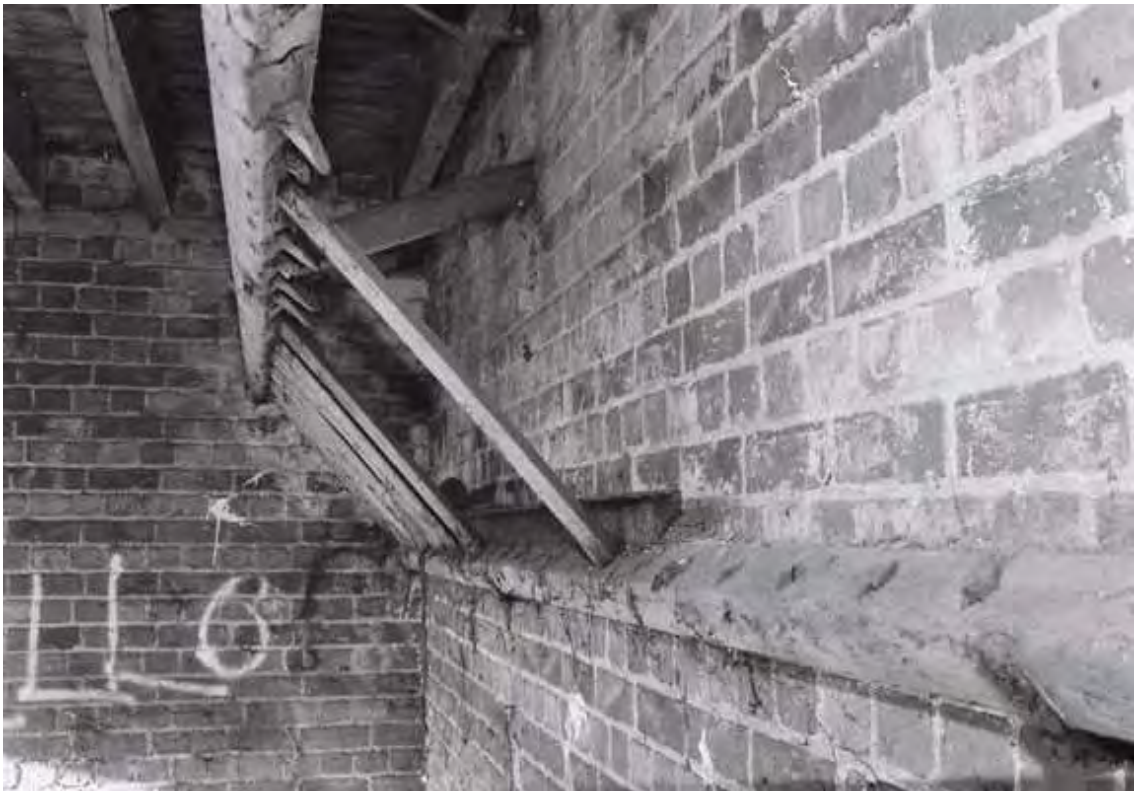
Plate 13. Dutch Barn: Interior – Ground Floor. Facing West.
