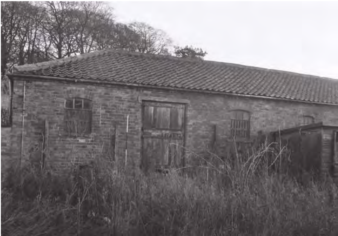
Plate 34. Brick Barn: Exterior – West Elevation. Facing East.
