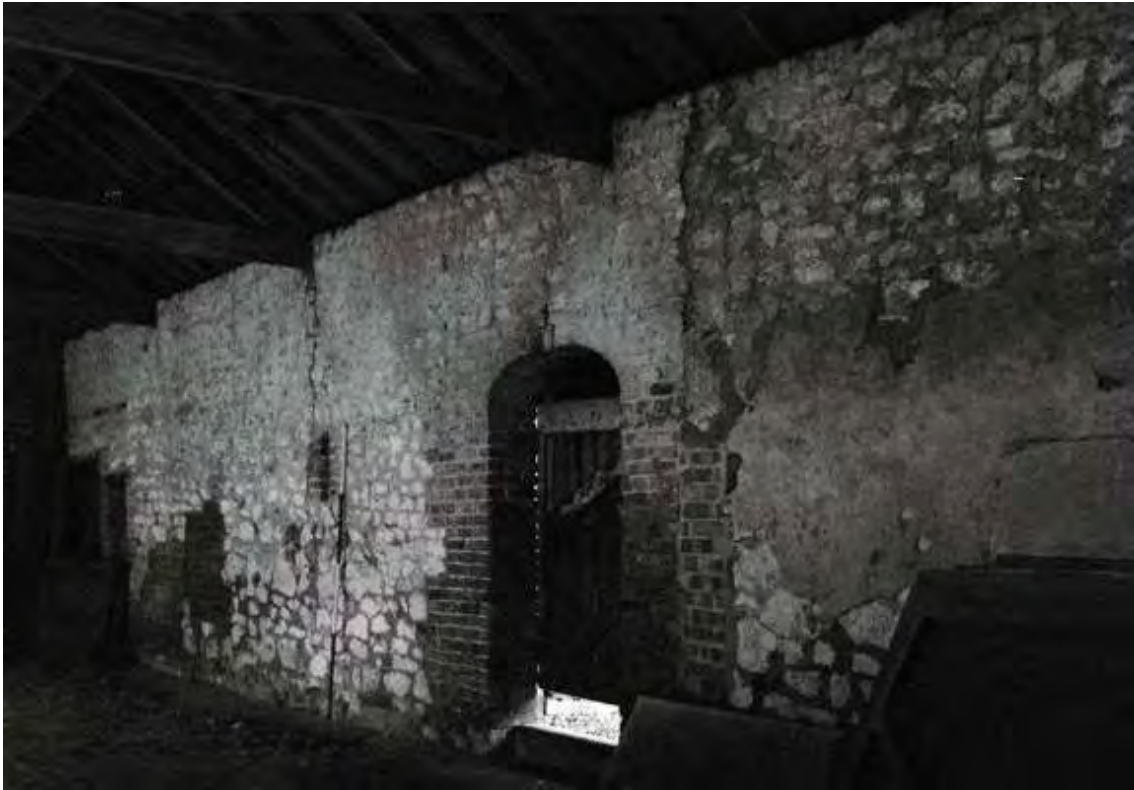
Plate 19. Chalk Barn: Interior. Facing South-west.
