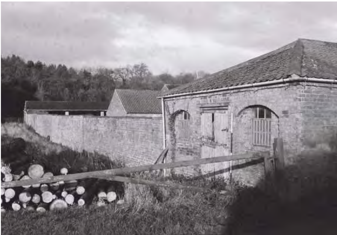
Plate 24. Brick Barn: Exterior – South Elevation. Facing North-west.
