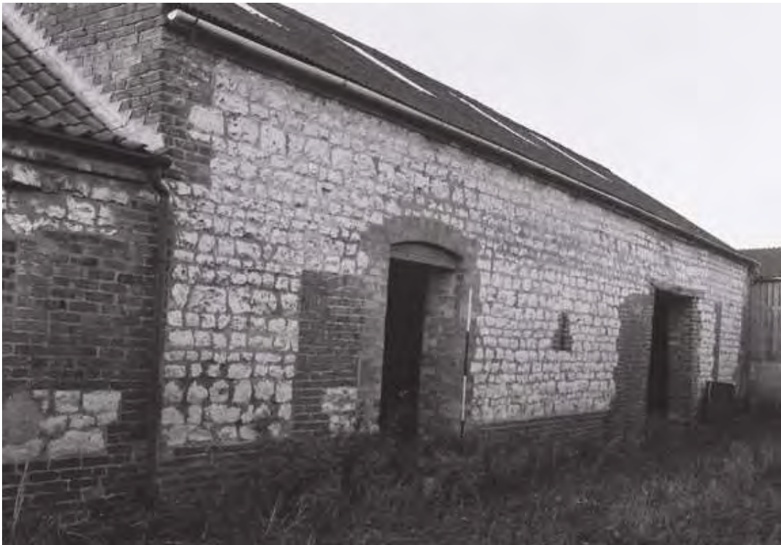
Plate 10. Chalk Barn: Exterior – East Elevation. Facing North-west.
