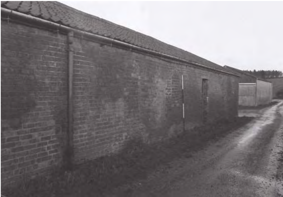
Plate 28. Brick Barn: Exterior – East Elevation. Facing North-west.
