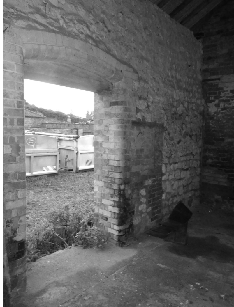
Plate 22. Chalk Barn: Interior. Facing South-east.
