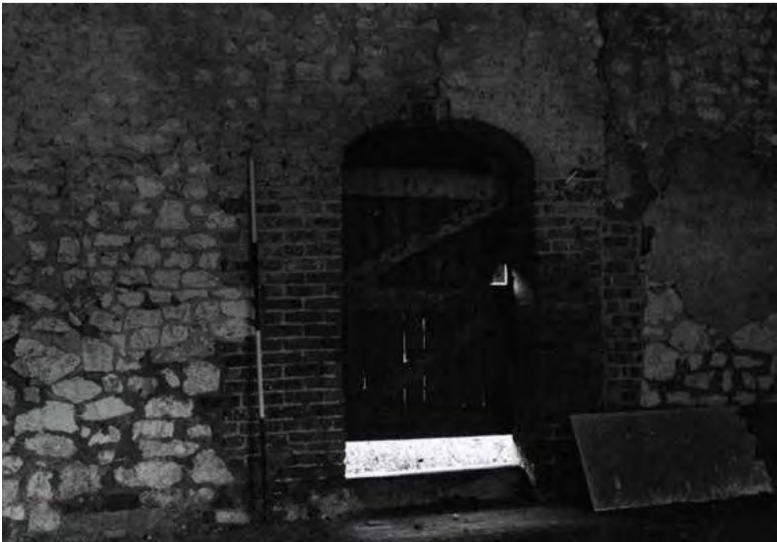
Plate 20. Chalk Barn: Interior. Facing West.
