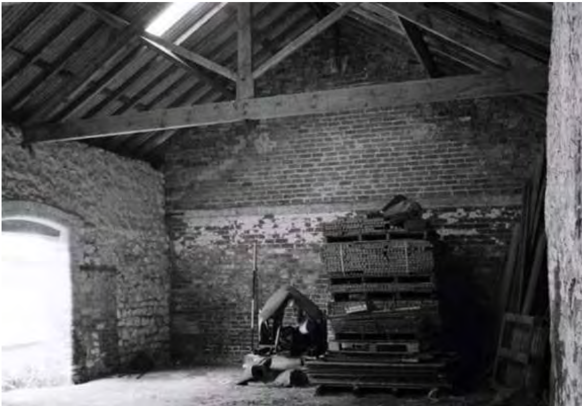
Plate 14. Chalk Barn: Interior. Facing South-east.
