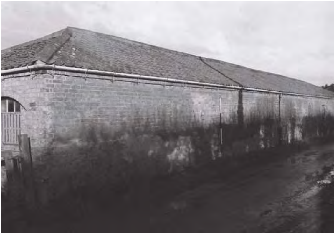
Plate 27. Brick Barn: Exterior – East Elevation. Facing North-west.
