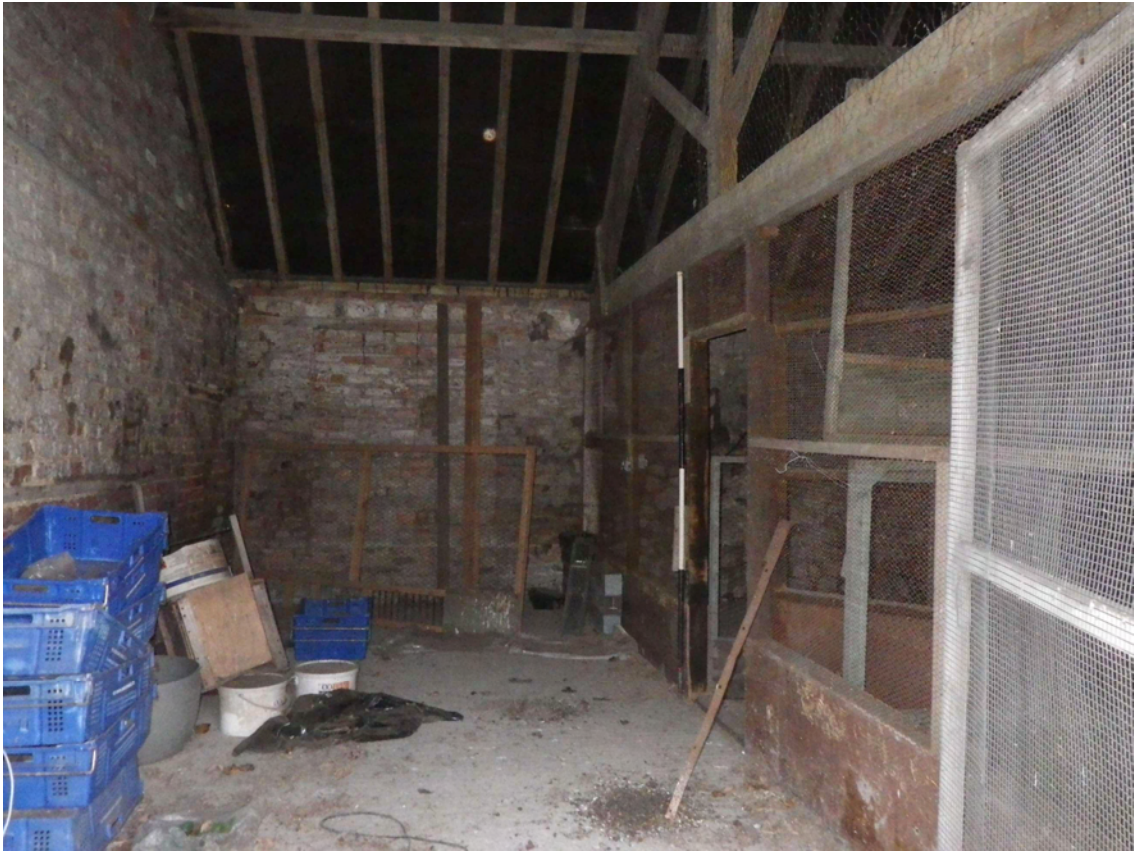
Plate 23. Chalk Barn: Interior. Facing West.
