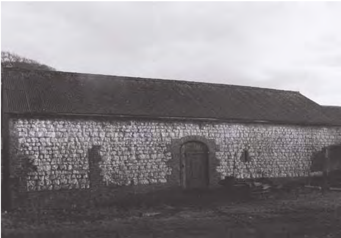
Plate 2. Chalk Barn: Exterior – West Elevation. Facing East.
