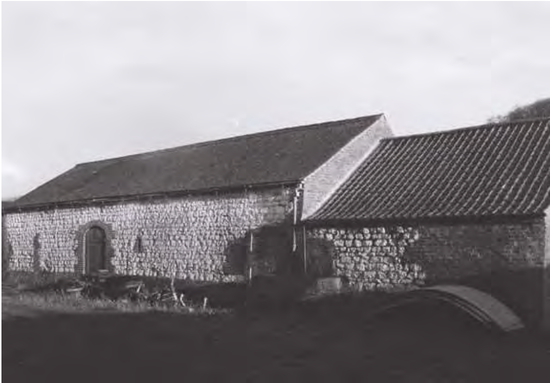
Plate 1. Chalk Barn: Exterior – West Elevation. Facing North-east.
