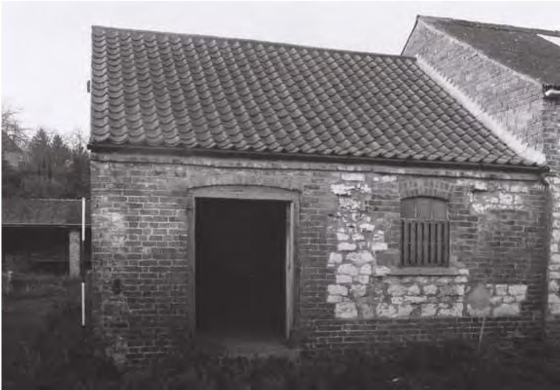
Plate 9. Chalk Barn: Exterior – East Elevation. Facing West.
