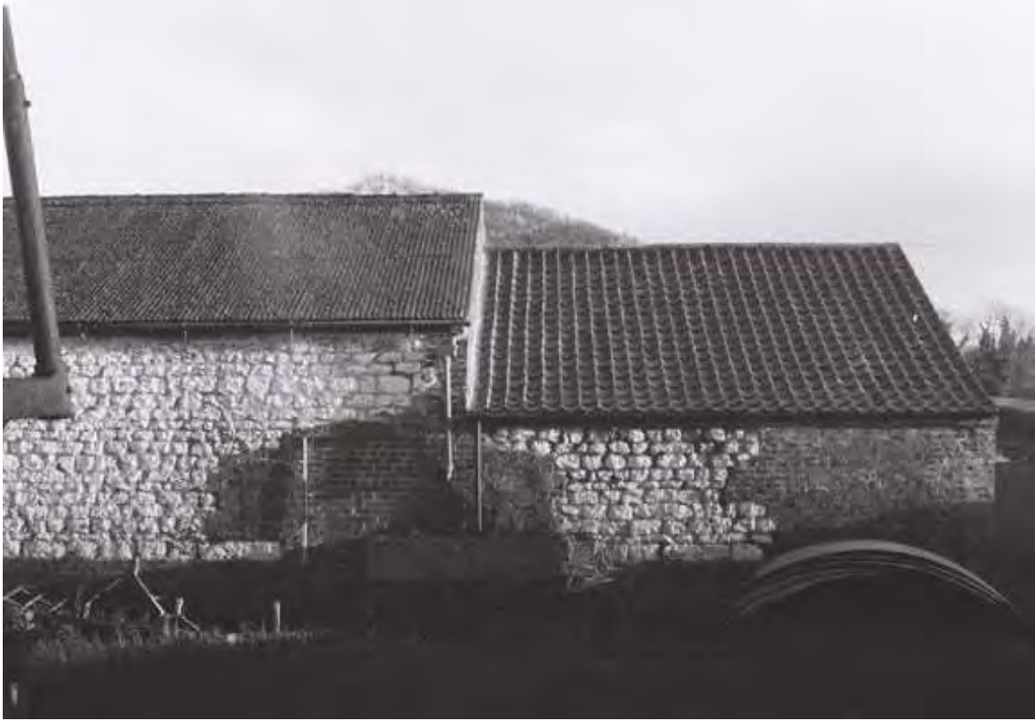
Plate 3. Chalk Barn: Exterior – West Elevation. Facing East.
