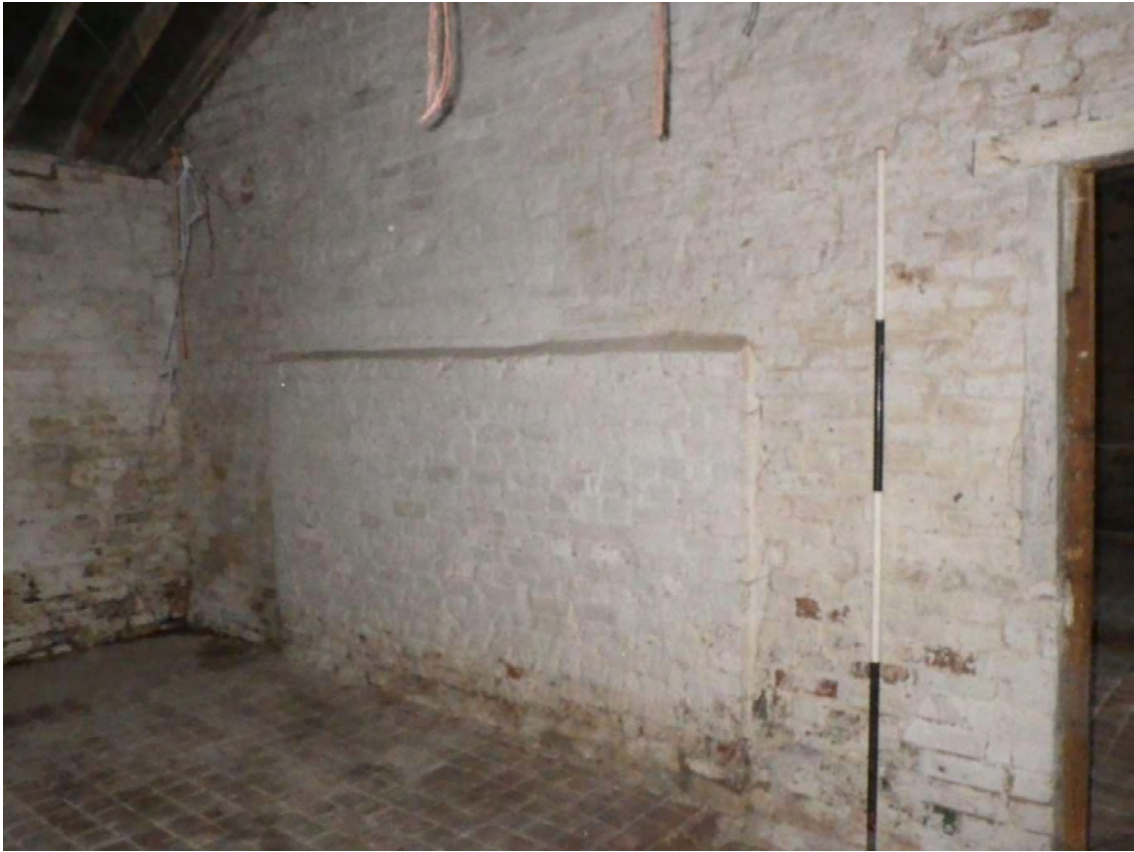
Plate 37. Brick Barn: Interior. Facing South-east.
