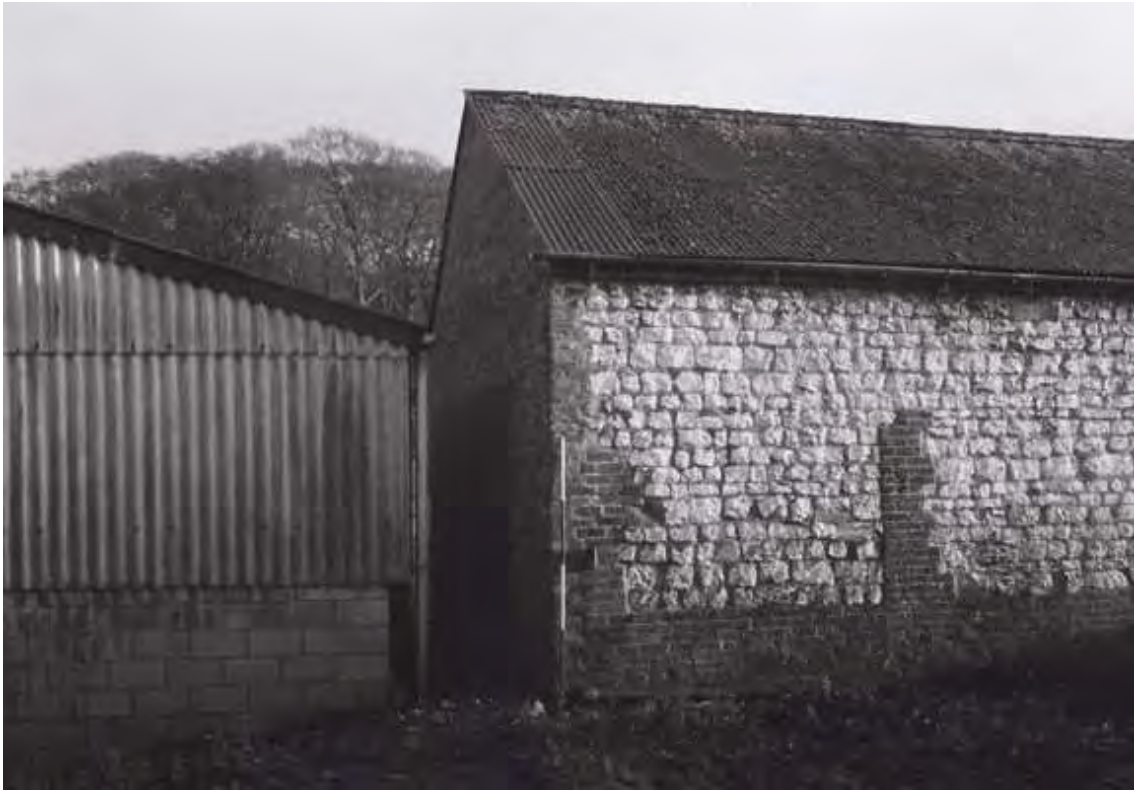
Plate 5. Chalk Barn: Exterior – North and West Elevations. Facing East.
