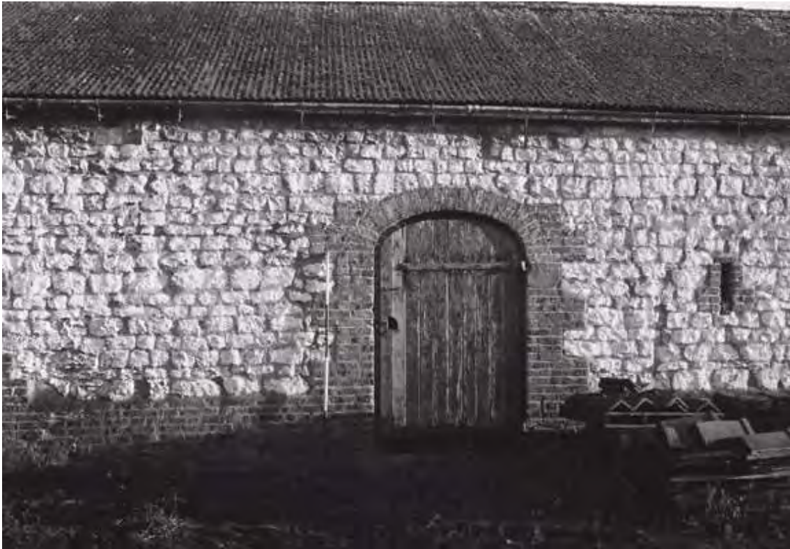
Plate 4. Chalk Barn: Exterior – West Elevation. Facing East.
