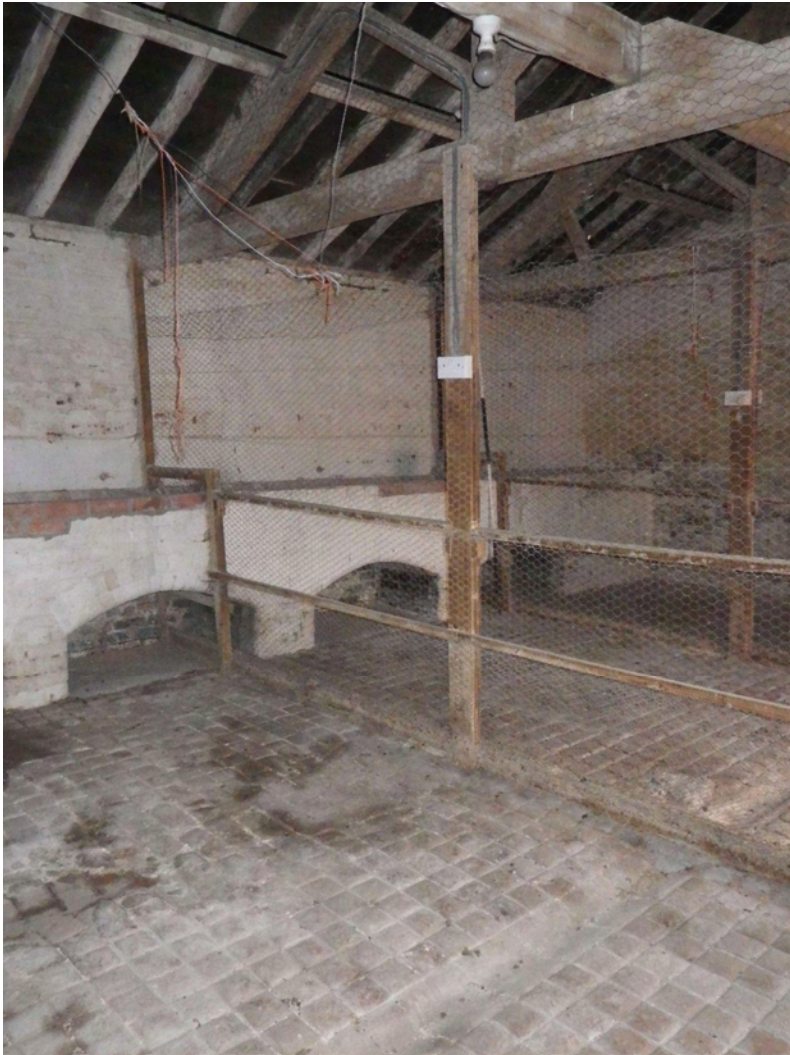
Plate 35. Brick Barn: Interior. Facing South-east.
