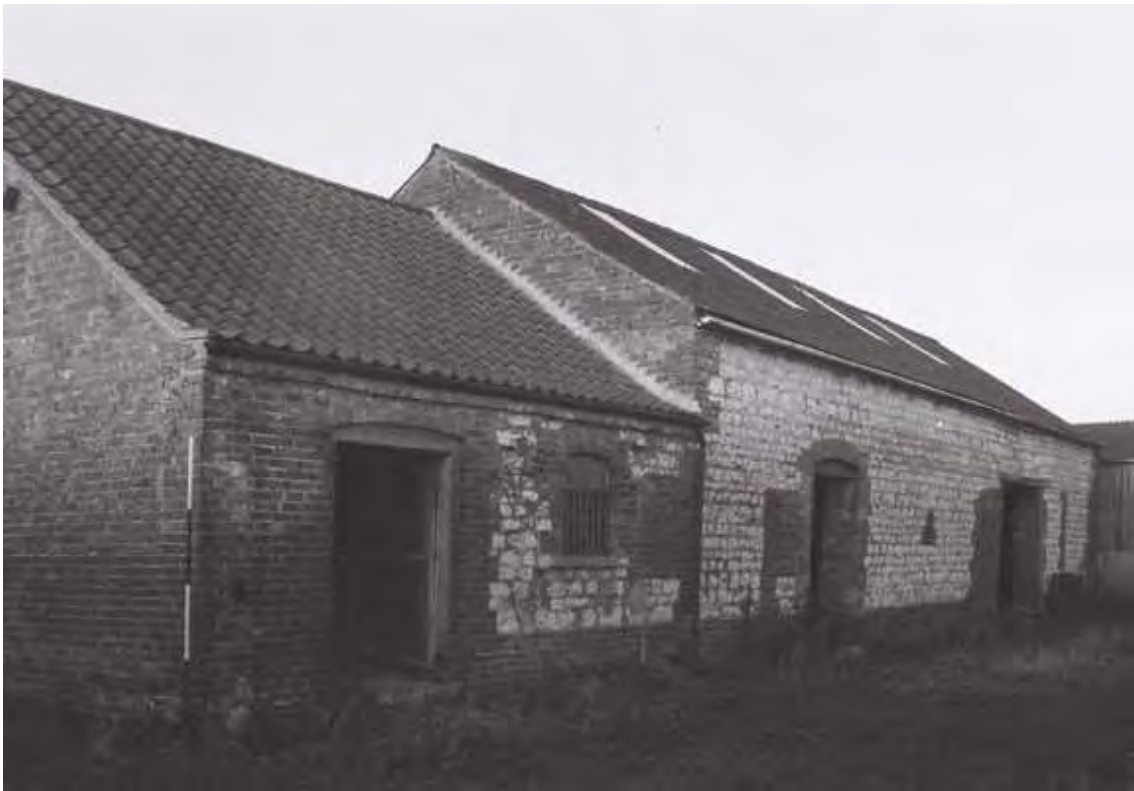
Plate 8. Chalk Barn: Exterior – East Elevation. Facing North-west.
