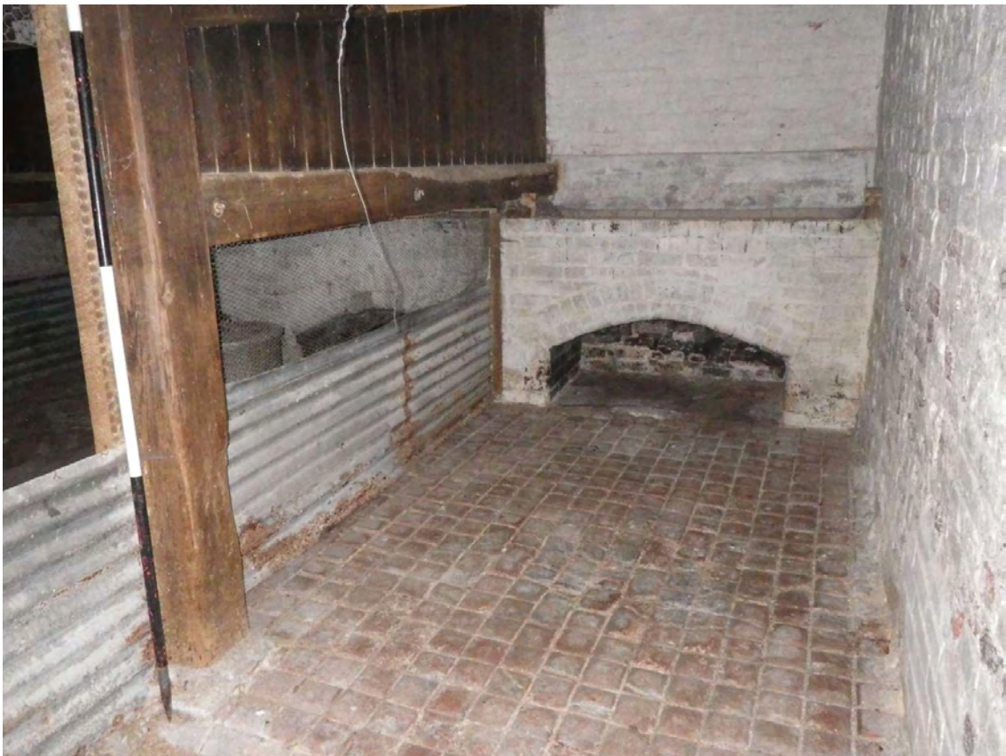
Plate 38. Brick Barn: Interior. Facing East.
