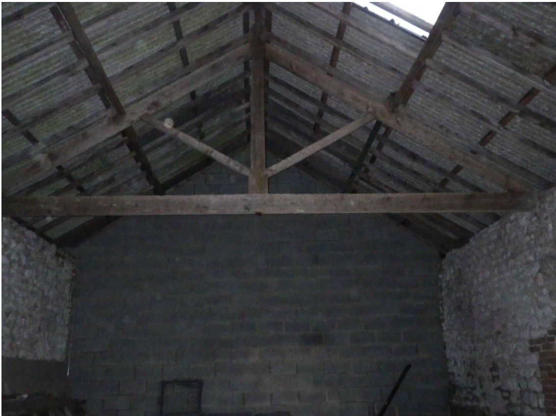
Plate 16. Chalk Barn: Interior. Facing North.
