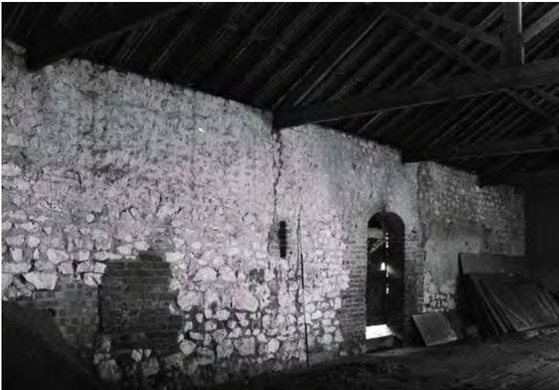
Plate 18. Chalk Barn: Interior. Facing North-west.
