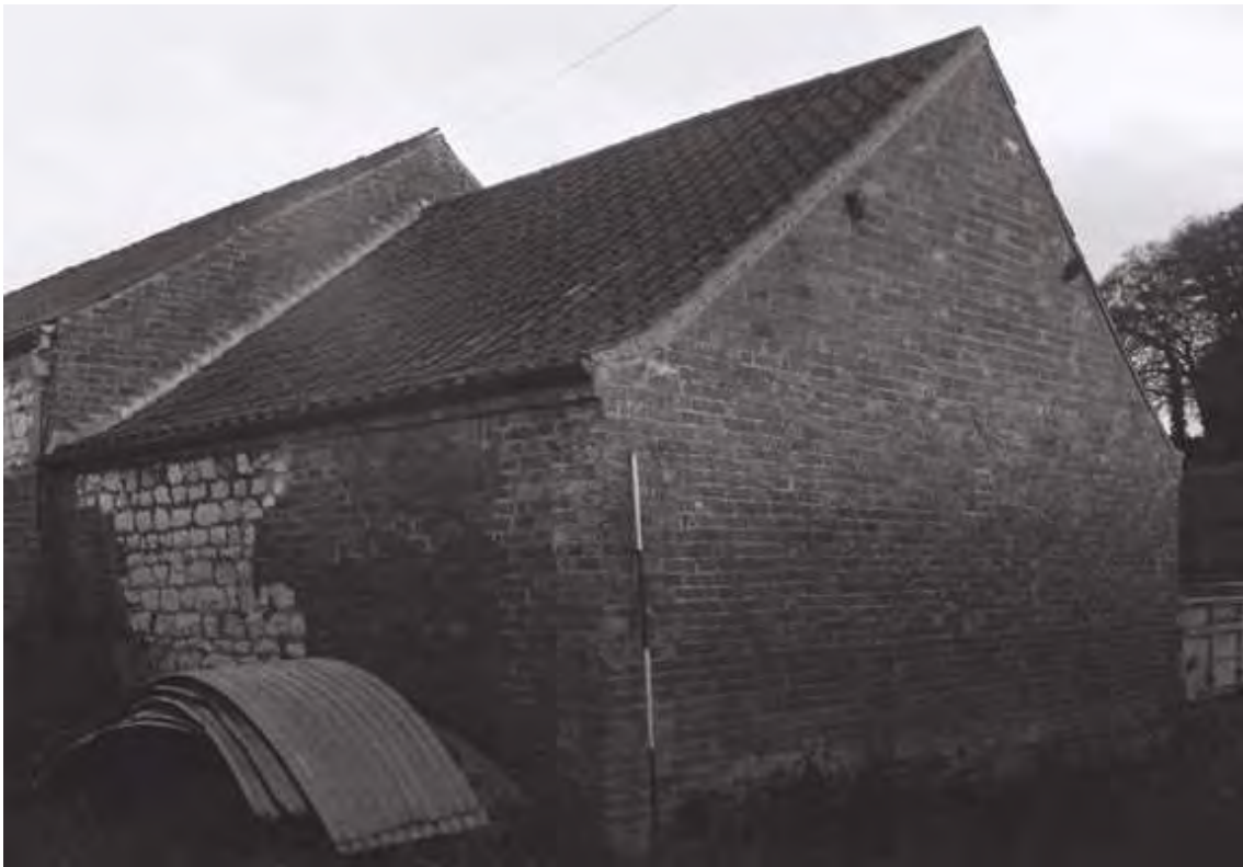
Plate 6. Chalk Barn: Exterior – West and South Elevations. Facing North-west.
