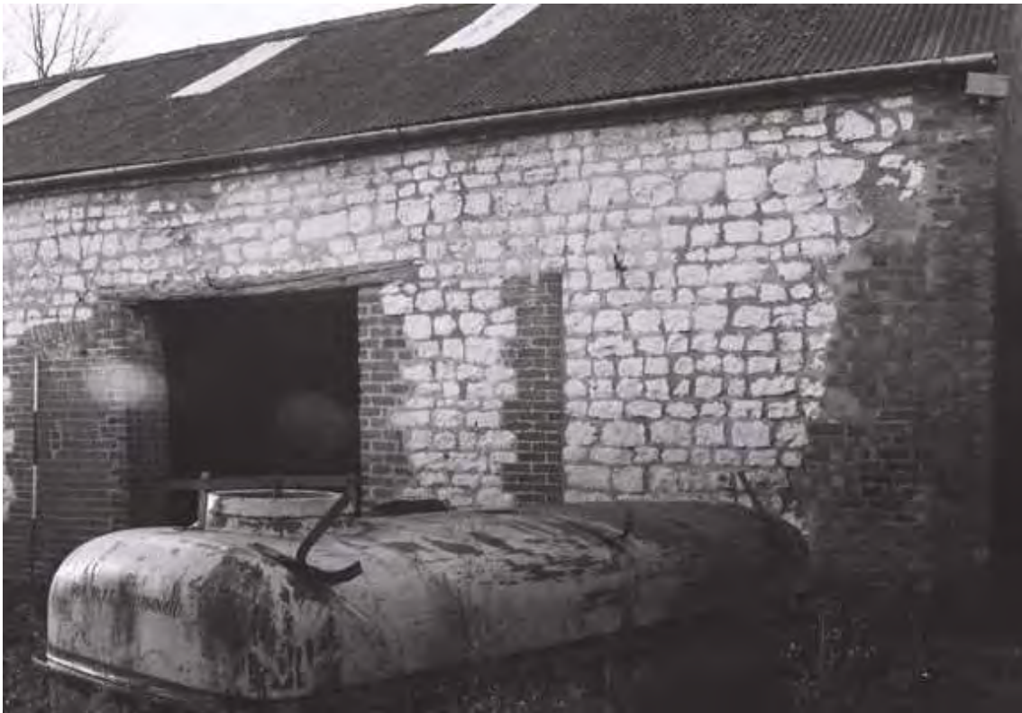
Plate 12. Chalk Barn: Exterior – East Elevation. Facing South-west.
