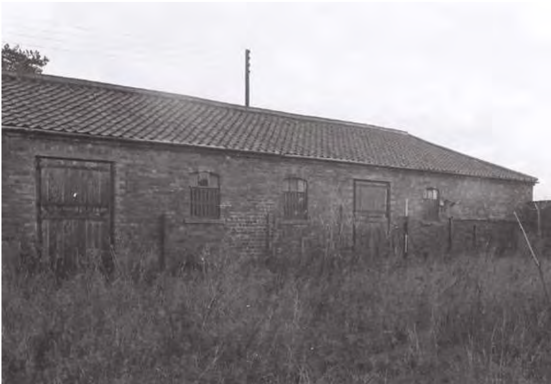
Plate 32. Brick Barn: Exterior – West Elevation. Facing South-east.
