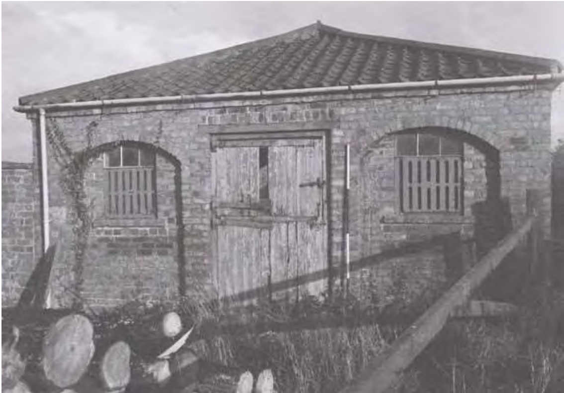
Plate 25. Brick Barn: Exterior – South Elevation. Facing North.
