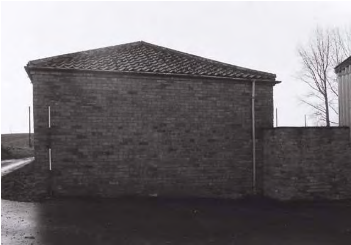
Plate 30. Brick Barn: Exterior – North Elevation. Facing South.
