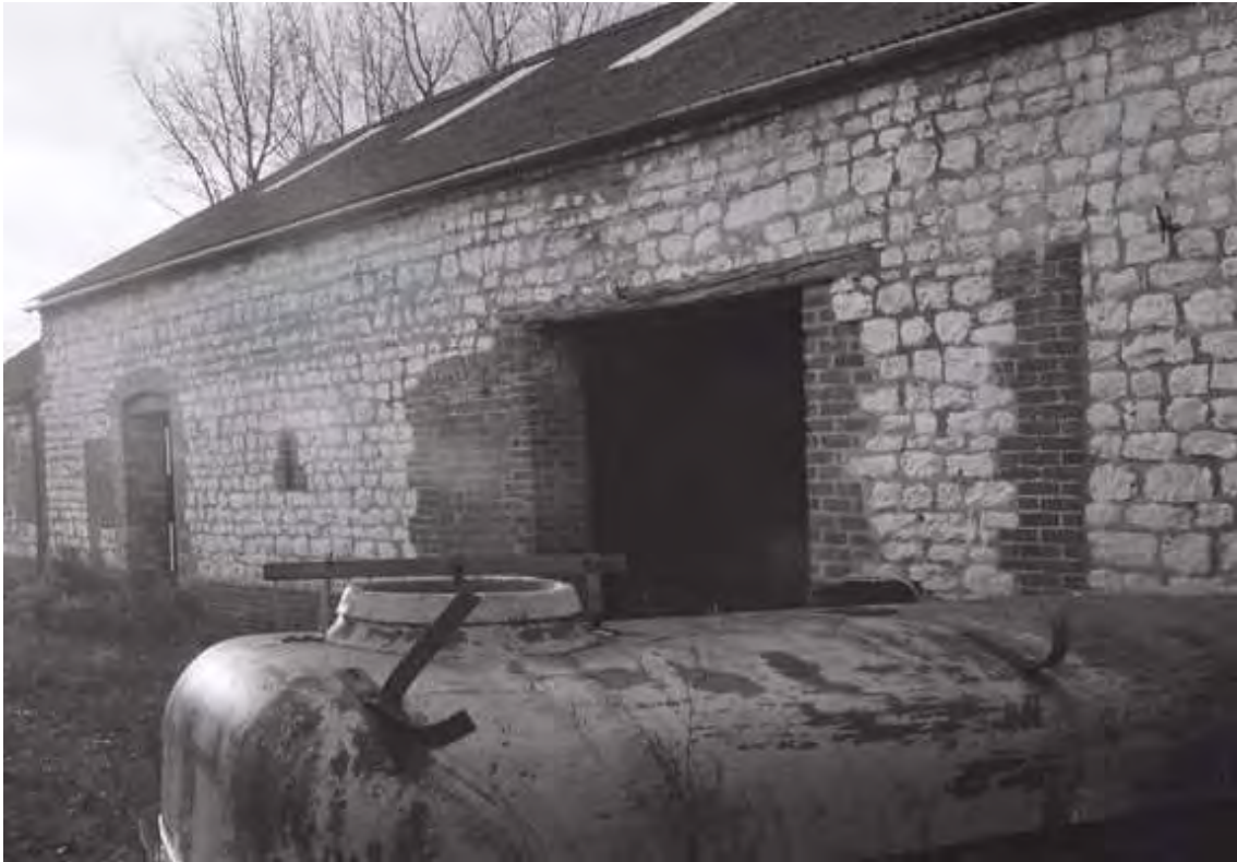
Plate 11. Chalk Barn: Exterior – East Elevation. Facing South-west.
