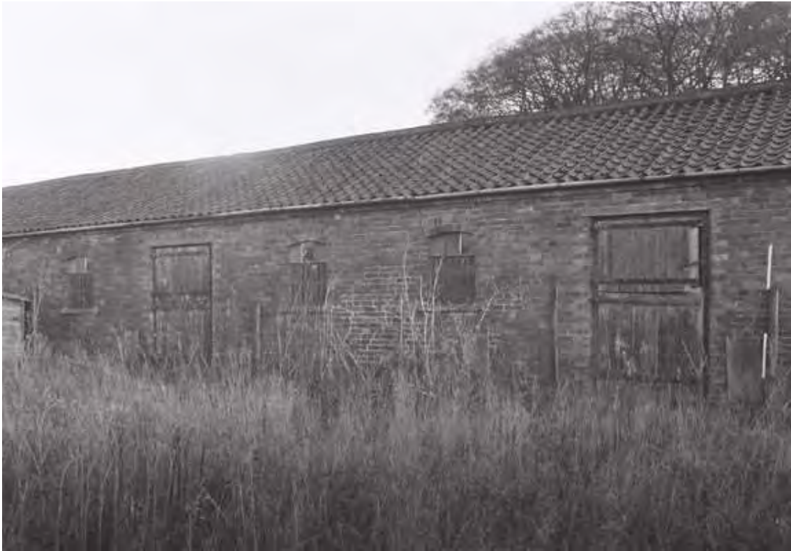
Plate 33. Brick Barn: Exterior – West Elevation. Facing East.
