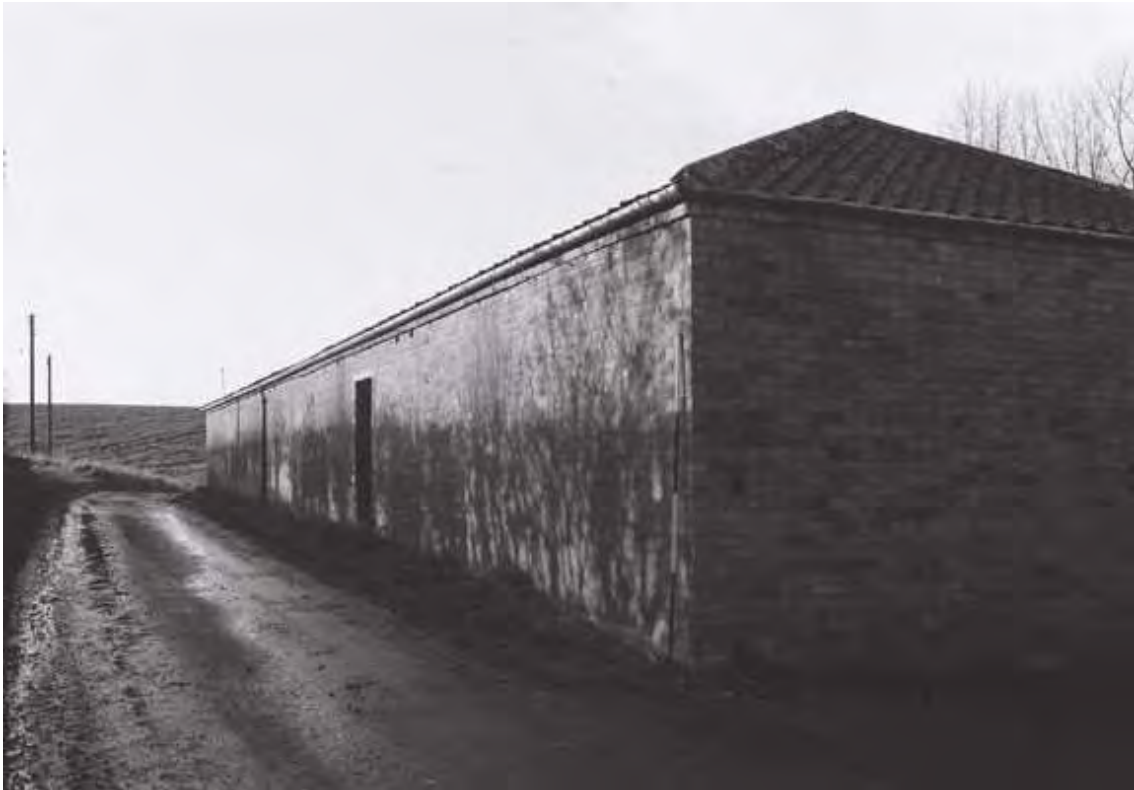
Plate 29. Brick Barn: Exterior – South Elevation. Facing South-west.
