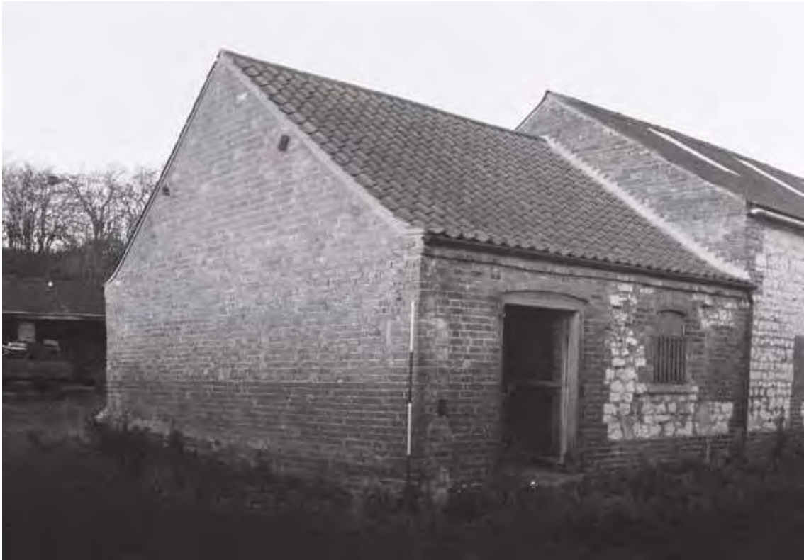
Plate 7. Chalk Barn: Exterior – South and East Elevations. Facing North-west.
