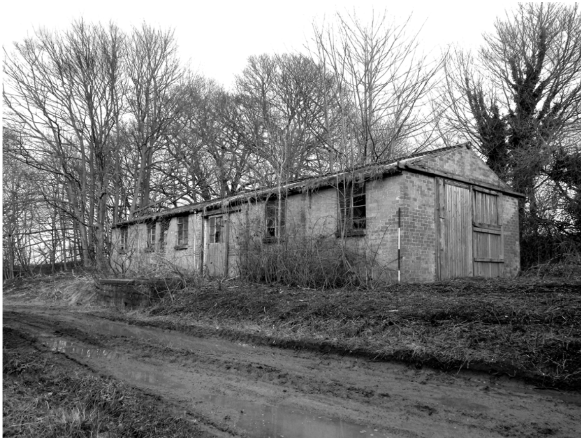
Plate 21. Store Exterior: West Elevation. Facing North-east.
