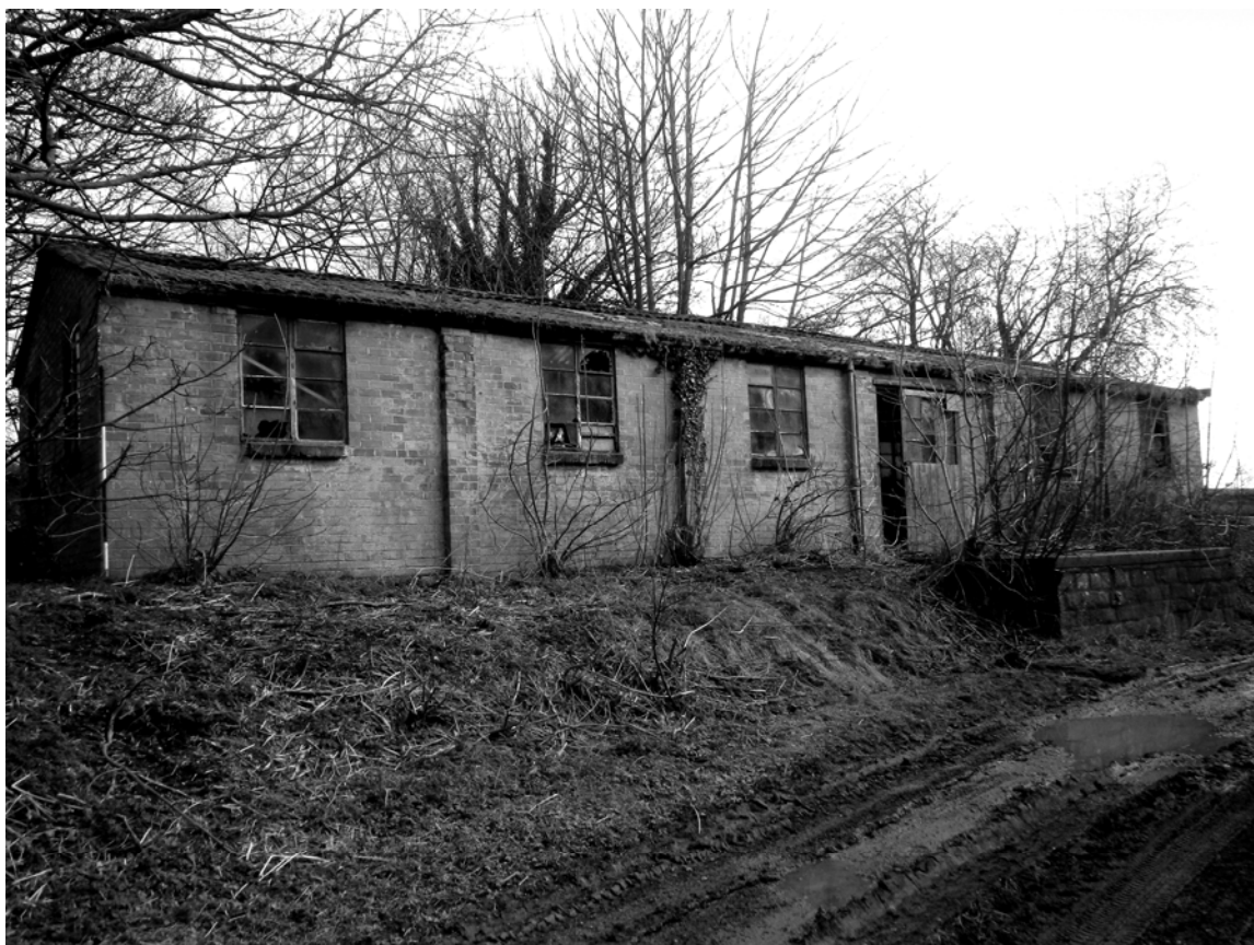
Plate 22. Store Exterior: West Elevation. Facing South-east.
