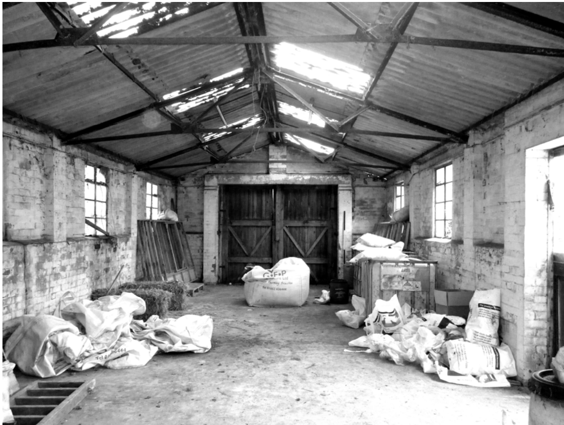
Plate 27. Store Interior. Facing South.
