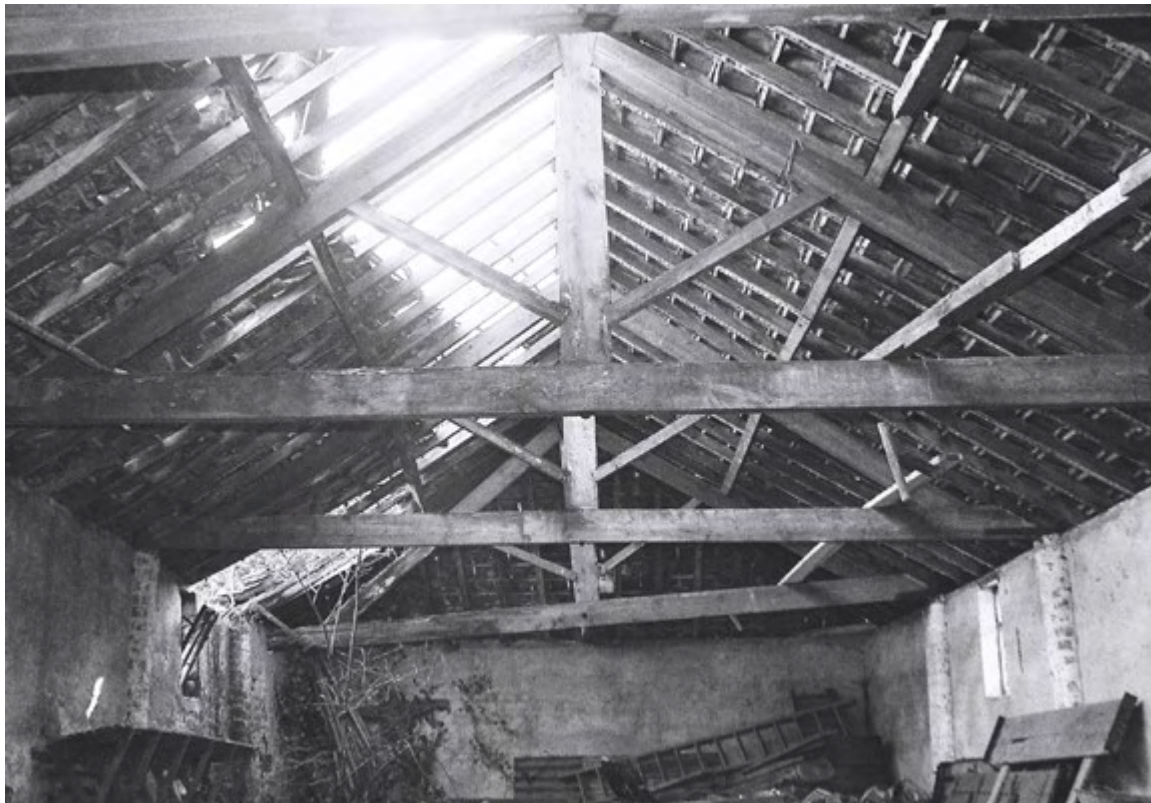
Plate 15. Cart Shed Interior: King Post Roof Truss. Facing South.
