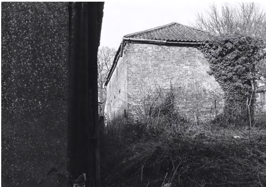
Plate 6. Cart Shed Exterior: South and West Elevations. Facing North-east.
