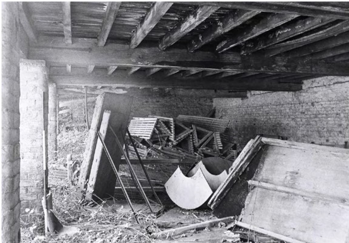
Plate 12. Cart Shed Interior: Ground Floor. Facing South.
