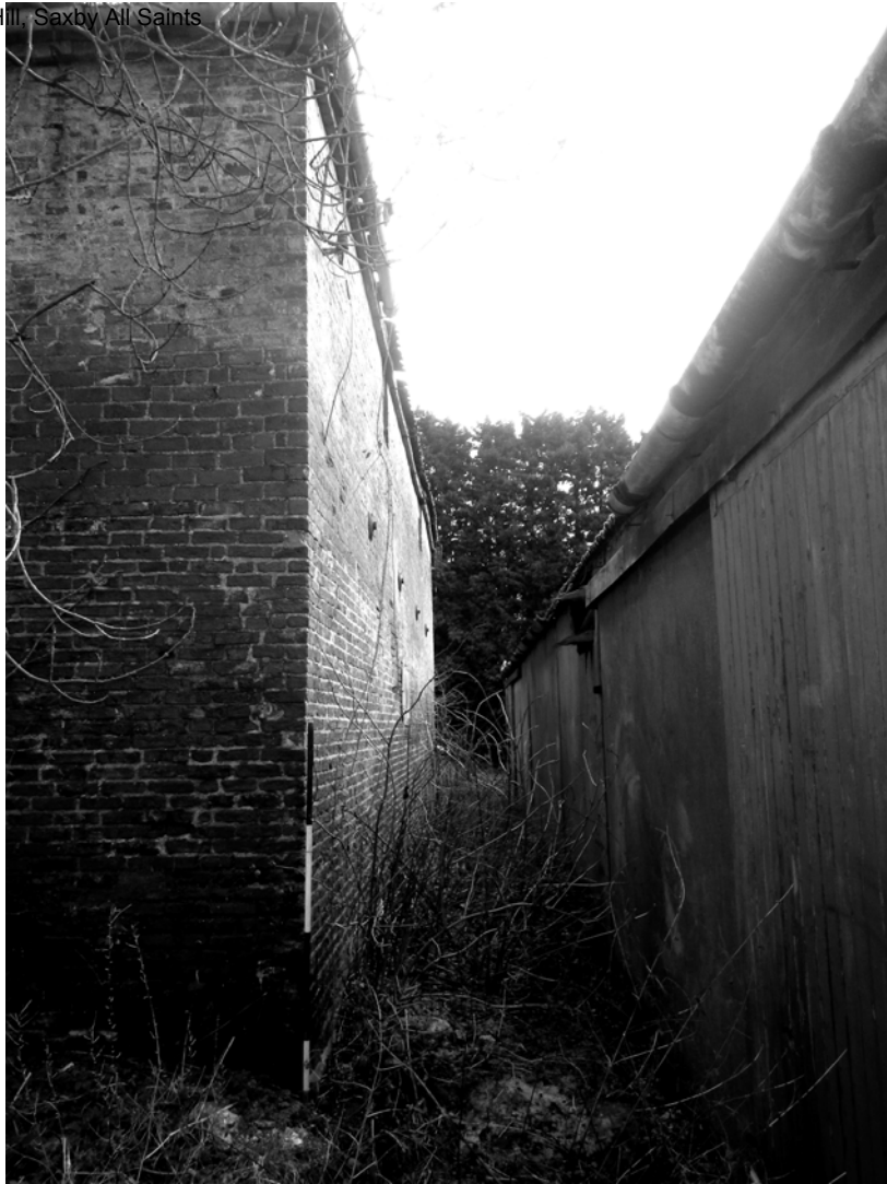
Plate 7. Cart Shed Exterior: West Elevation. Facing South.
