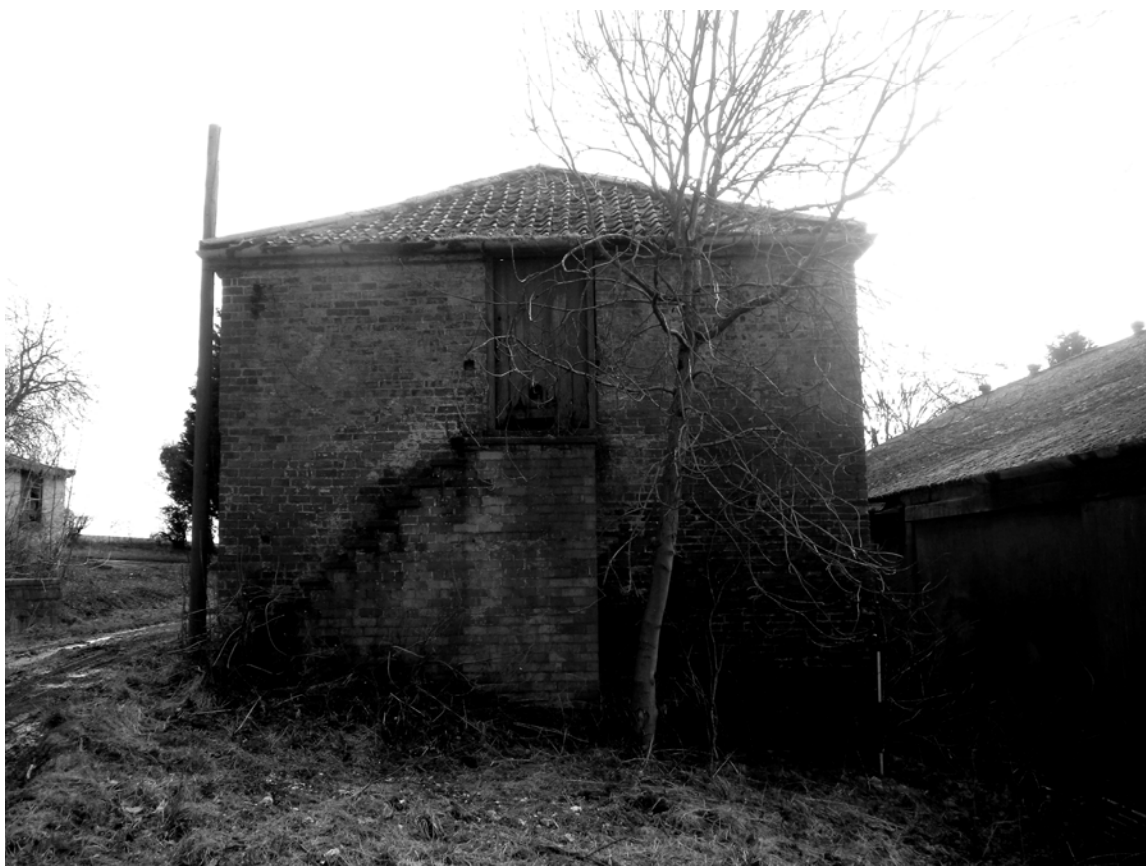
Plate 4. Cart Shed Exterior: North Elevation. Facing South.
