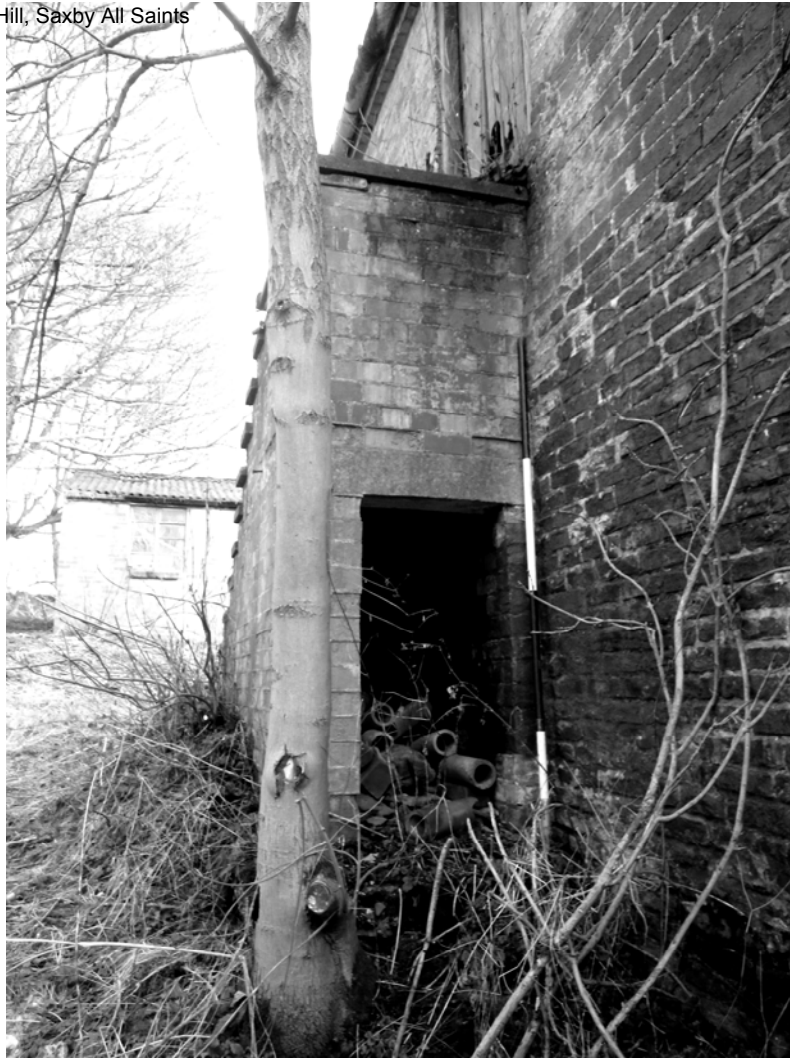
Plate 11. Cart Shed Exterior: Rear of External Steps. Facing East.
