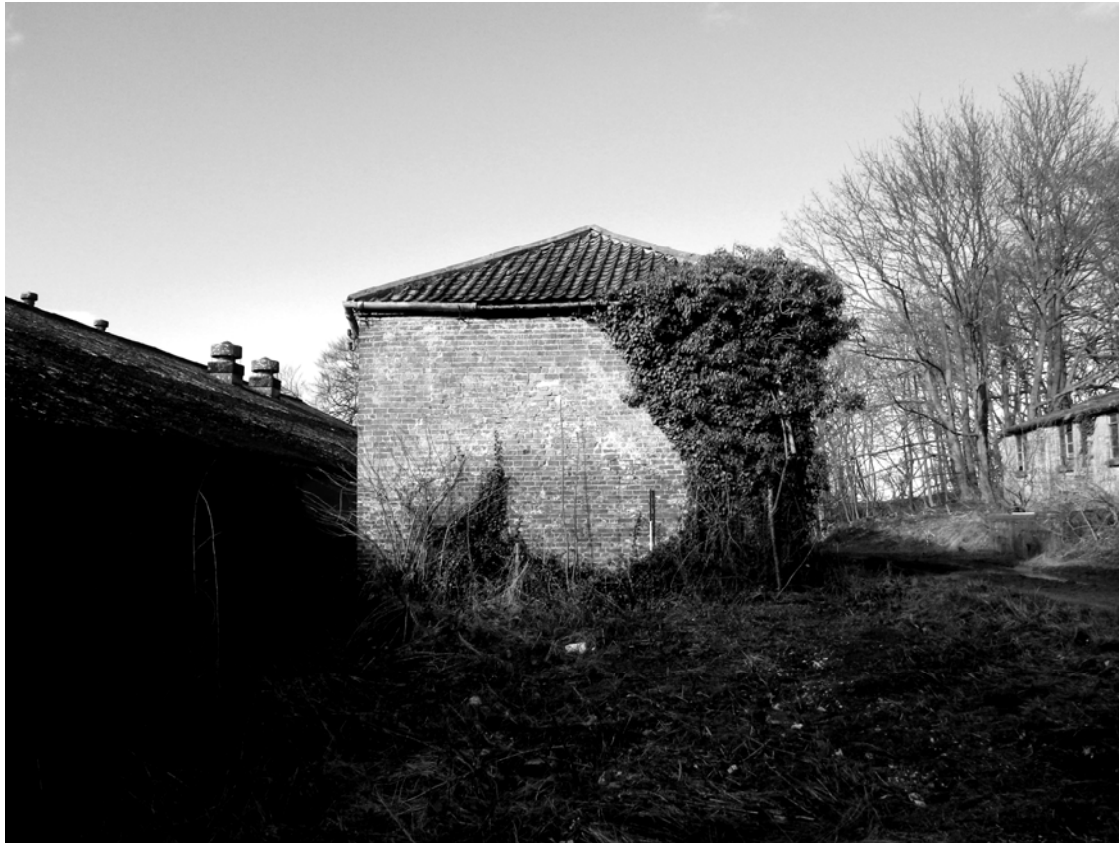
Plate 5. Cart Shed Exterior: South Elevation. Facing North.
