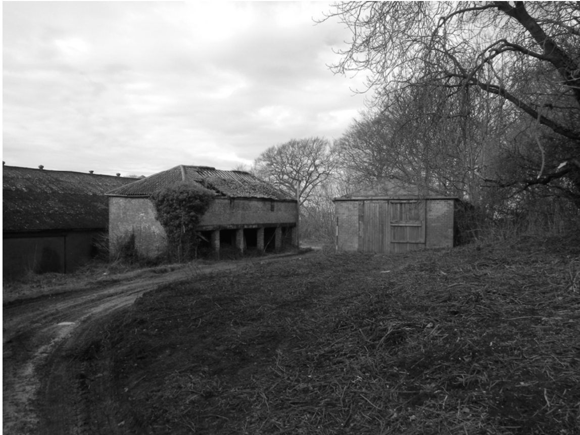
Plate 1. Cart Shed and Store. Facing North-west.
