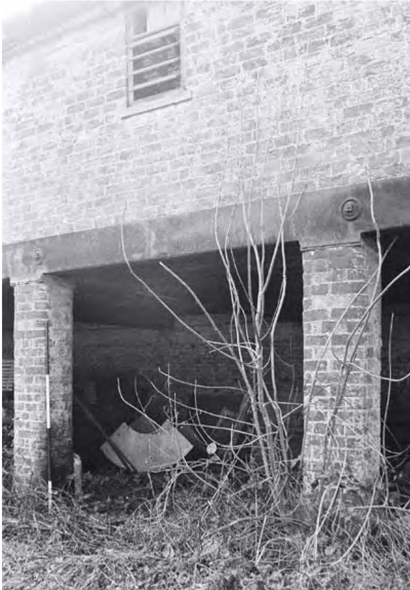
Plate 9. Cart Shed Exterior: East Elevation. Facing West.
