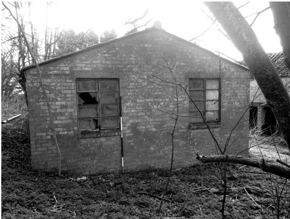
Plate 24. Store Exterior: North Elevation. Facing South.
