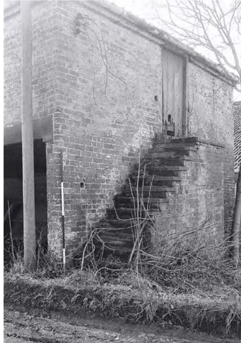
Plate 10. Cart Shed Exterior: Steps to Granary. Facing South-west.
