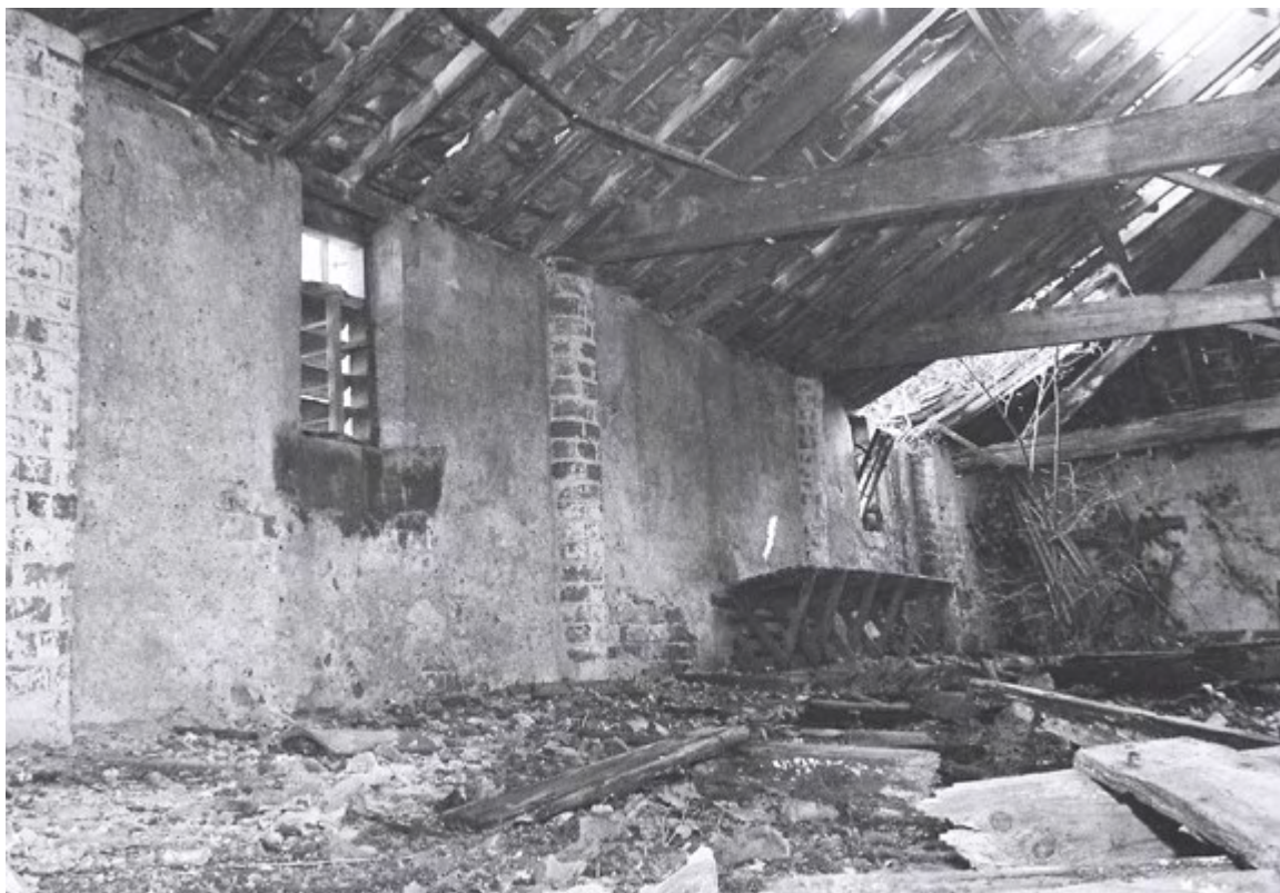
Plate 16. Cart Shed Interior: First Floor. Facing South-East.
