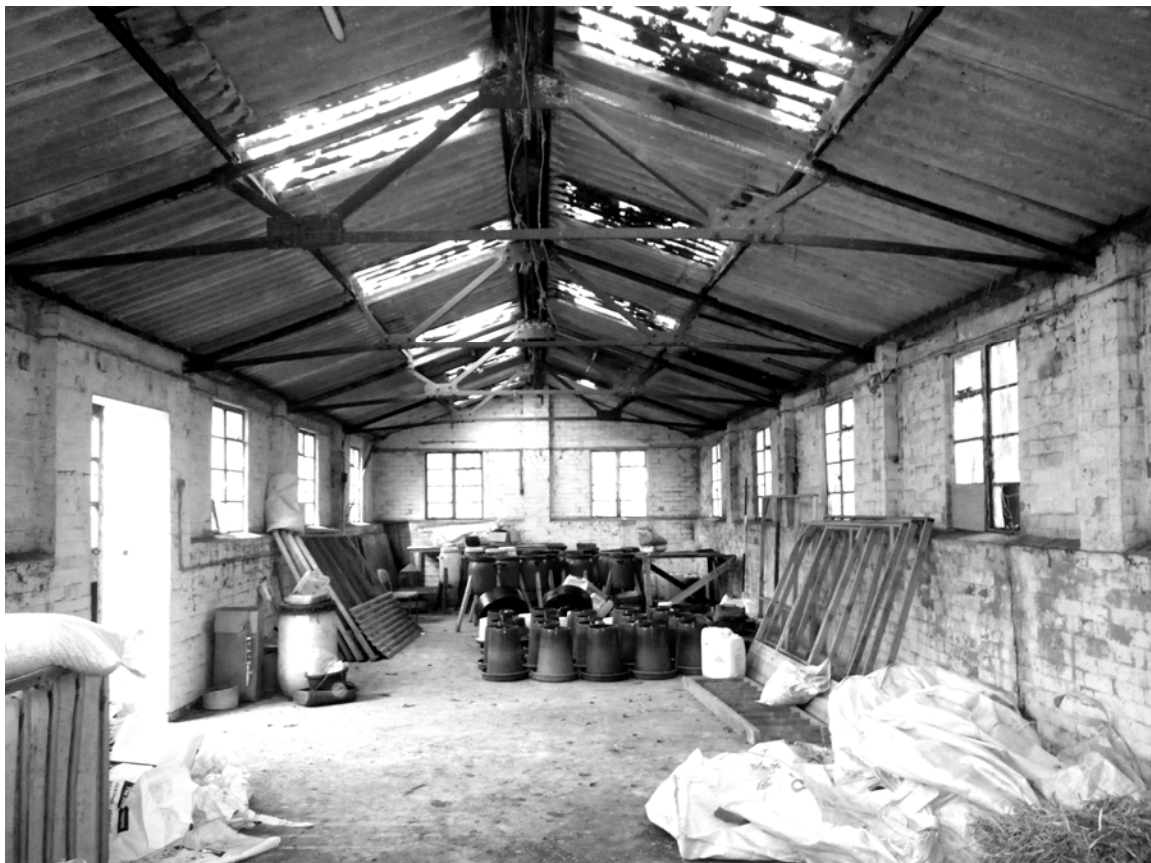
Plate. 26. Store Interior. Facing North.
