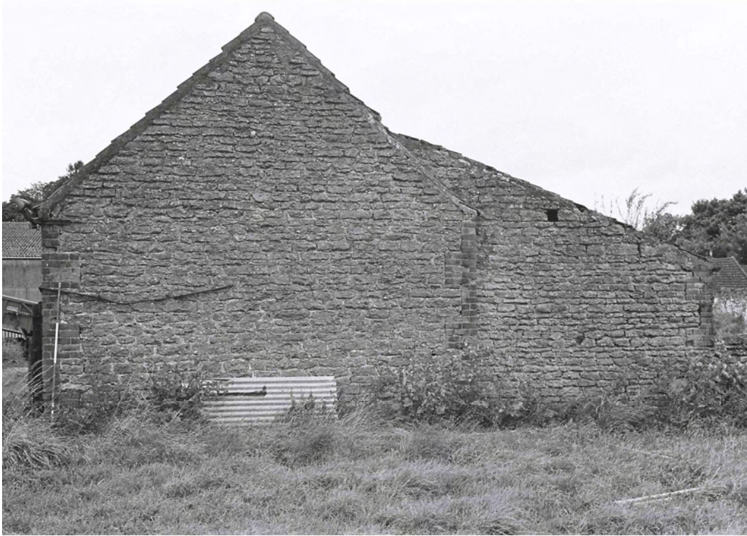
Plate 5. Building A Exterior: South Elevation. Facing North.
