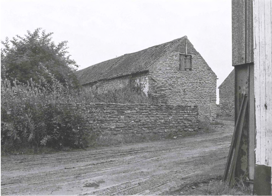
Plate 1. Building A Exterior. Facing South-west.
