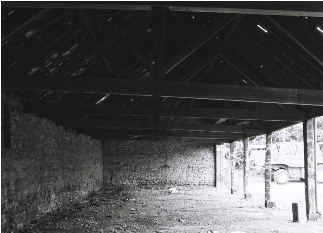
Plate 50. Building E Interior. Facing North.
