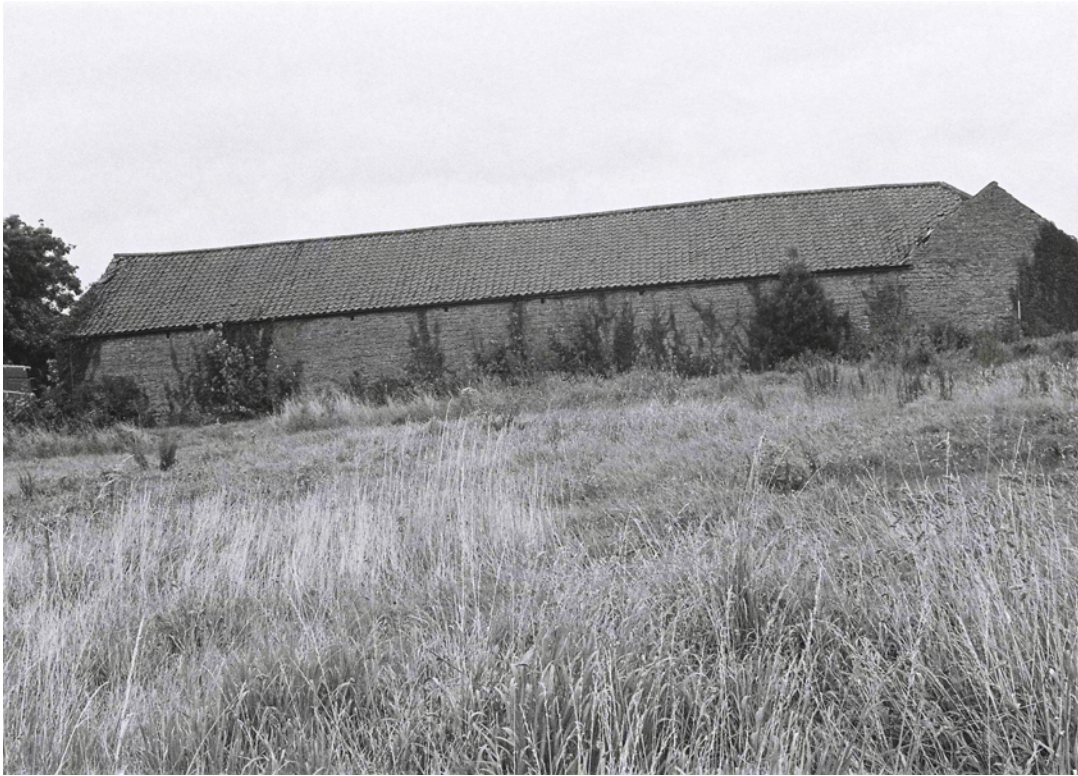
Plate 47. Building E Exterior: West Elevation. Facing East.
