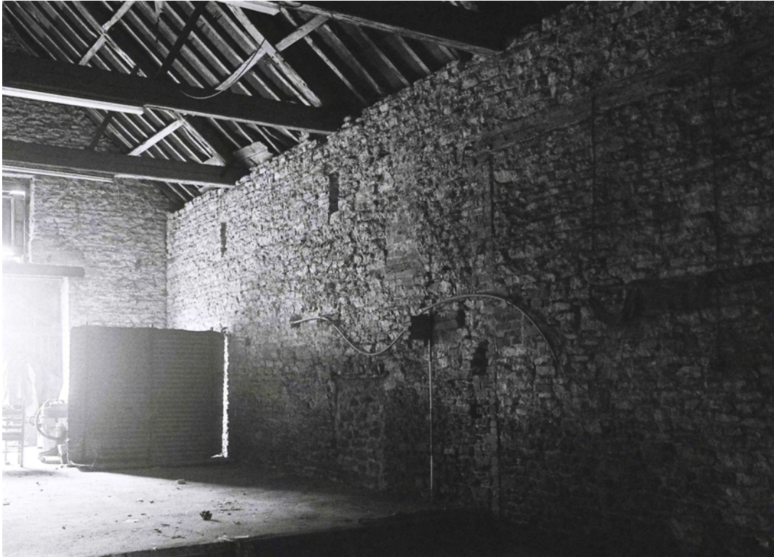
Plate 43. Building D Interior. Facing North-west.
