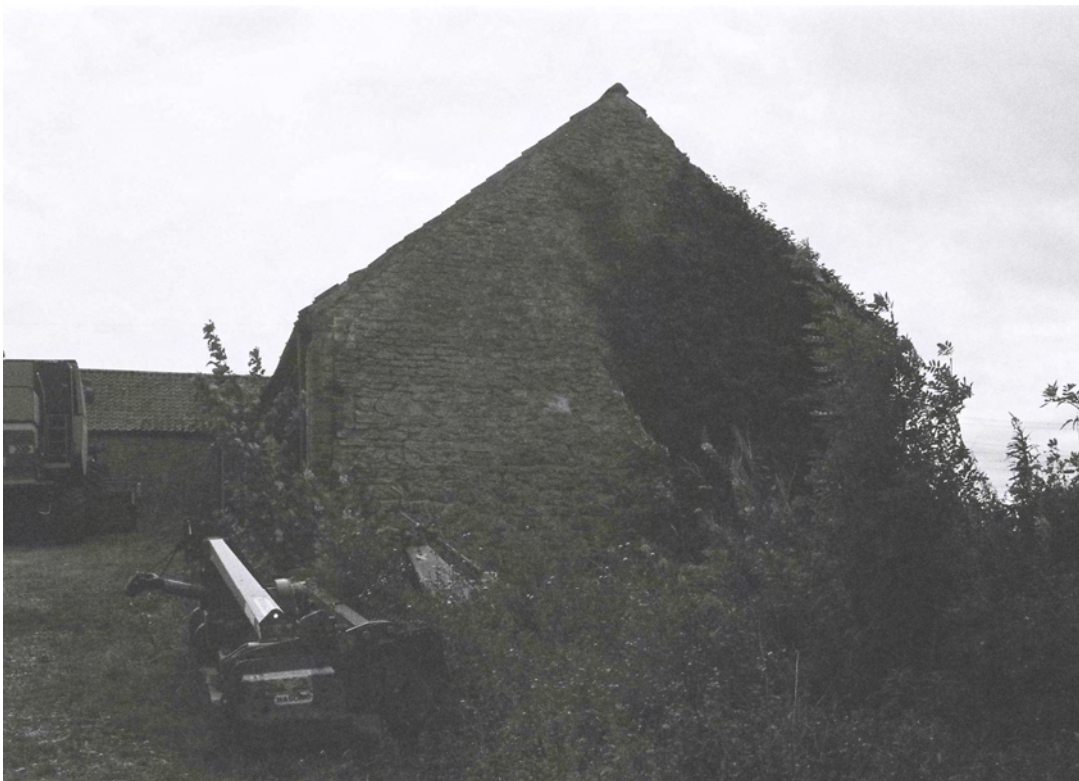
Plate 46. Building D Exterior: North Elevation. Facing South.
