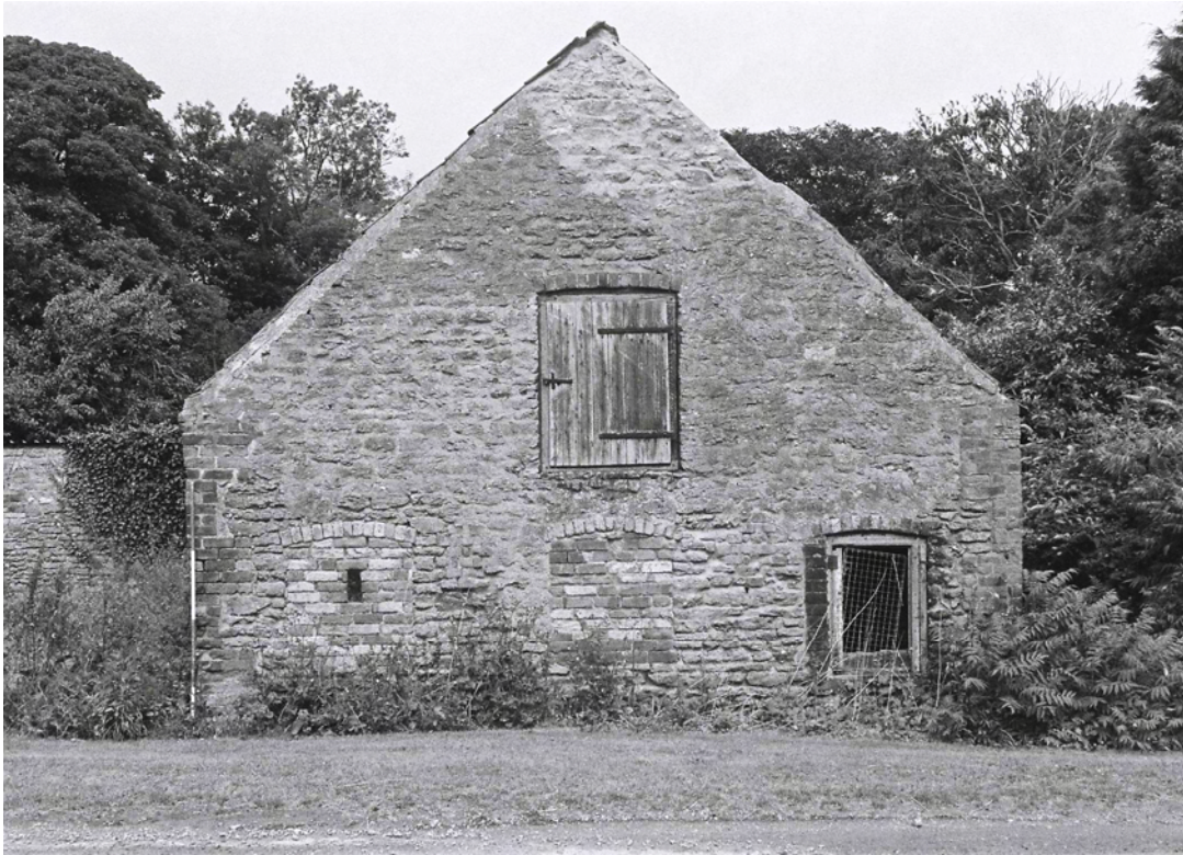
Plate 29. Building C Exterior: South Elevation. Facing North.
