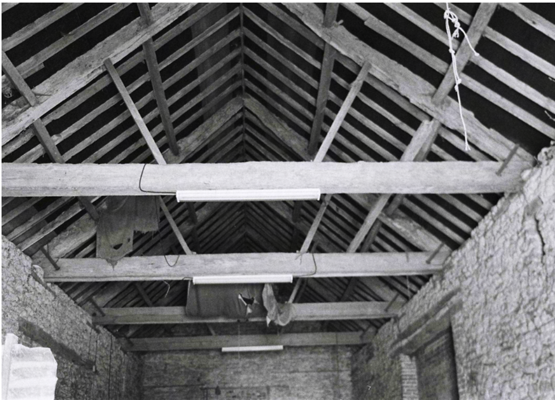
Plate 44. Building D Interior. Facing East.
