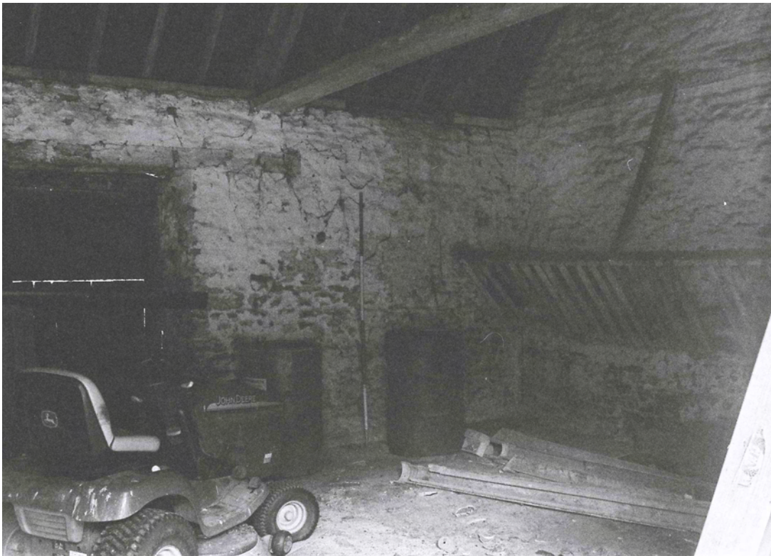
Plate 32. Building C Interior. Facing North-west.
