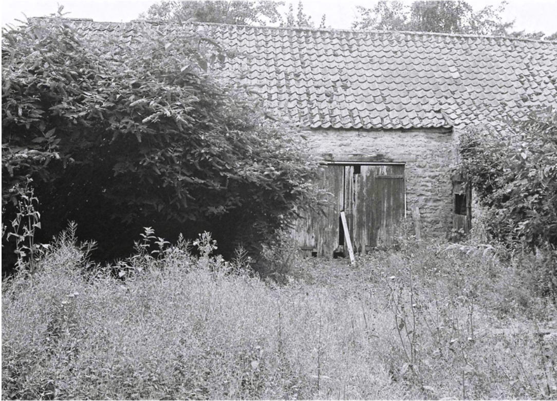
Plate 31. Building C Exterior: East Elevation. Facing West.
