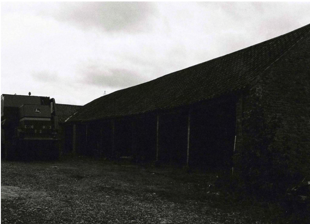
Plate 48. Building E Exterior: East Elevation. Facing South-west.
