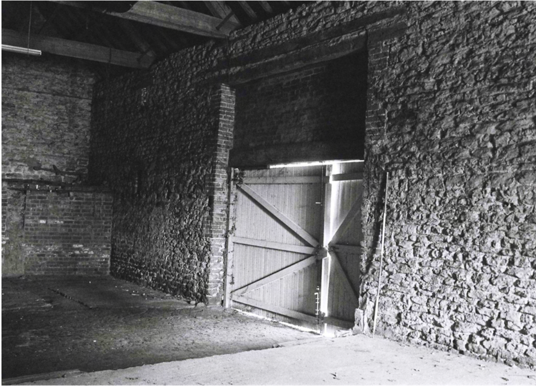
Plate 41. Building D Interior. Facing South-east.
