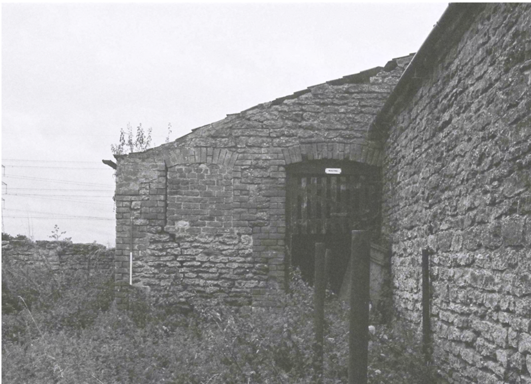
Plate 8. Building A Exterior: North Elevation. Facing South.
