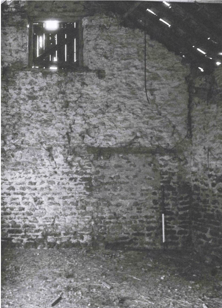
Plate 13. Building A Interior. Facing North.
