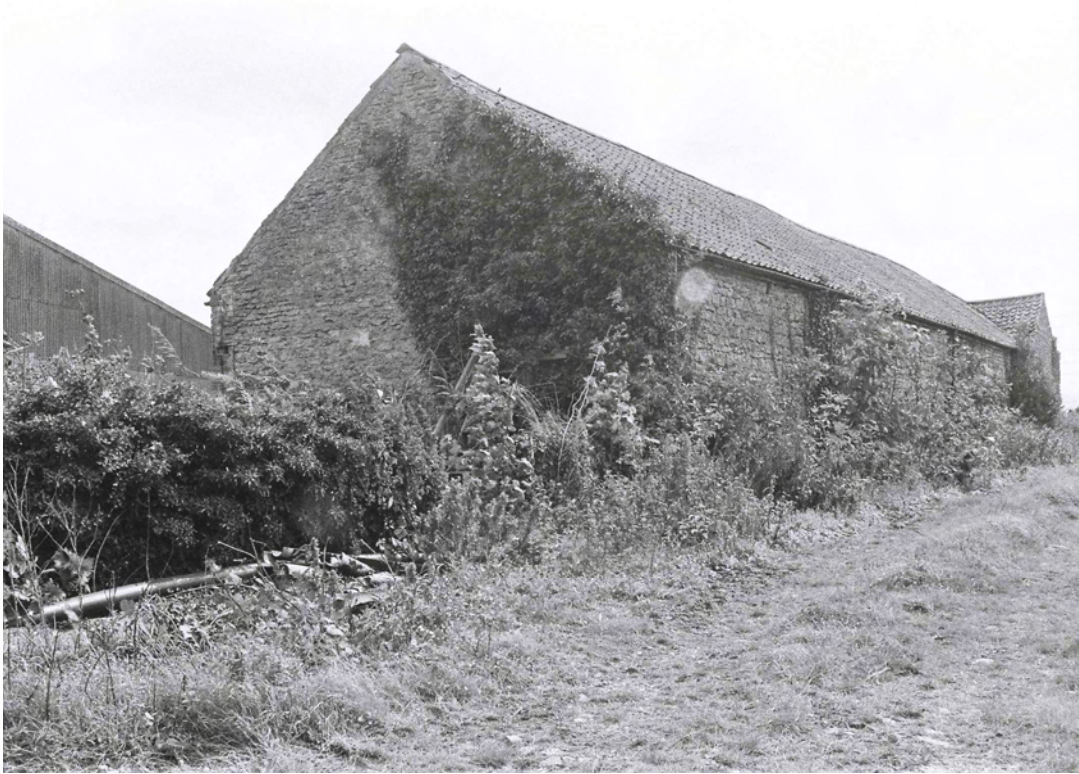
Plate 45. Building E Exterior: North and West Elevations. Facing South-east.
