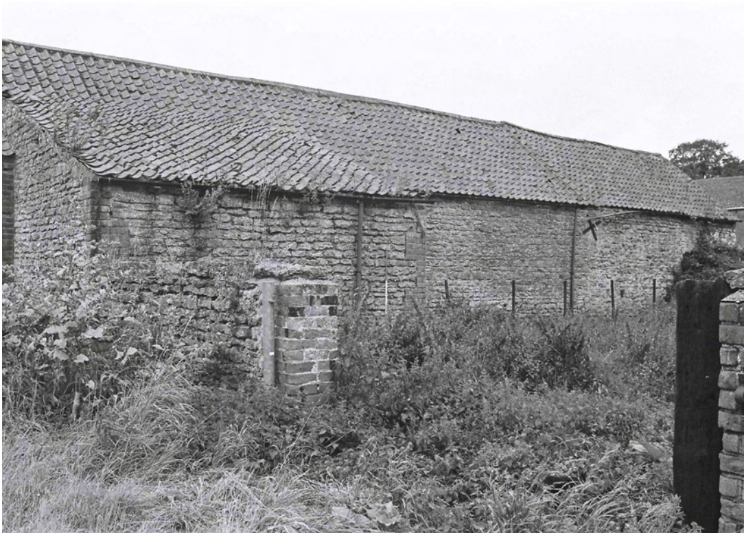
Plate 6. Building A Exterior: East Elevation. Facing North-west.
