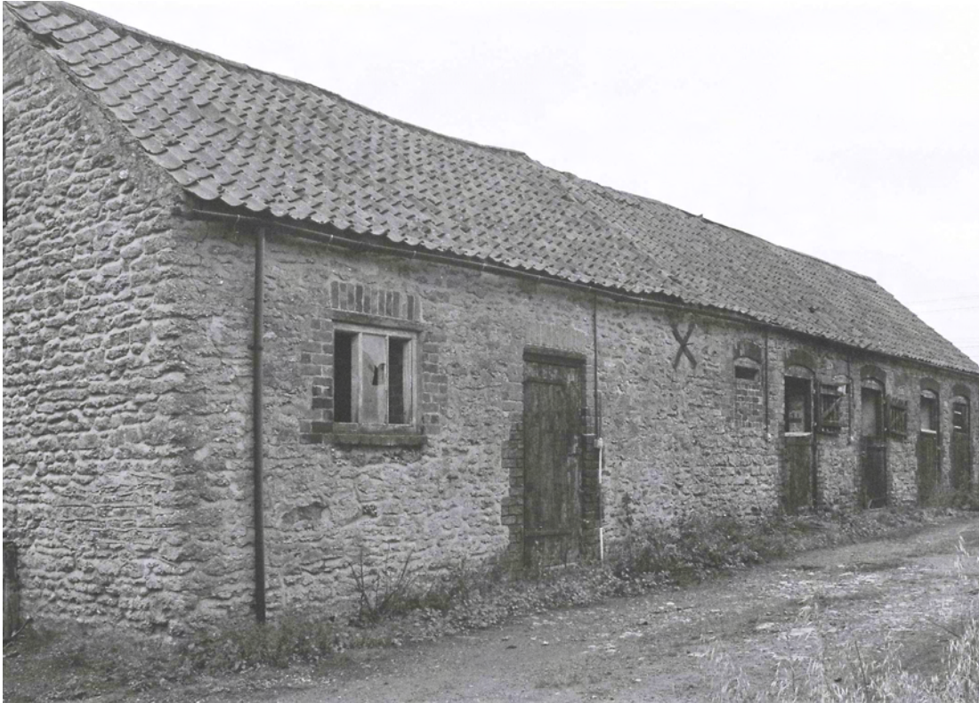
Plate 3. Building A Exterior: West Elevation. Facing South-east.
