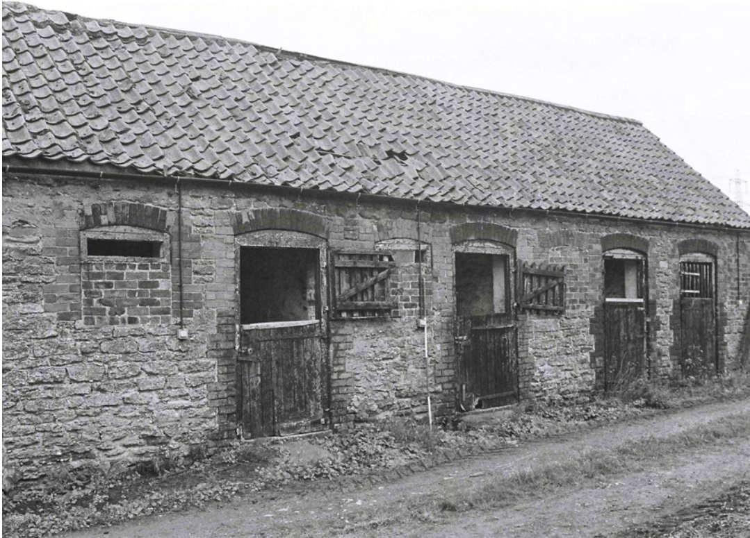
Plate 4. Building A Exterior: West Elevation. Facing South-east.
