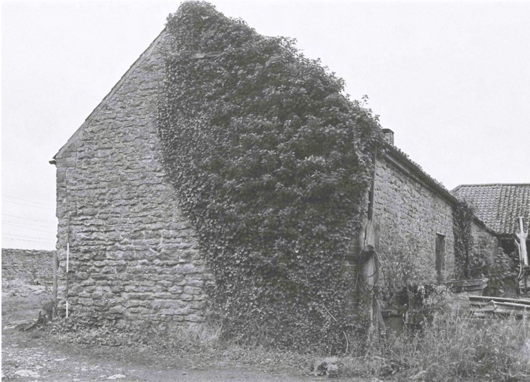
Plate 21. Building A Exterior: East Elevation. Facing West.
