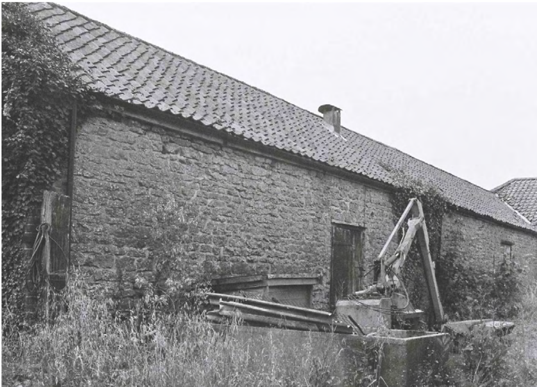
Plate 16. Building B Exterior: North Elevation. Facing South-west.
