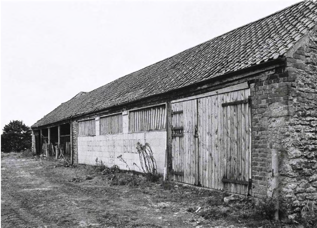
Plate 19. Building B Exterior: South Elevation. Facing North-west.
