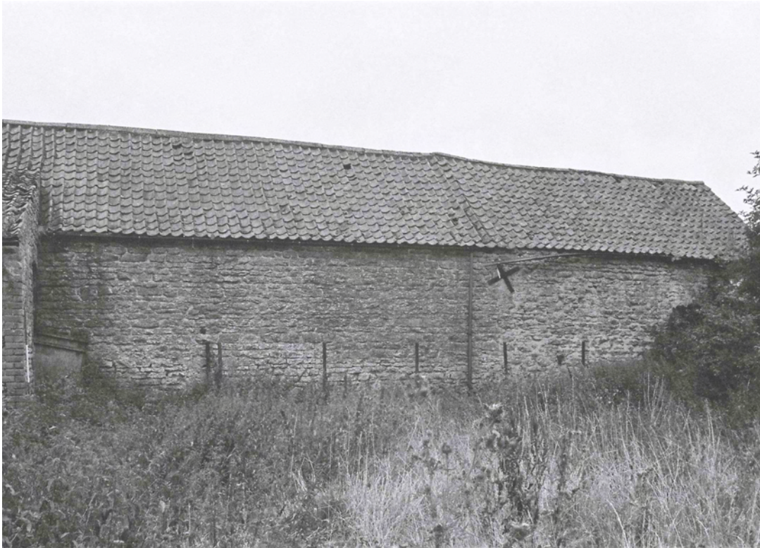
Plate 9. Building A Exterior: East Elevation. Facing West.
