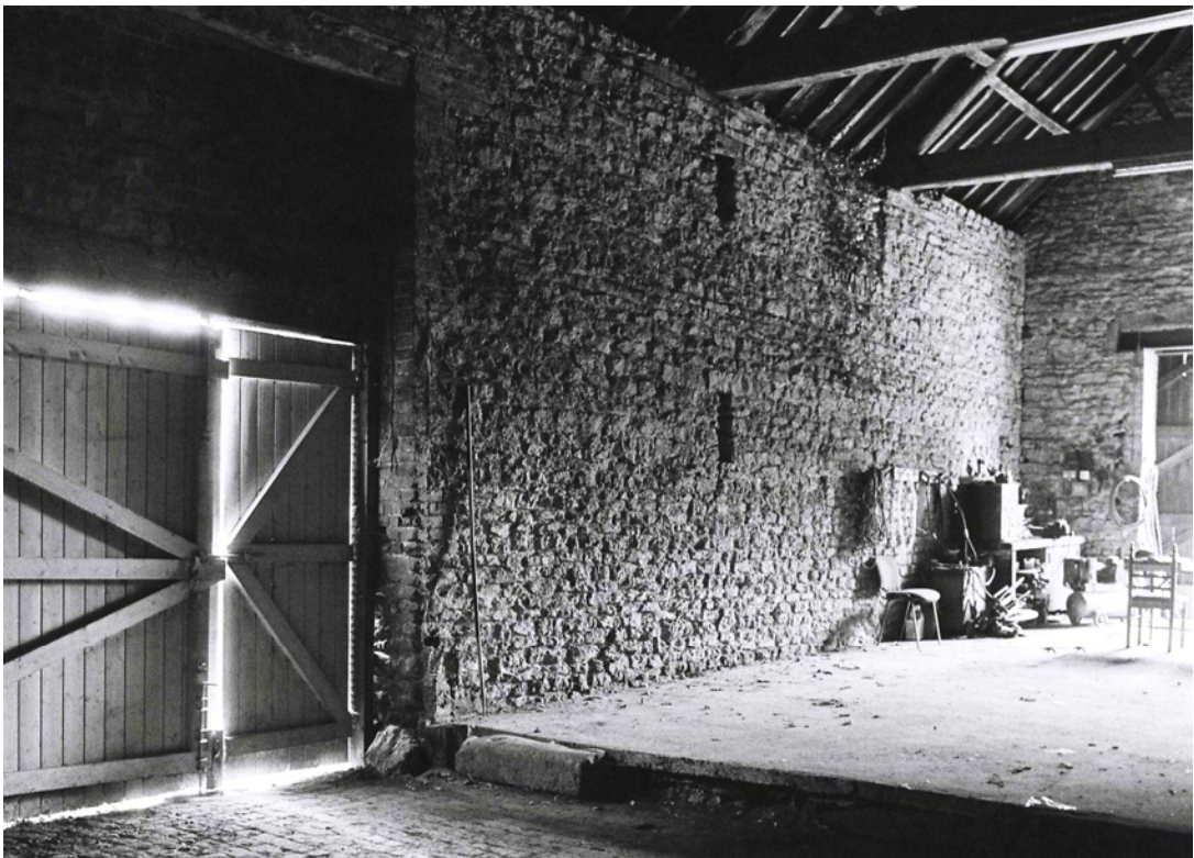
Plate 42. Building D Interior. Facing South-west.
