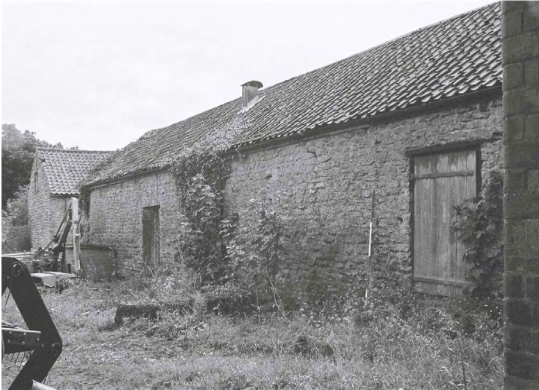
Plate 17. Building B Exterior: North Elevation. Facing South-east.
