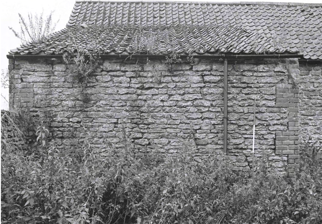
Plate 7. Building A Exterior: East Elevation. Facing West.
