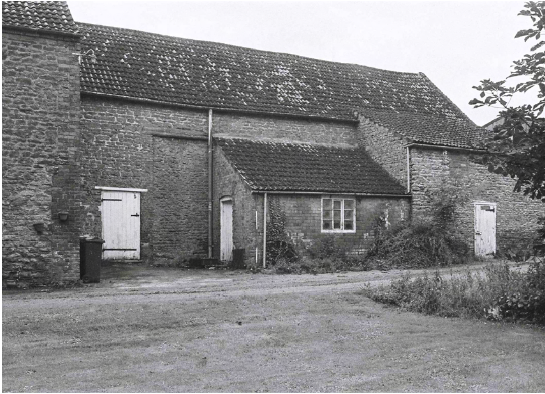
Plate 33. Building D Exterior: North Elevation. Facing South.
