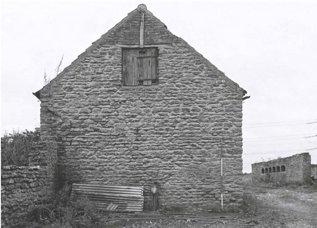
Plate 2. Building A Exterior: North Elevation. Facing South.
