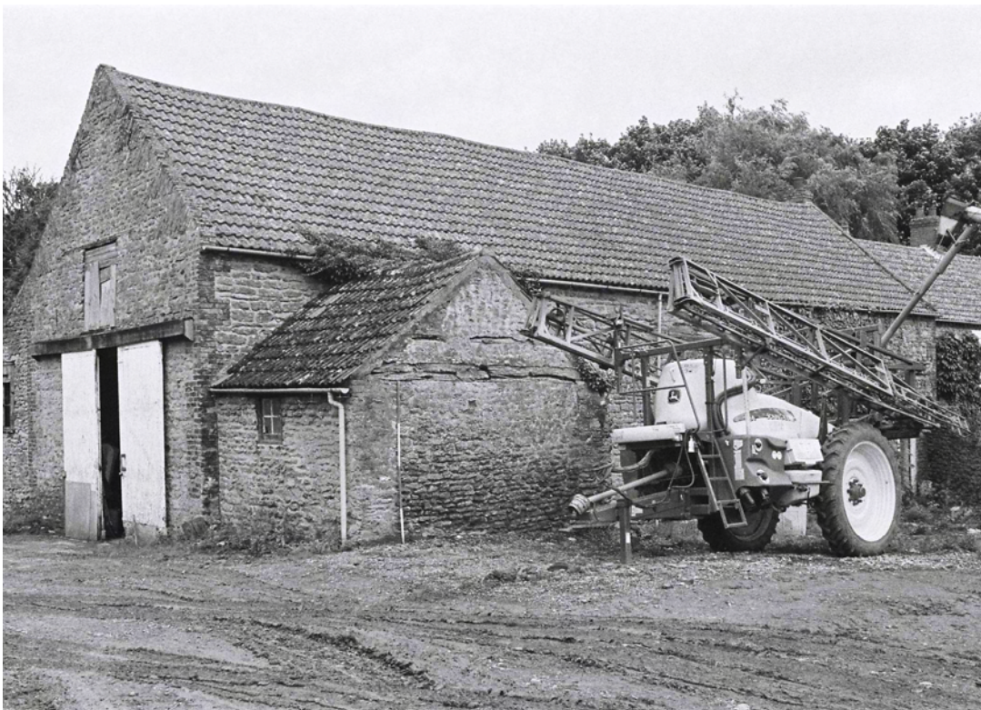
Plate 36. Building D Exterior: East and South Elevation. Facing North-east.
