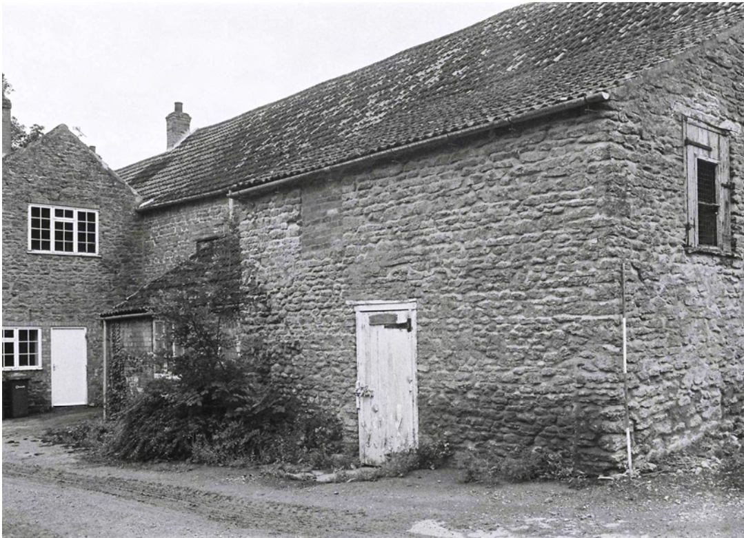
Plate 34. Building D Exterior: North Elevation. Facing South-east.
