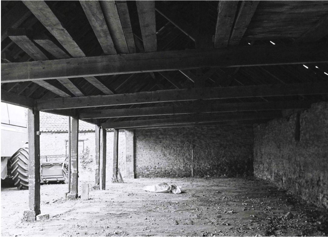
Plate 49. Building E Interior. Facing South.
