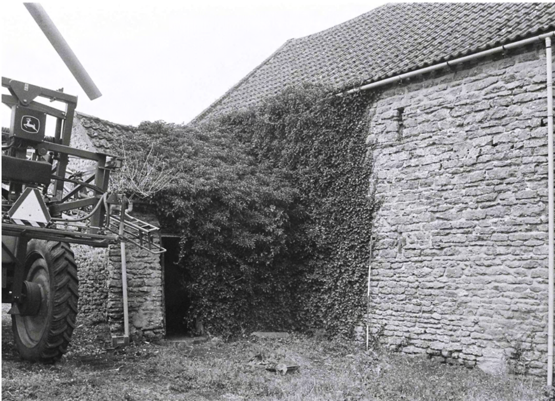
Plate 38. Building D Exterior: East and South Elevations. Facing North-west.
