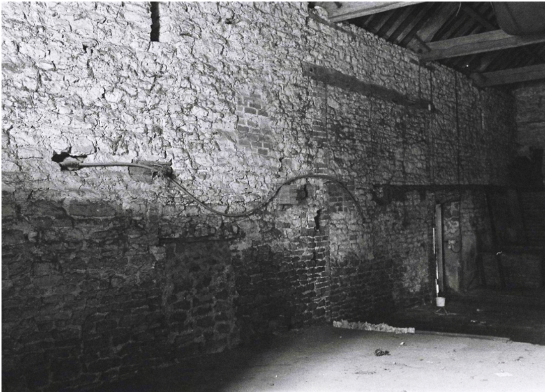
Plate 40. Building D Interior. Facing North-east.
