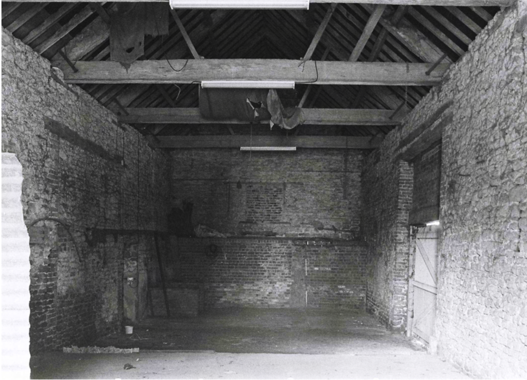
Plate 39. Building D Interior. Facing East.
