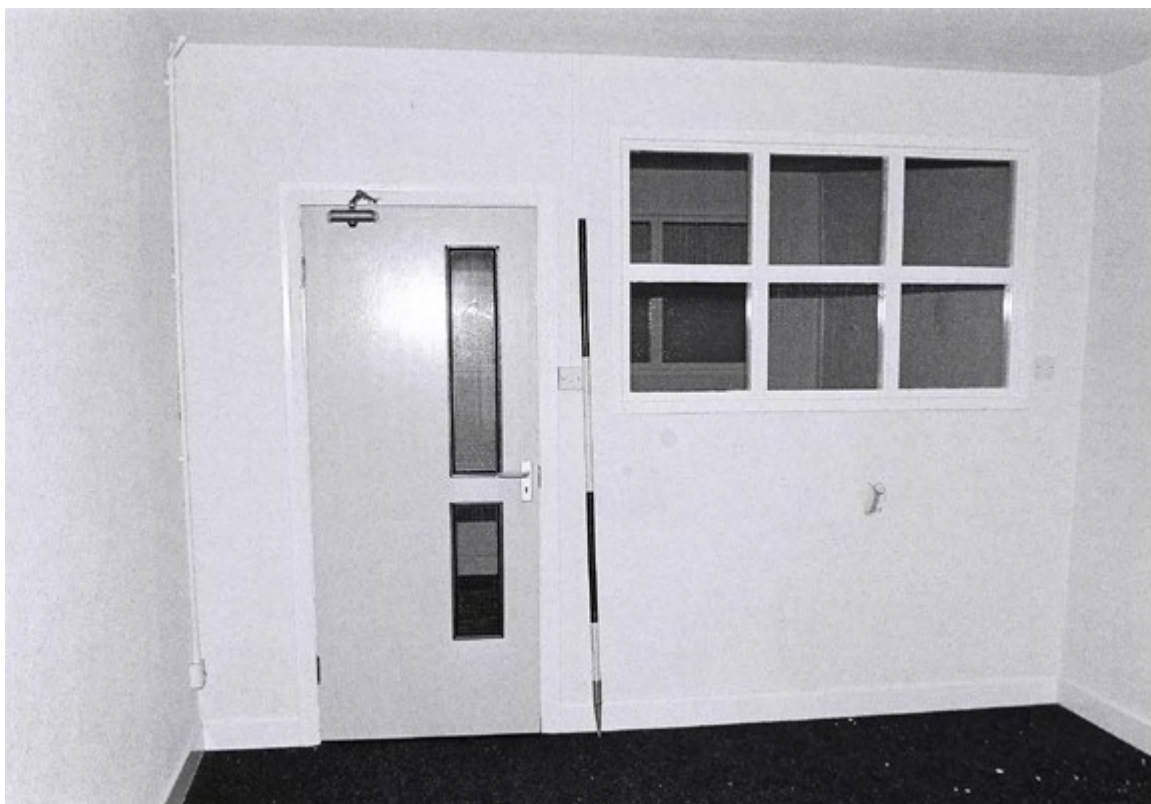
Plate 22. Barn Interior: First Floor. Facing North.
