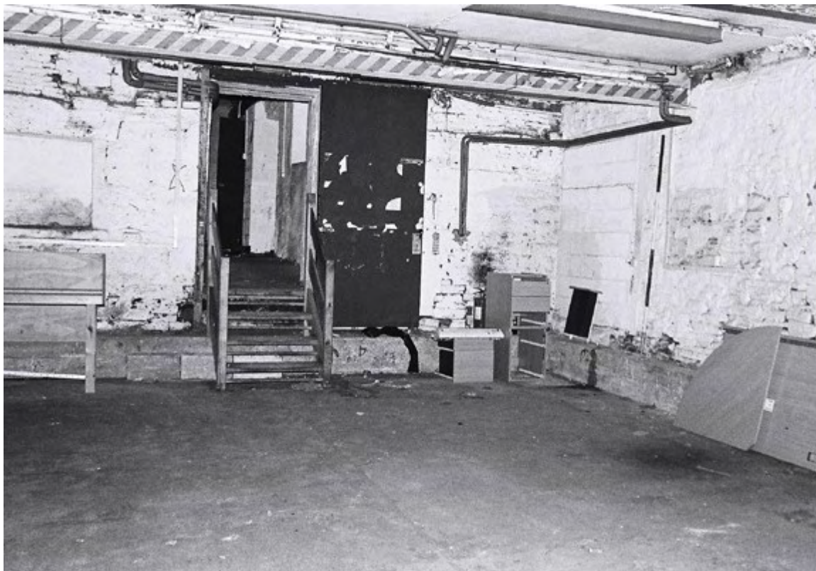
Plate 18. Barn Interior: Ground Floor. Facing East.
