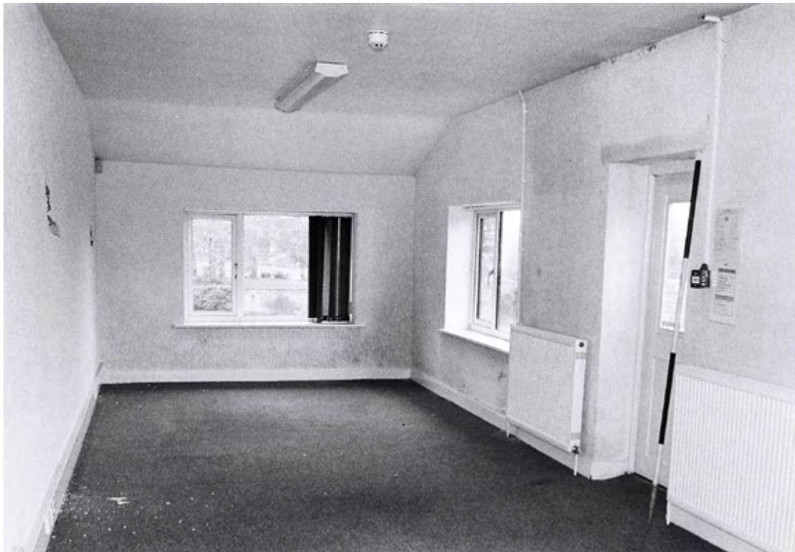
Plate 30. Barn Interior: First Floor. Facing South.
