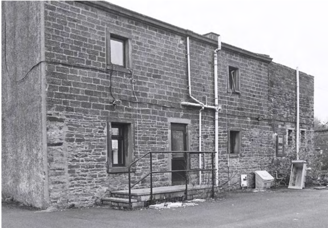
Plate 35. Cottage Exterior: West Elevation. Facing South-east.
