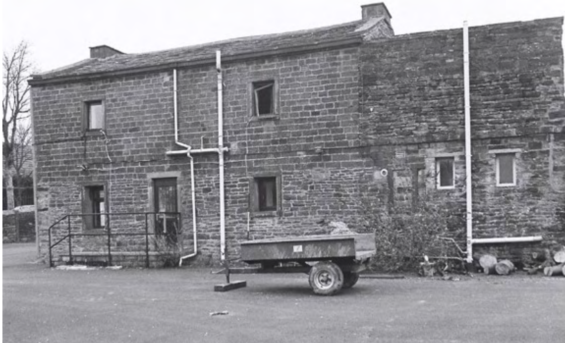
Plate 36. Cottage Exterior: West Elevation. Facing East.
