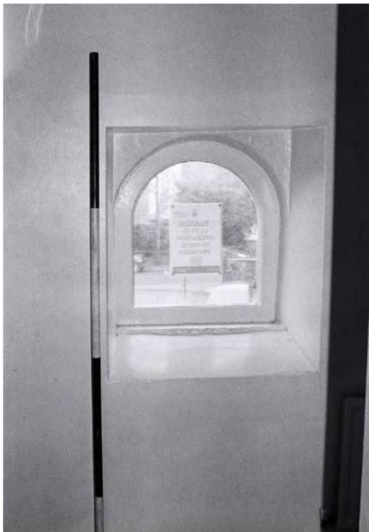
Plate 24. Barn Interior: First Floor. Facing North.
