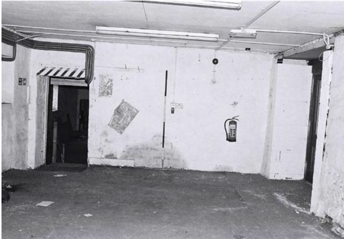
Plate 13. Barn Interior: Ground Floor. Facing East.
