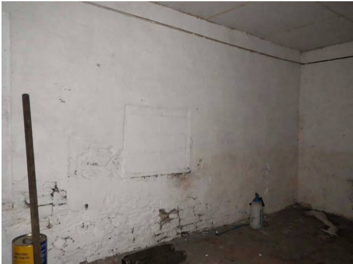
Plate 20. Barn Interior: Ground Floor. Facing South-west.
