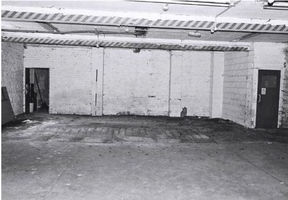
Plate 15. Barn Interior: Ground Floor. Facing West.
