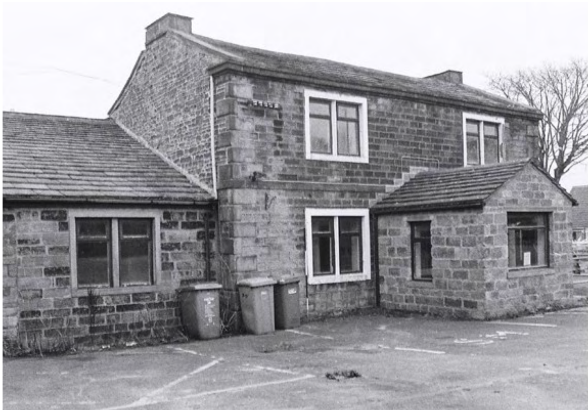
Plate 32. Cottage Exterior: East Elevation. Facing North-west.
