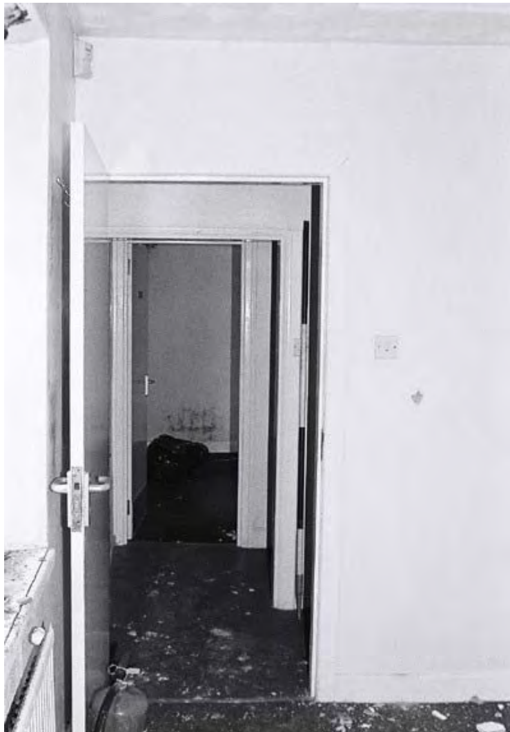
Plate 46. Cottage Interior: First Floor. Facing South.
