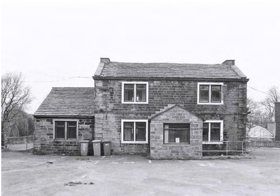
Plate 31. Cottage Exterior: East Elevation. Facing West.
