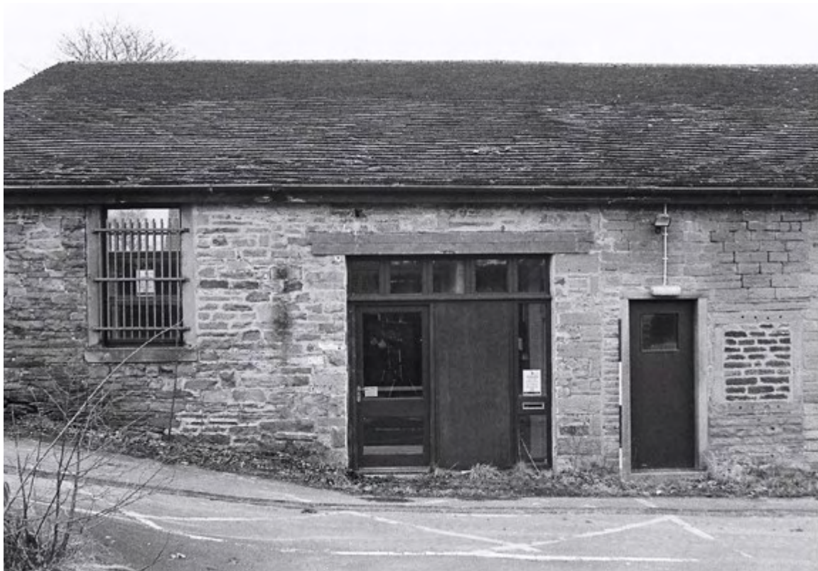
Plate 4. Barn Exterior: North Elevation. Facing South.
