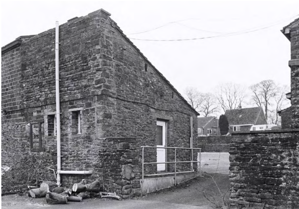
Plate 38. Cottage Exterior: West and South Elevations. Facing North-east.
