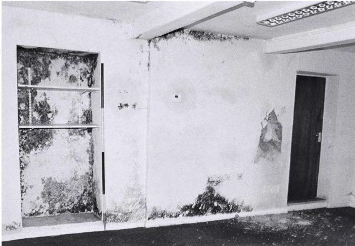
Plate 39. Cottage Interior: Ground Floor. Facing South.
