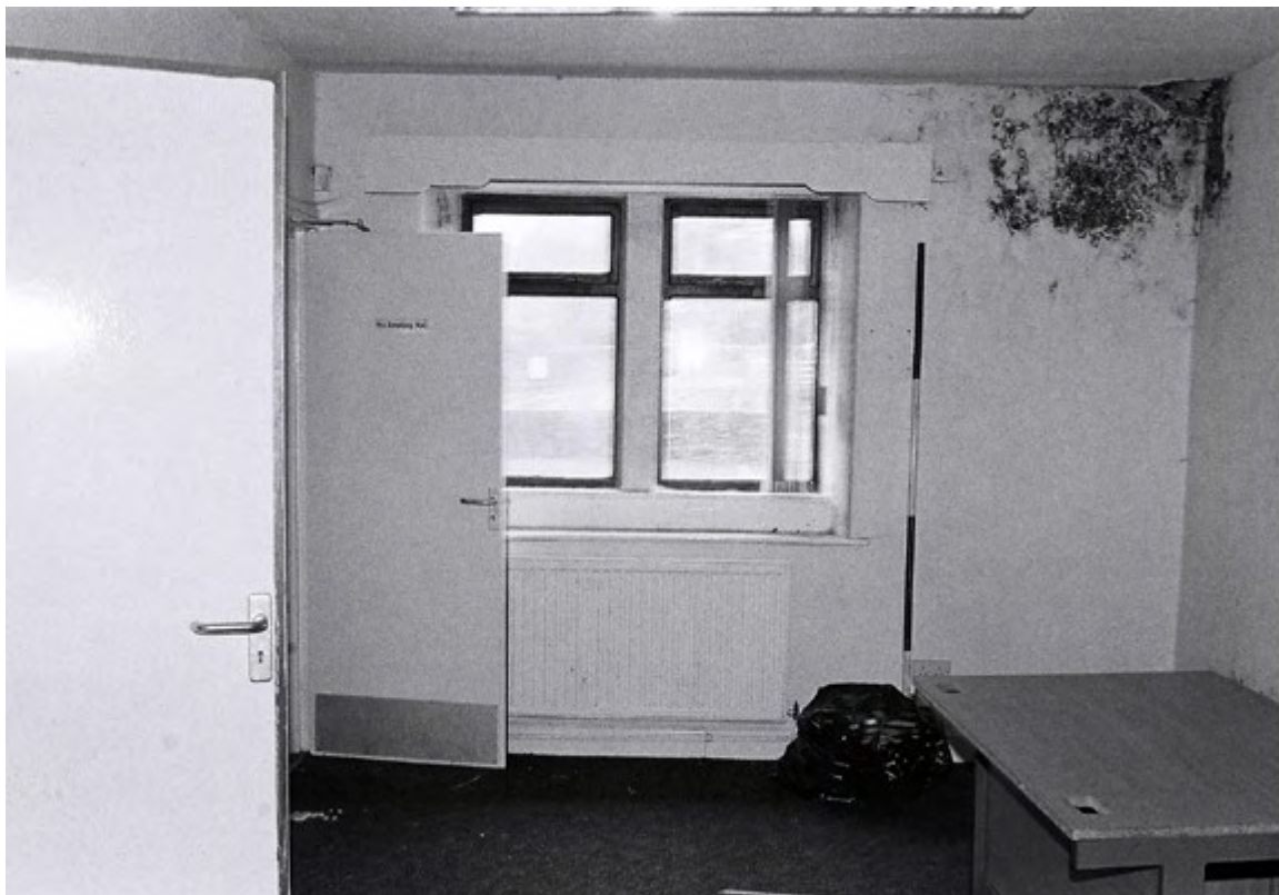
Plate 44. Cottage Interior: First Floor. Facing East.
