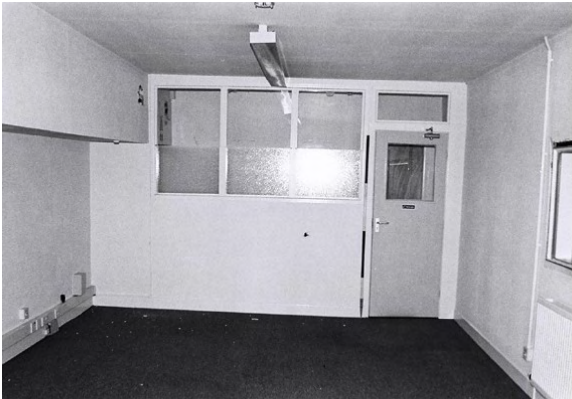
Plate 25. Barn Interior: First Floor. Facing North.
