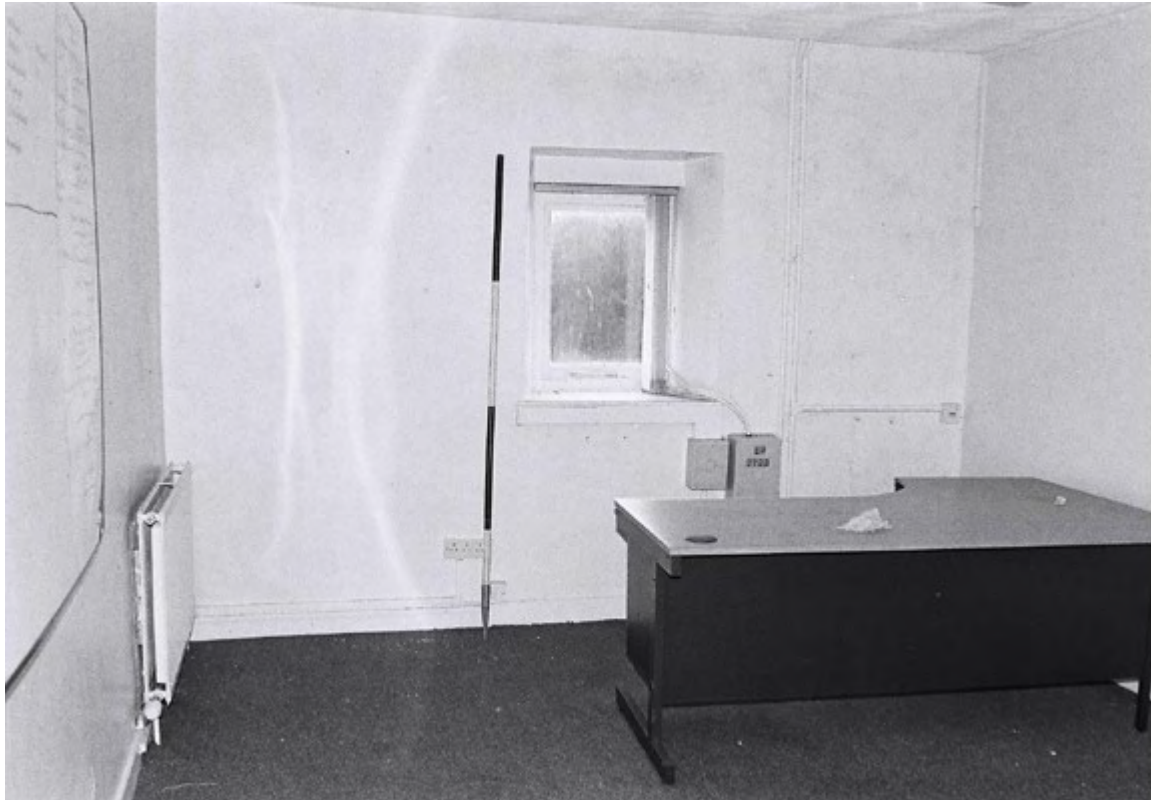
Plate 43. Cottage Interior: First Floor. Facing West.
