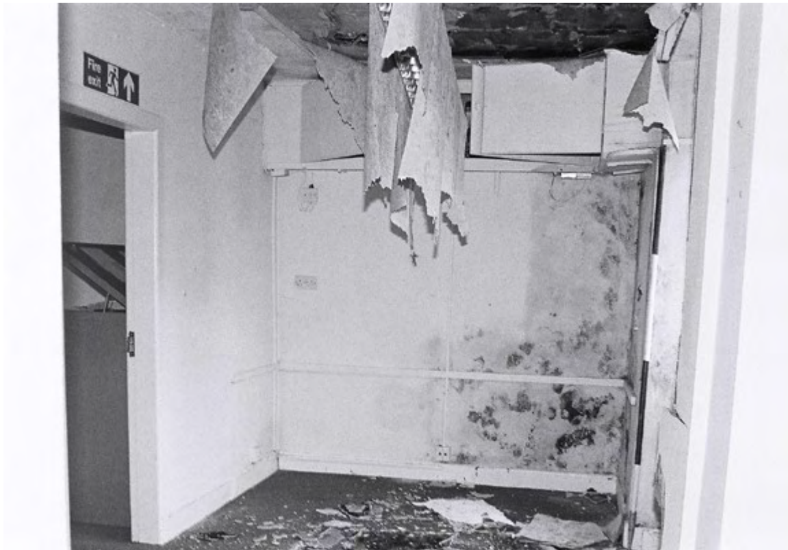
Plate 40. Cottage Interior: Ground Floor. Facing North.
