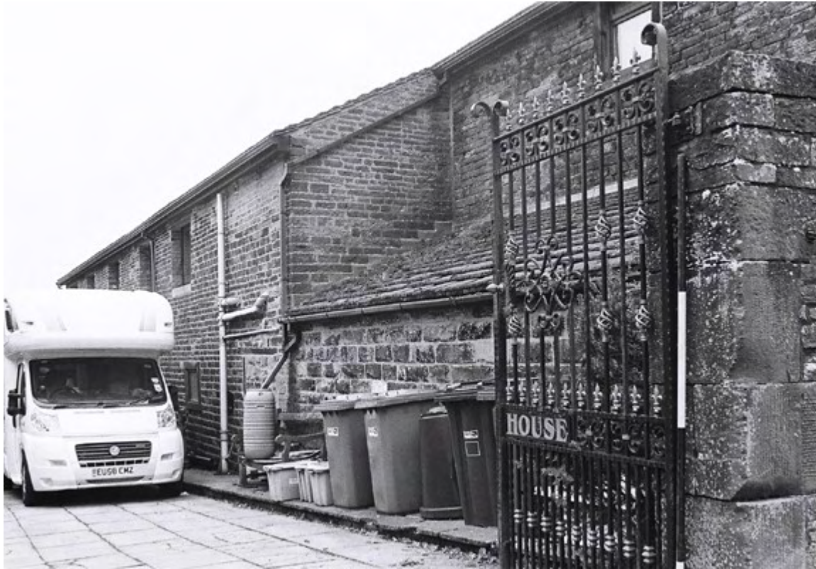
Plate 9. Barn Exterior: South Elevation. Facing North-west.
