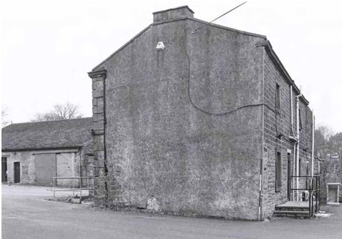
Plate 34. Cottage Exterior: North Elevation. Facing South.
