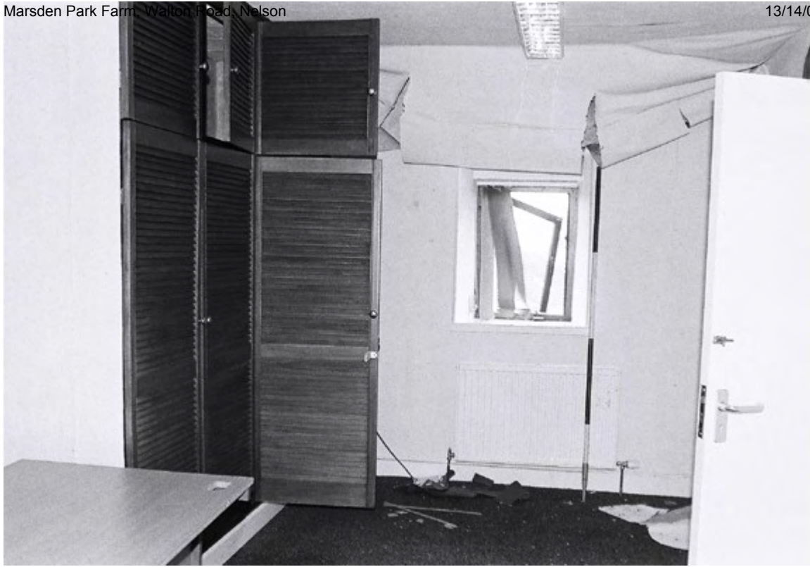
Plate 45. Cottage Interior: First Floor. Facing West.
