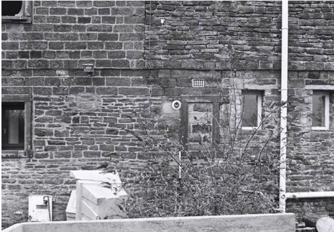
Plate 37. Cottage Exterior: West Elevation. Facing East.
