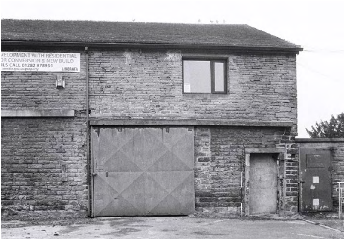
Plate 6. Barn Exterior: North Elevation. Facing South.
