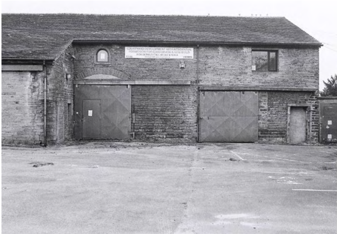
Plate 3. Barn Exterior: North Elevation. Facing South.
