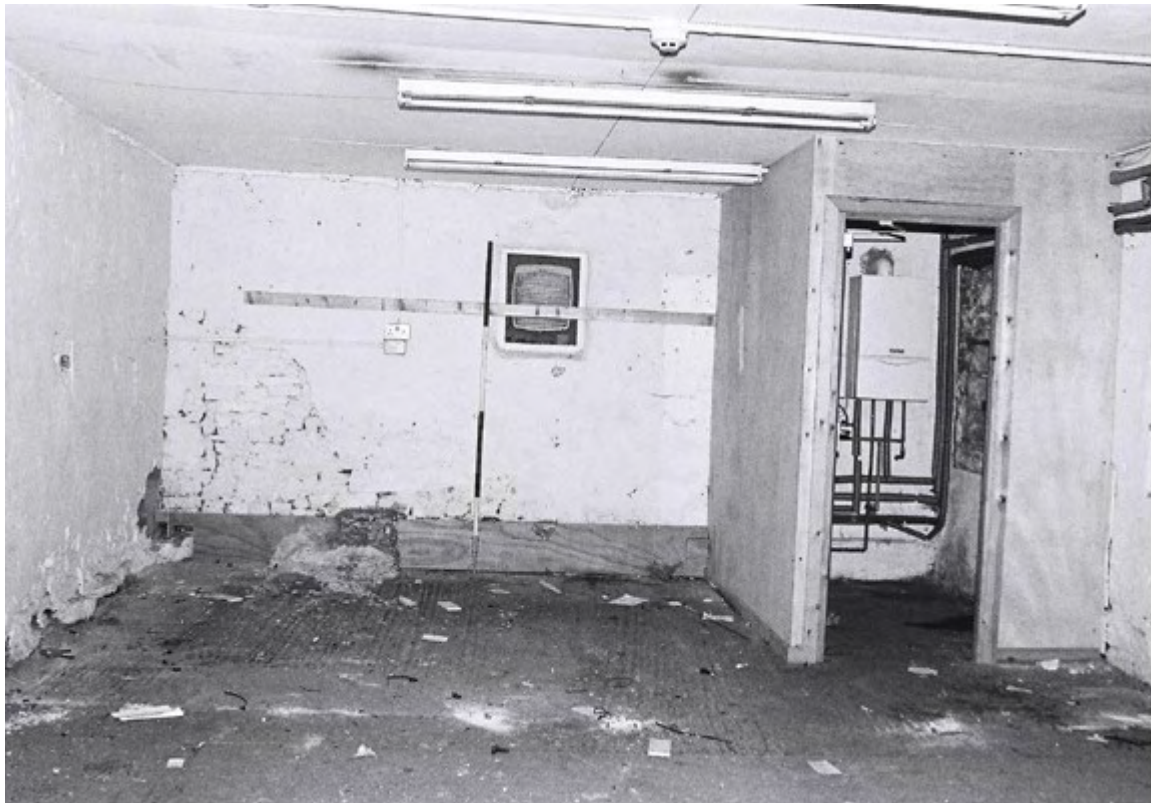
Plate 12. Barn Interior: Ground Floor. Facing East.
