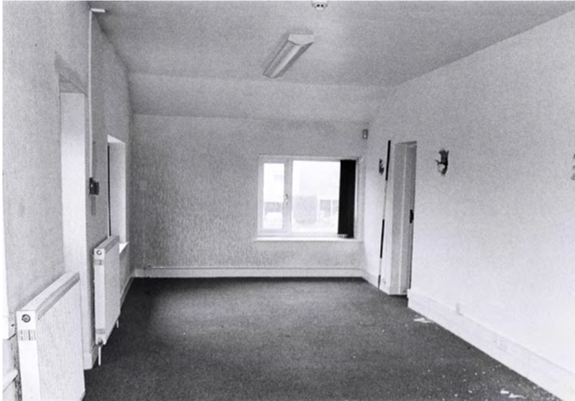
Plate 29. Barn Interior: First Floor. Facing North.
