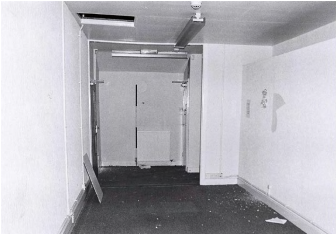
Plate 28. Barn Interior: First Floor. Facing North.
