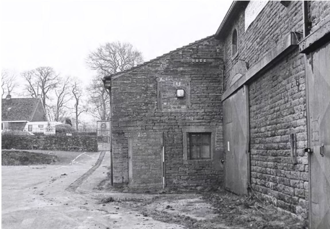
Plate 7. Barn Exterior: West Elevation. Facing East.
