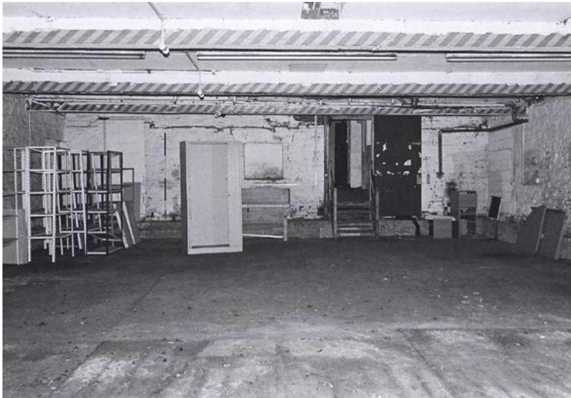
Plate 16. Barn Interior: Ground Floor. Facing East.
