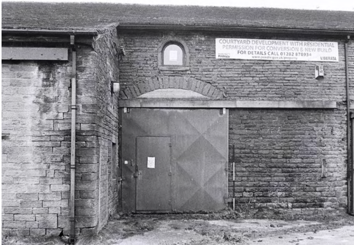
Plate 5. Barn Exterior: North Elevation. Facing South.
