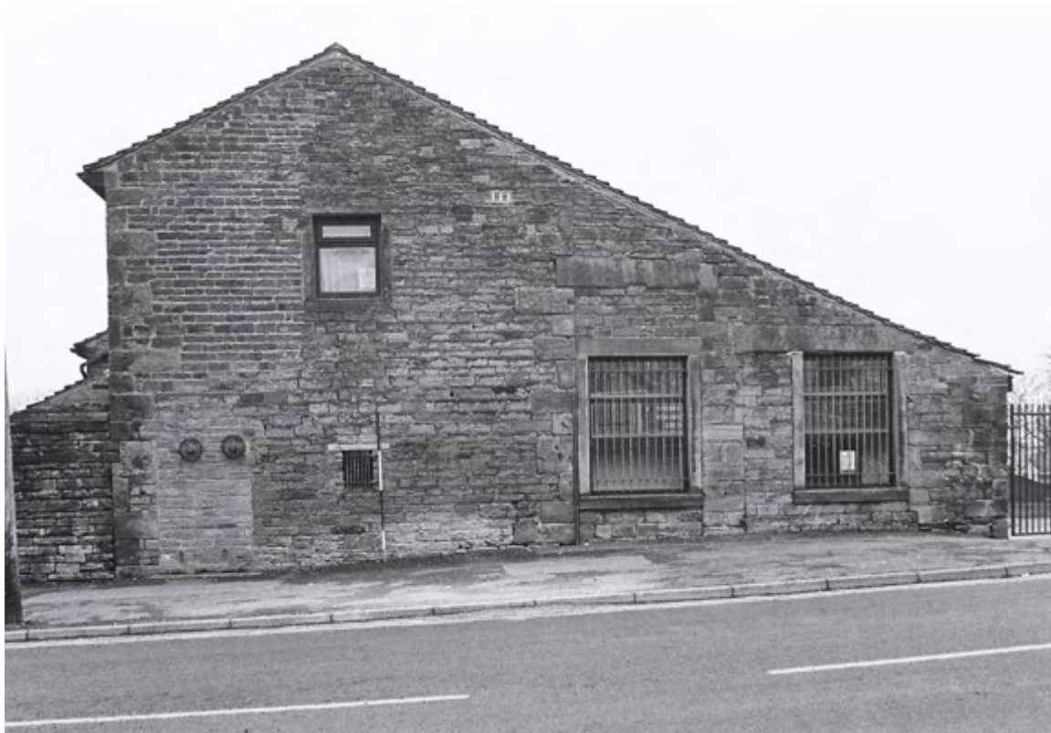
Plate 10. Barn Exterior: East Elevation. Facing West.
