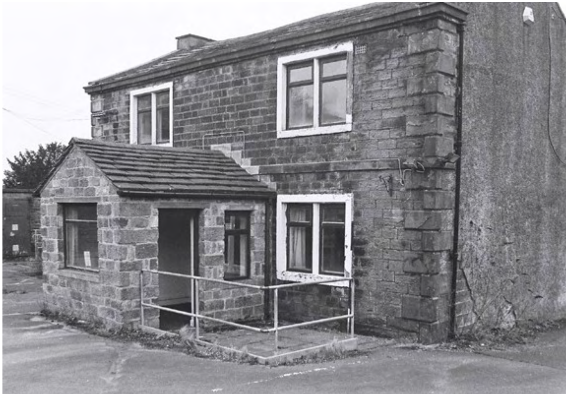
Plate 33. Cottage Exterior: East Elevation. Facing South-west.
