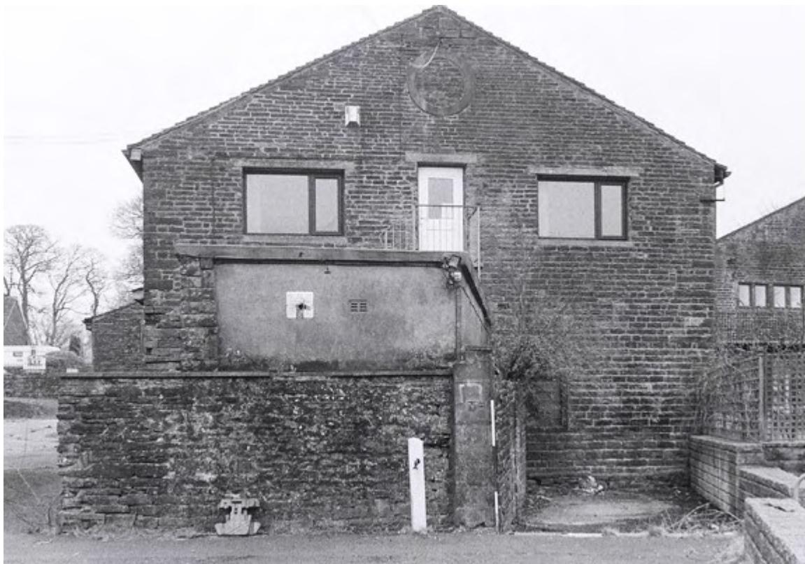
Plate 8. Barn Exterior: West Elevation. Facing East.
