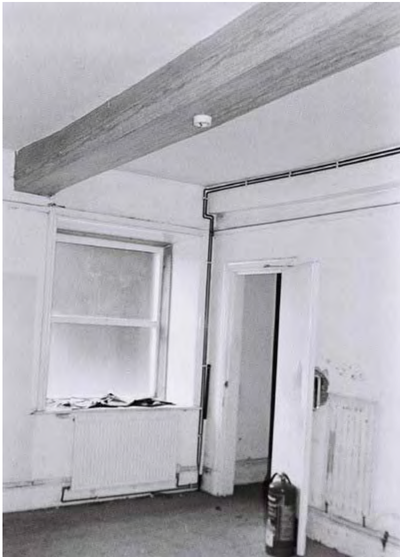
Plate 25. Marsden Park Cottage Interior. Ground Floor. Facing West.
