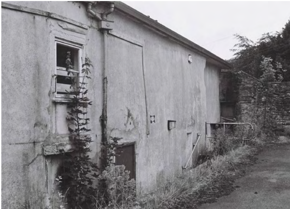
Plate 12. Marsden Park Cottage Exterior. Facing West.
