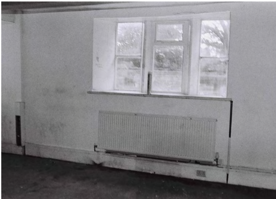
Plate 28. Marsden Park Cottage Interior. Ground Floor. Facing South.
