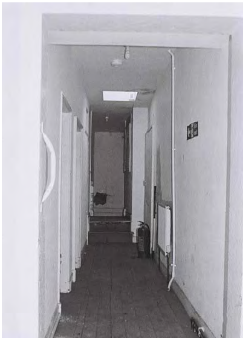
Plate 45. Marsden Park Cottage Interior. First Floor. Facing North-west.
