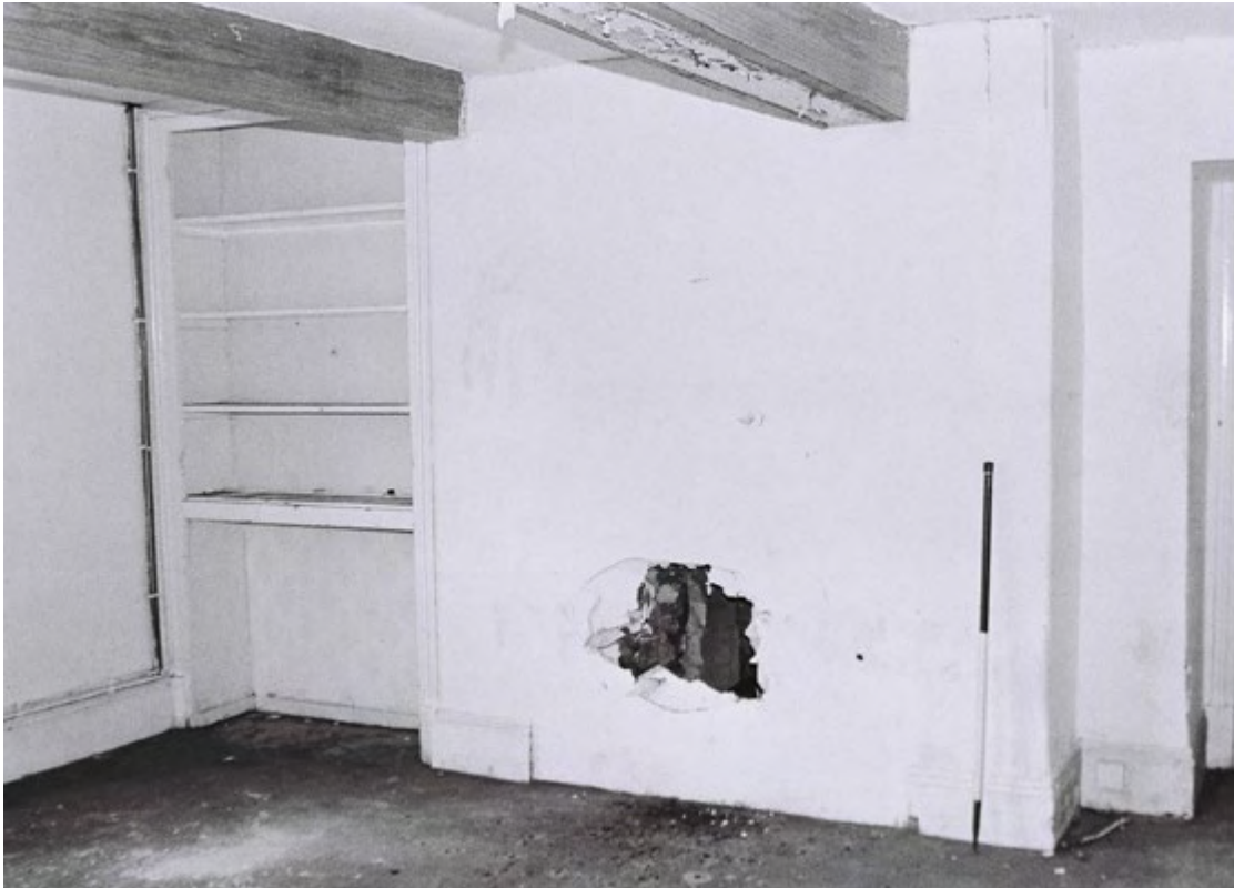
Plate 27. Marsden Park Cottage Interior. Ground Floor. Facing West.
