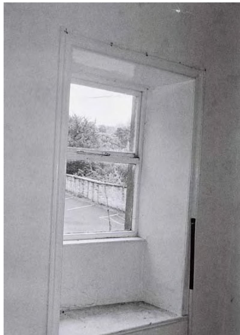
Plate 48. Marsden Park Cottage Interior. First Floor. Facing South-east.
