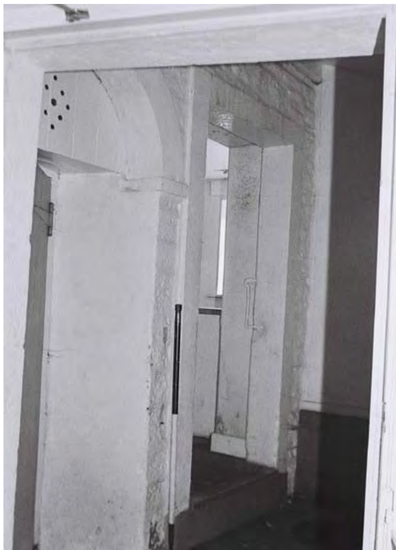
Plate 31. Marsden Park Cottage Interior. Ground Floor. Facing East.
