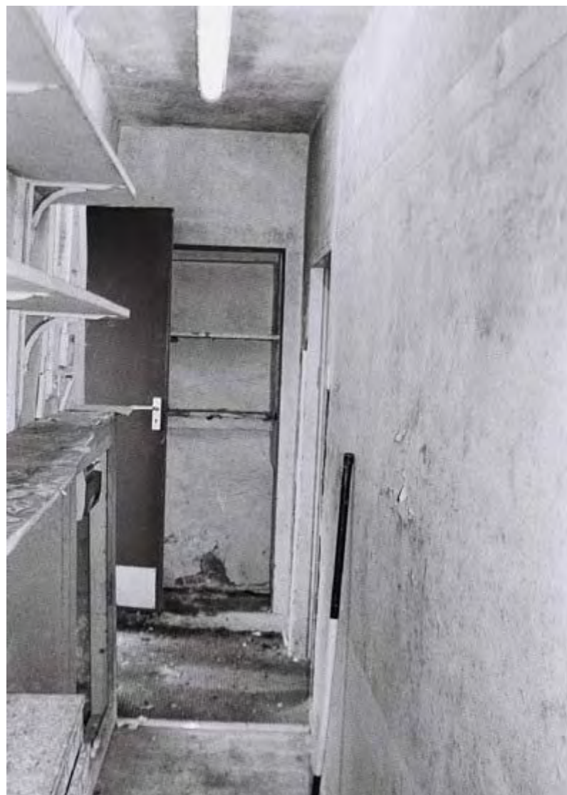
Plate 36. Marsden Park Cottage Interior. Ground Floor. Facing East.
