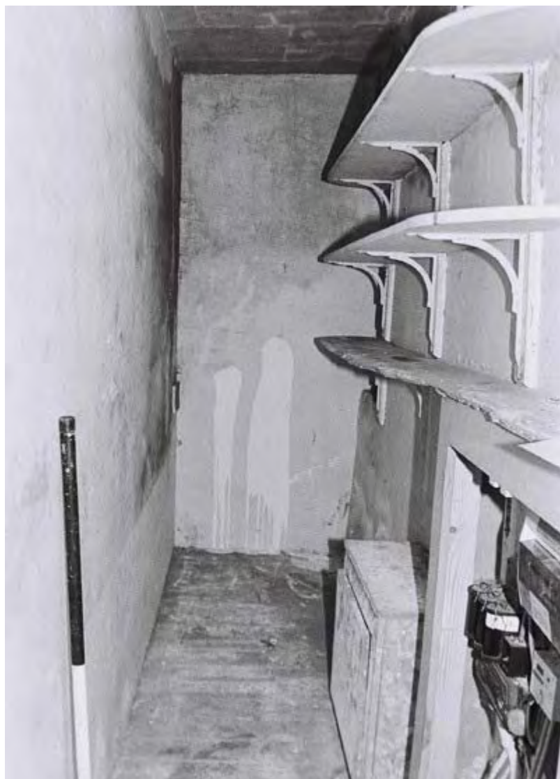
Plate 35. Marsden Park Cottage Interior. Ground Floor. Facing West.
