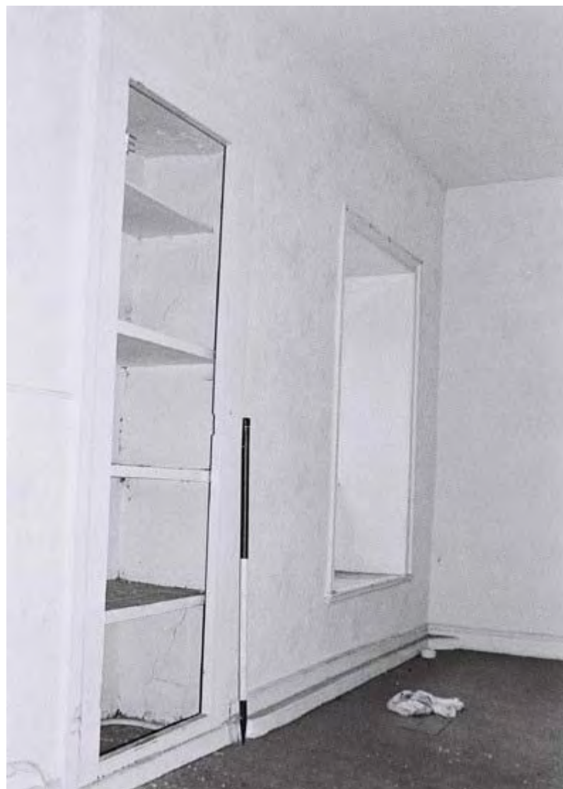
Plate 46. Marsden Park Cottage Interior. First Floor. Facing South.
