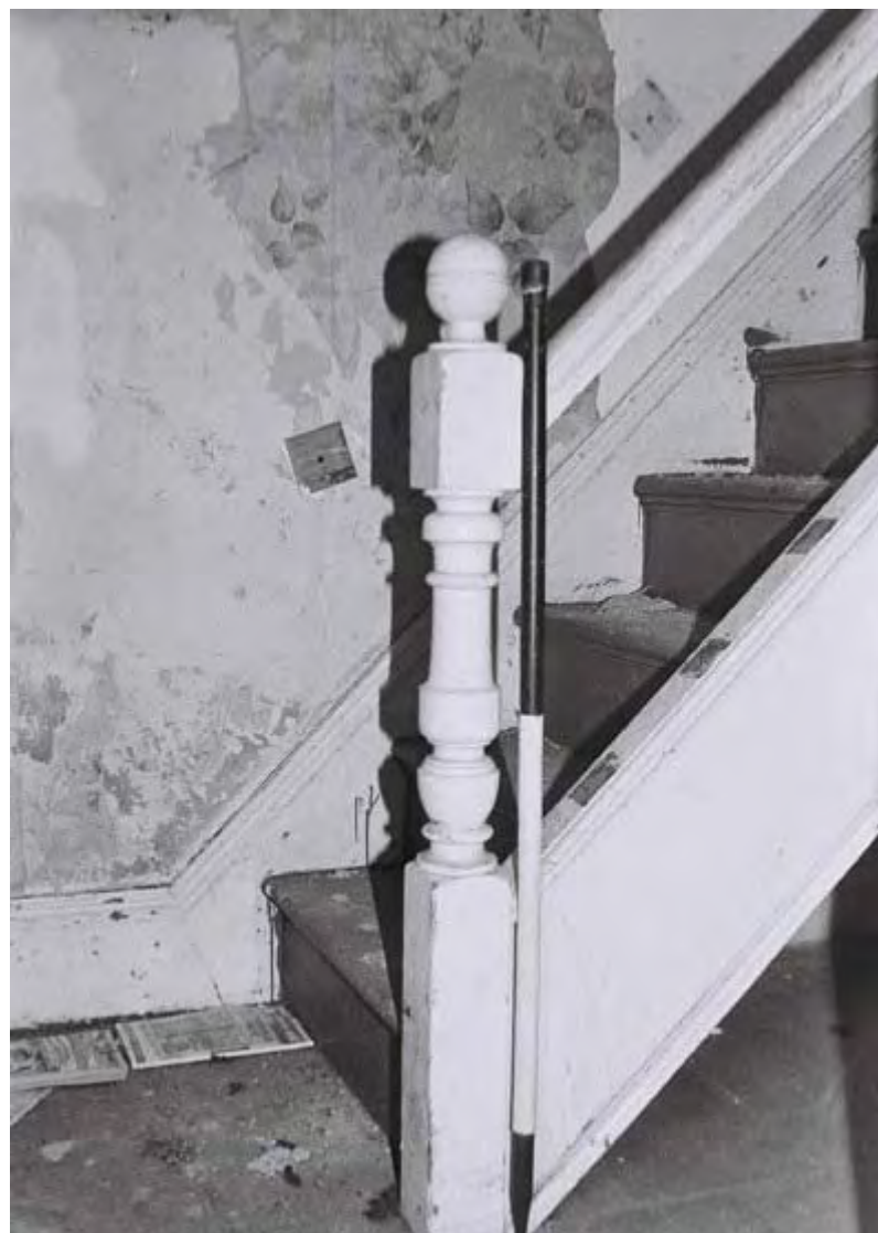
Plate 22. Marsden Park Cottage Interior. Ground Floor. Facing North.
