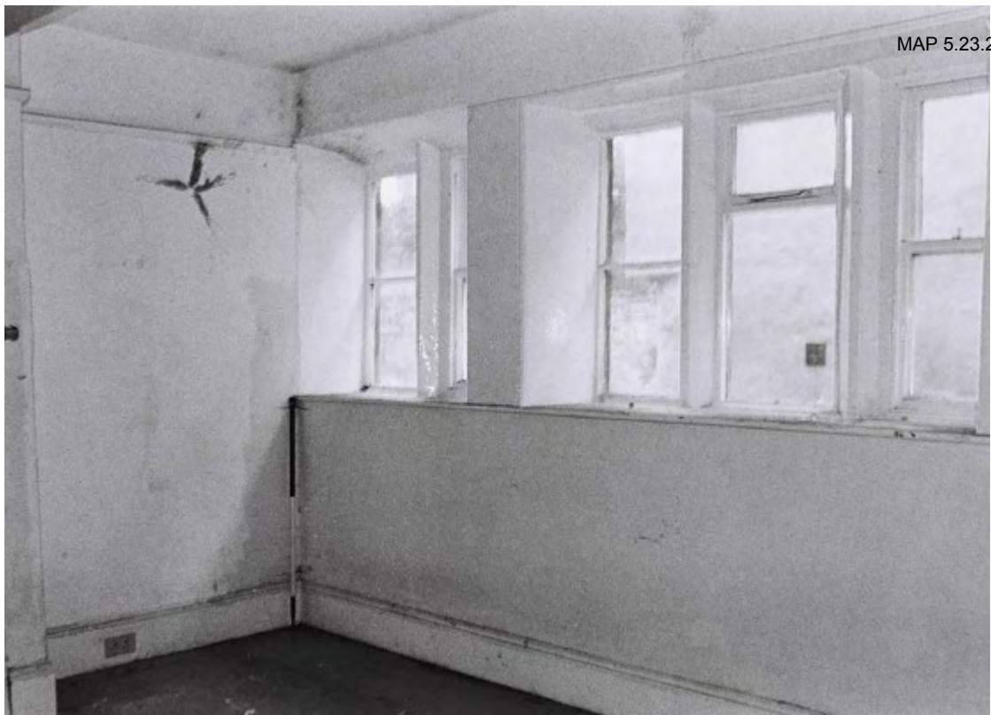
Plate 23. Marsden Park Cottage Interior. Ground Floor. Facing South.
