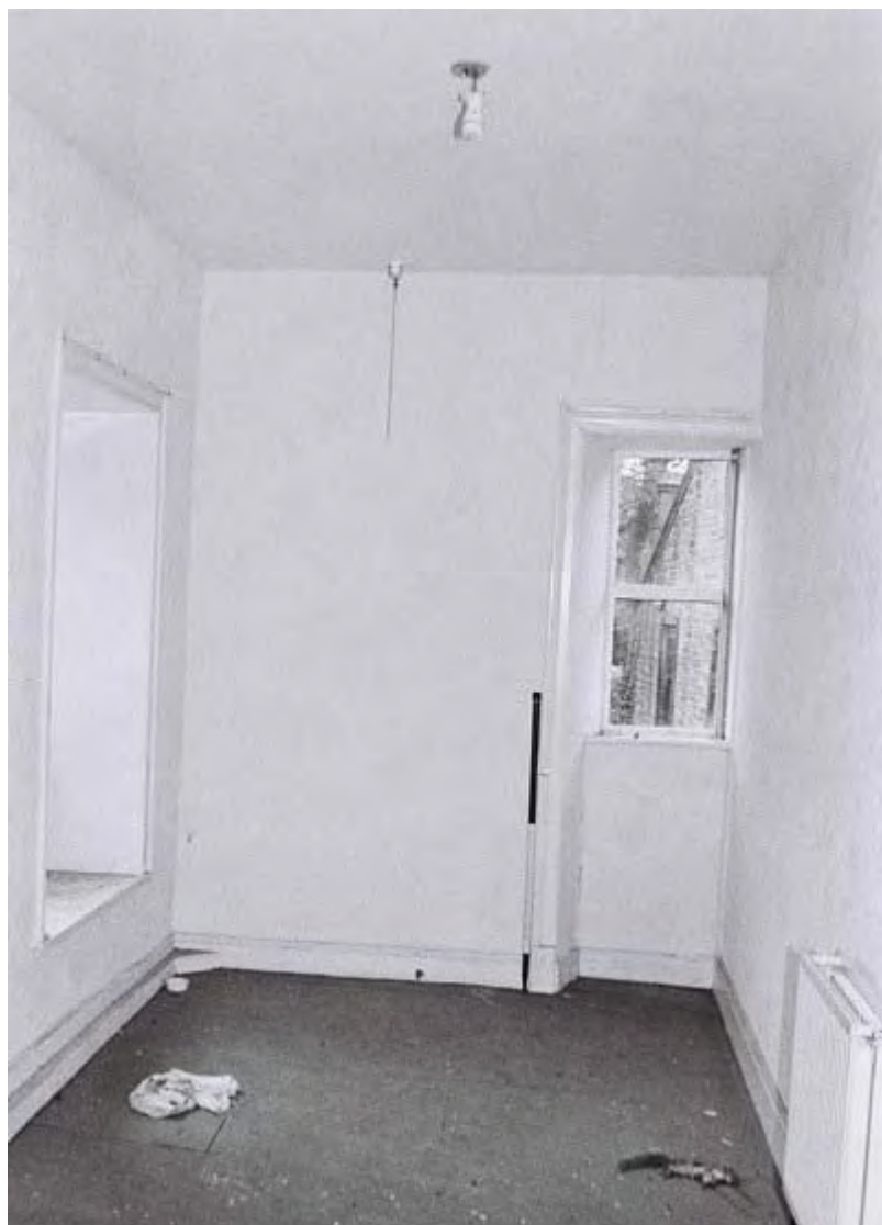
Plate 47. Marsden Park Cottage Interior. First Floor. Facing South
