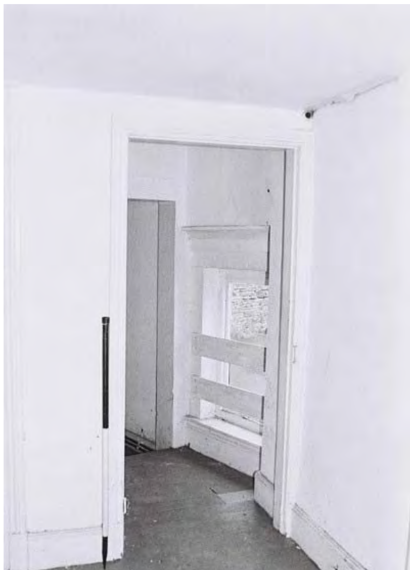
Plate 49. Marsden Park Cottage Interior. First Floor. Facing North.
