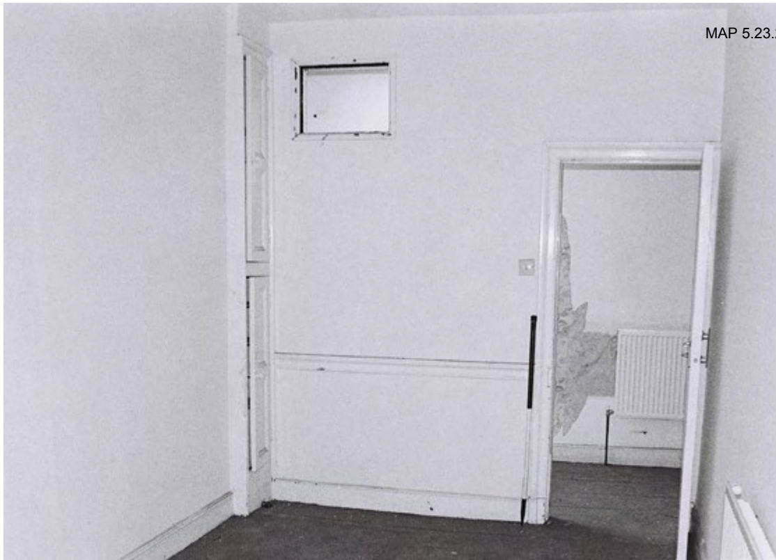
Plate 43. Marsden Park Cottage Interior. First Floor. Facing North.
