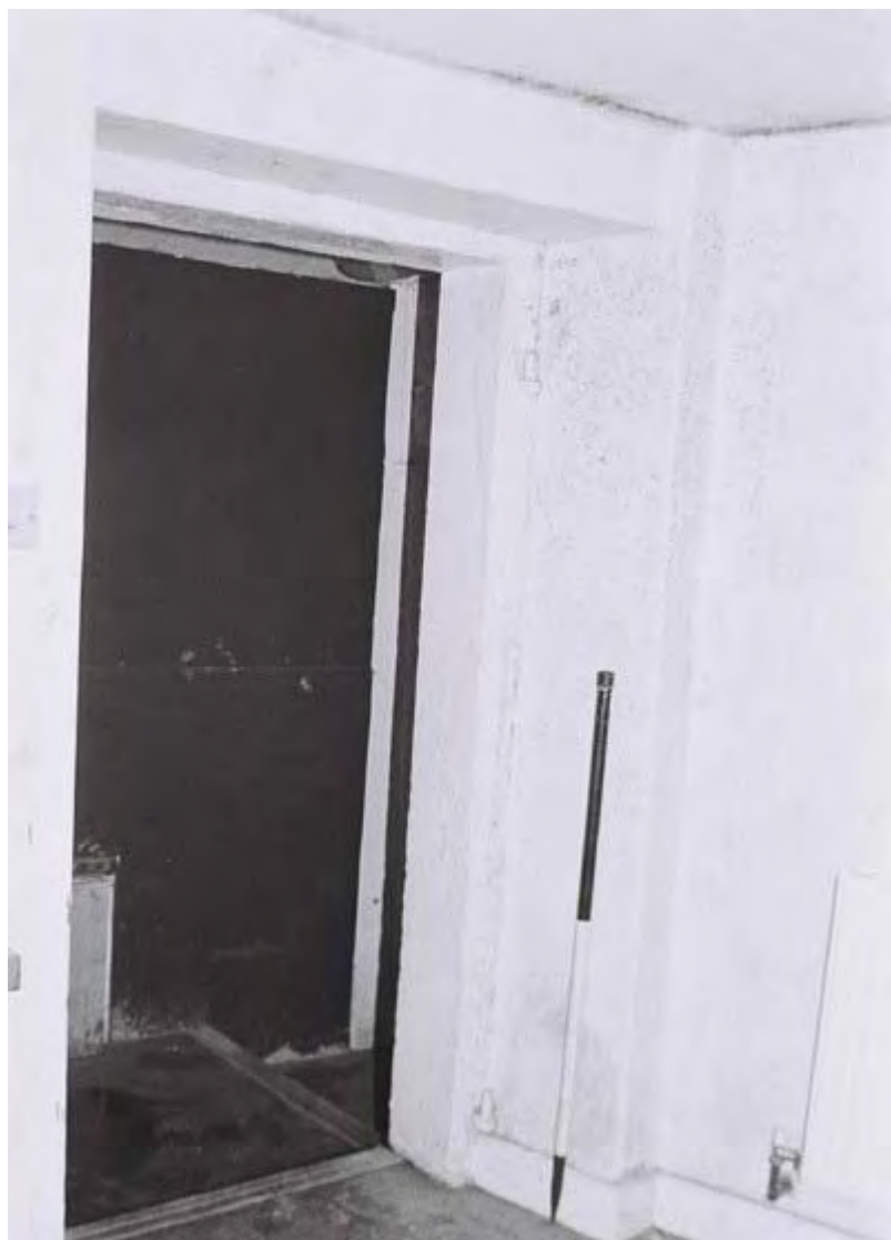
Plate 33. Marsden Park Cottage Interior. Ground Floor. Facing North.
