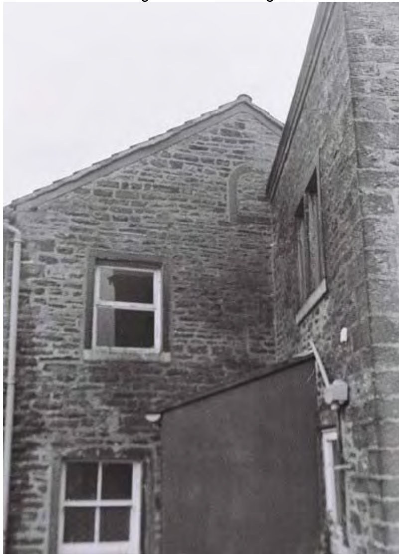
Plate 14. Marsden Park Cottage Exterior : Blocked Attic Window. Facing South.
