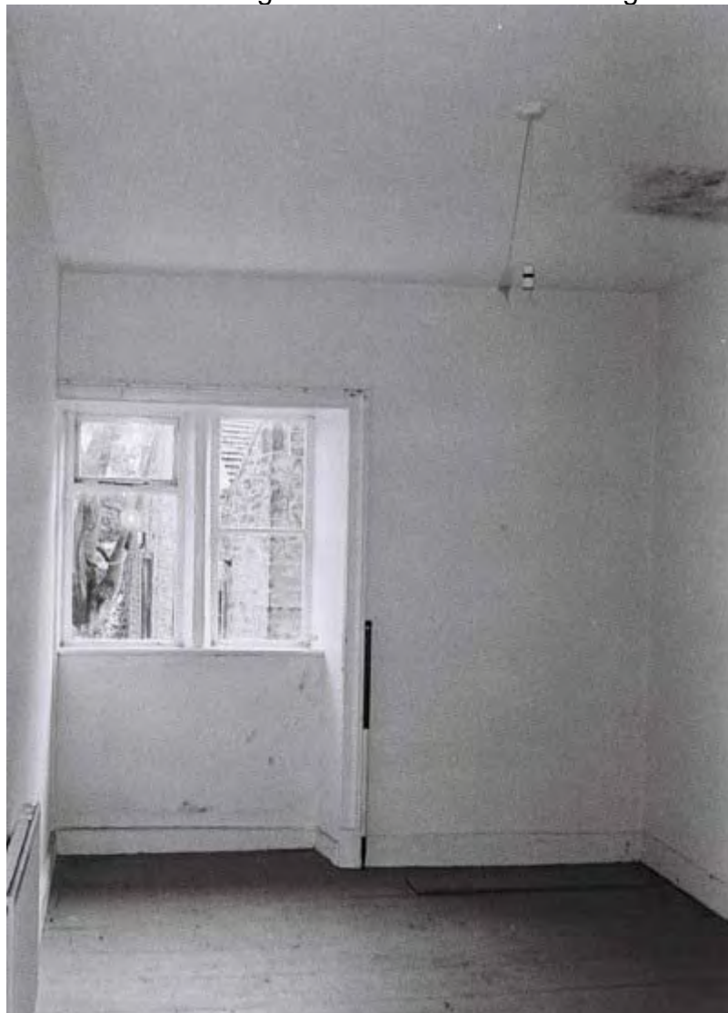
Plate 44. Marsden Park Cottage Interior. First Floor. Facing South.
