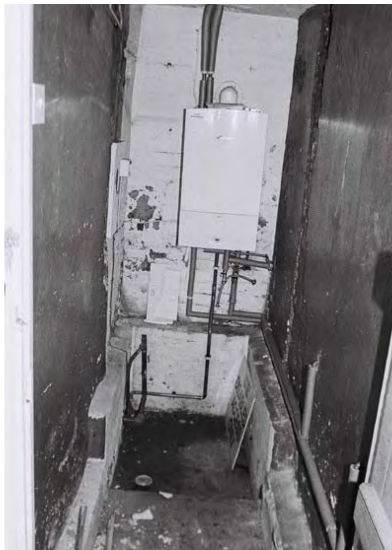
Plate 34. Marsden Park Cottage Interior. Ground Floor. Facing North.
