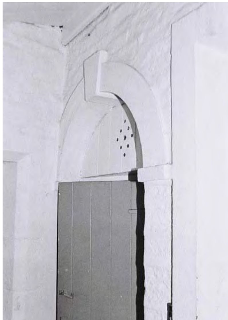
Plate 32. Marsden Park Cottage Interior. Ground Floor. Facing North.
