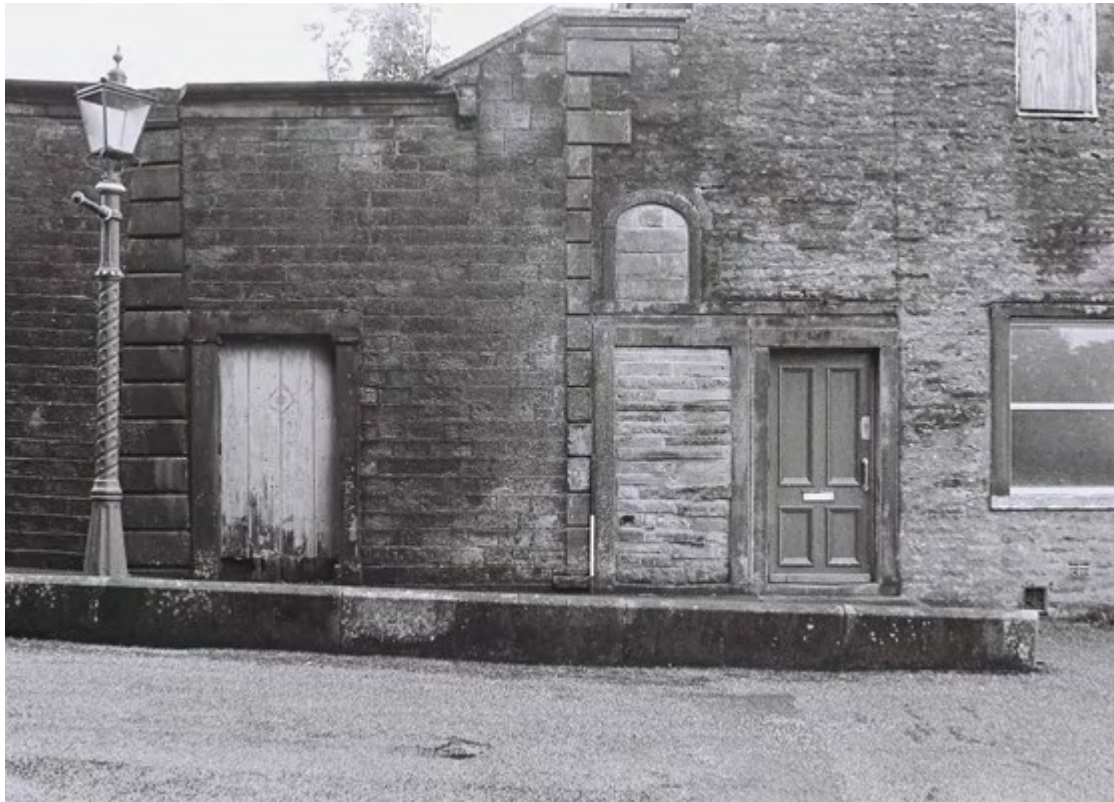
Plate 5. Marsden Park Cottage Exterior. Facing East.
