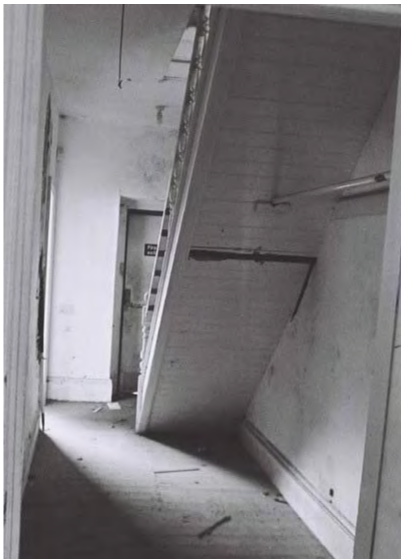
Plate 21. Marsden Park Cottage Interior. Ground Floor. Facing West.
