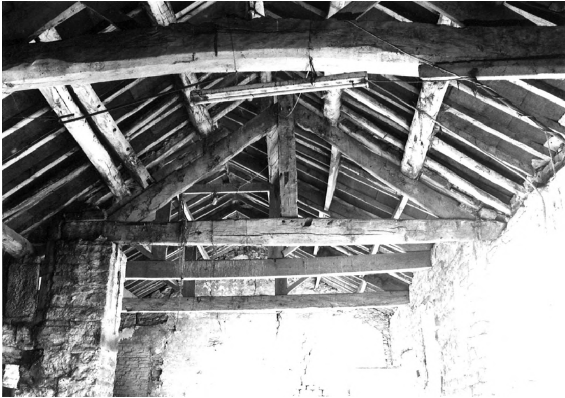
Plate 45. Shaw House Farm: Aisled Barn Interior Roof Truss. Facing East.
