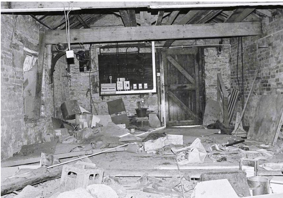
Plate 56. Shaw House Farm: Later Barn Interior First Floor. Facing South.
