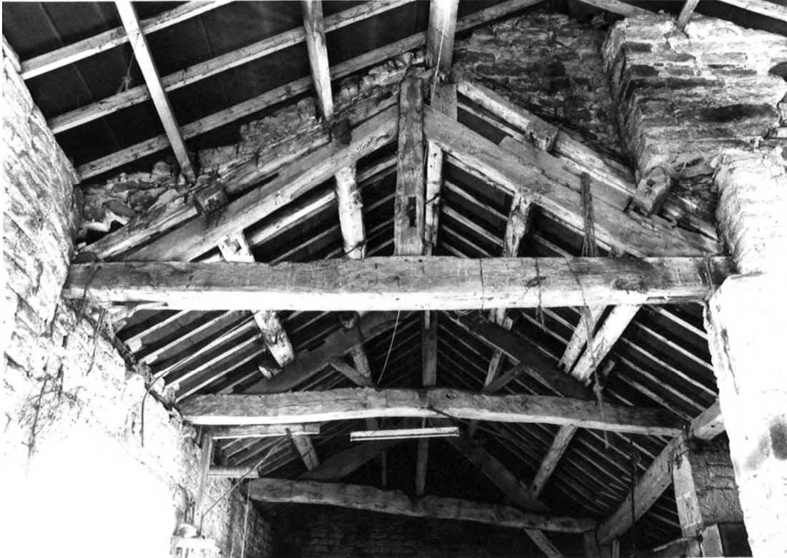
Plate 47. Shaw House Farm: Aisled Barn Interior Roof Truss. Facing West.
