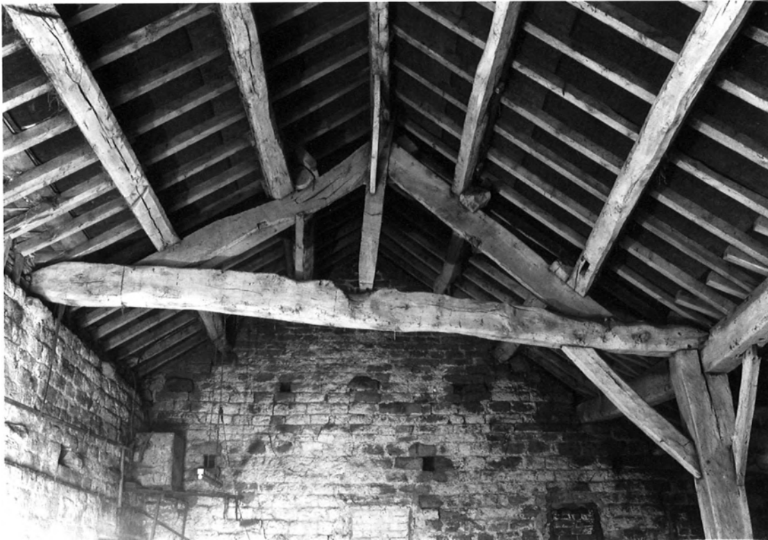
Plate 49. Shaw House Farm: Aisled Barn Interior Roof Truss. Facing West.
