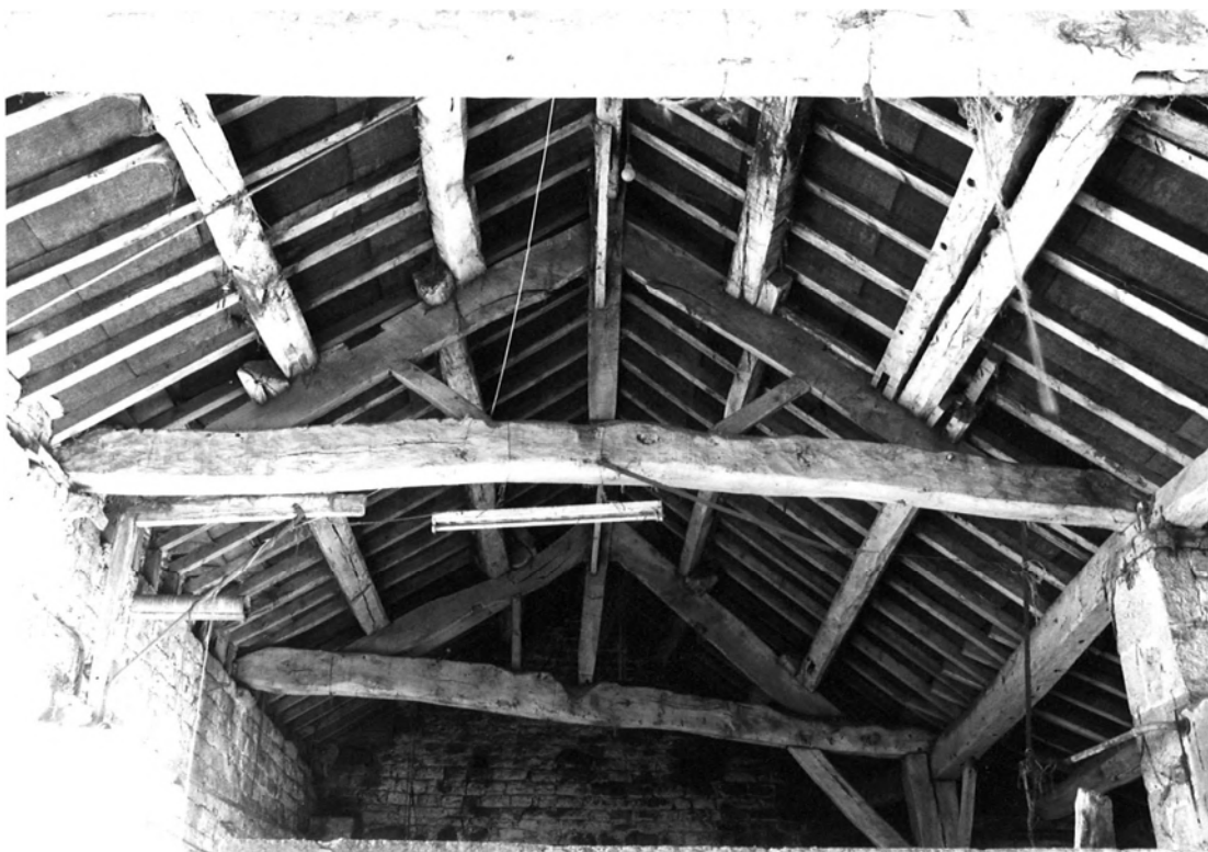
Plate 48. Shaw House Farm: Aisled Barn Interior Roof Truss. Facing West.
