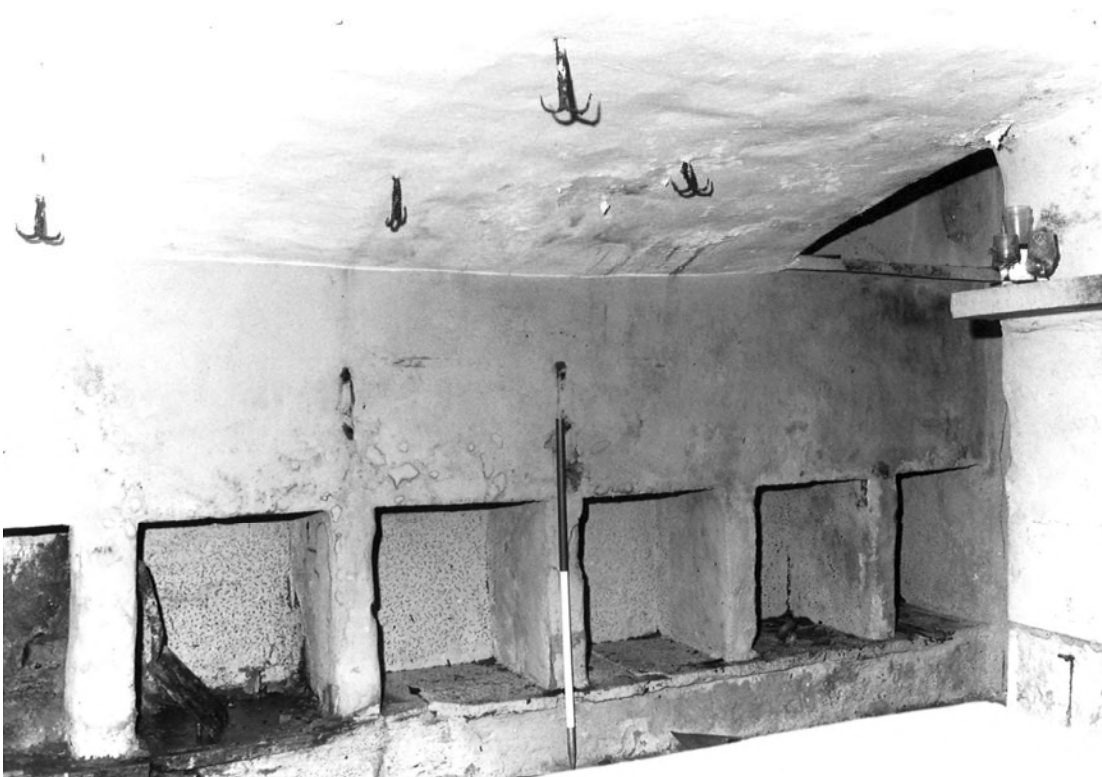
Plate 60. Shaw House Farm: Cottage Interior Cellar. Facing South.
