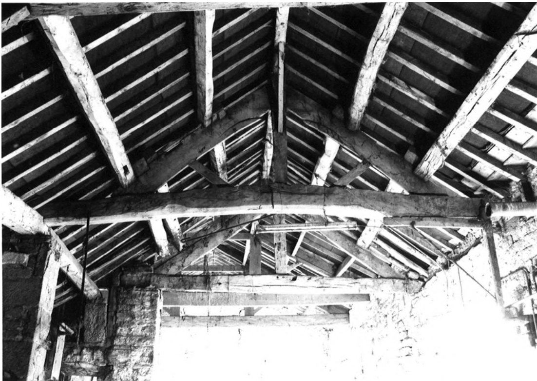
Plate 46. Shaw House Farm: Aisled Barn Interior Roof Truss. Facing East.
