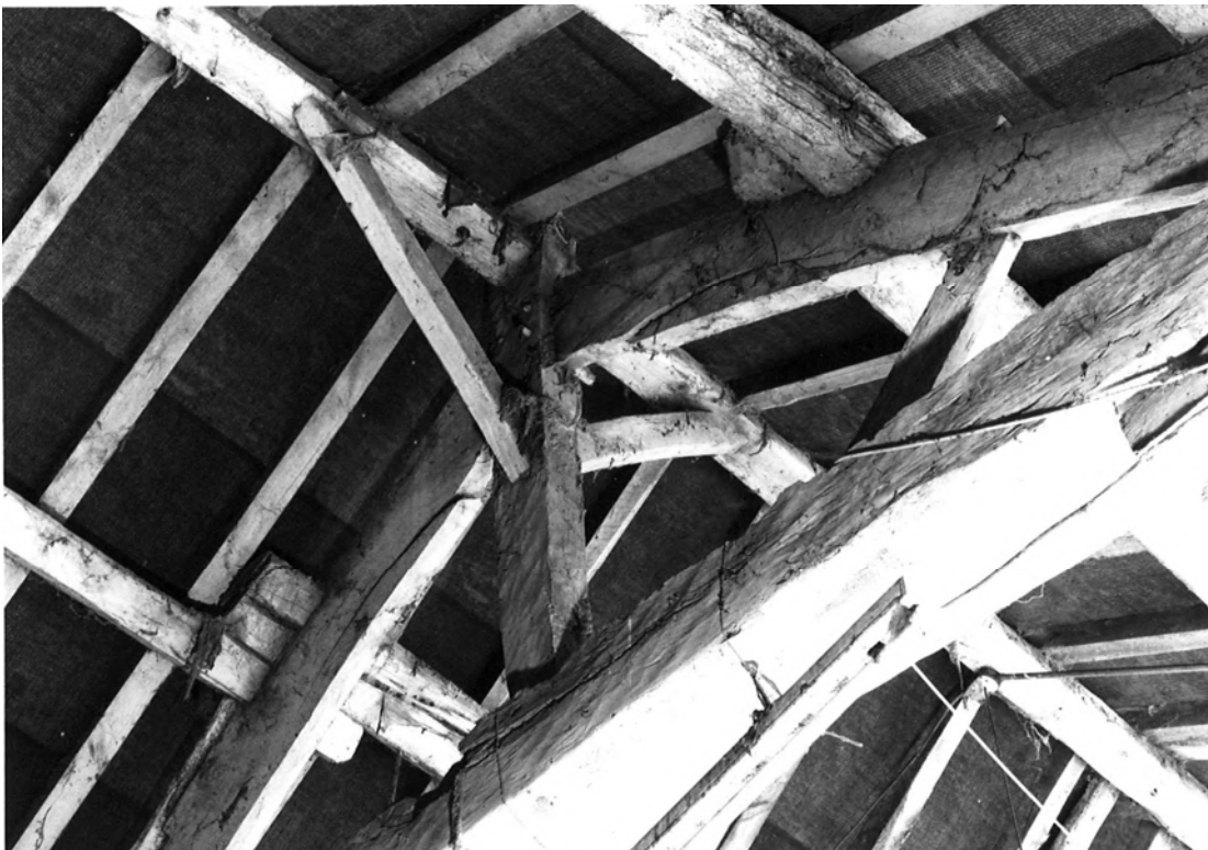
Plate 50. Shaw House Farm: Aisled Barn Interior Roof Truss. Facing North-west.
