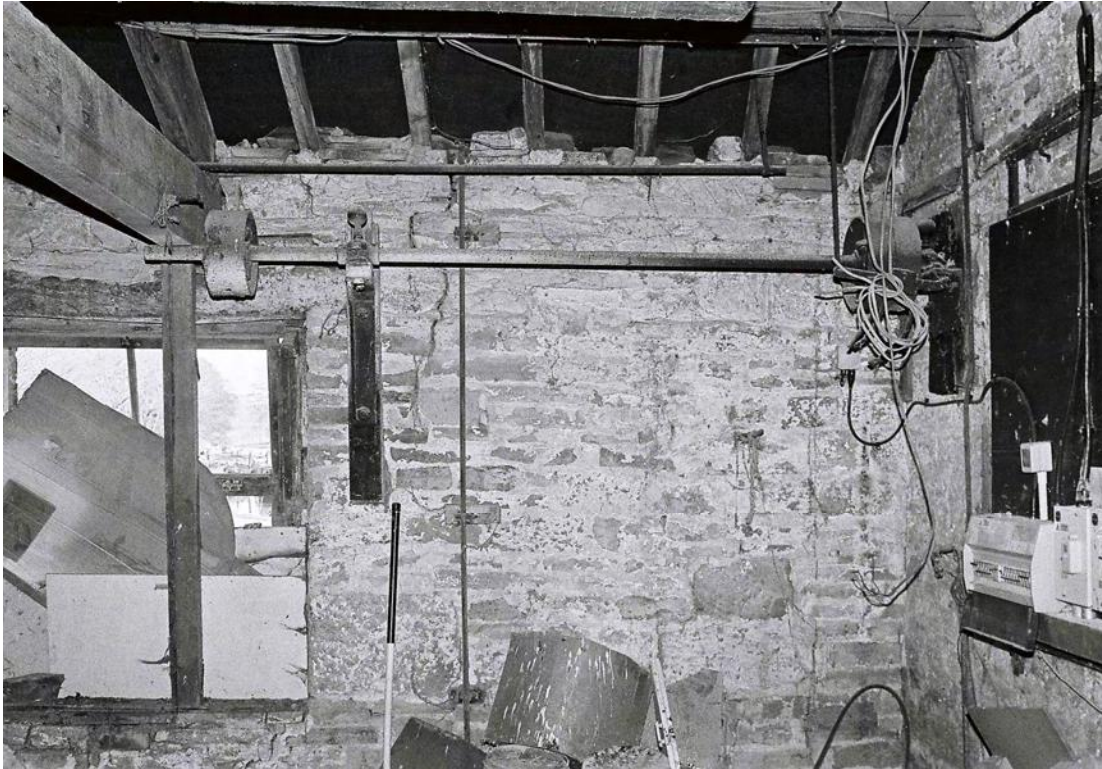
Plate 59. Shaw House Farm: Later Barn Interior First Floor. Facing East.
