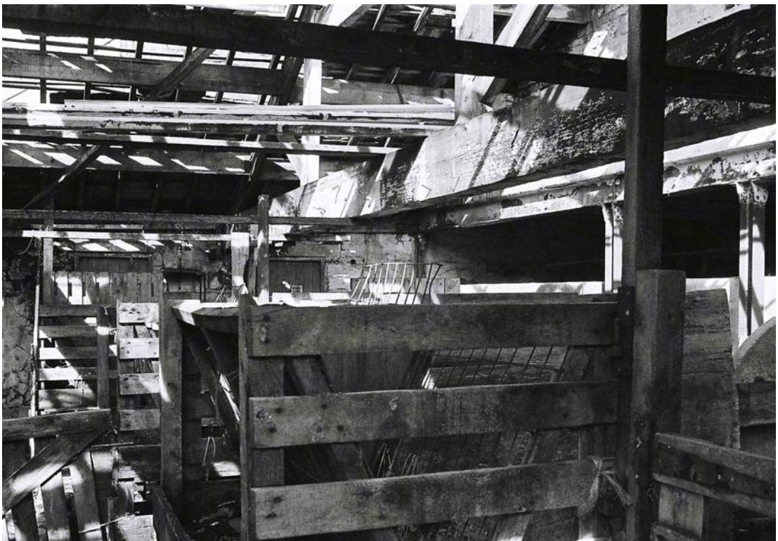
Plate 52. Shaw House Farm: Later Barn Interior Ground Floor. Facing North.
