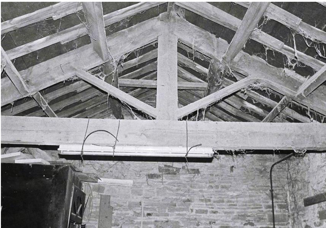
Plate 58. Shaw House Farm: Later Barn Interior First Floor. Facing South.
