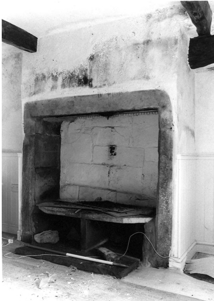
Plate 62. Shaw House Farm: Cottage Interior Ground Floor. Facing East.
