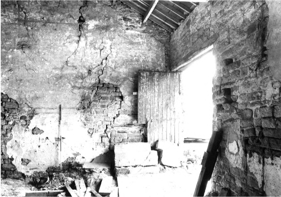
Plate 29. Shaw House Farm: Aisled Barn Interior. Facing East.
