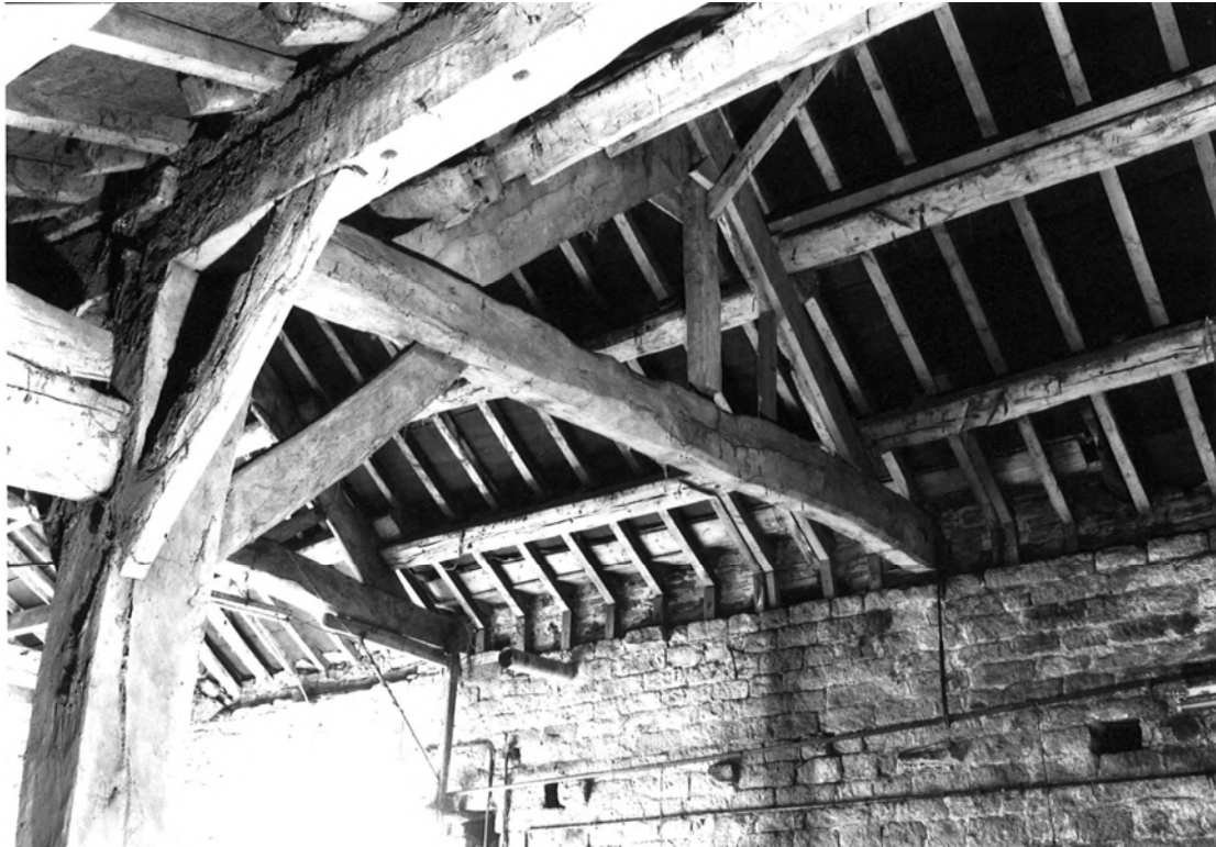
Plate 41. Shaw House Farm: Aisled Barn Interior Roof Truss. Facing South-east.
