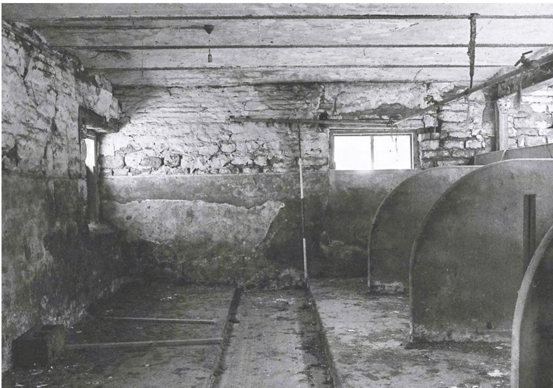
Plate 54. Shaw House Farm: Later Barn Interior Ground Floor. Facing North.
