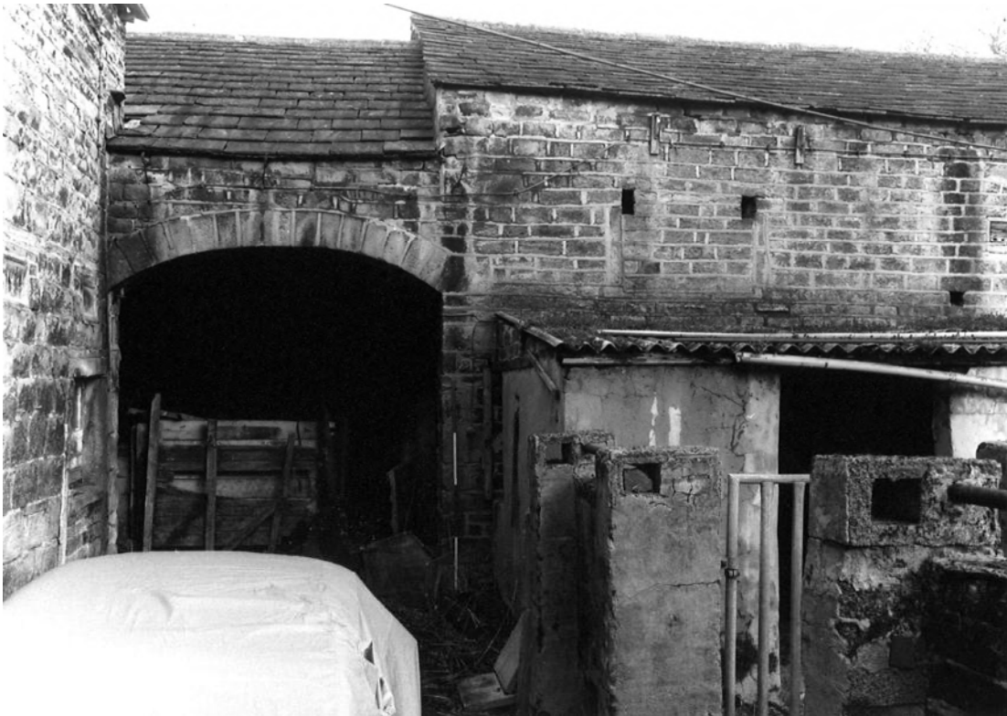
Plate 9. Shaw House Farm: Barn Exterior. Facing North.
