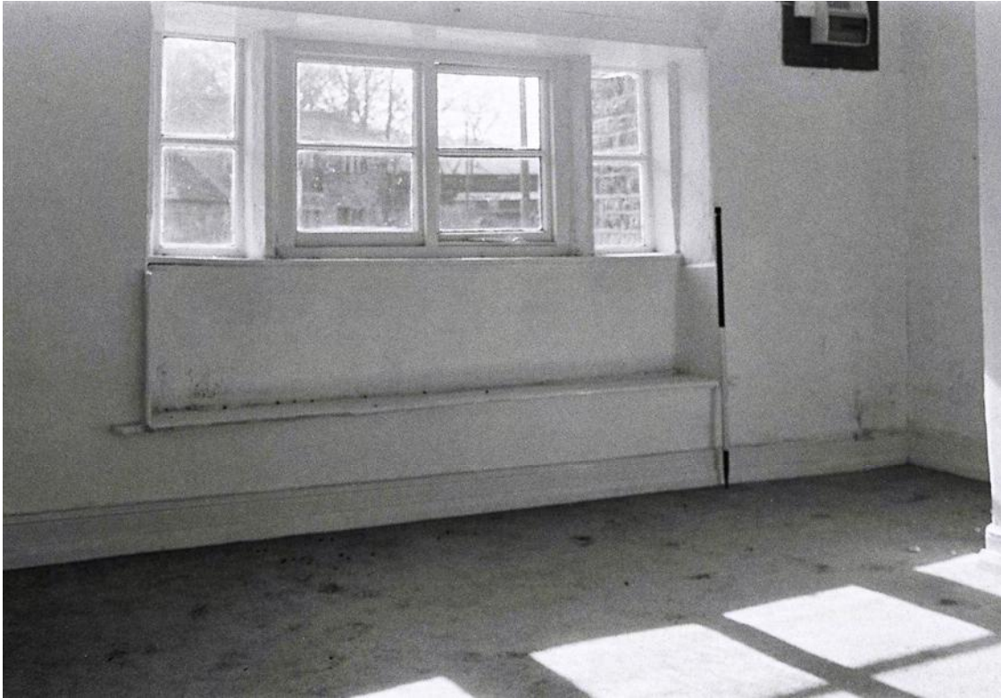
Plate 65. Shaw House Farm: Cottage Interior First Floor. Facing South.
