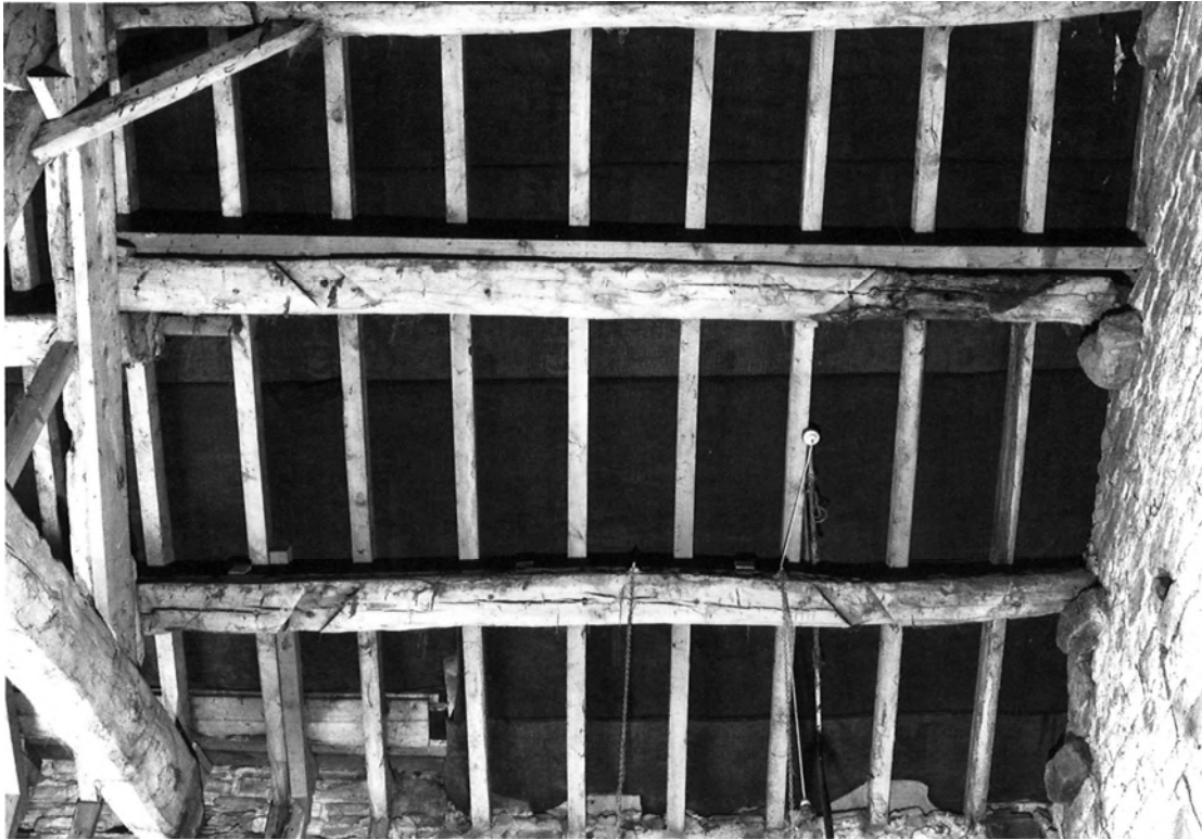
Plate 51. Shaw House Farm: Aisled Barn Interior Reused Cruck. Facing South.
