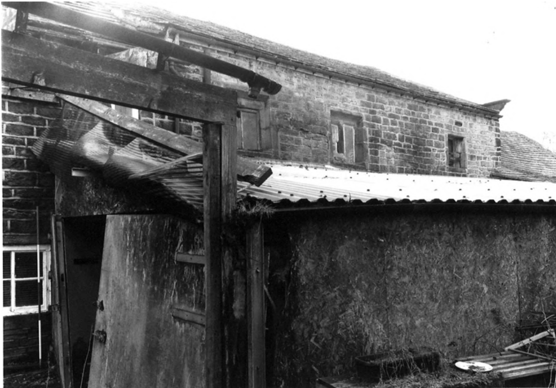
Plate 13. Shaw House Farm: Barn Exterior. Facing South-west.
