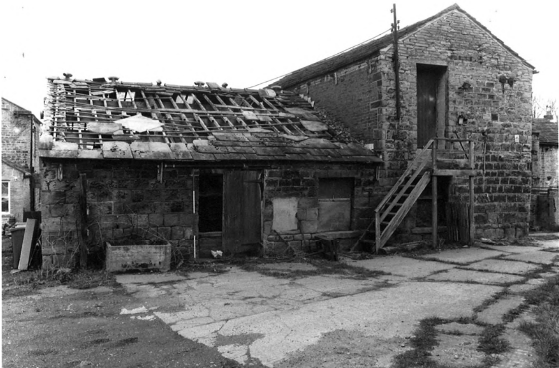
Plate 6. Shaw House Farm: Barn Exterior. Facing North.
