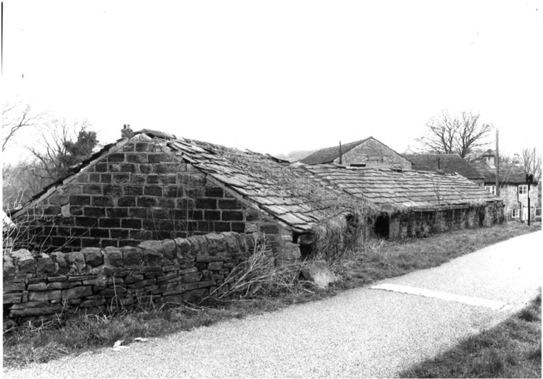
Plate 24. Shaw House Farm: Stables Exterior. Facing East.
