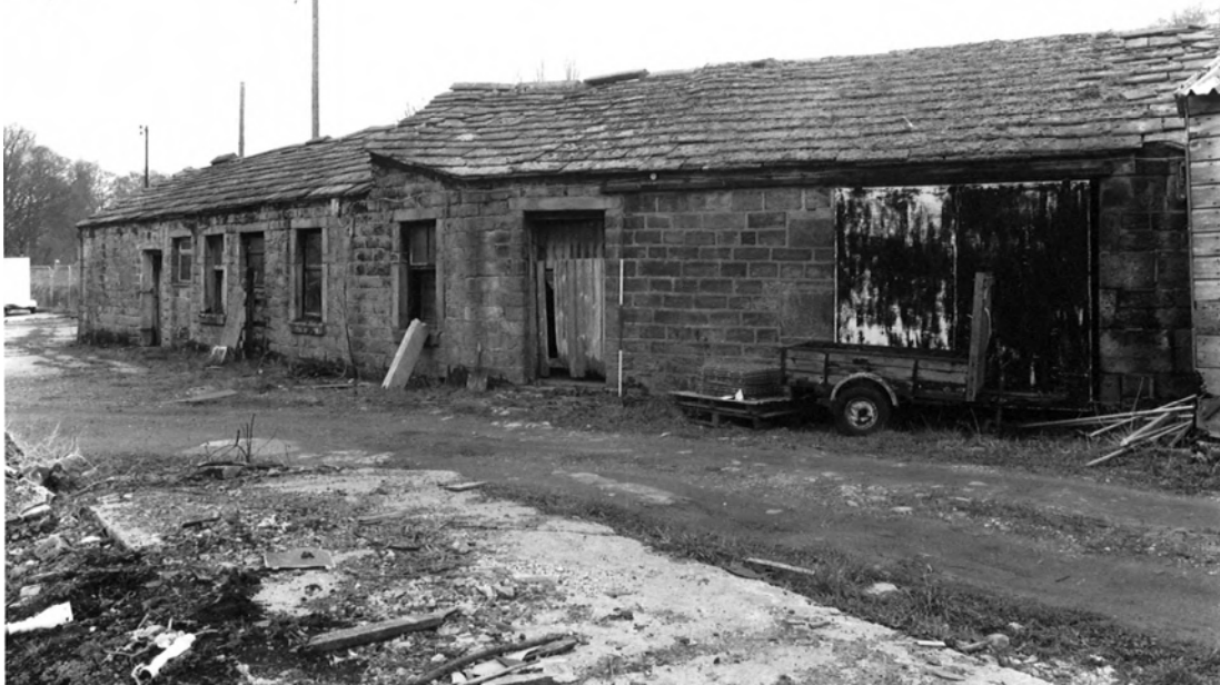
Plate 21. Shaw House Farm: Stables Exterior. Facing South.
