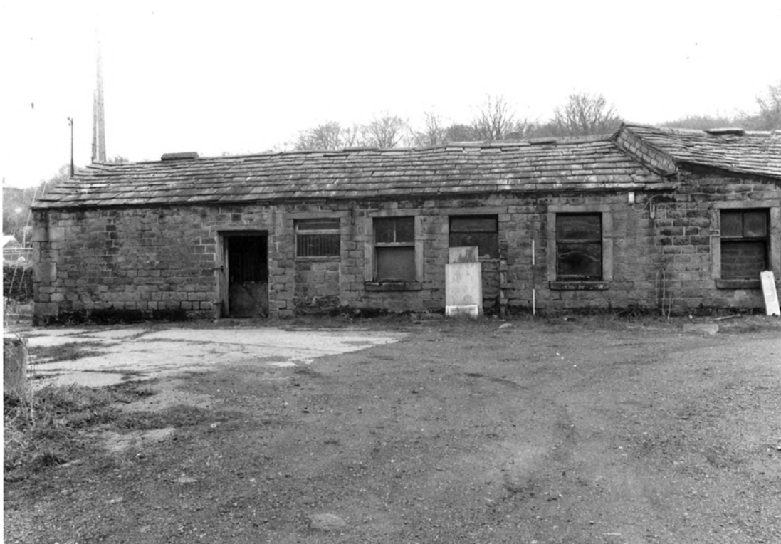
Plate 22. Shaw House Farm: Stables Exterior. Facing South-east.
