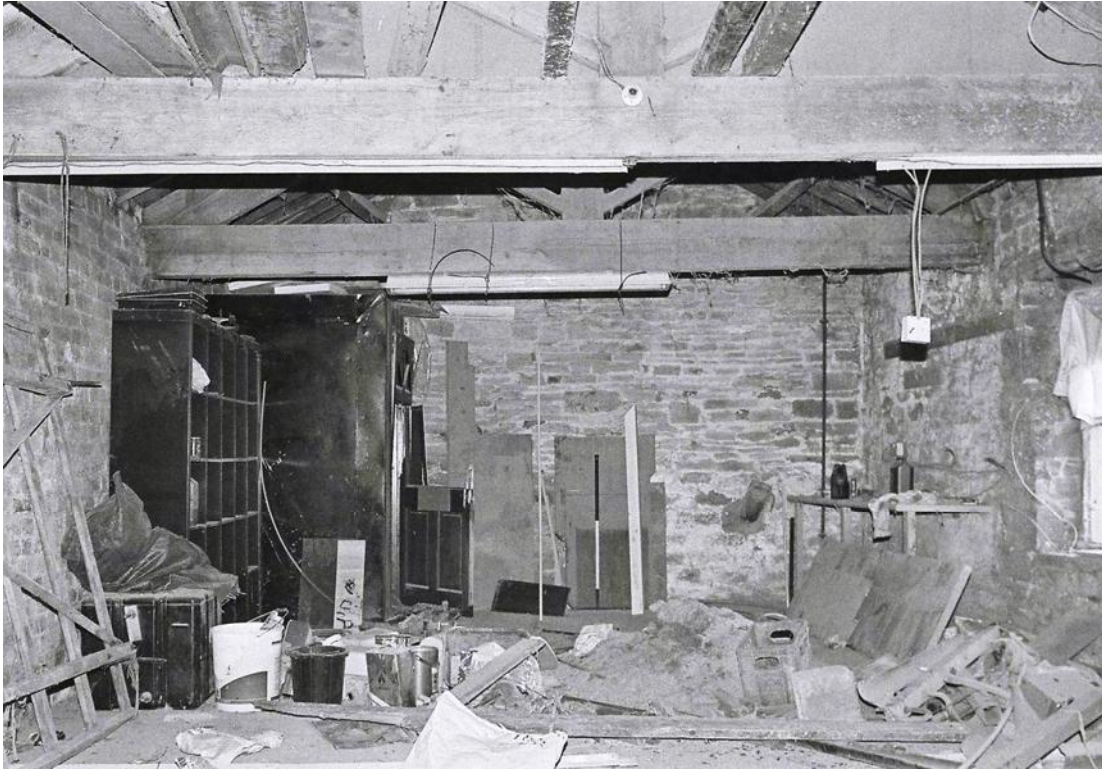
Plate 57. Shaw House Farm: Later Barn Interior First Floor. Facing North.
