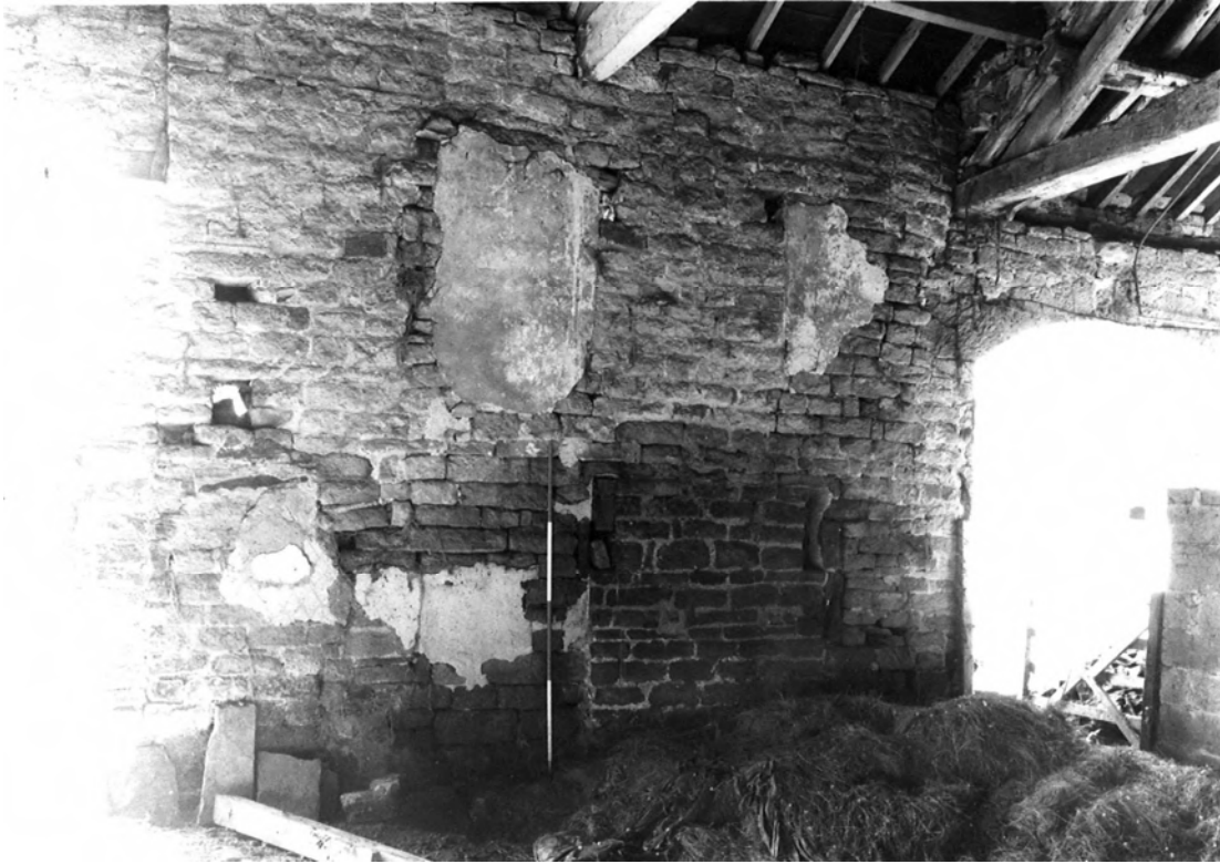
Plate 35. Shaw House Farm: Aisled Barn Interior. Facing South-west.
