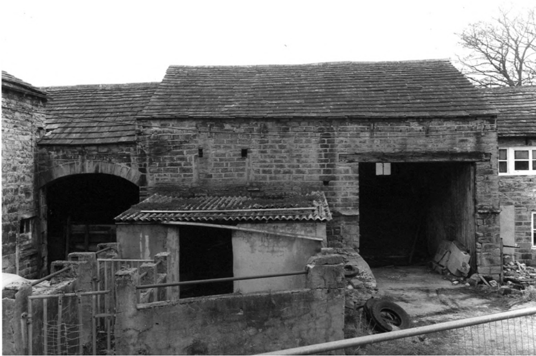
Plate 3. Shaw House Farm: Barn Exterior. Facing North.
