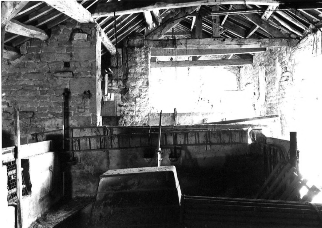
Plate 25. Shaw House Farm: Aisled Barn Interior. Facing East.
