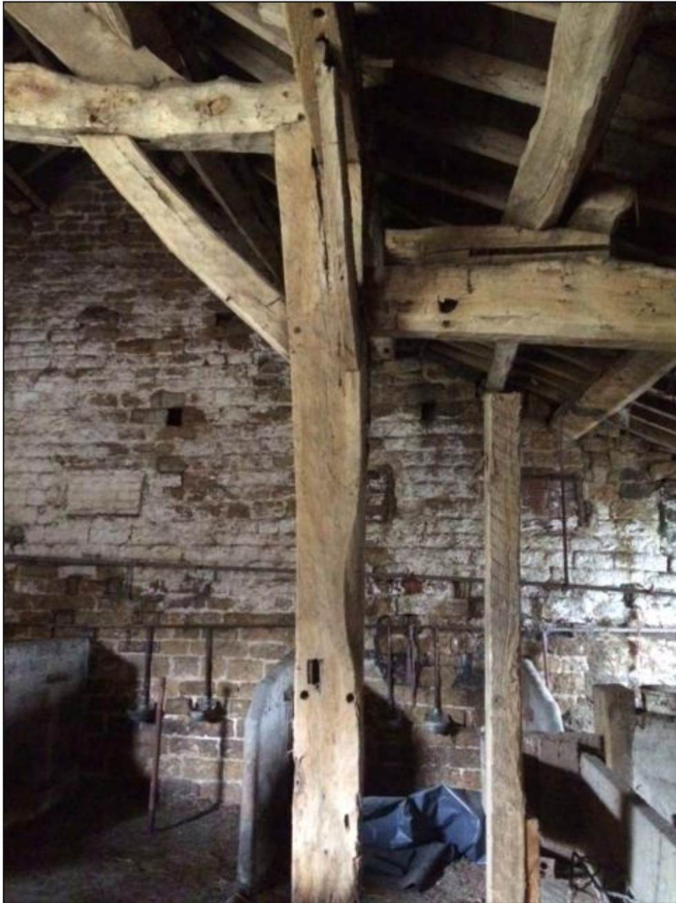
Figure 5: North aisle post of truss 1, photograph taken from the east
