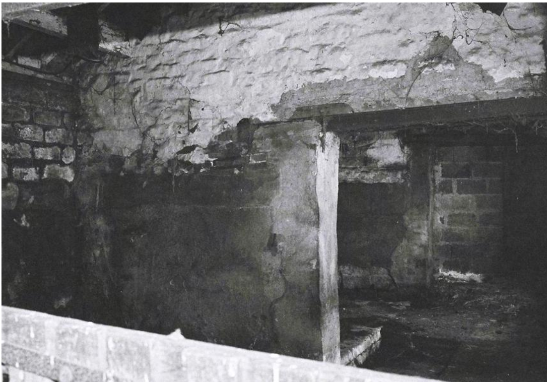
Plate 66. Shaw House Farm: Stables Interior. Facing South-west.
