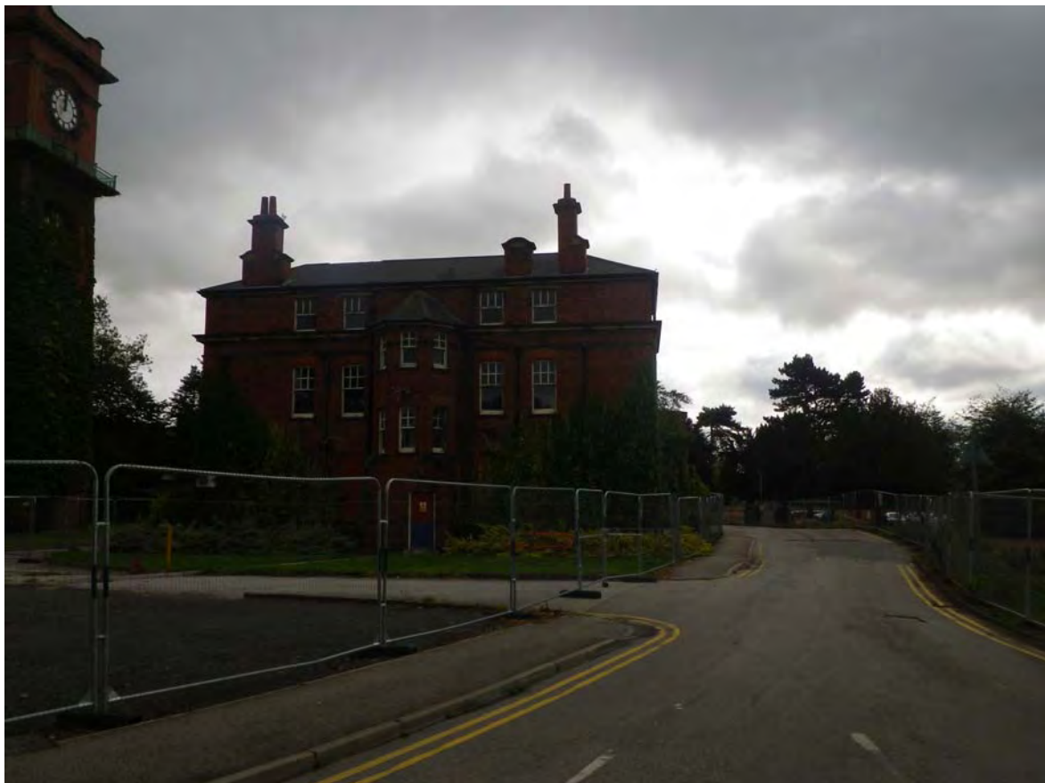
Plate 8. Administration Building. Facing East.
