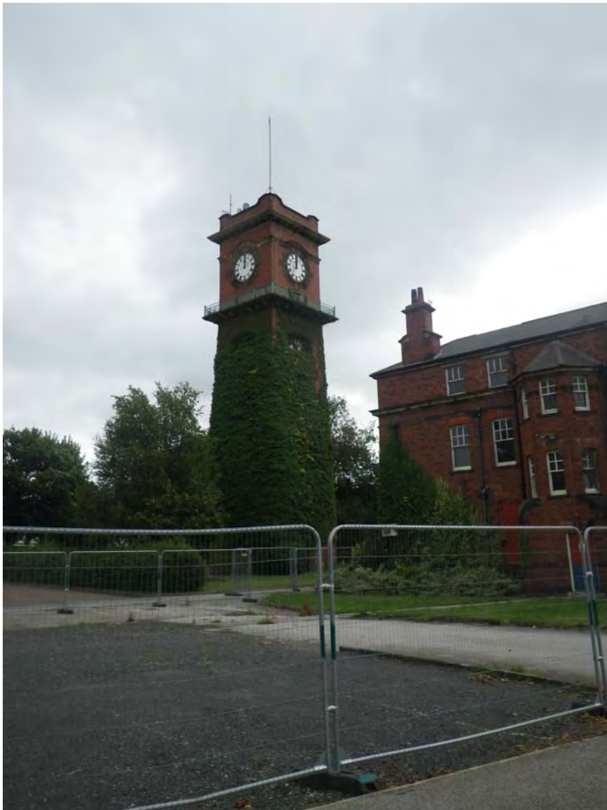
Plate 1. Clock Tower. Facing North-east.
