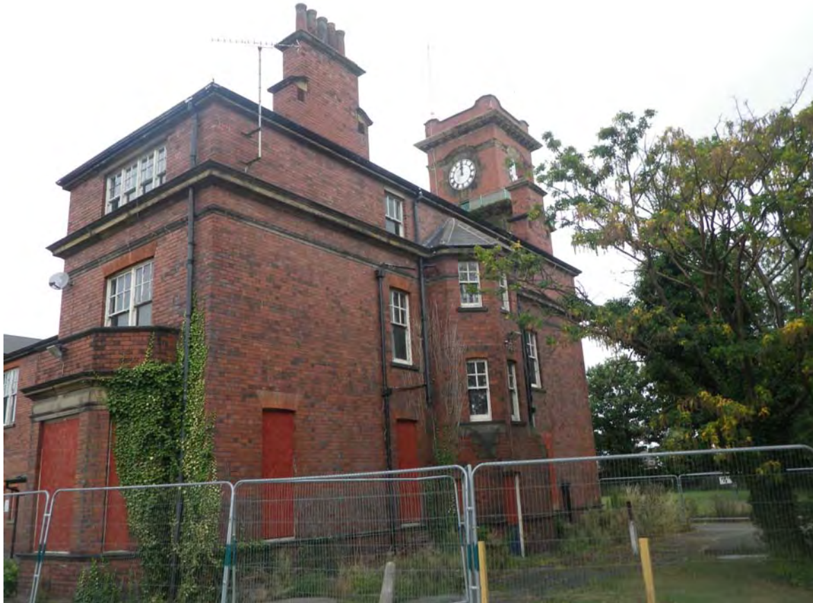
Plate 9. Administration Building. Facing South-west.
