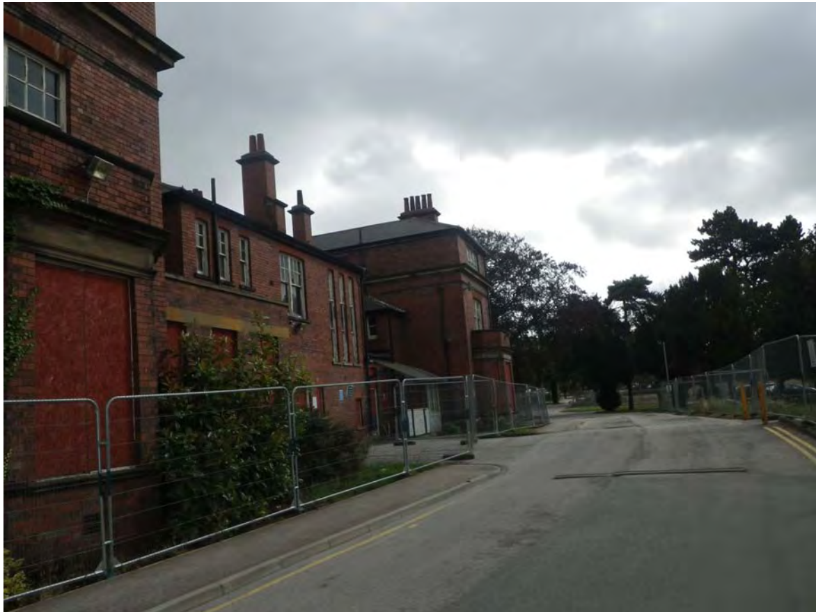
Plate 7. Administration Building. Facing East.
