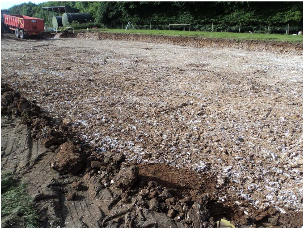
Plate 4. General View of Stripped Area. Facing South.
