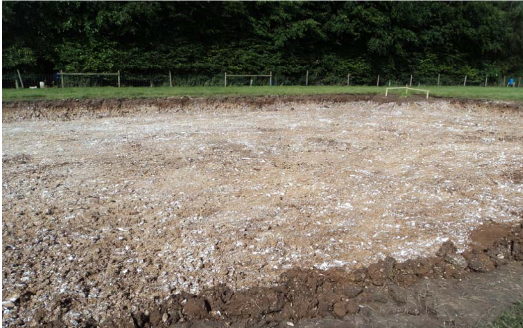
Plate 3. General View of Stripped Area. Facing North-west.
