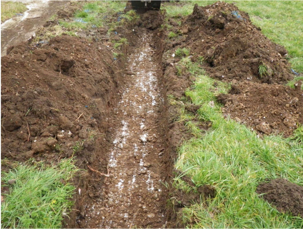
Plate 1. Foundation Trench. Facing North-east.
