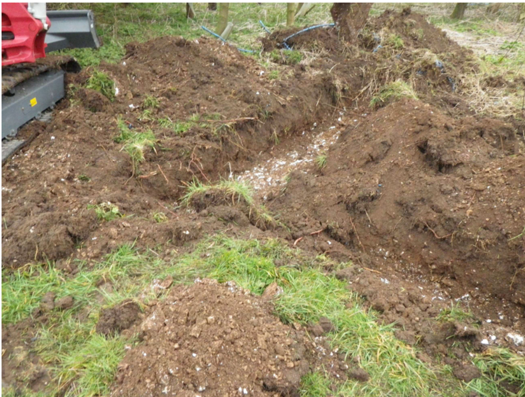
Plate 2. Foundation Trench. Facing North.
