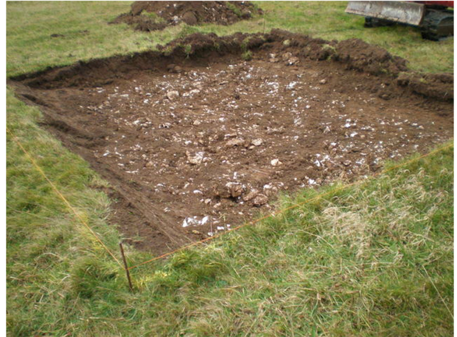
Plate 2. Wind Turbine Base after Topsoil Strip. Facing South-east.
