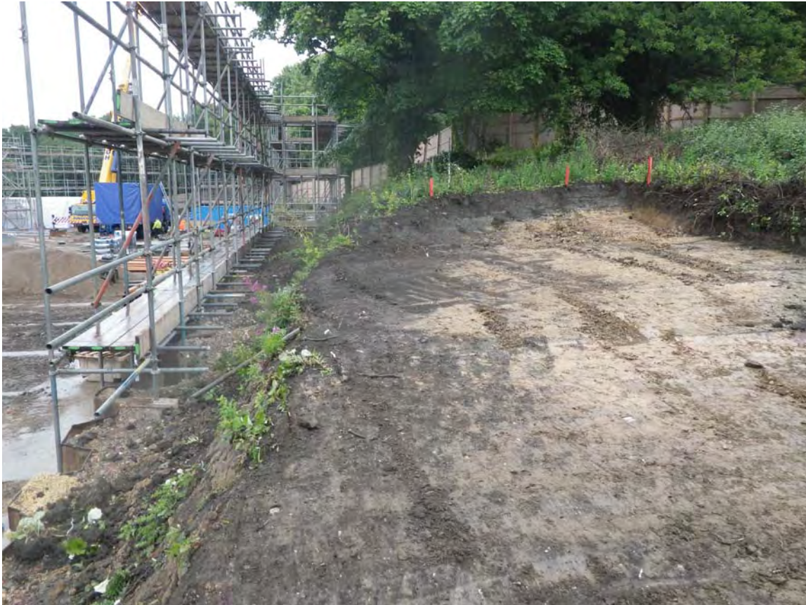
Plate 5. Area of Path after Topsoil Strip. Facing East.
