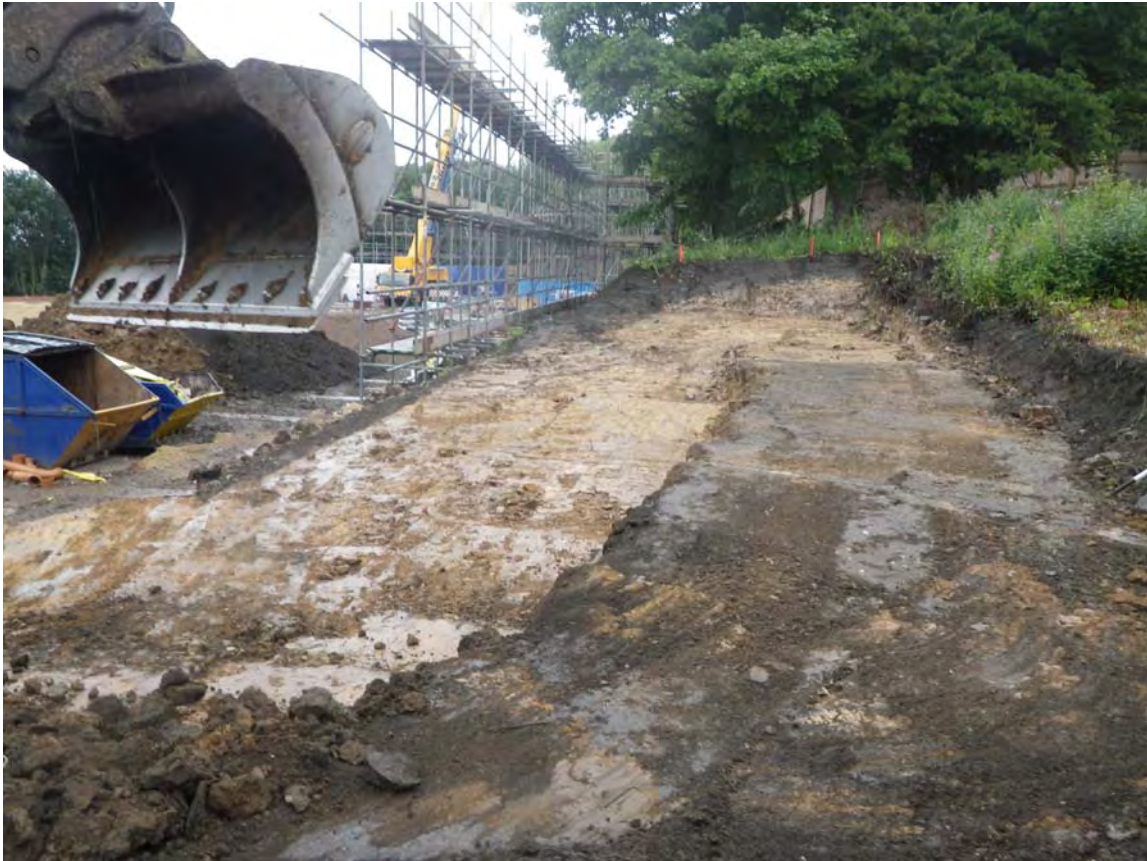
Plate 7. Area of Path after reduced level dig. Facing East.
