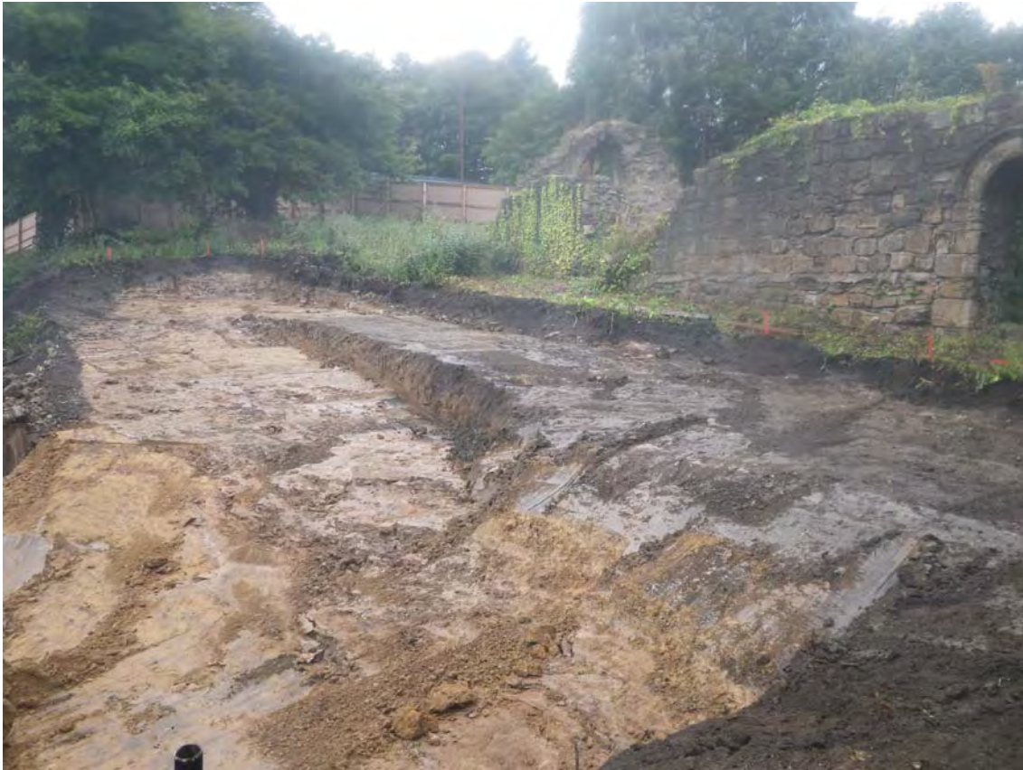
Plate 9. Area of Path and Stairs after reduced level dig. Facing East.
