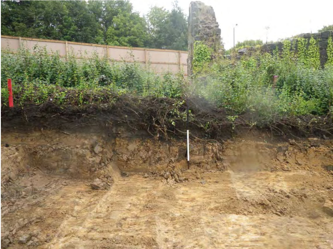
Plate 6. Area of Path after reduced level dig. Facing South.
