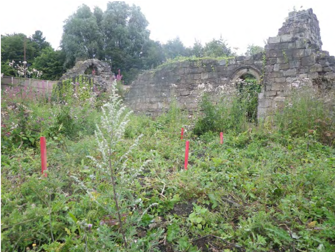
Plate 1. View of Area of Stairs. Facing South.
