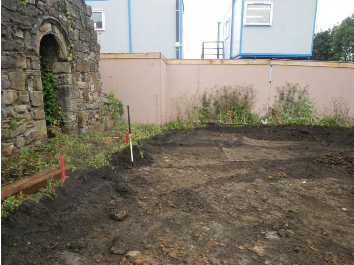
Plate 8. Area of Stairs after topsoil strip. Facing West.
