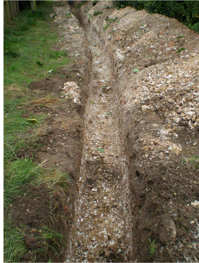
Plate 4. Cable Trench. Facing West.
