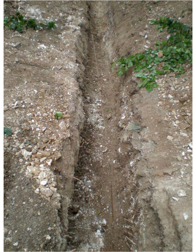
Plate 6. Modern Service in Cable Trench. Facing North-west.
