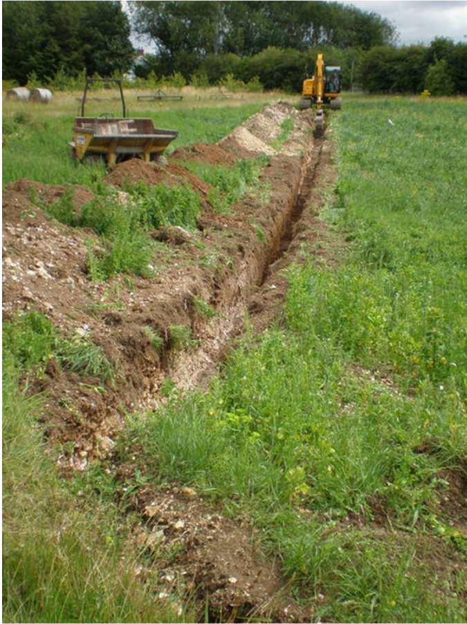
Plate 3. Cable Trench Showing Changes in Natural. Facing South-east.
