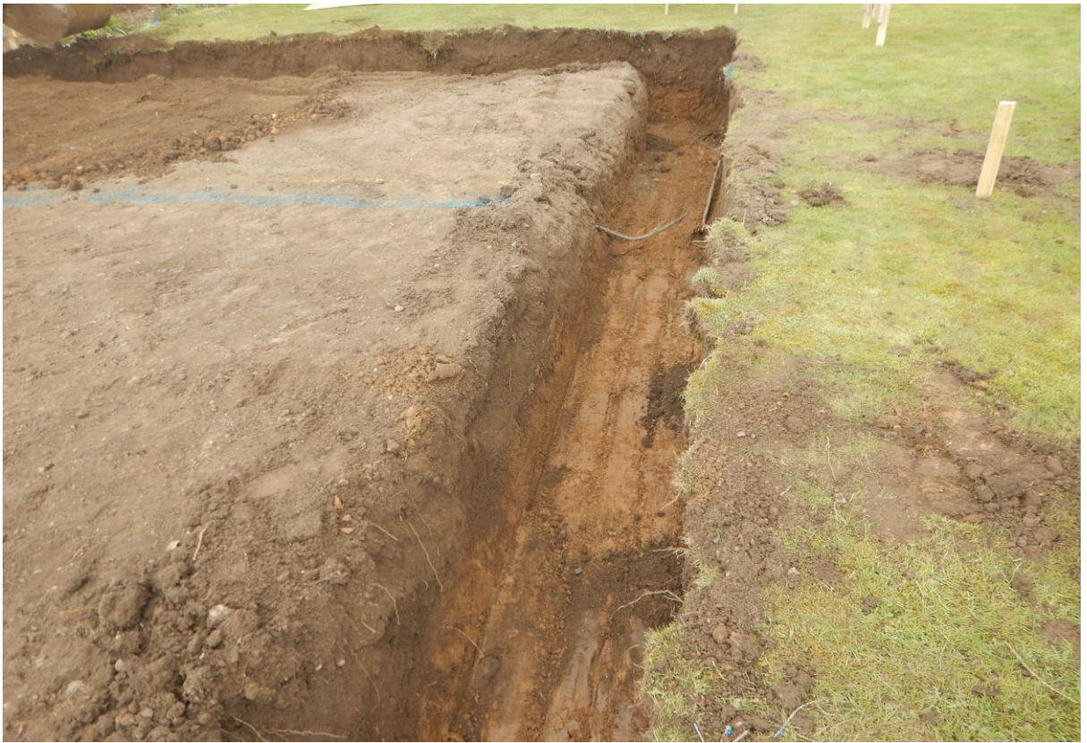
Plate 5. Foundations of Northern Most Plot.
