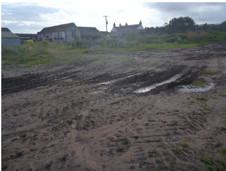
Plate 2: General View of Development Area. Facing Southeast.
