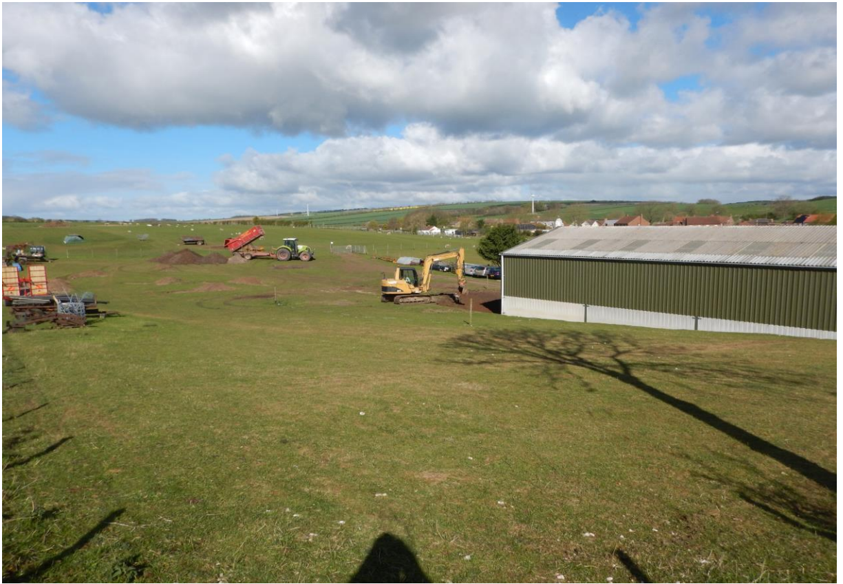
Plate 5. General View of Site, Facing North West.
