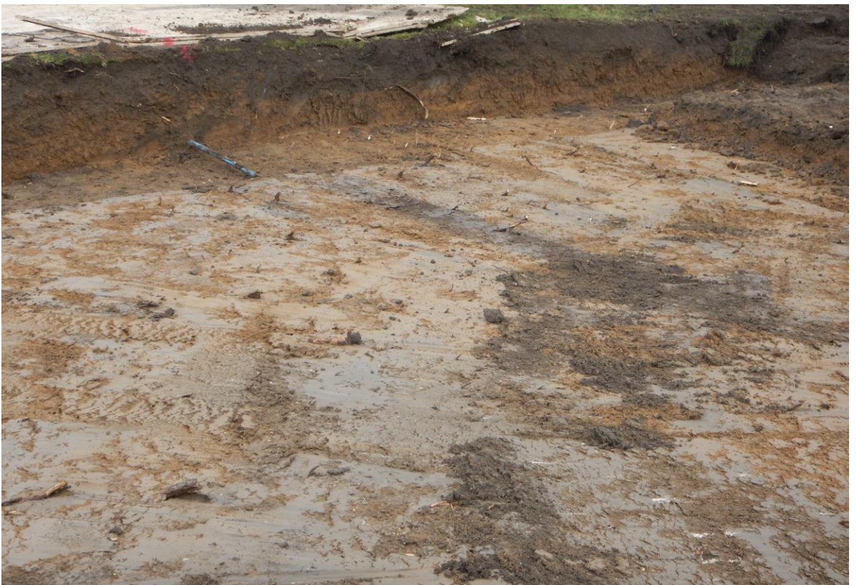
Plate 4. Stripped Area Showing Services.
