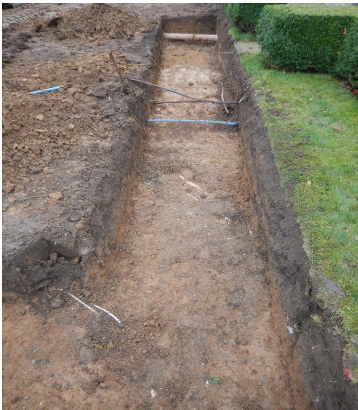
Plate 2. Foundation Trench Looking East Showing Services.
