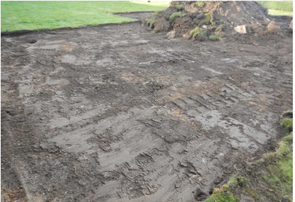
Plate 1. Work During Topsoil Stripping.
