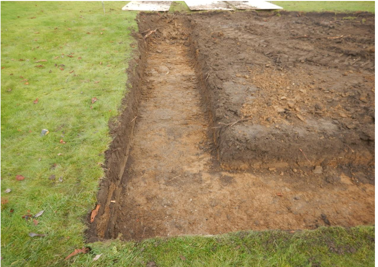
Plate 3. Foundation Trench Looking North.
