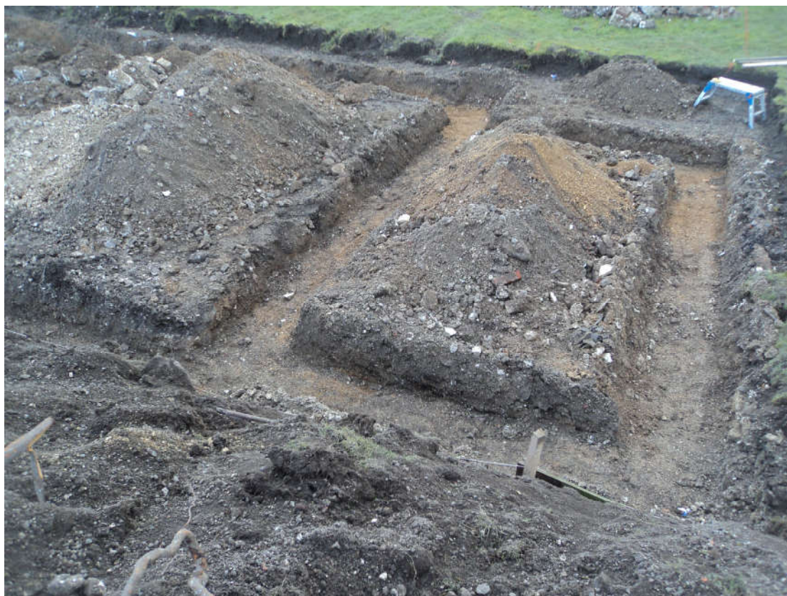
Plate 6. General View of Footings. Facing South-west.
