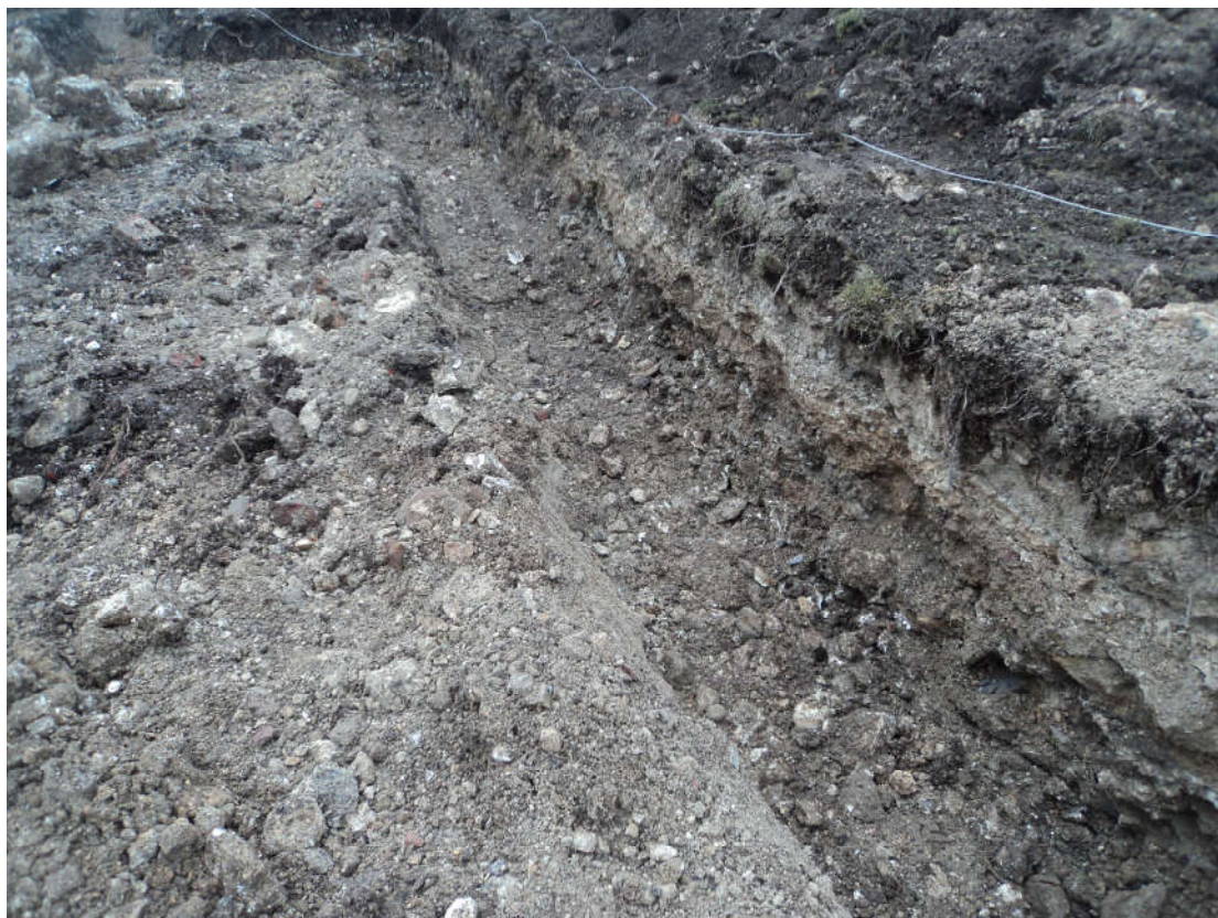
Plate 5. Eastern Foundation Trench. Facing North-west.
