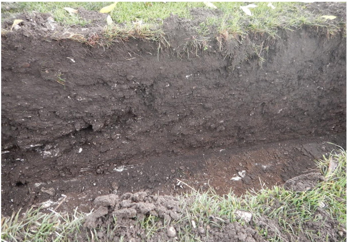
Plate 2. Section of Footings Facing East.
