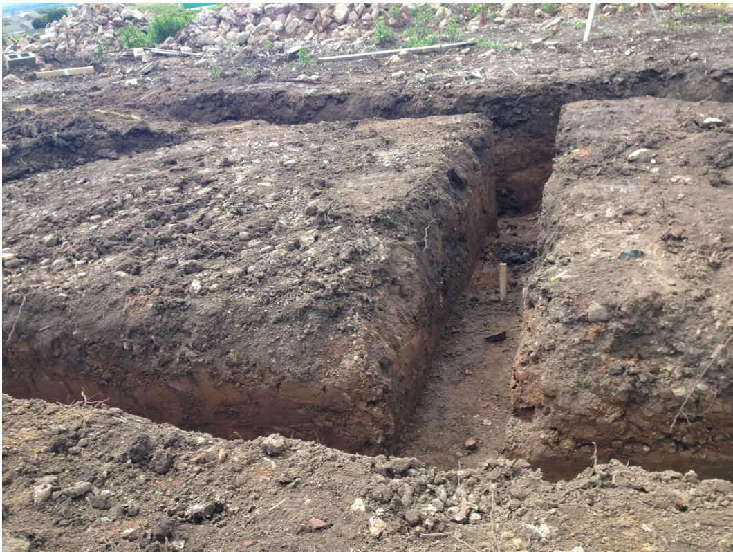
Plate 3. View of Foundation Trenches. Facing West.
