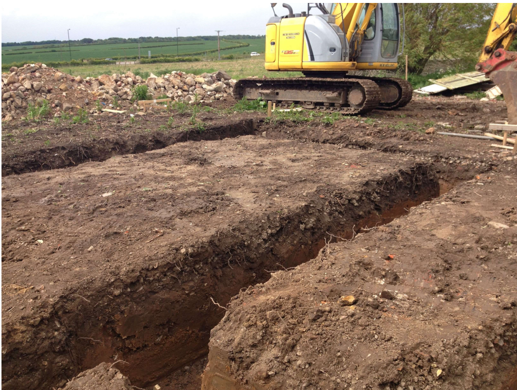
Plate 2. View of Foundation Trenches. Facing North-West.
