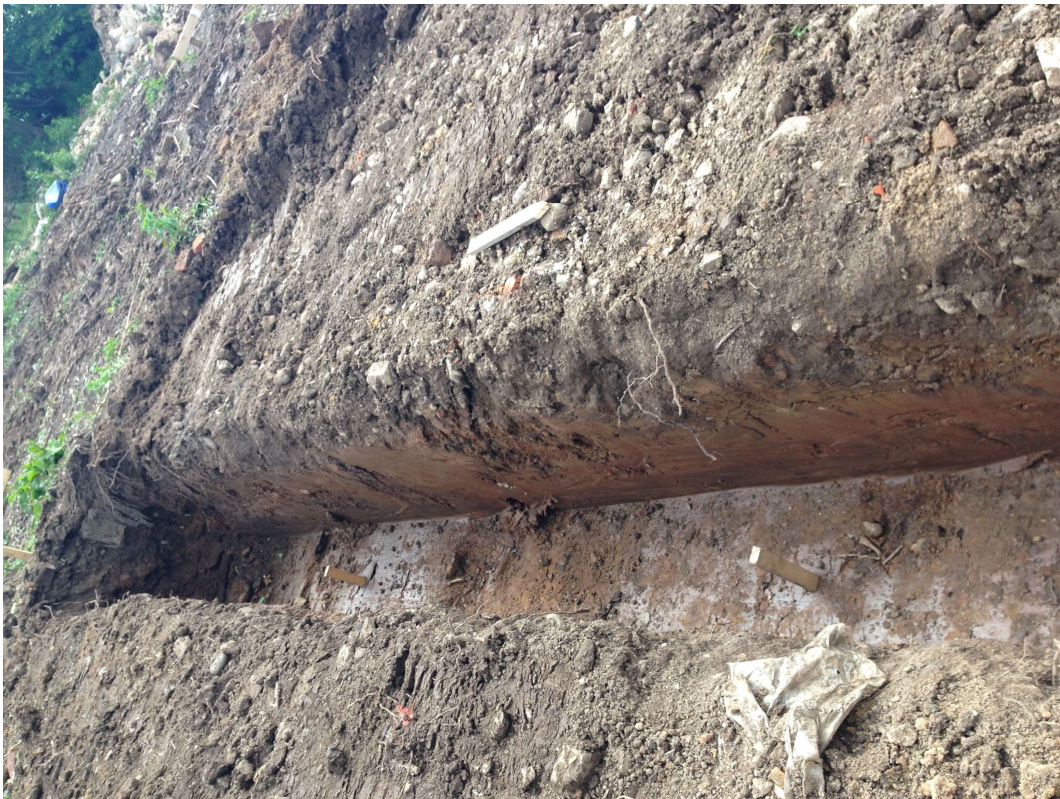
Plate 4. View of Foundation Trench. Facing South.
