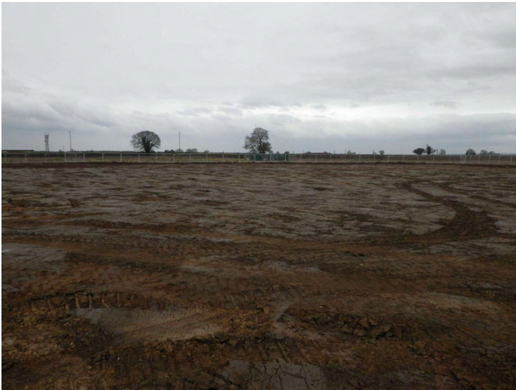
Plate 4. Site after Topsoil Strip. Facing West.
