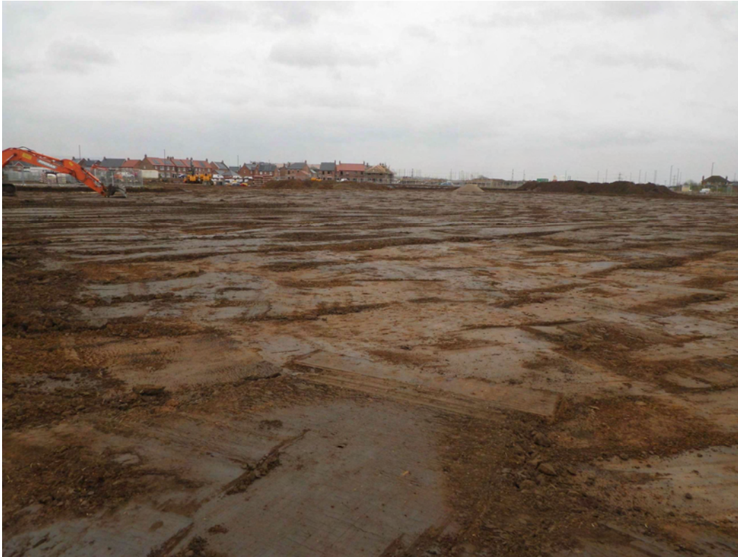
Plate 3. Site after Topsoil Strip. Facing East.
