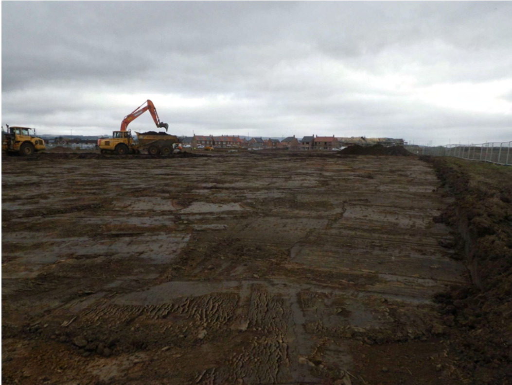
Plate 1. Site after Topsoil Strip. Facing East.
