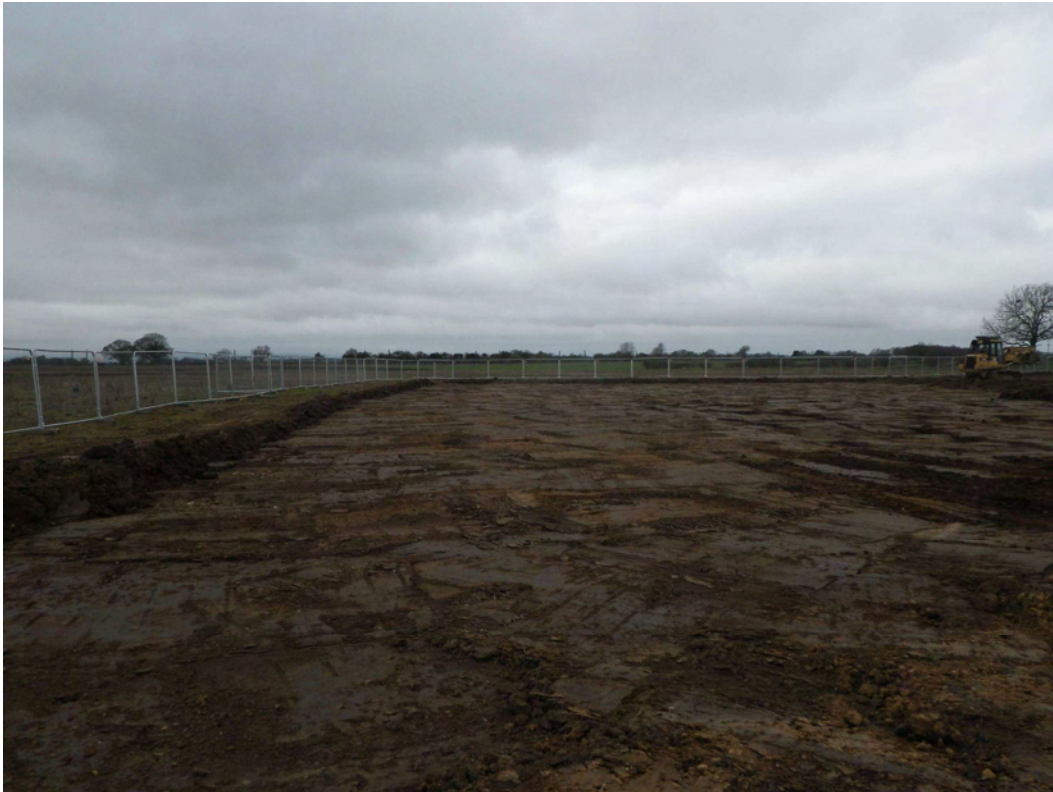
Plate 2. Site after Topsoil Strip. Facing West.
