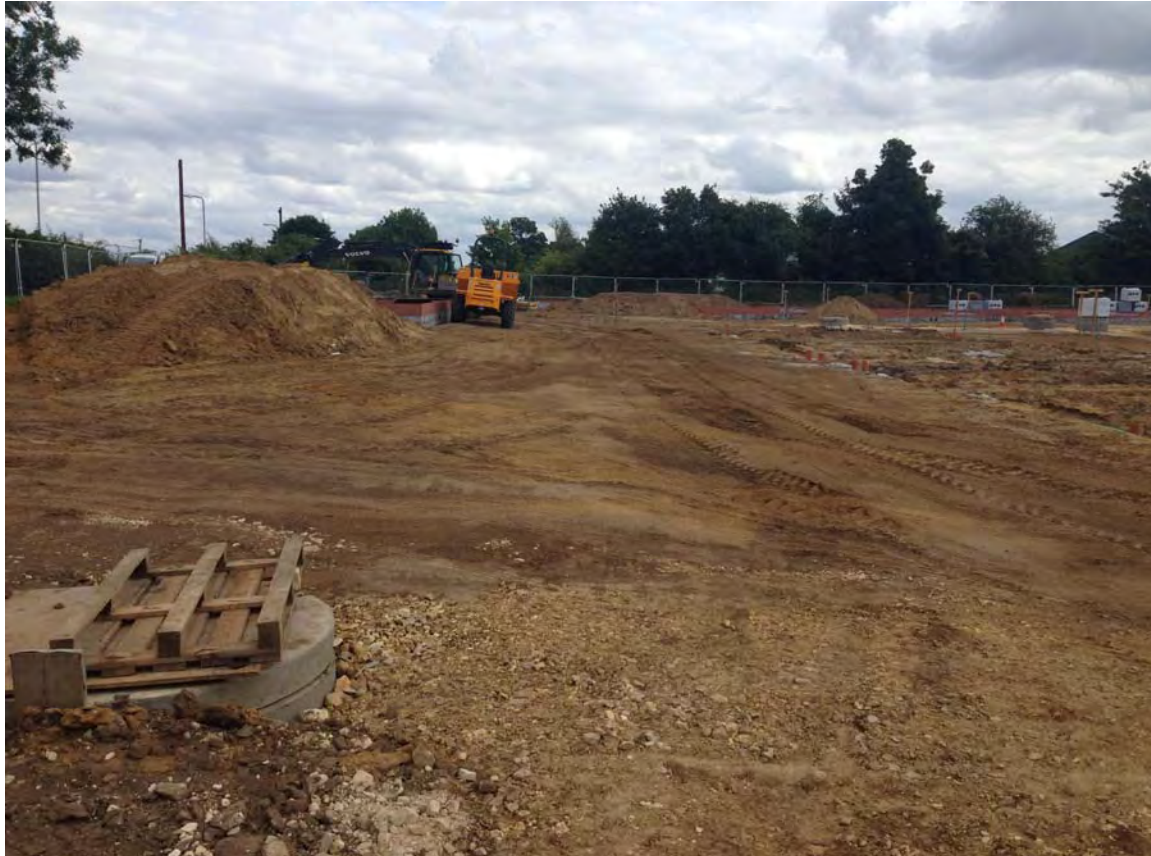
Plate 6. Foundations. Facing West.
