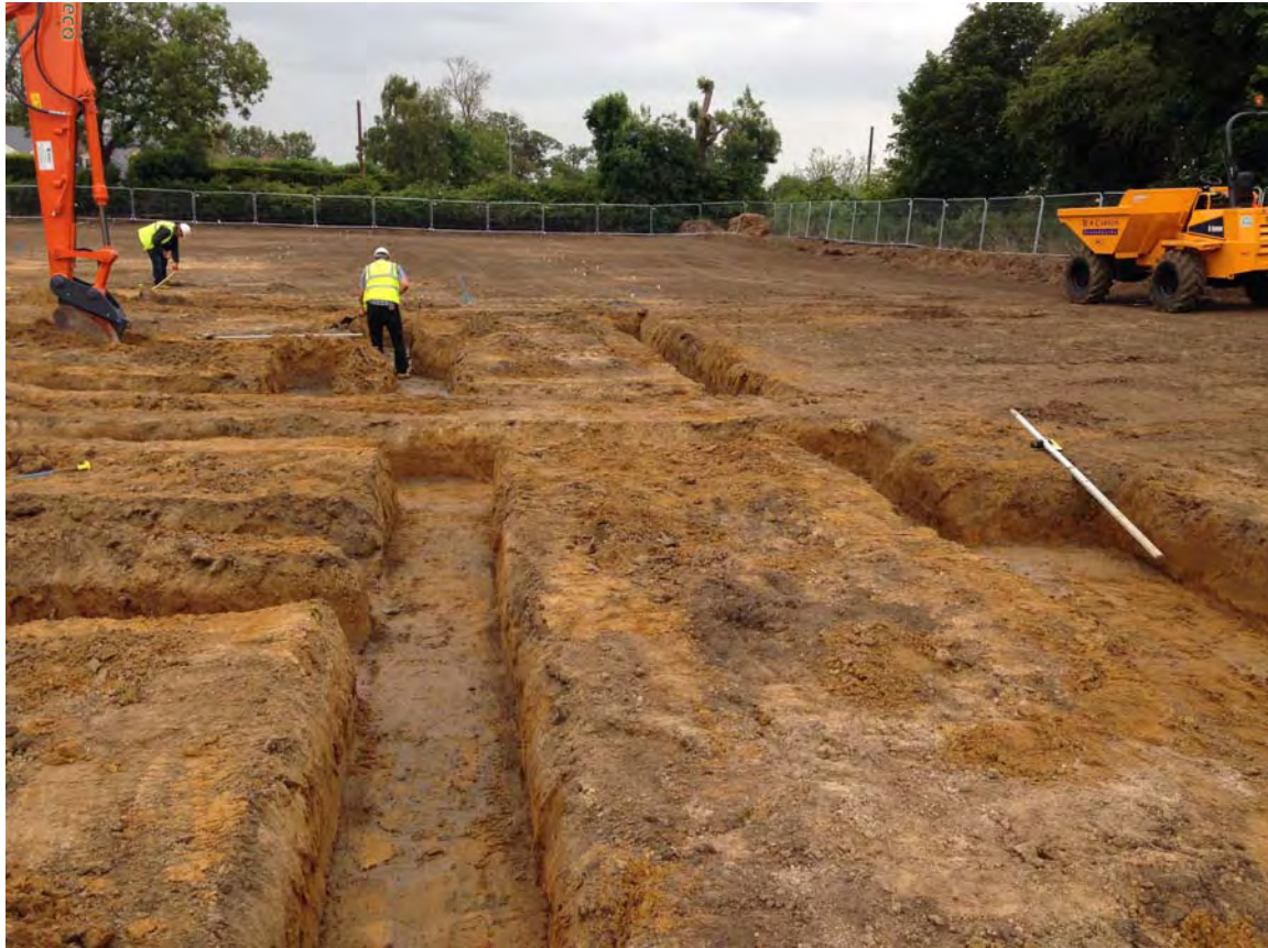
Plate 5. Foundations. Facing North.
