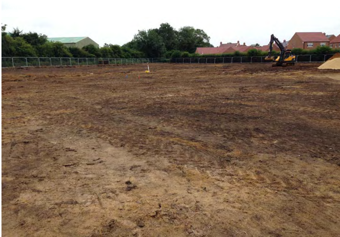
Plate 4. Area after Topsoil Strip. Facing South-west.
