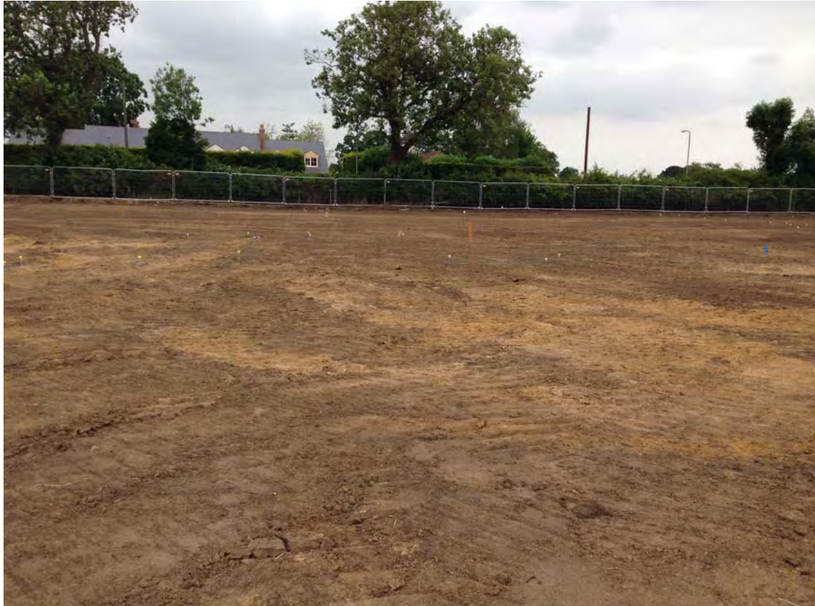
Plate 2. Area after Topsoil Strip. Facing North.
