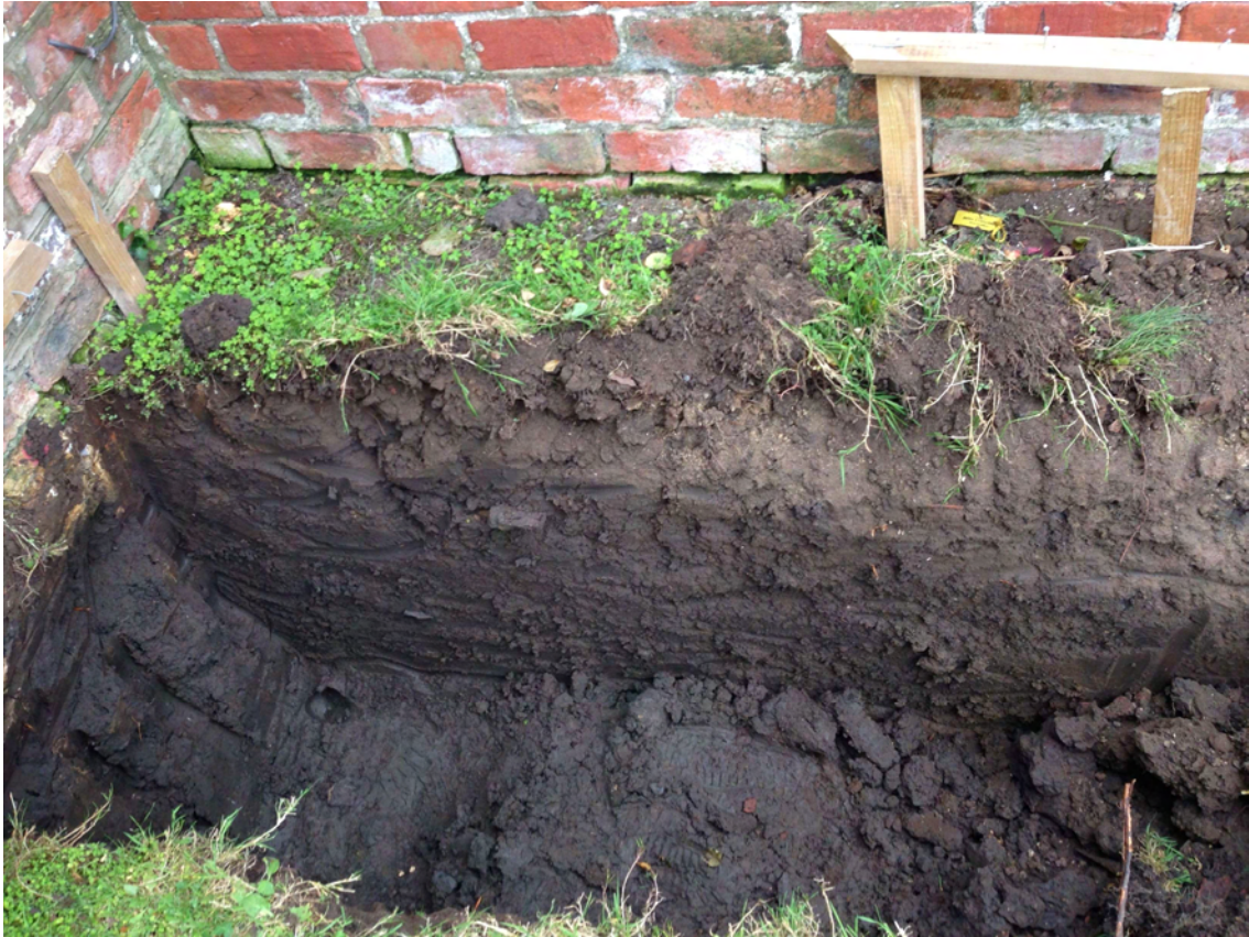
Plate 1. Foundation Trench. Facing East.
