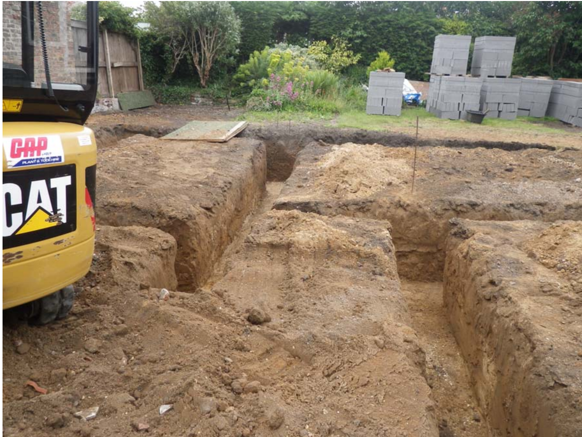
Plate 3. View of Strip Foundation Trench. Facing South.
