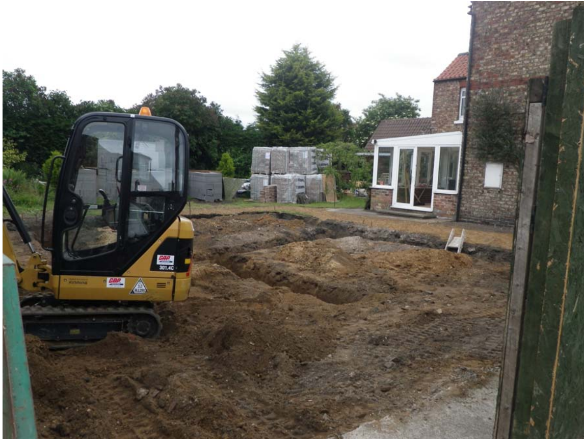
Plate 1. View of Building Plot. Facing South-west.
