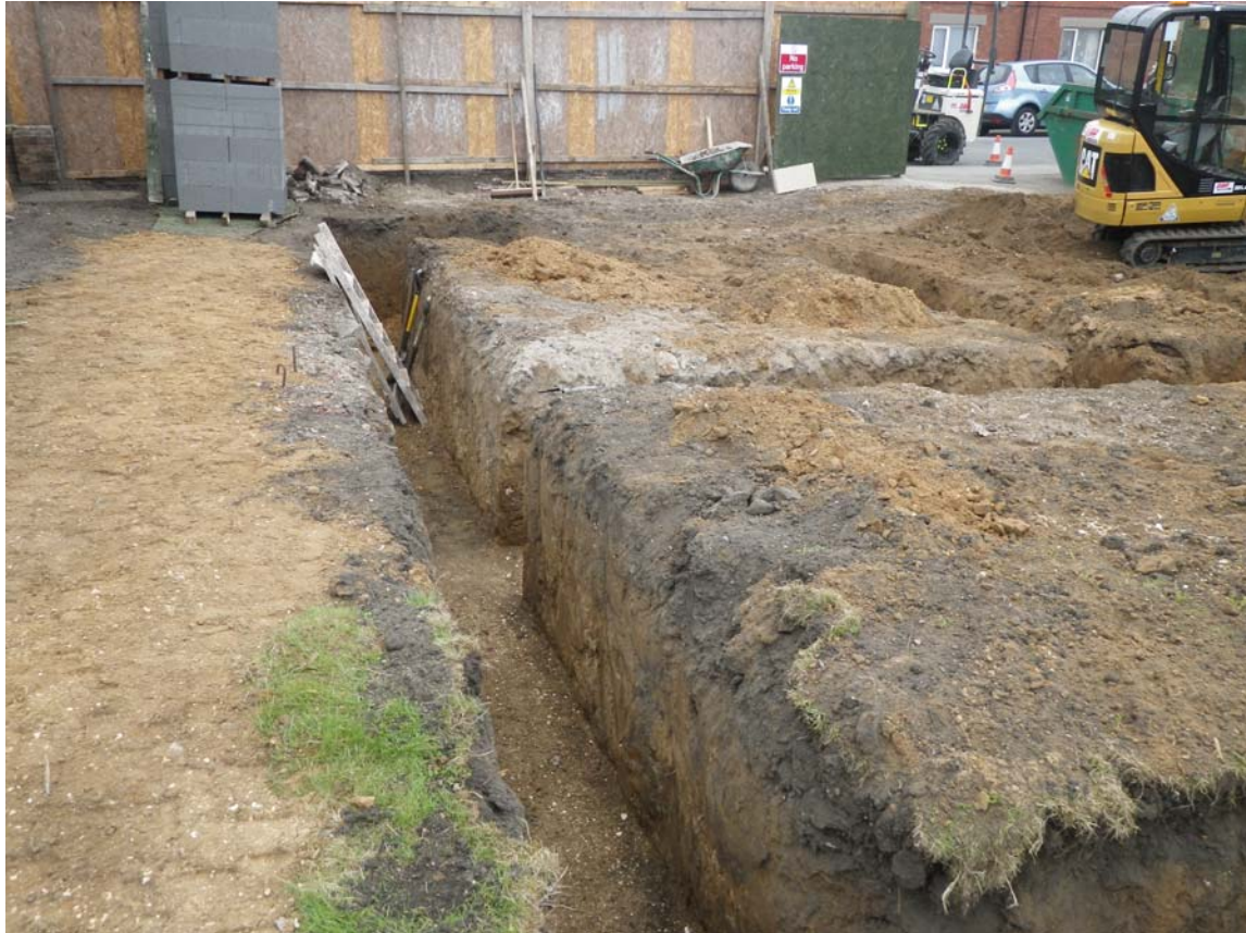
Plate 2. View of Strip Foundation Trench. Facing North.
