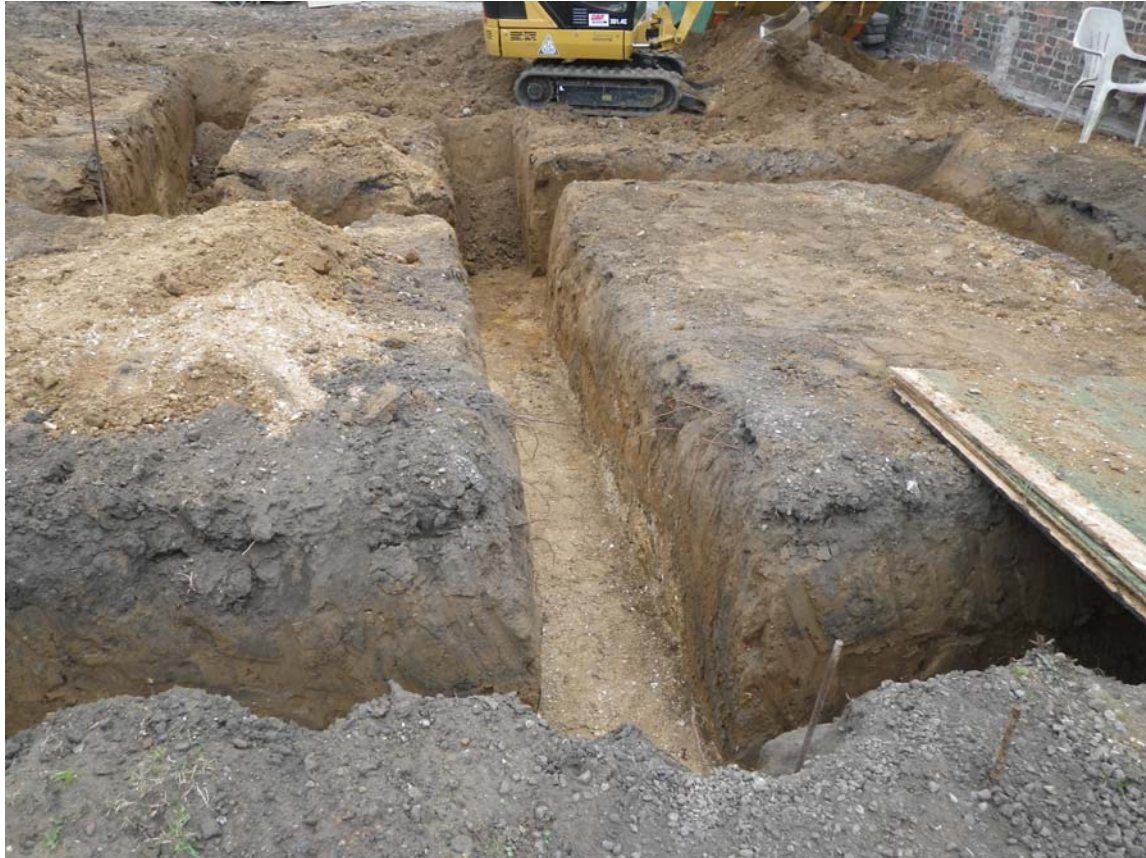
Plate 4. View of Strip Foundation Trench. Facing North.
