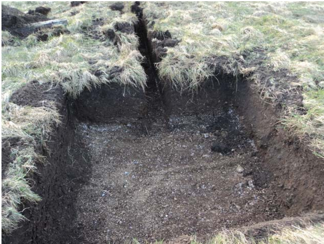
Plate 6. Soakaway & Water Pipe Trench. Facing South-west.
