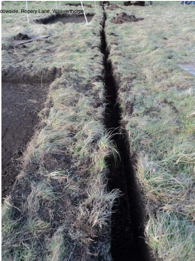
Plate 5. Water Pipe Trench. Facing North-west.
