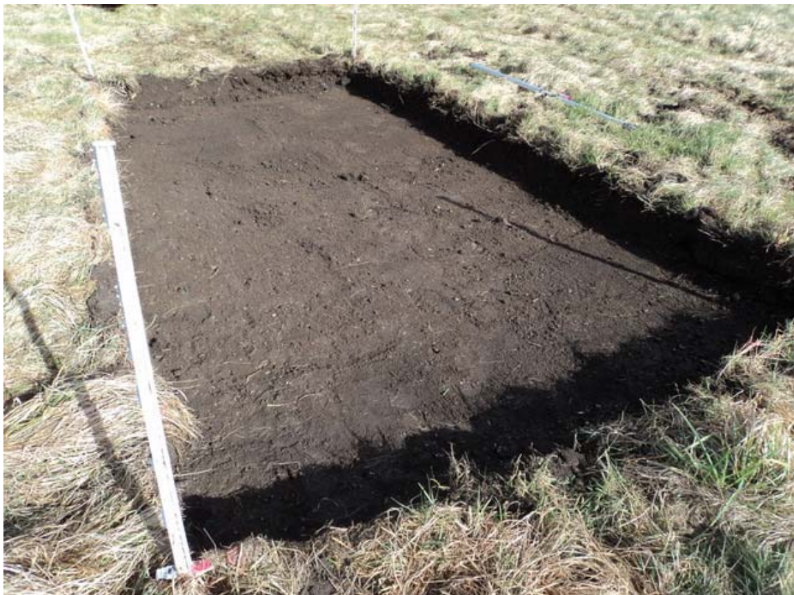
Plate 2. Temporary Glamping Unit Base. Facing North-east.
