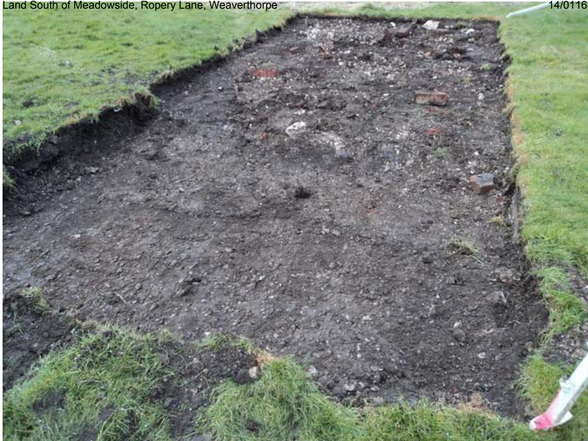
Plate 3. Temporary Glamping Unit Base. Facing West.
