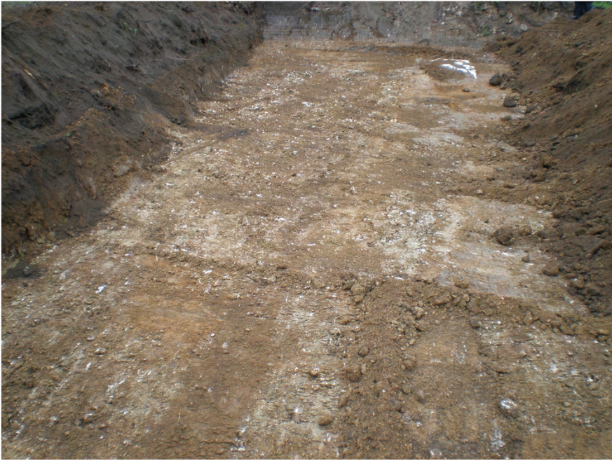
Plate 5. View of Stripped Area. Facing North.
