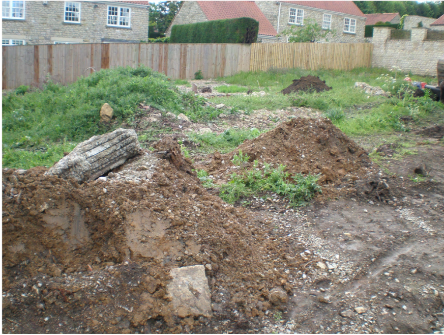
Plate 2. Site Prior to Clearance. Facing South-east.
