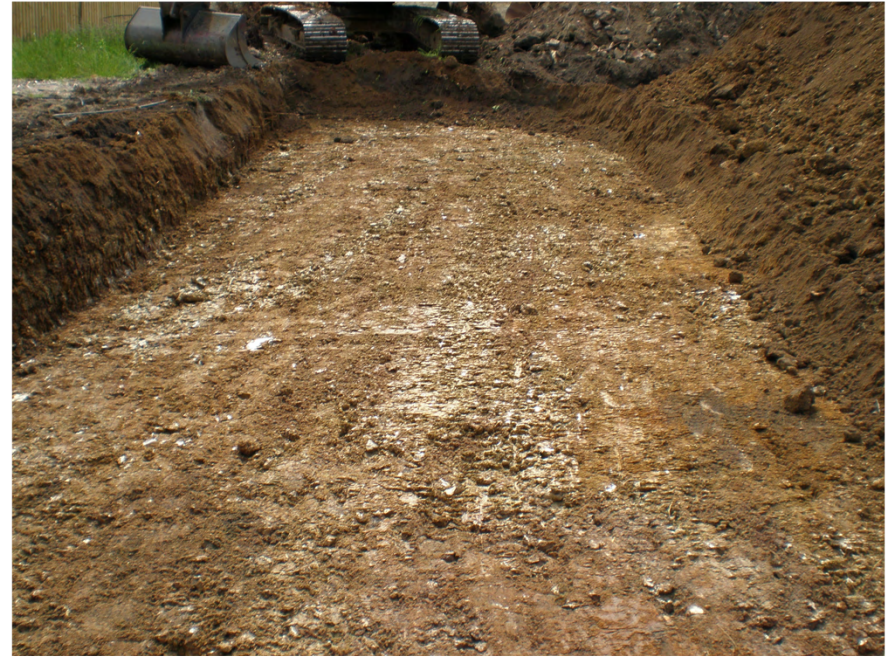
Plate 6. View of Stripped Area. Facing South.
