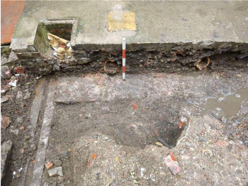
Plate 2. Foundation for new Raft. Facing East.
