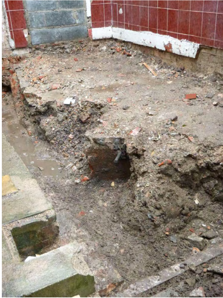
Plate 1. General View of Site of Raft. Facing South West.
