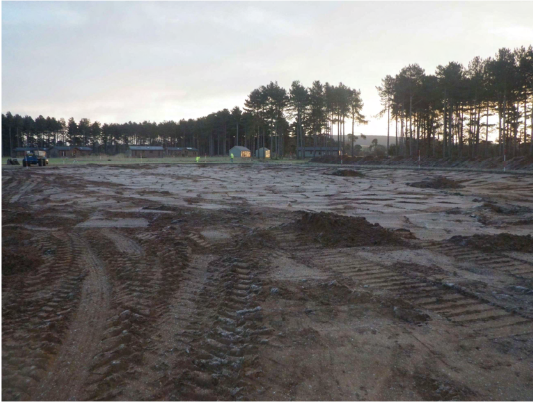
Plate 3. Phase 2 Pond during stripping. Facing South-east.
