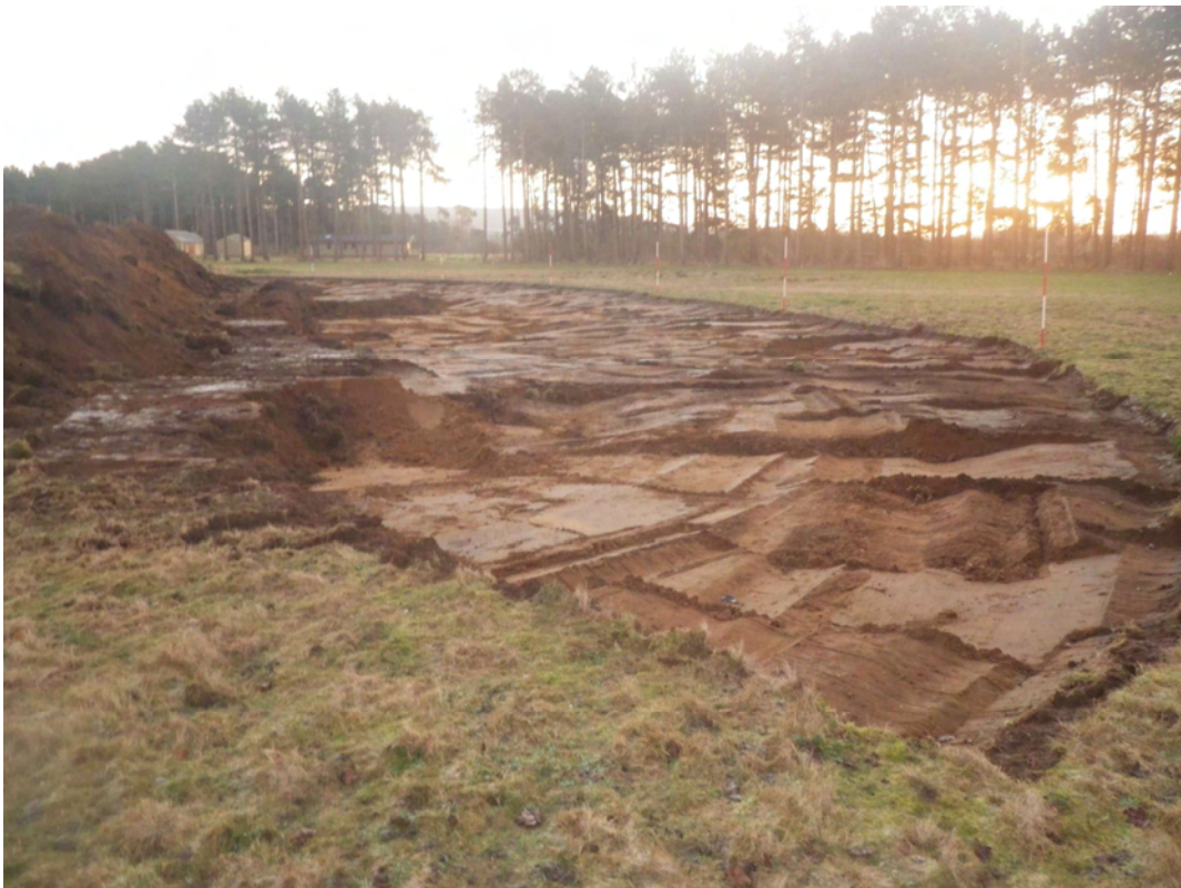
Plate 2. Phase 2 Pond during stripping. Facing East.
