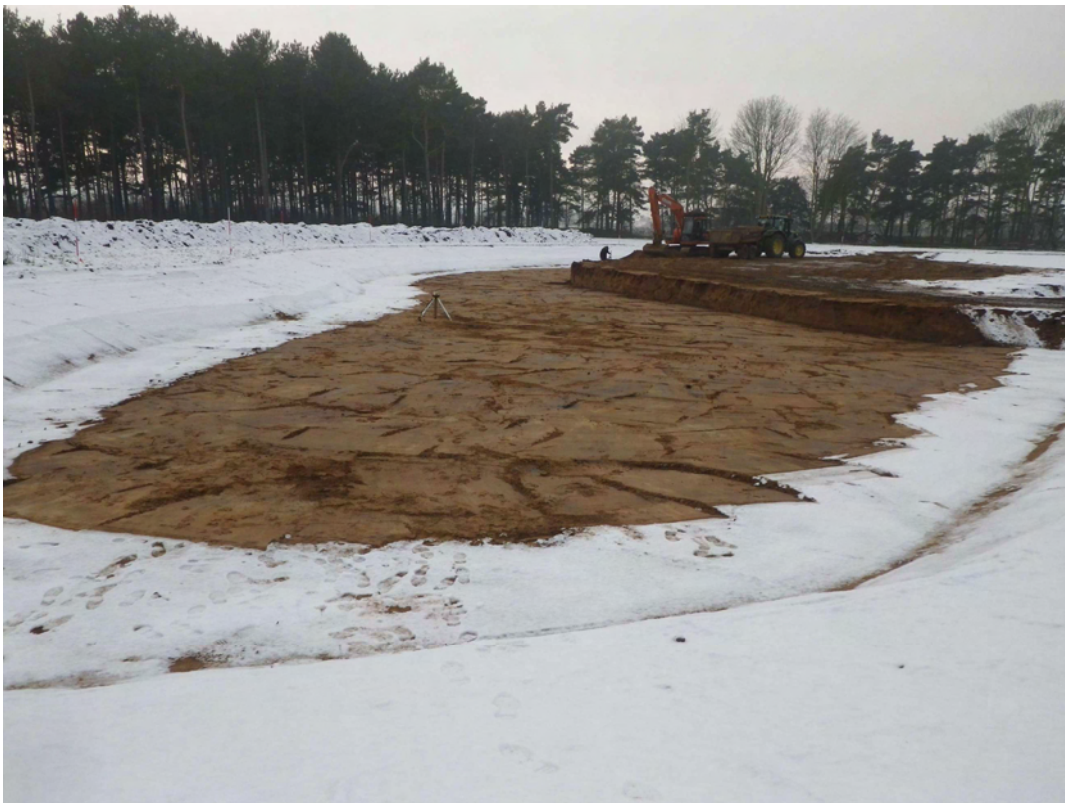
Plate 4. Phase 2 Pond after reduced level dig. Facing West.
