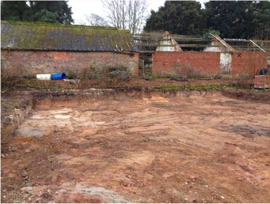
Plate 1. General View of Site.
