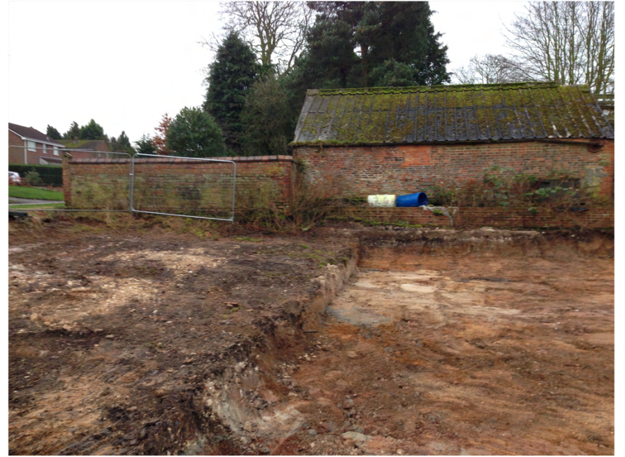
Plate 2. General View of Site.
