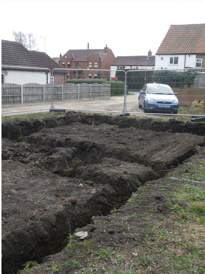
Plate 1. Foundation Trenches. Facing South.
