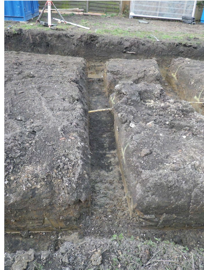
Plate 2. Foundation Trenches. Facing West.
