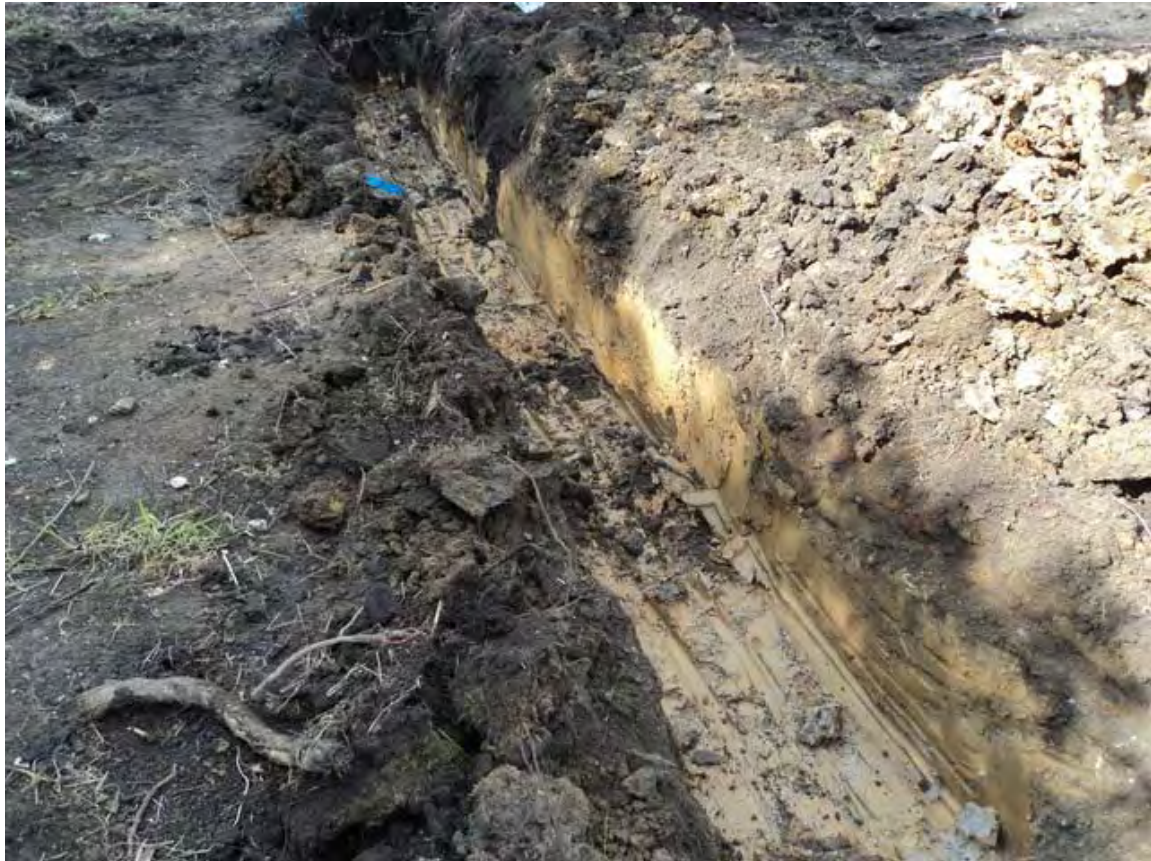
Plate 3. Western Foundation Trench. Facing North.
