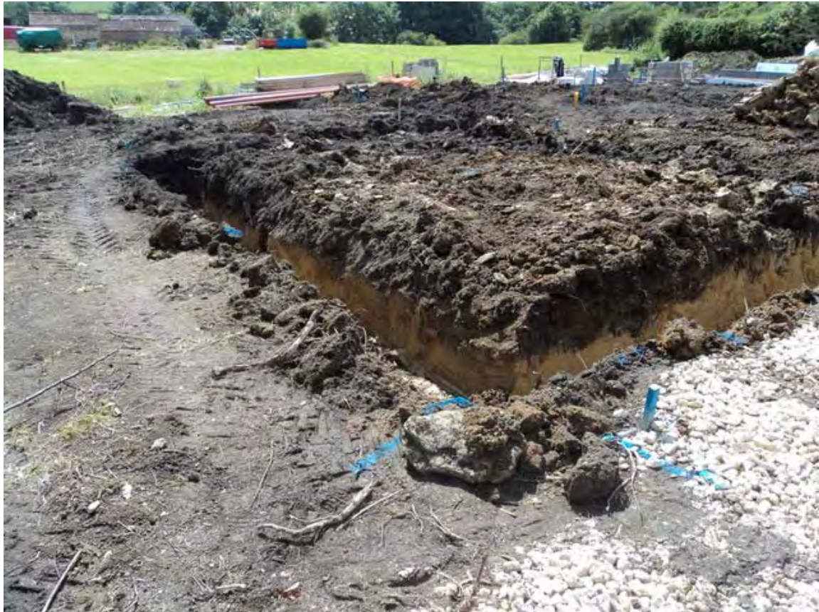
Plate 4. Overall View after Excavation. Facing South-west.
