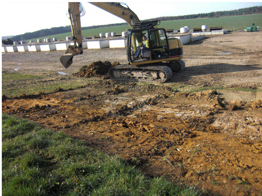
Plate 1. Area during Topsoil Strip. Facing South-west.
