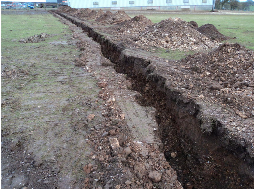
Plate 5. Cable Trench Route. Facing North-west.
