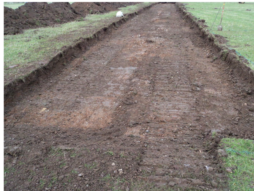
Plate 2. Access Track after Topsoil Strip. Facing North-west.
