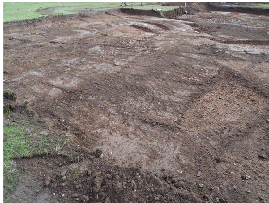
Plate 4. Crane Pad after Topsoil Strip. Facing South-east.
