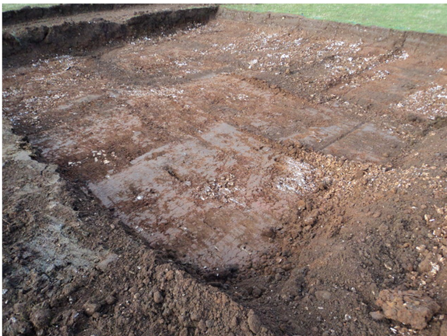
Plate 3. Wind Turbine Base after Topsoil Strip. Facing West.
