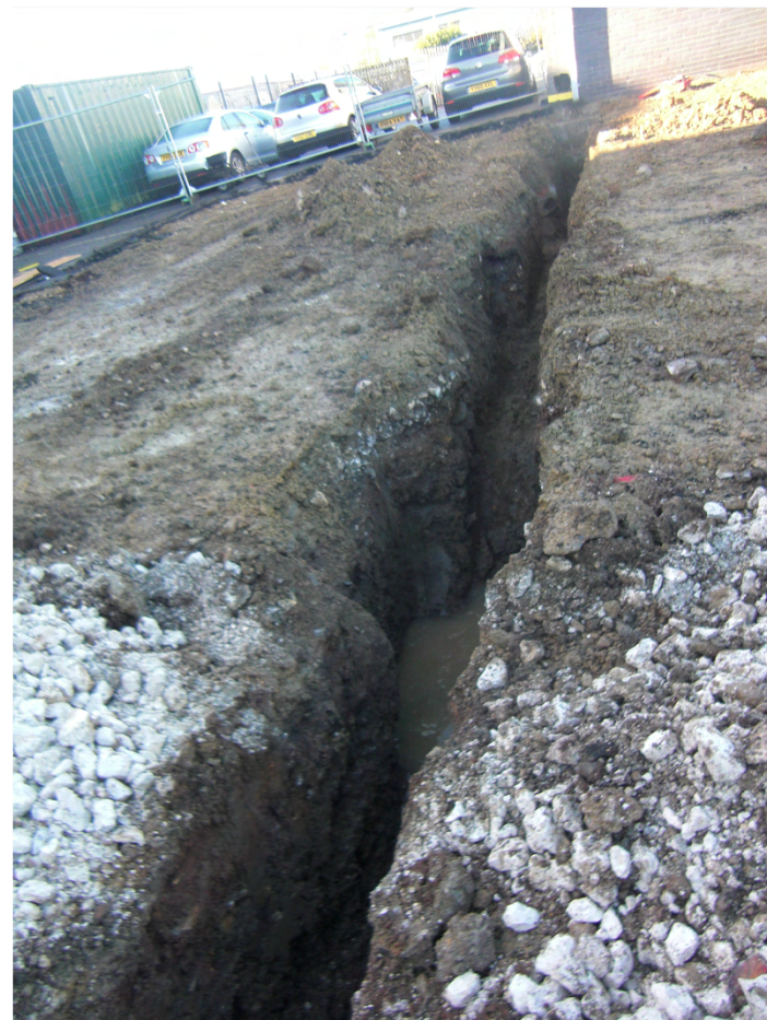
Plate 4. View of Foundation Trench. Facing West.
