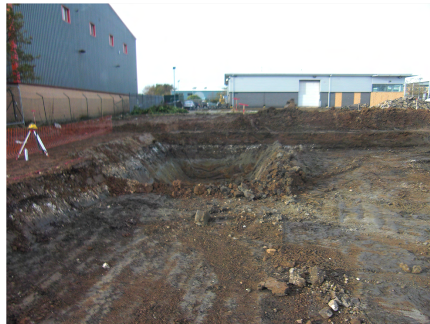
Plate 2. View of Site during excavation of Tank. Facing West.
